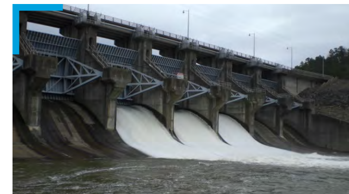
Broken Bow and Hugo Lake Closure Structure Study and Design – Broken Bow and Hugo, Oklahoma
