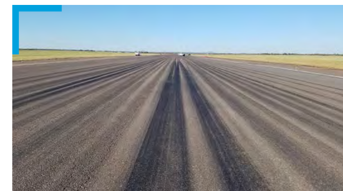
Repair Assault Landing Zone (ALZ) Runway 175/355 Altus AFB, Oklahoma
