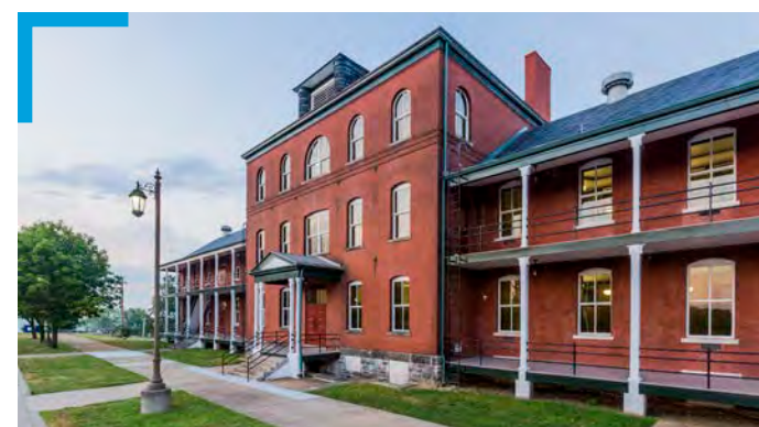
Repair/Renovate Building 29 Jefferson Barracks ANG, Missouri
