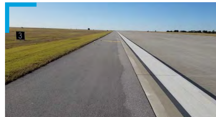
Repair Outside Runway and Taxiways Vance AFB, Oklahoma
