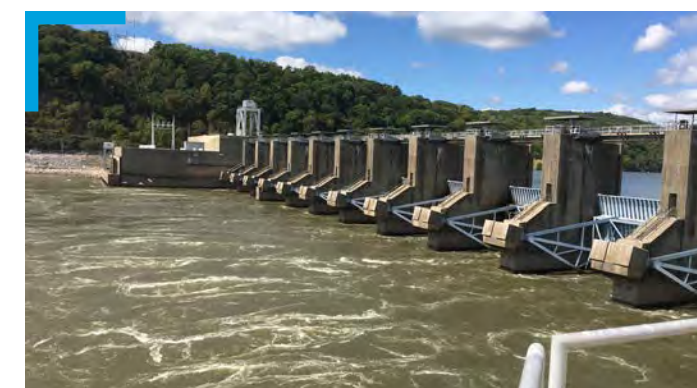
Webbers Falls Lock and Dam Repair of Scour Holes Tulsa, Oklahoma
