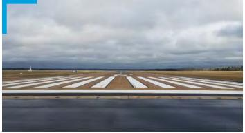
Reconstruct Runway 13L/31R Columbus AFB, Mississippi Reconstruction of 8,000-foot long by 150-foot wide runway 13L/31R with a combination of concrete and asphalt surfaces
