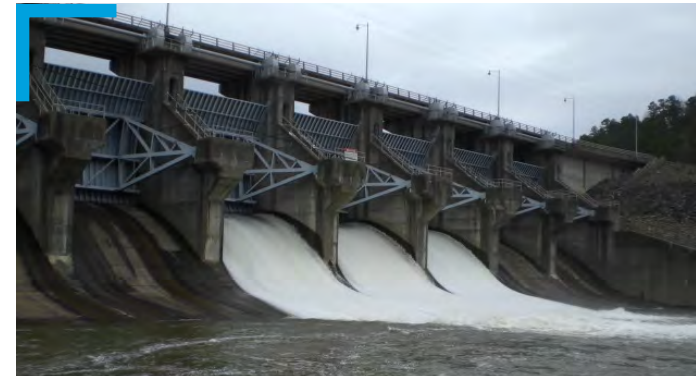
Broken Bow and Hugo Lake Closure Structure Study and Design – Broken Bow and Hugo, Oklahoma Feasibility study of multiple temporary gate closures resulting in design of a single segmental bulkhead system for both lakes
