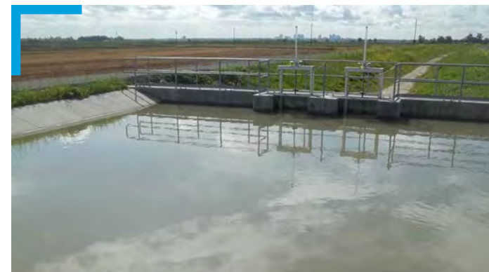
Riverside Canal and Pipeline Relocation Sacramento, California Relocation of Riverside Canal, including pump stations and borrow sites for levee construction
