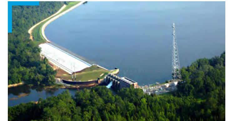
Jackson Bluff Dam Safety Tallahassee, Florida High hazard dam consisting of decommissioned powerhouse, tainter gate spillway, auxiliary spillway and an earthen embankment
