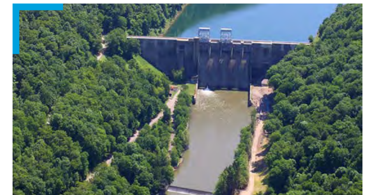
Mahoning Creek Hydroelectric Project New Bethlehem, Pennsylvania Six-megawatt hydroelectric development at Mahoning Creek Dam which went online five days prior to federally required deadline
