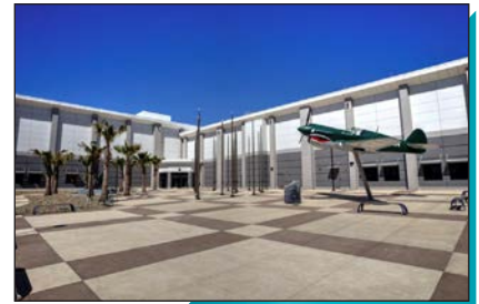
Renovate/Remodel Joint Space Operations Center (JSPOC)
