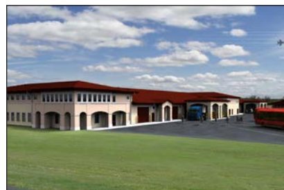
Renovate Deployment Facility Aviano AFB, Italy
