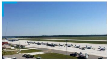
Repair Parking Apron A01B and A08B Alpena CRTC, Michigan Removal and replacement of the 350-FT by 2,400-FT concrete apron including 25-FT asphalt shoulders
