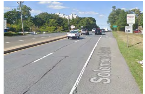
Figure 3: Existing Principal Arterial Roadway - MD 2 (Solomons Island)
