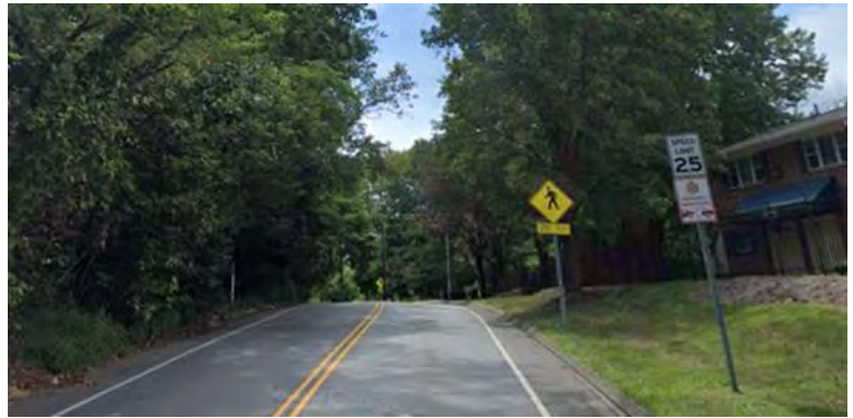
Figure 9: Existing Collector Roadway – Admiral Drive
