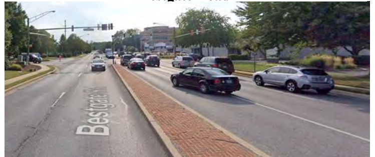
Figure 6: Existing Minor Arterial Roadway – Bestgate Road
