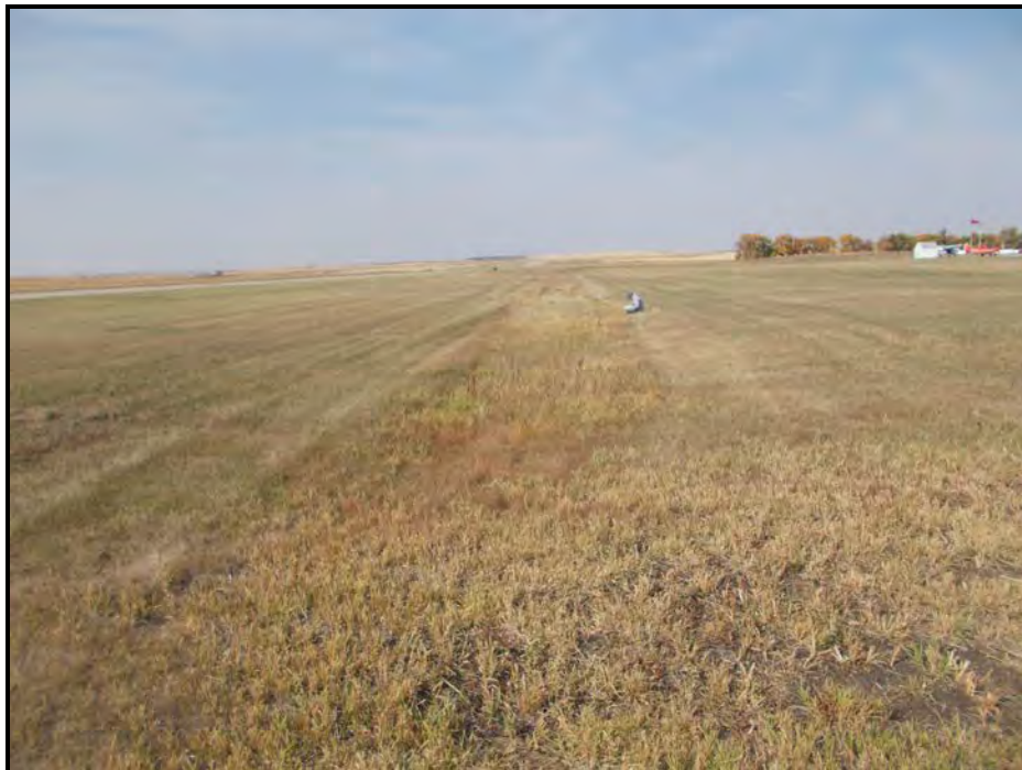
Photograph 4. View of Wetland 2b taken facing west. Wetlands 2a and 2b are slightly deeper areas of the Airport's storm water removal system. Storm water is conveyed to the west into a large culvert under the runway and then it flows south.
