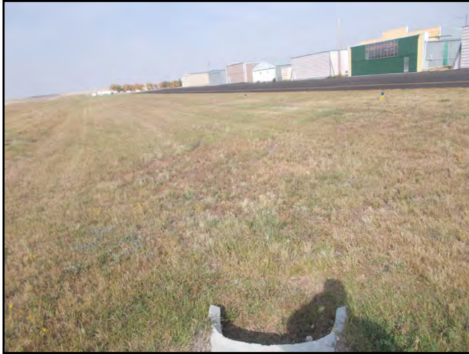
Photograph 3. View of Wetland 1c taken facing west. Wetland 1c is part of the storm water removal system and is a slightly deeper area at the lip of the culvert. The culvert connects to Ephemeral Drain 1b and flows water away from the Airport.
