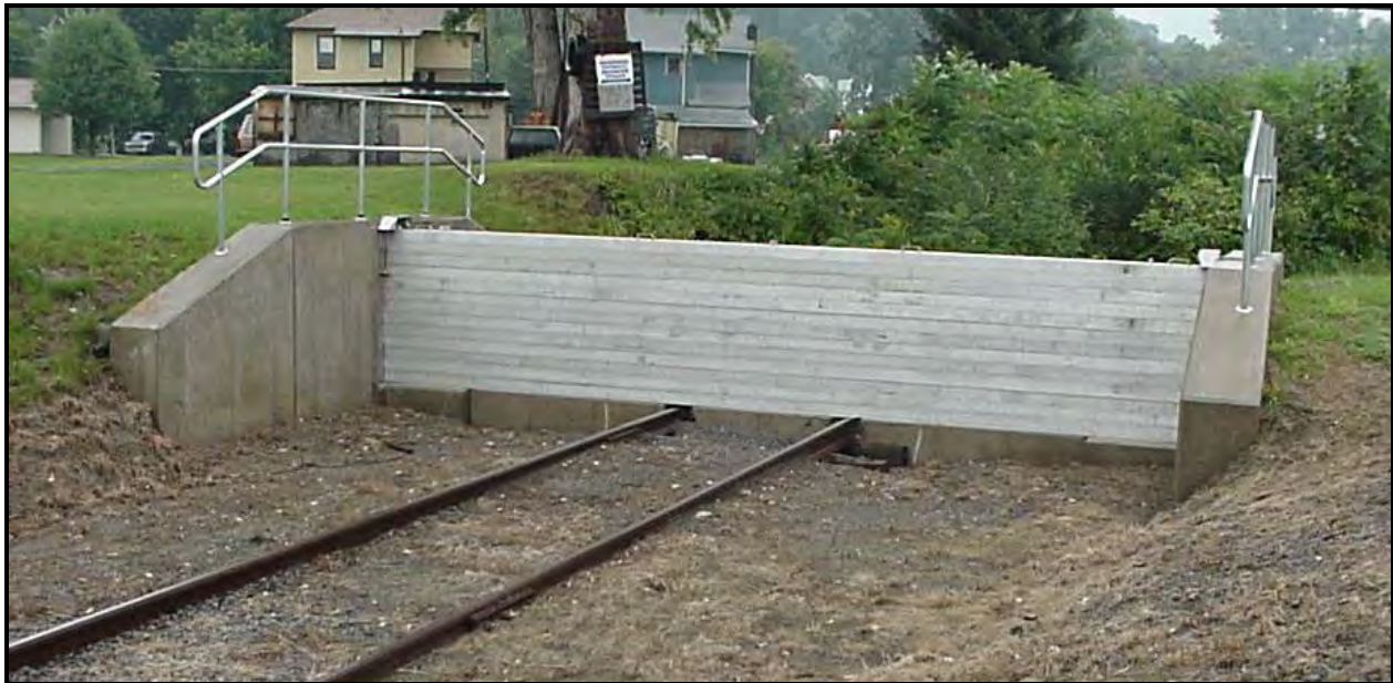
Figure 4.4: Example of Stoplog Closure Structure
