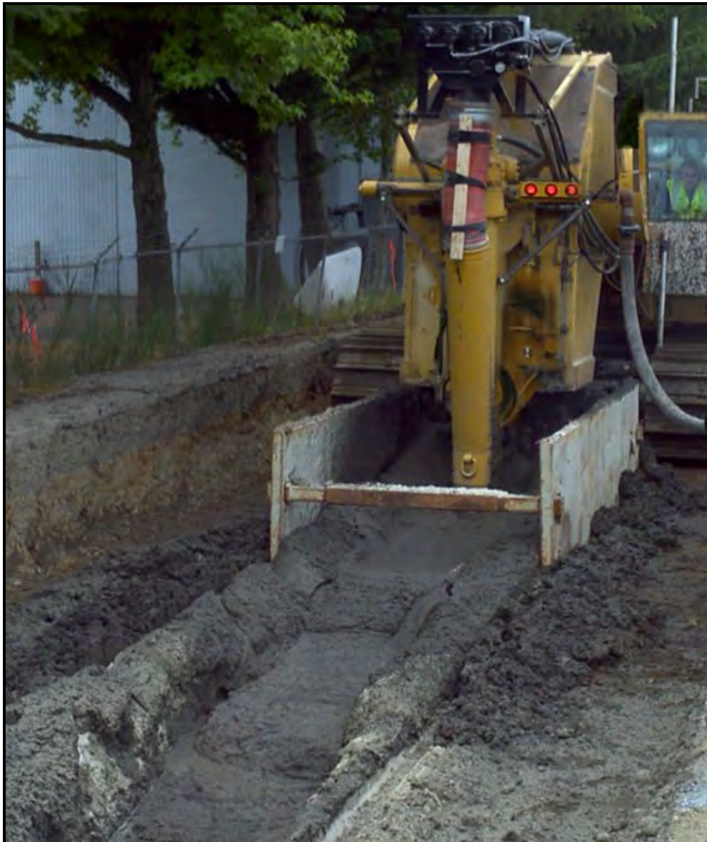
Figure 4.5: Slurry Wall under Construction
