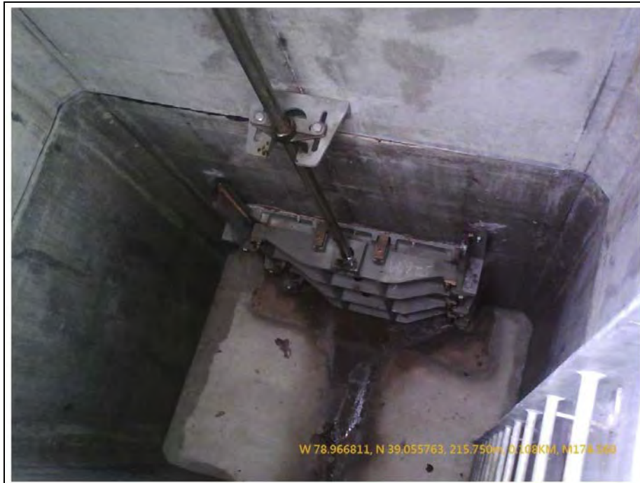
Figure 4.9: Typical Control Manhole with Sluice Gate
