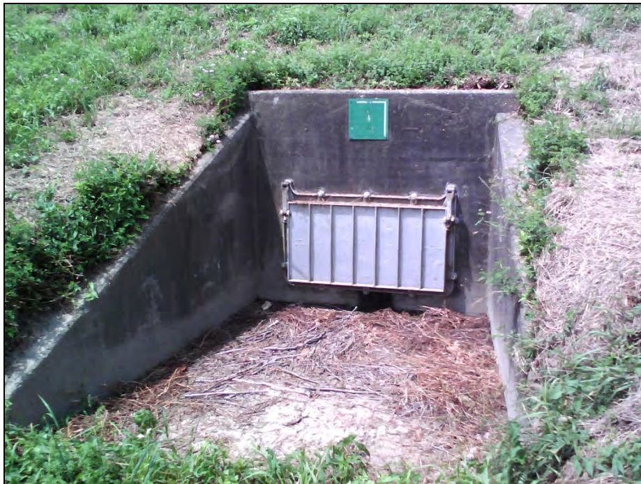
Figure 4.8: Typical Rectangular Flap-Gate on Headwall
