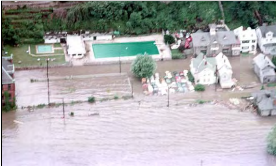
Figure 1.2: Flooding in Port Deposit from Agnes ( courtesy of cecildaily.com )
