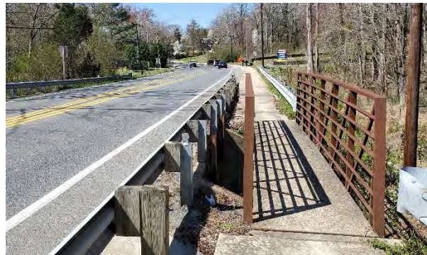
FIGURE 4. CHARLES ST FOOTBRIDGE OVER CLARK RUN
