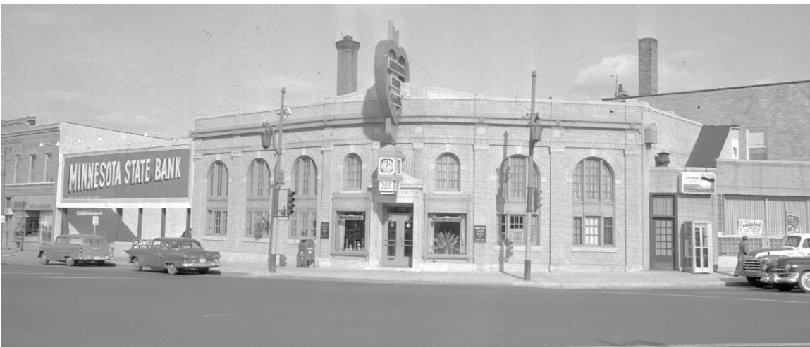
Figure 1. 1957 photograph of the Minnesota State Bank. Note the original windows openings and entrance. Courtesy of Minnesota Historical Society. 7
