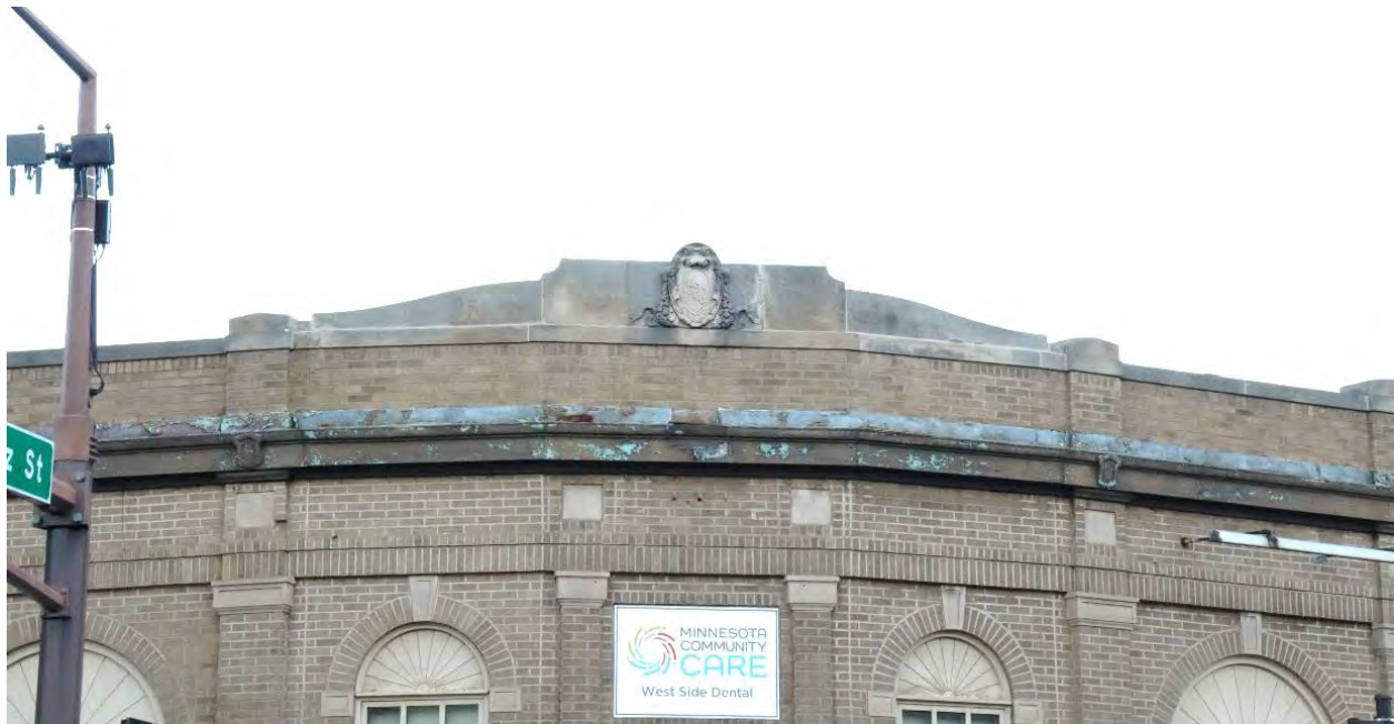
RA-SPC-03189, January 31, 2024, front (southeast) facade featuring parapet detail, view facing northwest.
