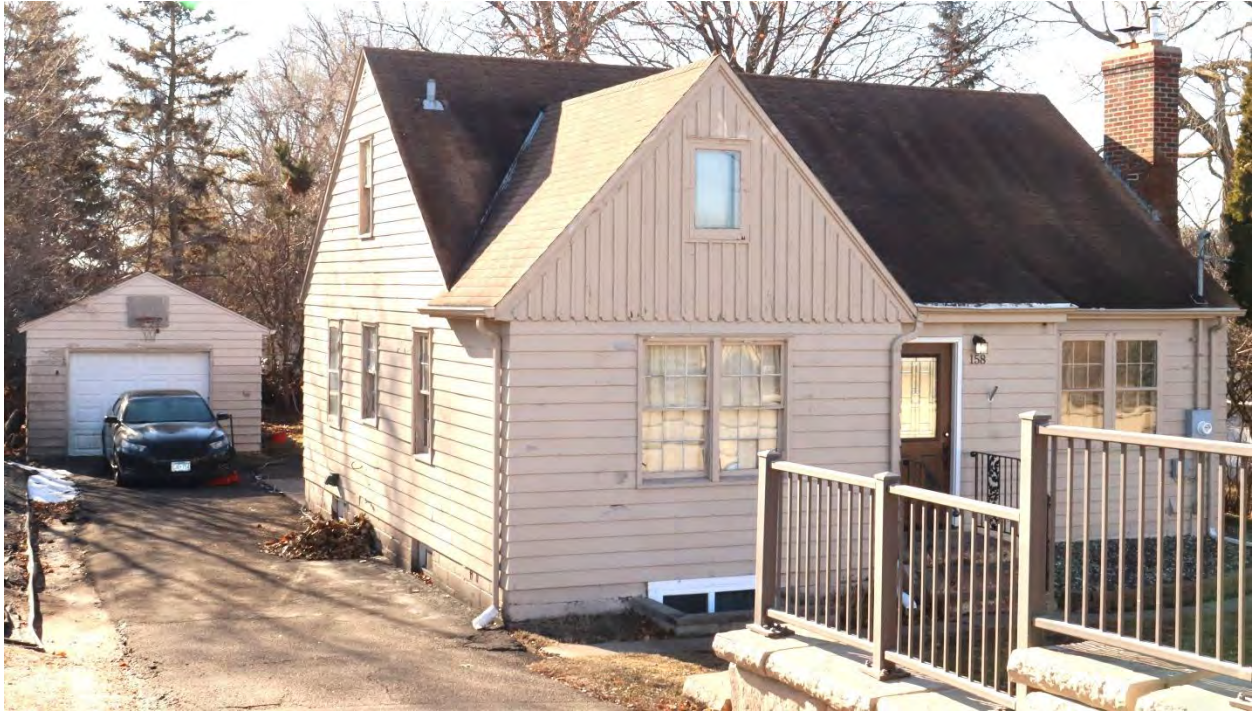
RA-RVC-00055, January 29, 2024, front (north) facade, side (east) elevation, and detached garage, view facing southwest.
