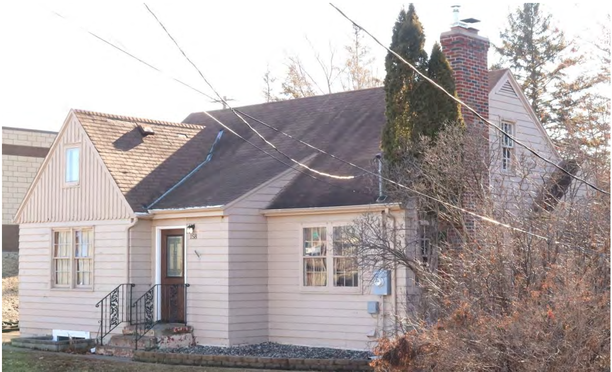
RA-RVC-00055, January 29, 2024, front (north) facade and side (west) elevation, view facing southeast.
