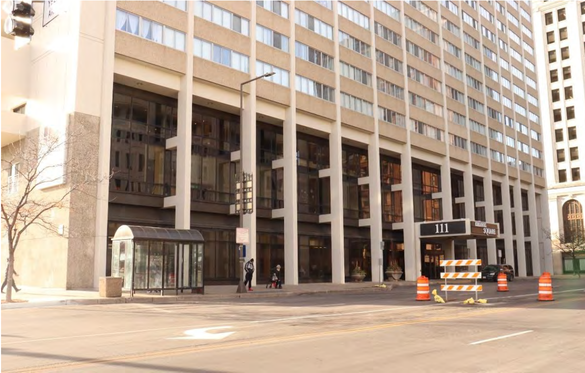
Figure 52. Kellogg Square Apartments, facing west from Robert Street North.
