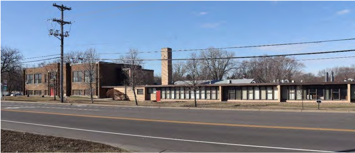
Figure 8. Overview of original 1935 North Heights School (left) with 1950s additions (center and right), facing southwest from Rice Street.
