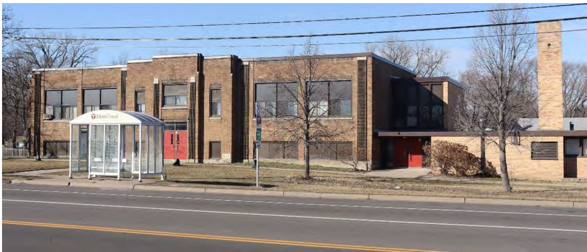
Figure 7. Original 1935 North Heights School with existing bus shelter (to be removed and relocated), facing west-southwest from Rice Street.
