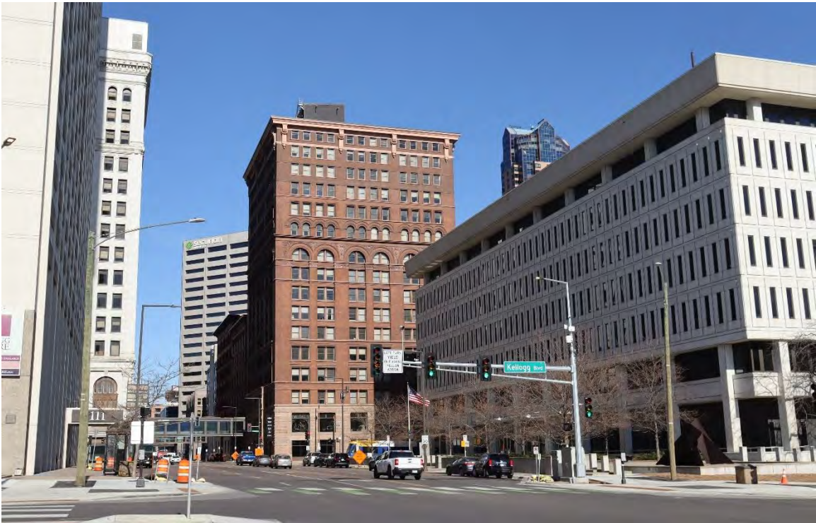
Figure 51. Warren E. Burger Federal Building and US Courthouse (right), facing northwest from Robert Street.
