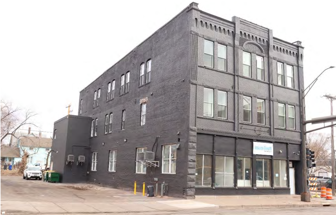
Figure 22. Side (north) elevation and front (west) facade of Arvidson Block, facing southeast from Rice Street.
