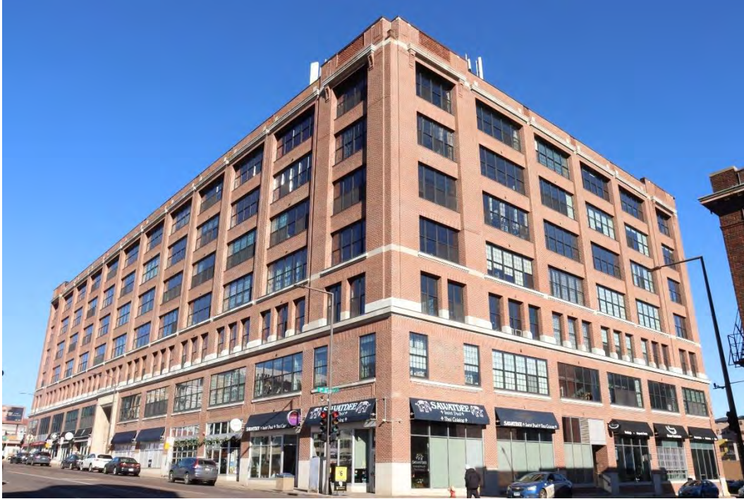
Figure 43. Front (southwest) facade and side (southeast) elevation of Foot, Schulze and Company Building, facing north from the intersection of Robert Street North and 9th Street East.
