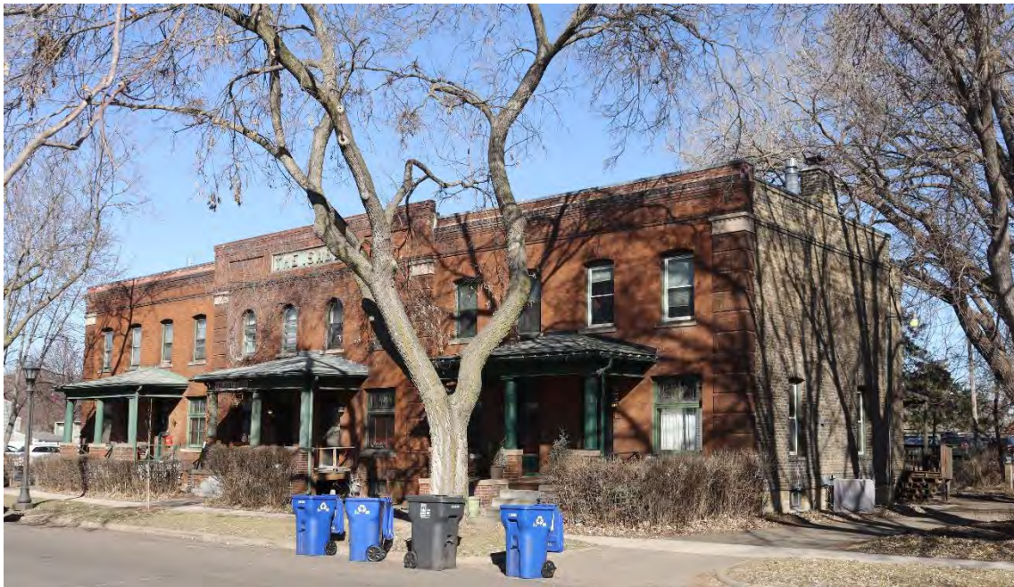
Figure 2. Front (south) facade and side (east) elevation, view toward northwest.
