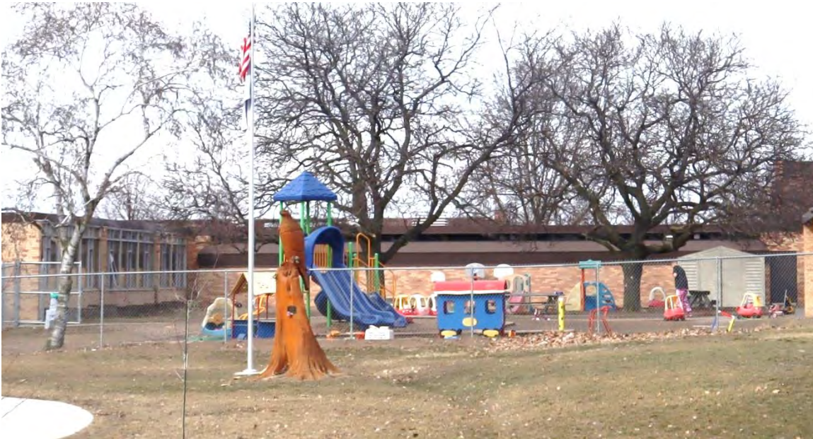
Figure 25. Obstructed view of side (south) elevation of 1973 library addition, view facing north.
