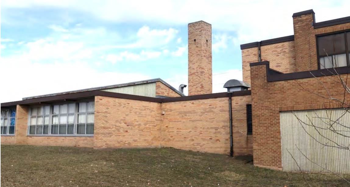
Figure 13. Rear (west) elevation of 1953 addition, view facing northeast.
