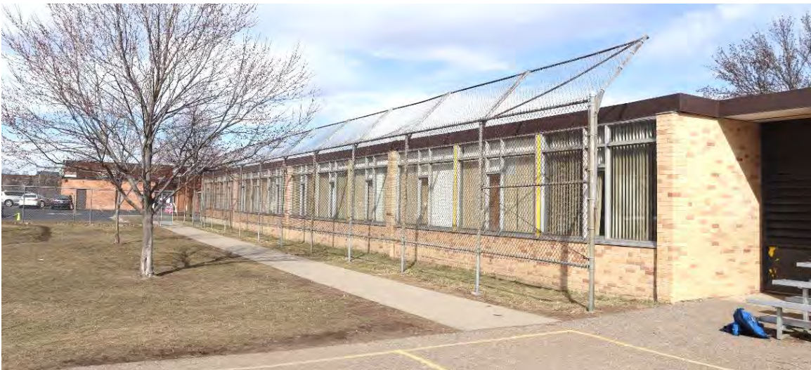
Figure 21. Rear (west) elevation of 1961 linear classroom addition, view facing northeast.
