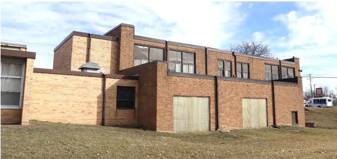
Figure 8. Rear (west) elevation of original 1935 North Heights School with portion of 1953 addition (left), view facing east-southeast.
