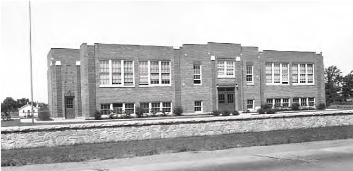
Figure 32. Undated photograph of the school shortly after completion in 1935. 28
