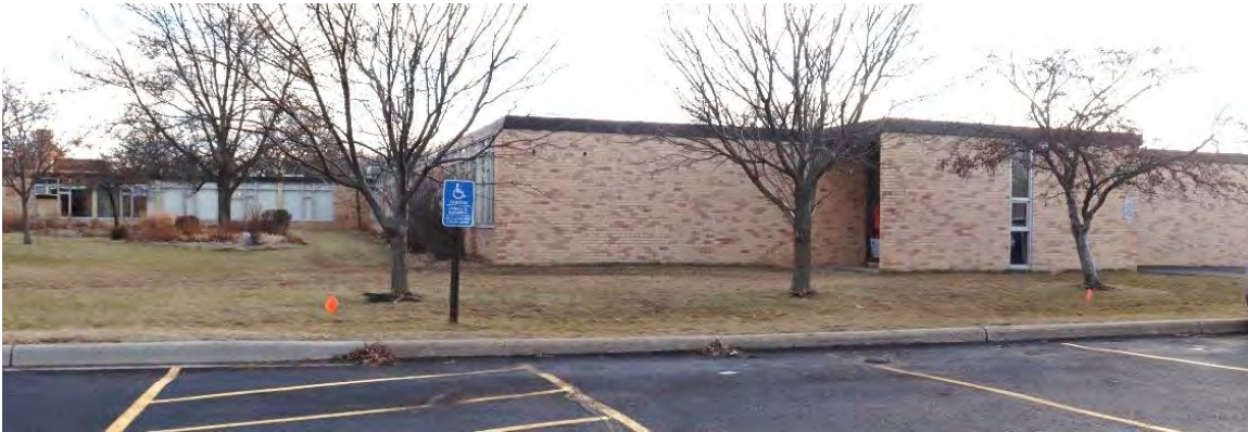
Figure 23. Side (north) elevation of 1961 linear classroom addition (right) and library hyphen addition (background left), view facing south.
