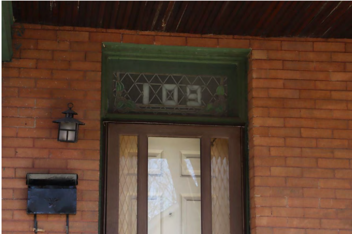
Figure 5. Detail view of stained-glass transom above an entrance door, view toward north.
