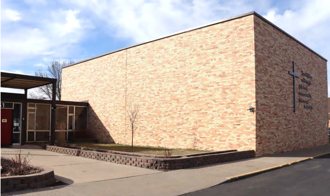
Figure 27. Side (south) elevation and front (east) facade of 1975 gymnasium addition, view facing northwest.
