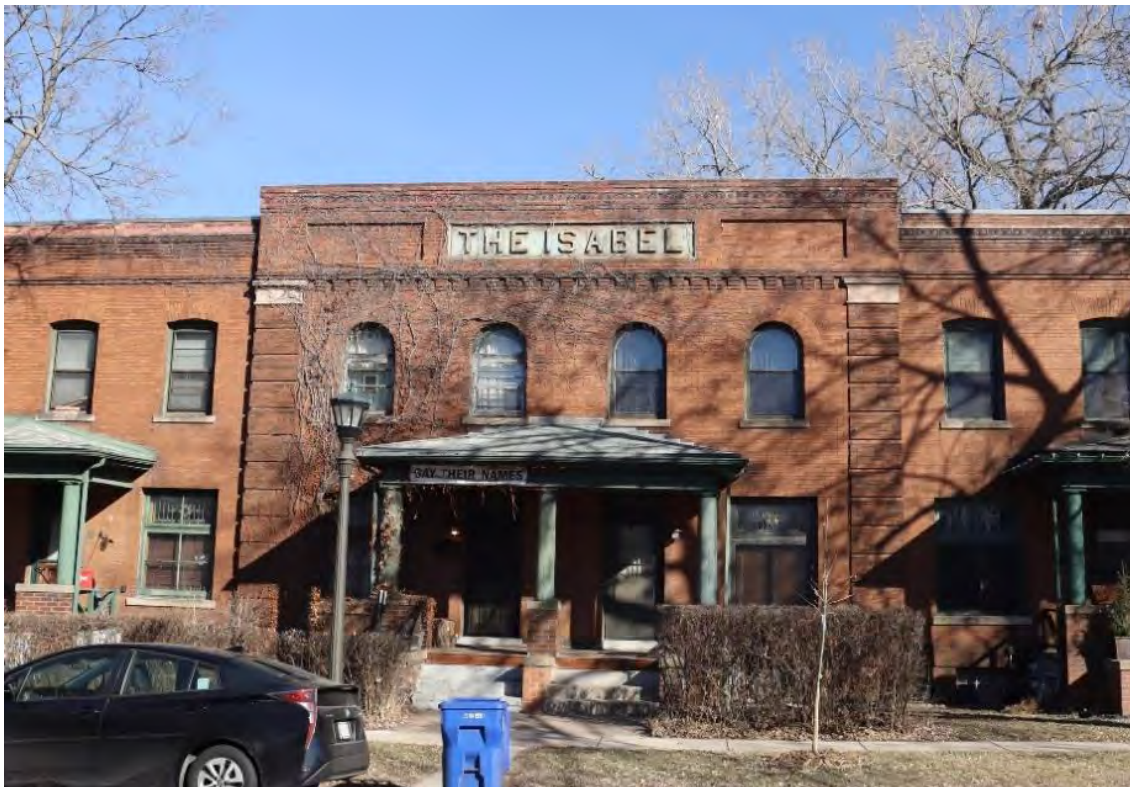
Figure 4. Front (south) facade, view toward north.
