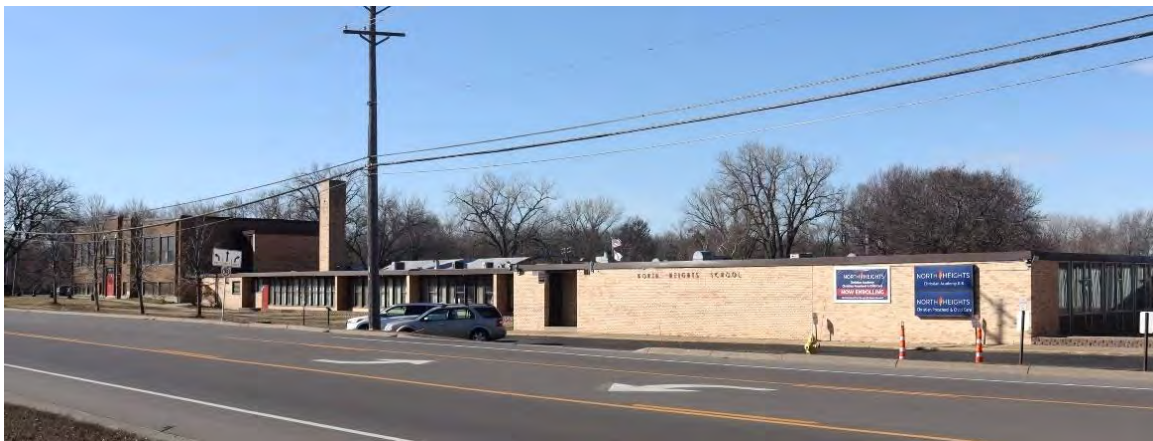
Figure 30. Original 1935 building (far left), 1953 addition (left), 1958 addition (center), and part of 1961 addition (right), view facing southwest.
