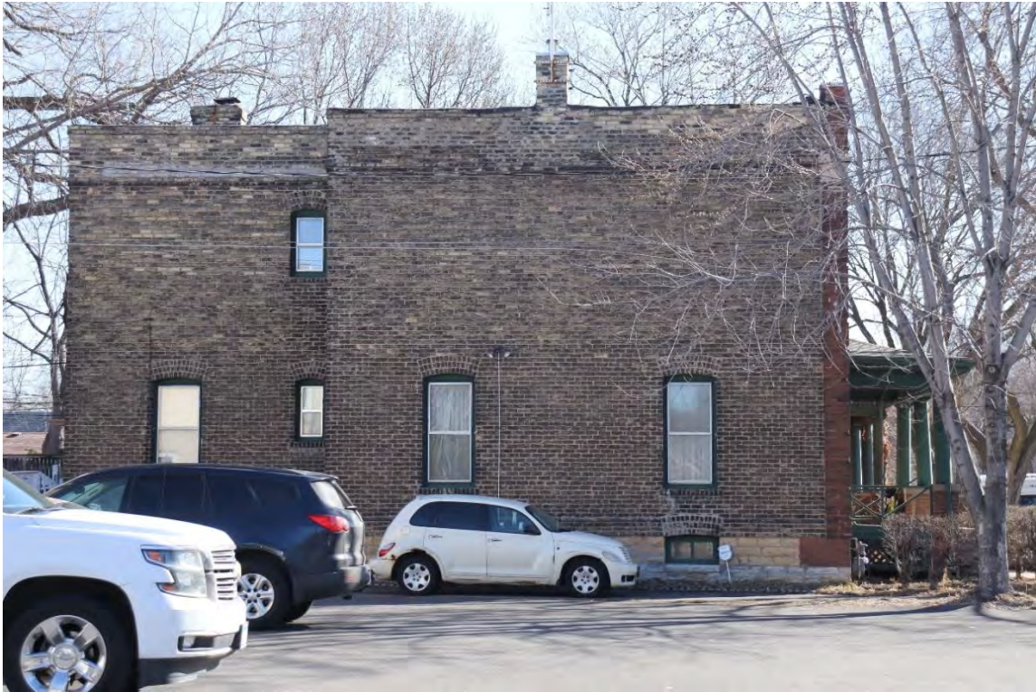
Figure 7. Side (west) elevation, view toward east.
