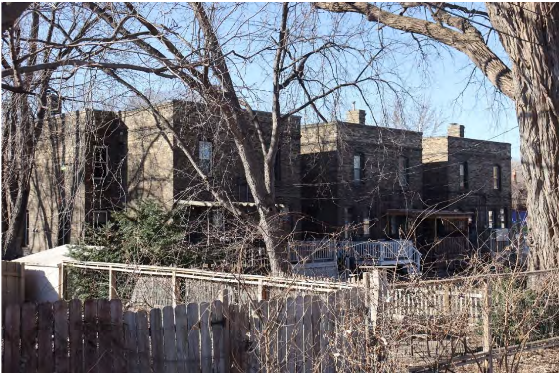
Figure 8. Rear (north) elevation and side (east) elevation, view toward southwest.
