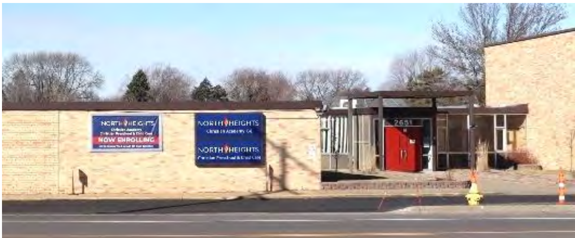
Figure 18. Facade of 1961 addition with cafeteria expansion (left) and new primary entrance, view facing west.
