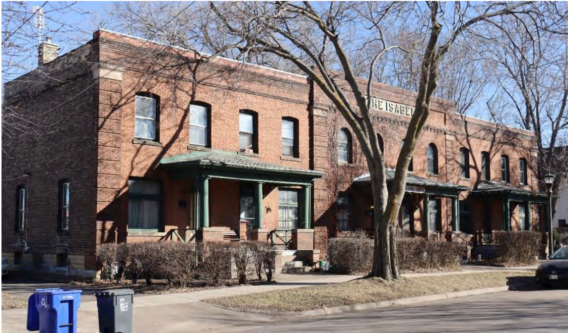
Figure 3. Front (south) facade and side (west) elevation, view toward northeast.
