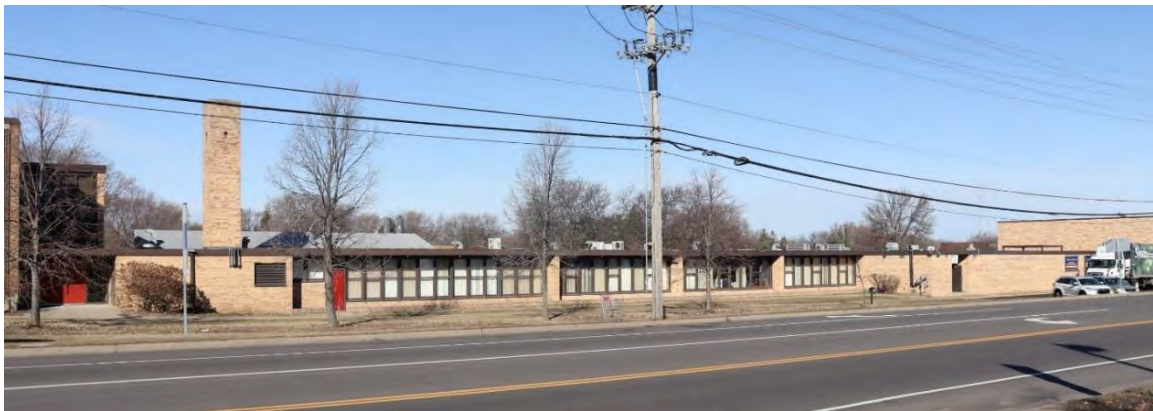
Figure 29. Facade of 1953 addition (left) and 1958 addition (right), view facing northwest.
