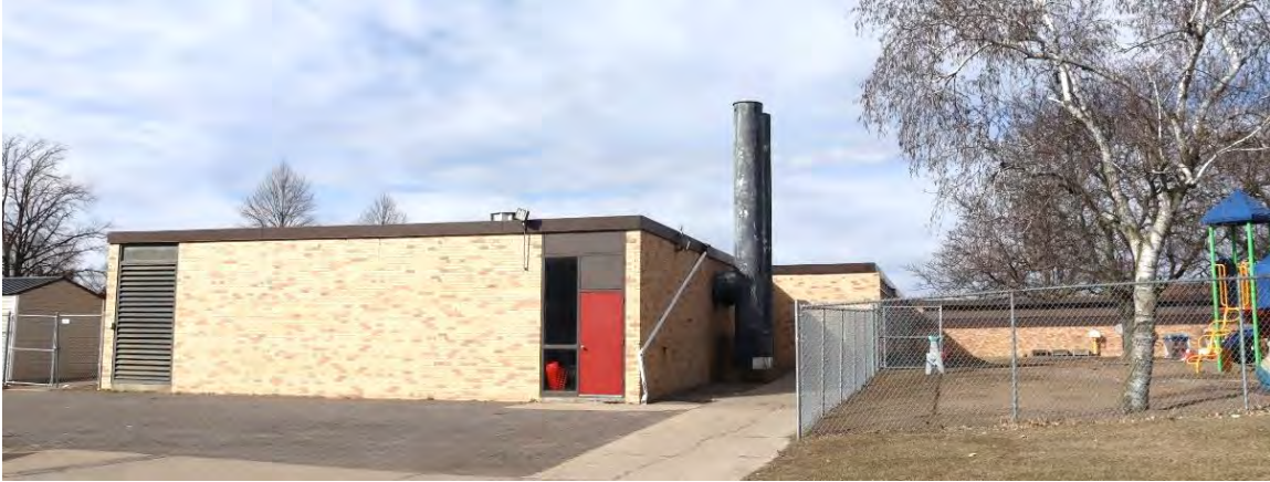
Figure 22. Side (south) elevations of 1961 linear classroom addition (left) and library hyphen addition (right), view facing north.
