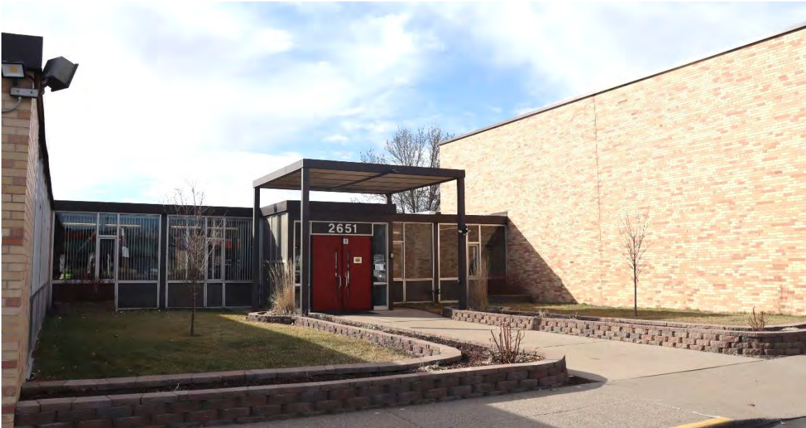
Figure 19. Facade of 1961 addition with new primary entrance, view facing west-northwest.
