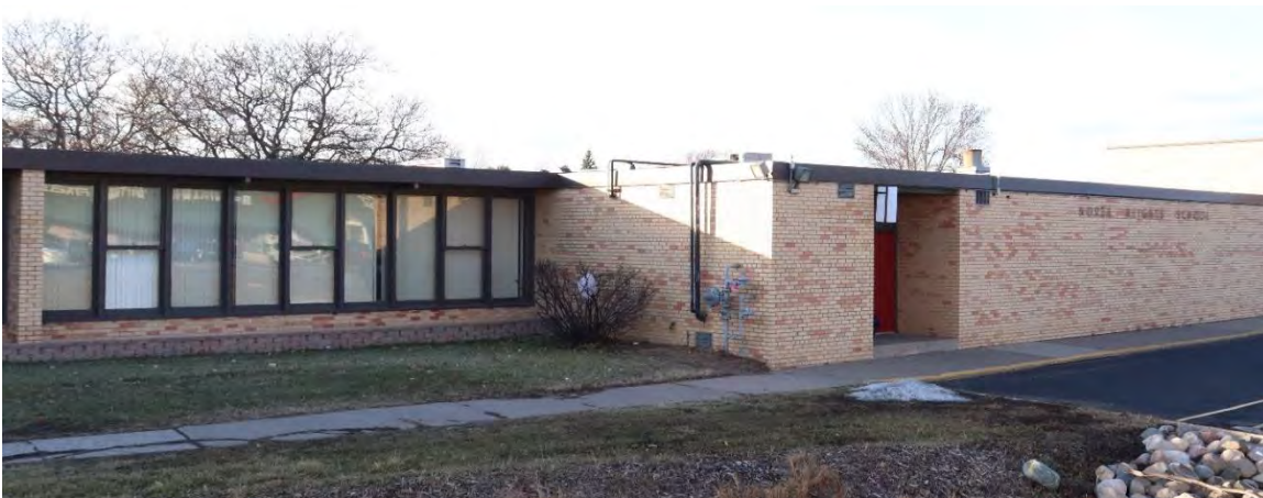
Figure 16. Detail of facade of 1958 addition, view facing northwest.
