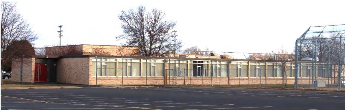
Figure 20. Side (north) and rear (west) elevations of 1961 linear classroom addition, view facing southeast.
