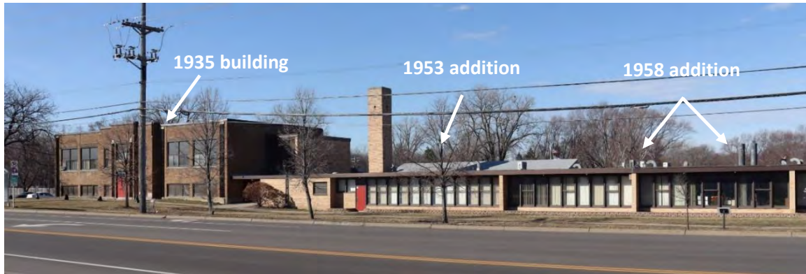
Figure 28. Facade of original 1935 building (left), with 1953 addition (center), and 1958 addition (right), view facing southwest.
