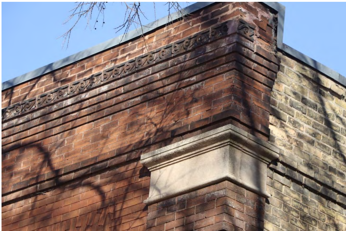
Figure 6. Detail view of molded band motif, stone capital, and brick work, view toward northwest.
