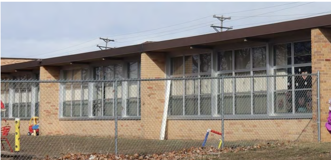
Figure 17. Rear (west) elevation of 1958 addition with replacement windows, view facing northeast.
