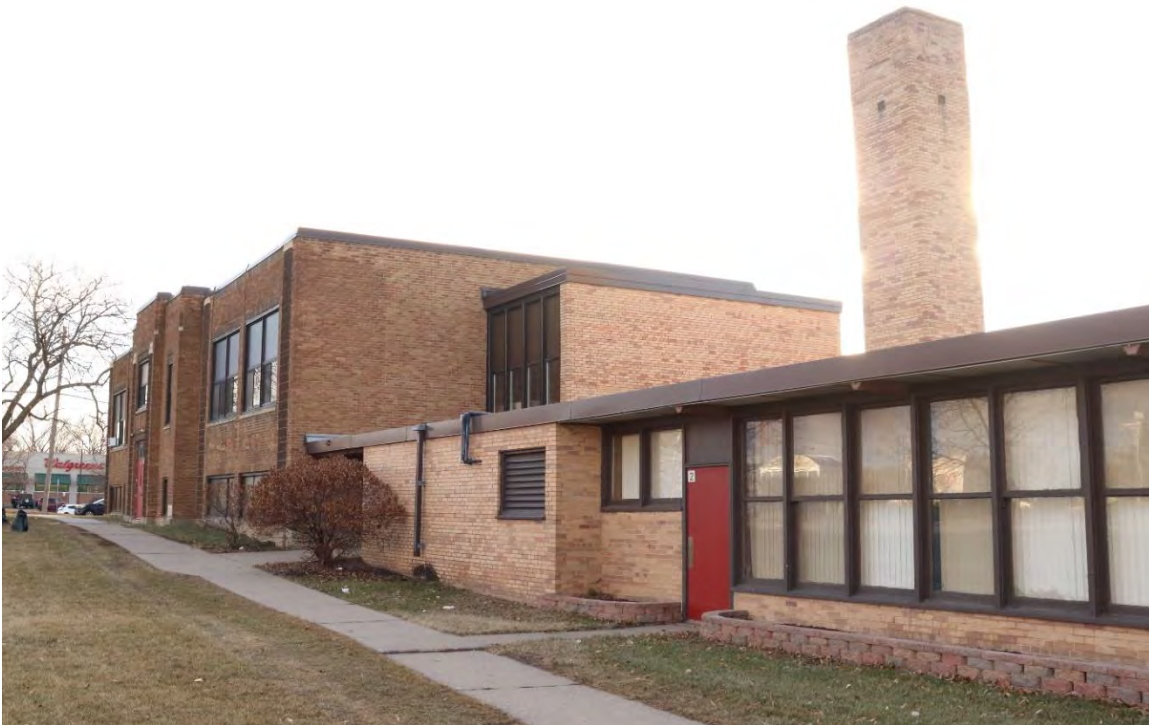
Figure 12. Facade of 1953 addition with original 1935 school building (left), view facing southwest.
