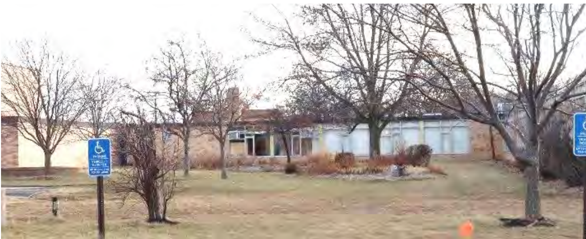
Figure 24. Side (north) elevation of 1961 library hyphen addition, view facing south.
