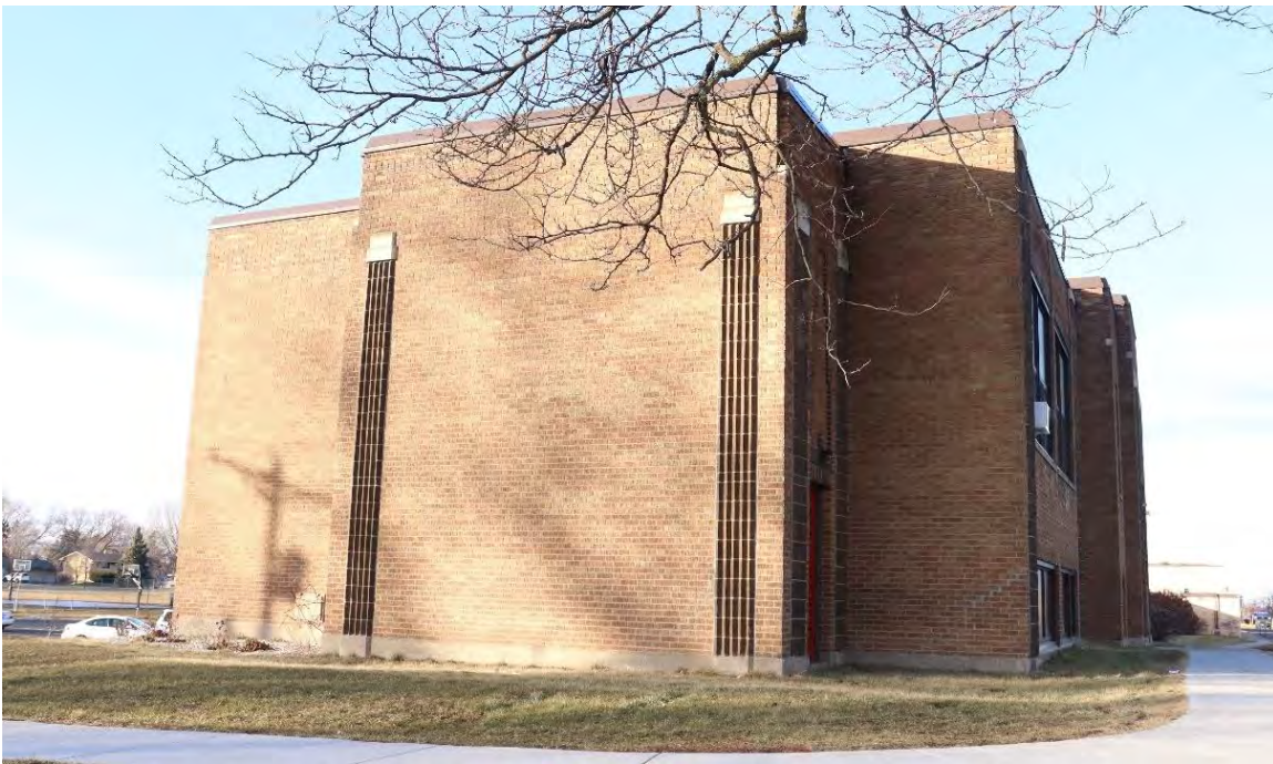
Figure 6. Side (south) elevation of original 1935 North Heights School, view facing north.
