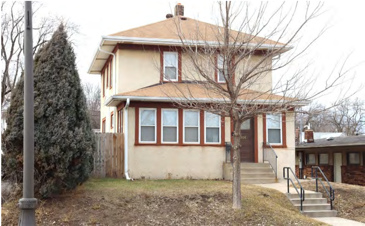
DK-WPC-00087, March 06, 2024, front (east) facade and side (south) elevation, view facing northwest.
