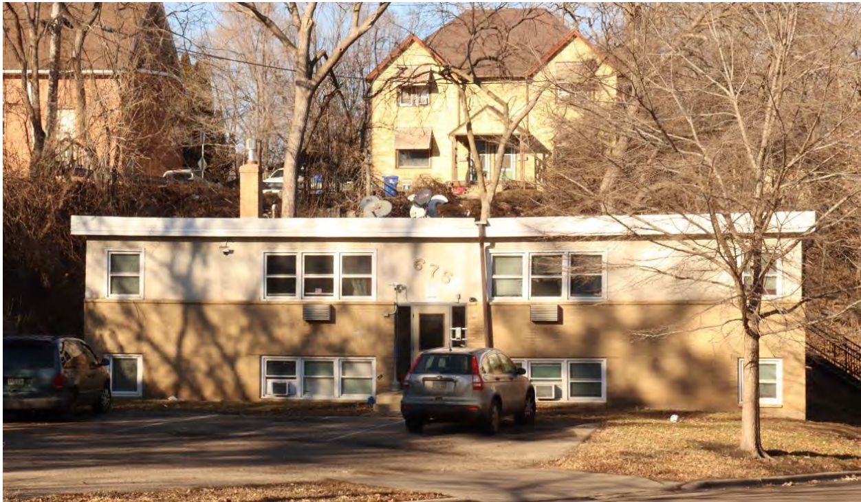
RA-SPC-11935, January 31, 2024, front (south) facade, view facing north.
