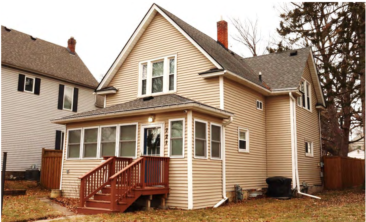
RA-SPC-09005, February 02, 2024, front (east) facade and side (north) elevation, view facing southwest.
