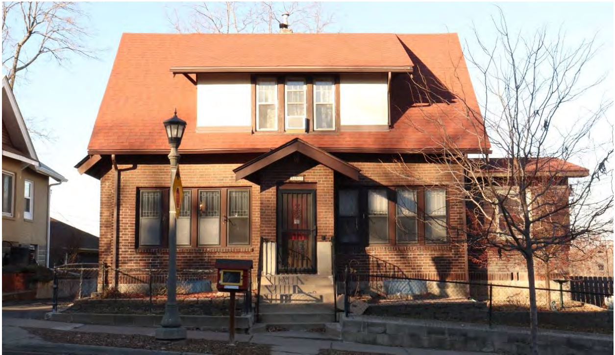
RA-SPC-11921, January 31, 2024, front (south) facade, view facing north.
