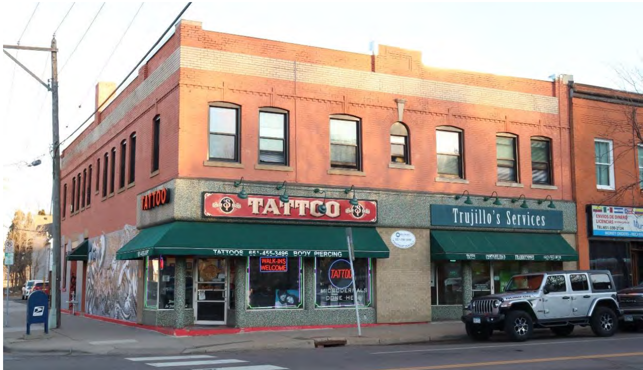
RA-SPC-03187, January 31, 2024, Front (west) facade and side (north) elevation, view facing southeast.
