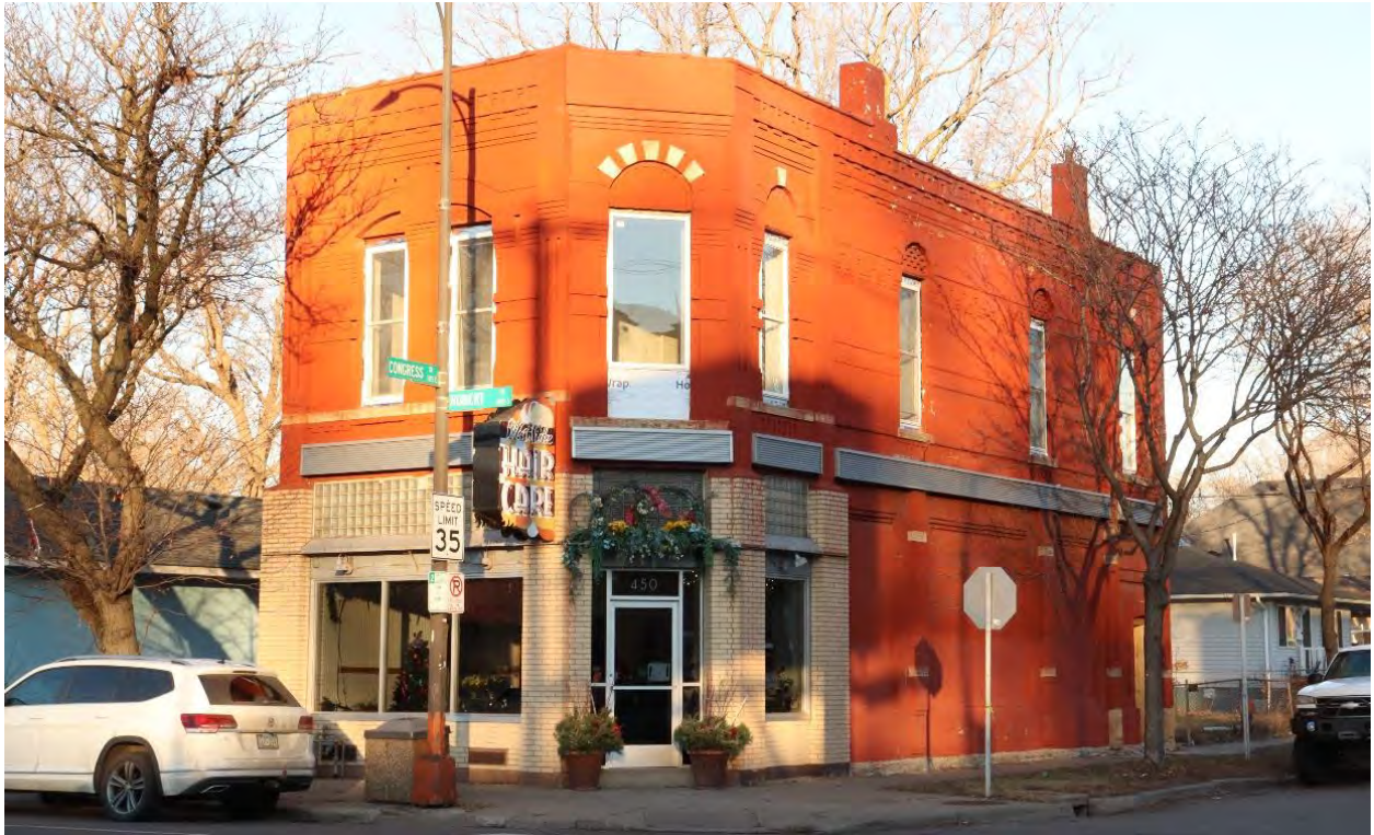
RA-SPC-03186, January 31, 2024, front (west) facade and side (south) elevation, view facing northeast.
