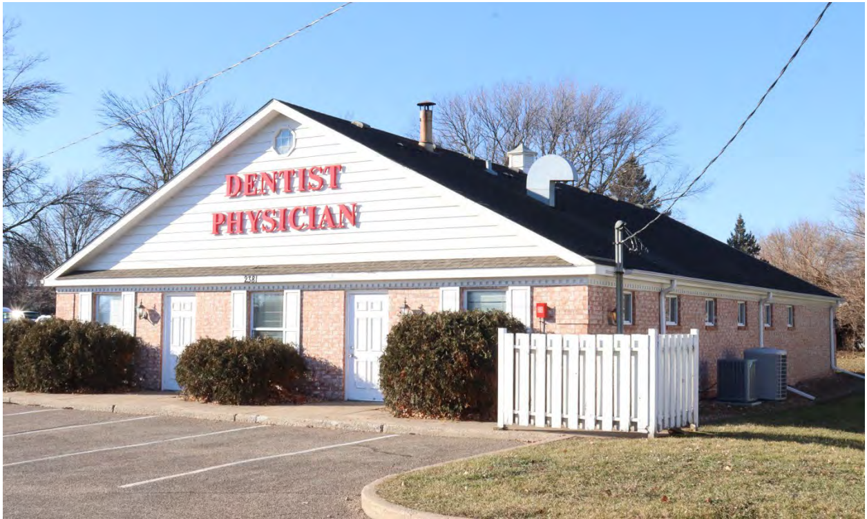
RA-RVC-00062, January 29, 2024, side (east) elevation, rear (north) elevation, and small fence adjacent to the northeast corner of the building, view facing southwest.
