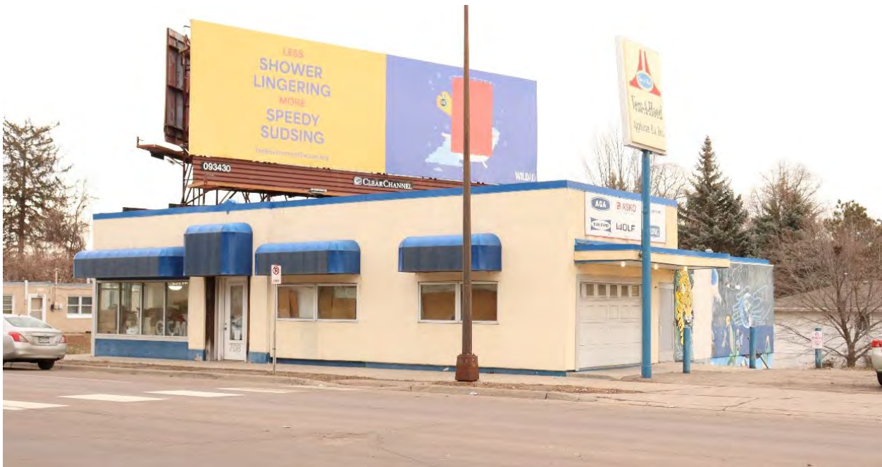
RA-SPC-09002, January 29, 2024, front (west) facade and side (south) elevation, view facing northeast.
