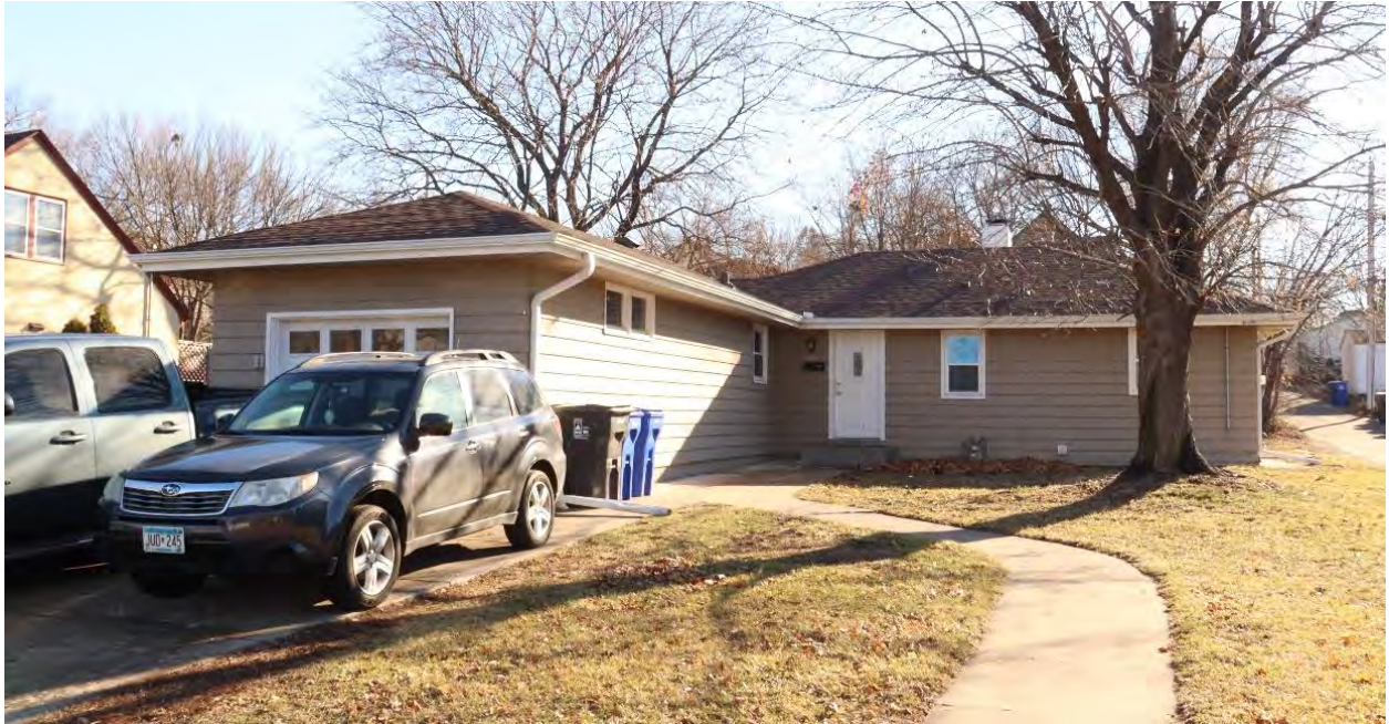
RA-SPC-11911, January 31, 2024, front (north) facade featuring garage extension, view facing southeast.
