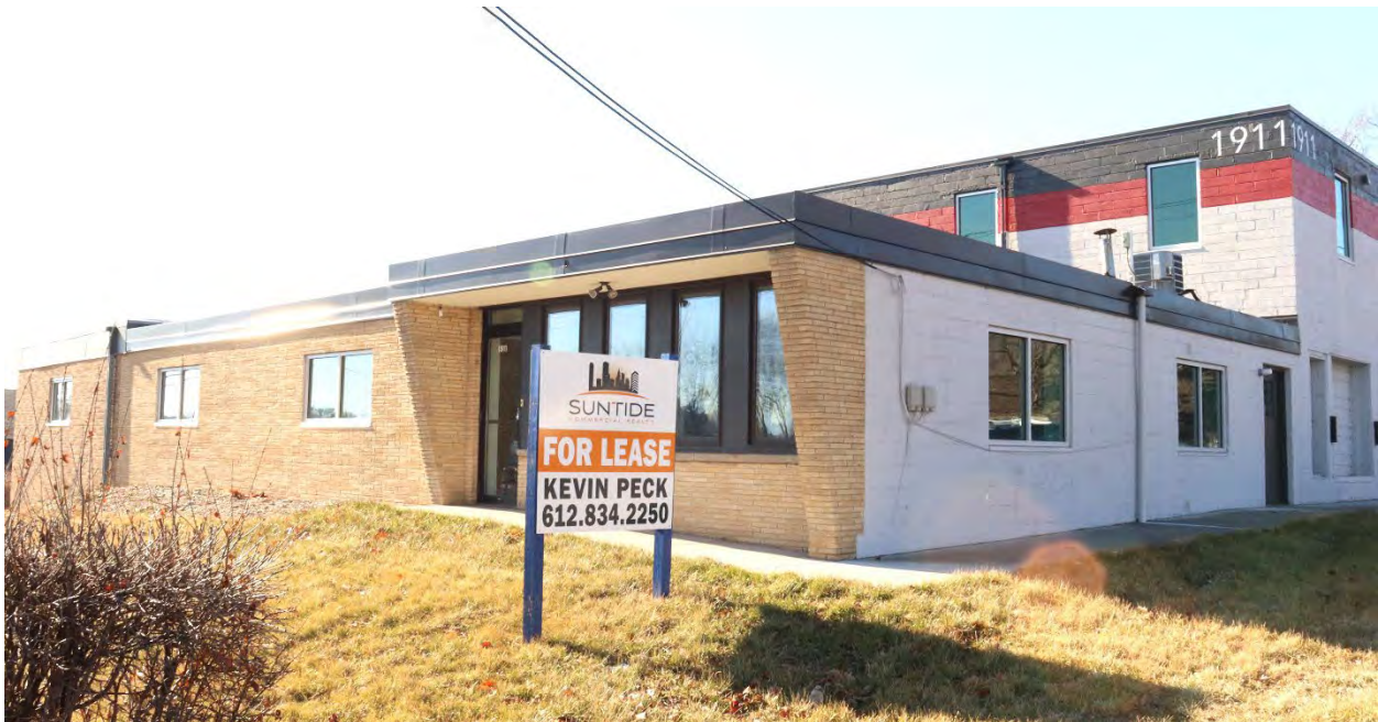
RA-RVC-00016, January 29, 2024, front (north) facade and side (west) elevation, view facing southeast.
