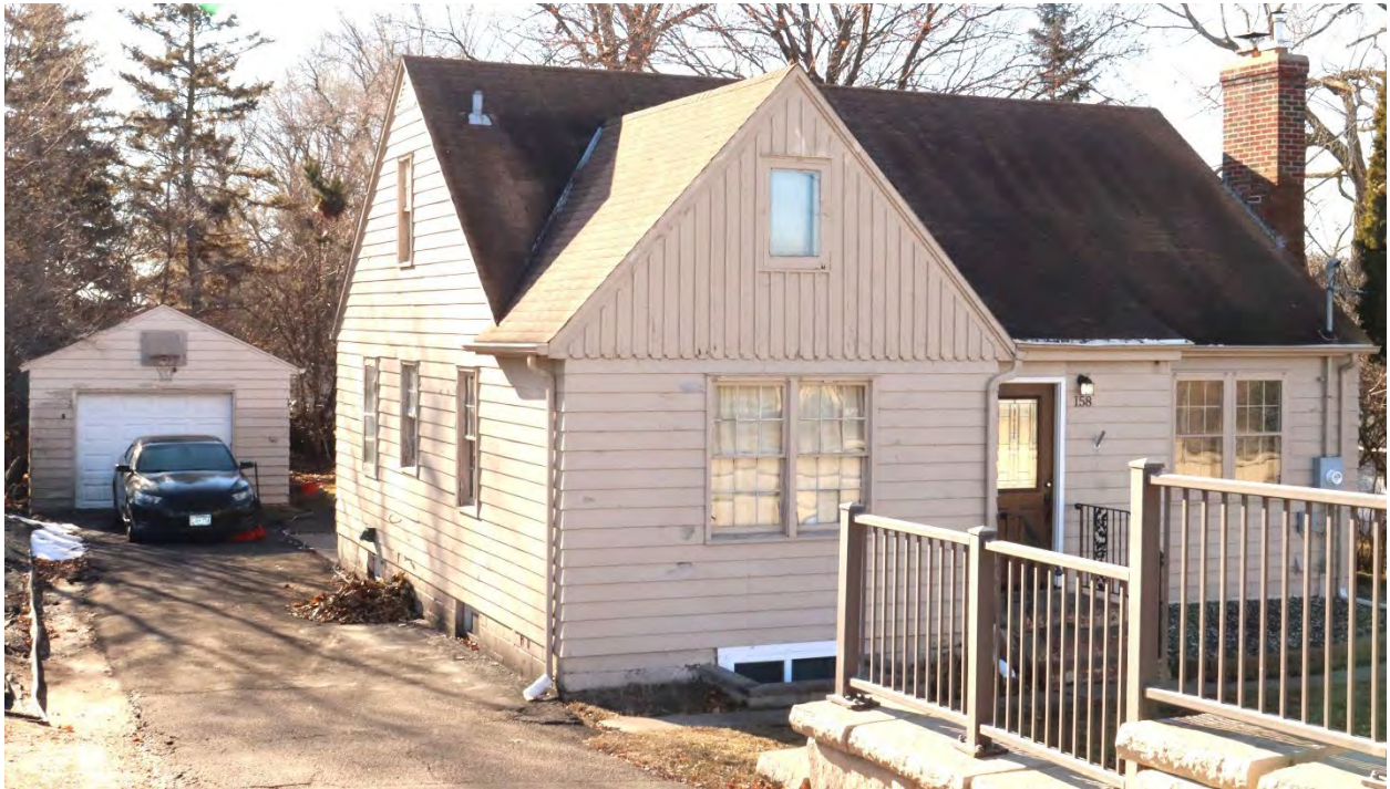
RA-RVC-00055, January 29, 2024, front (north) façade, side (east) elevation, and detached garage, view facing southwest.
