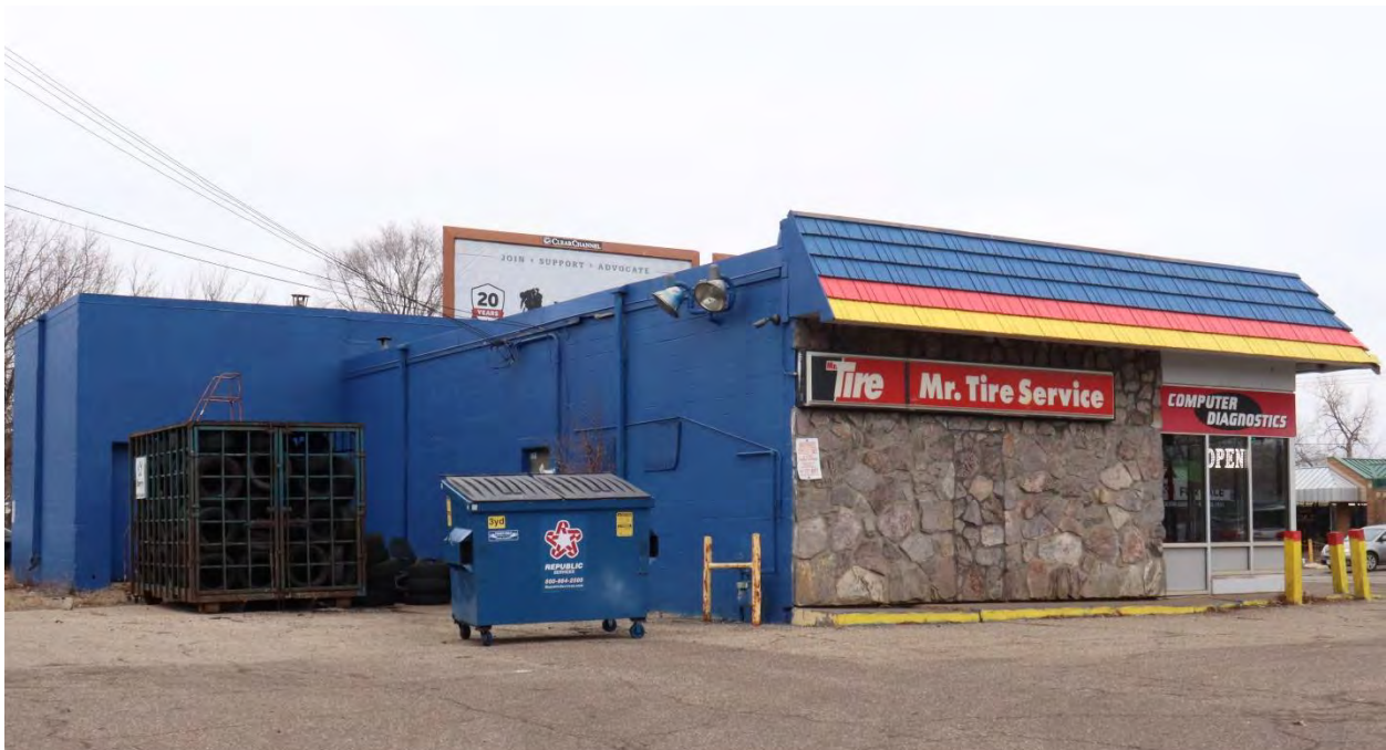
RA-SPC-11903, January 30, 2024, side (south) elevation and rear (west) elevation, view facing northeast.
