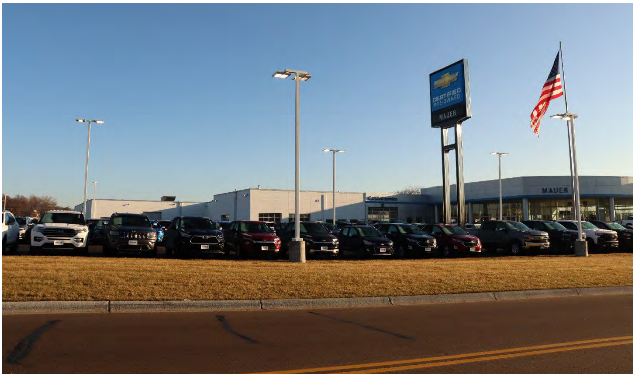
DK-IVG-00063, January 31, 2024, front (southwest) facade and side (northwest) elevation, view facing northeast.
