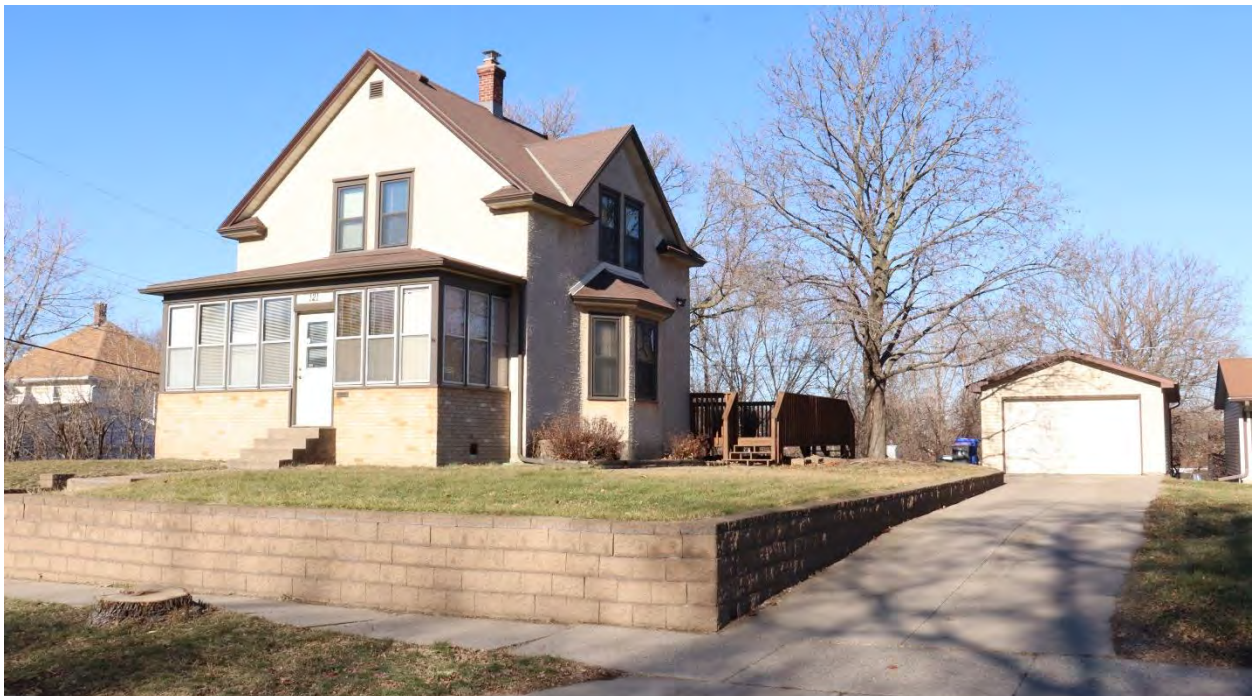
RA-SPC-11906, January 31, 2024, front (south) facade, side (east) elevation, and garage, view facing northwest.
