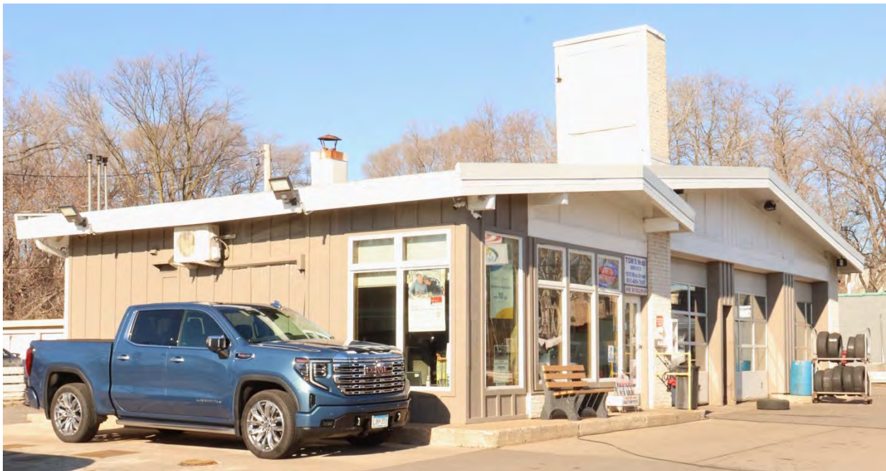
RA-RVC-00059, January 29, 2024, front (east) facade and side (south) elevation, view facing northwest.
