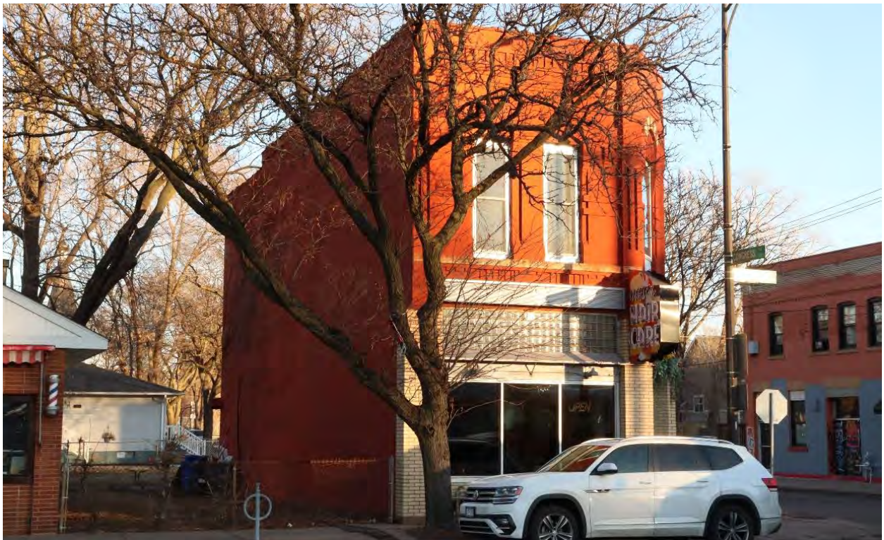
RA-SPC-03186, January 31, 2024, front (west) facade and side (north) elevation, view facing southeast.
