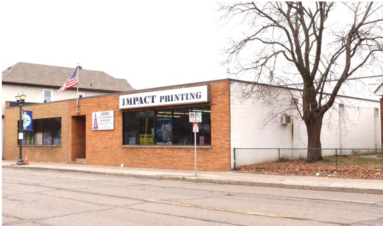
RA-SPC-11894, January 30, 2024, front (east) facade and side (north) elevation, view facing southwest.
