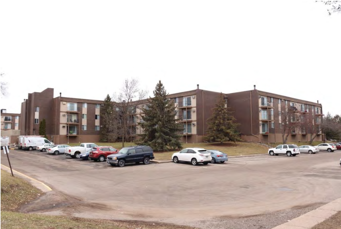
RA-RVC-00065, January 30, 2024, building 2855 front (east) façade and side (north) elevation, view facing southwest.
