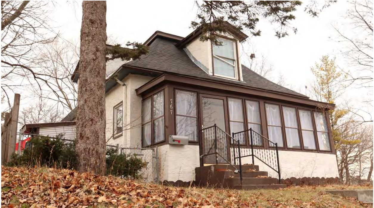
RA-SPC-09020, February 02, 2024, front (east) facade and side (south) elevation, view facing northwest.
