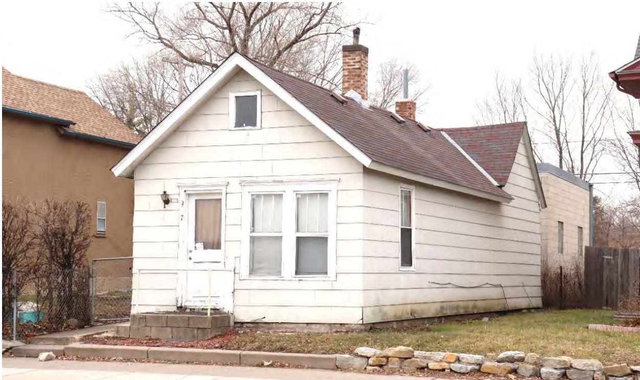
RA-SPC-03084, January 30, 2024, front (east) facade and side (north) elevation, view facing southwest.
