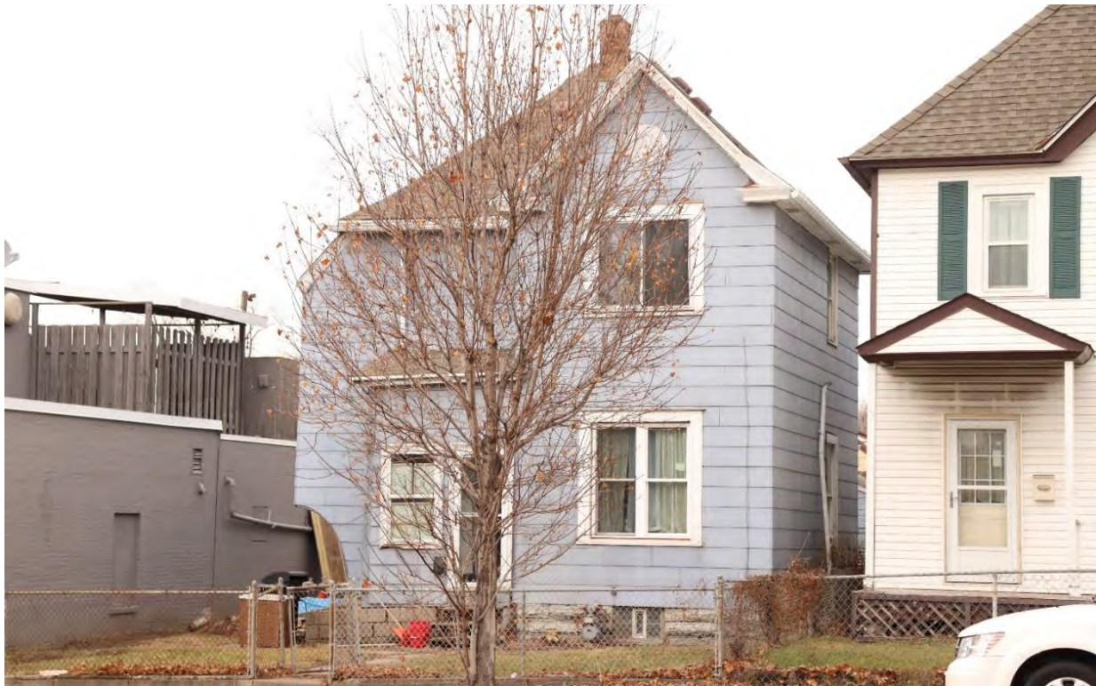
RA-SPC-09009, January 31, 2024, front (west) facade and side (south) elevation, view facing northeast.
