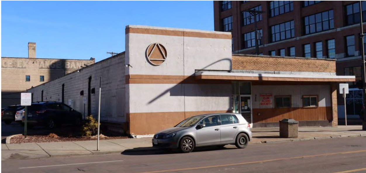
RA-SPC-08961, February 01, 2024, front (southwest) and side (northwest) elevation, view facing east.
