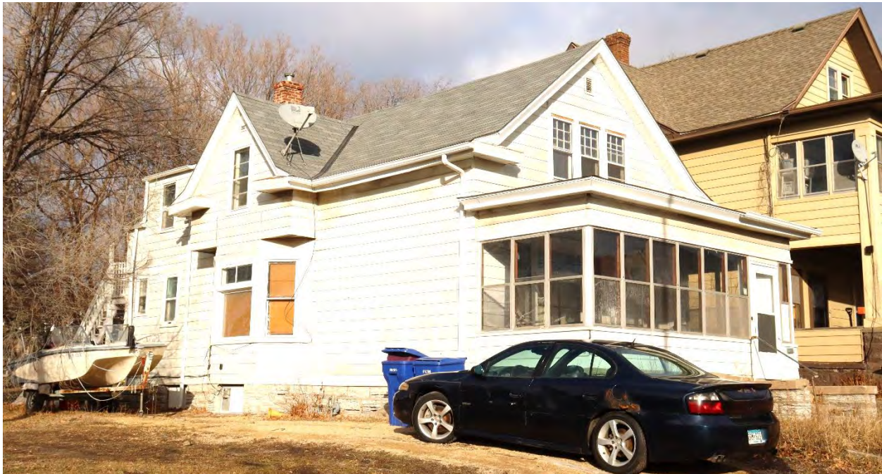
RA-SPC-11910, January 30, 2024, front (south) facade and side (west) elevation, view facing northeast.
