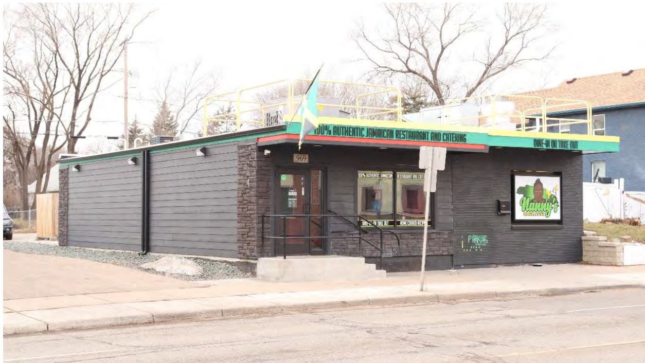
RA-SPC-11940, January 30, 2024, Front (east) facade and side (south) elevation, view facing northwest.
