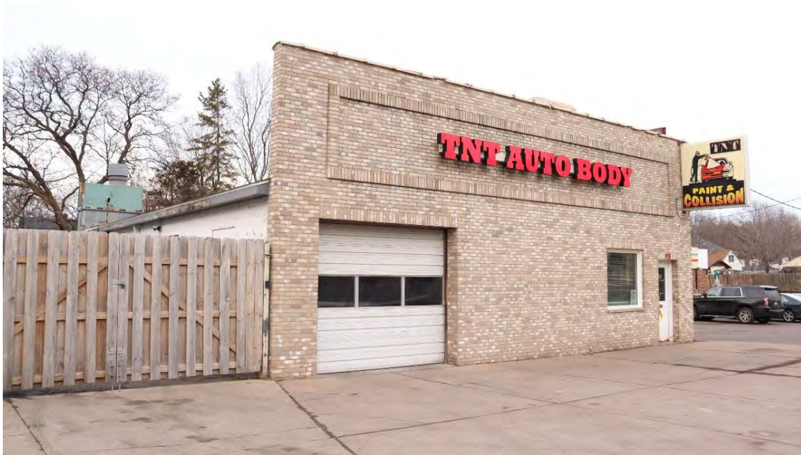
RA-SPC-11937, January 29, 2024, Side (south) elevation, view facing northeast.
