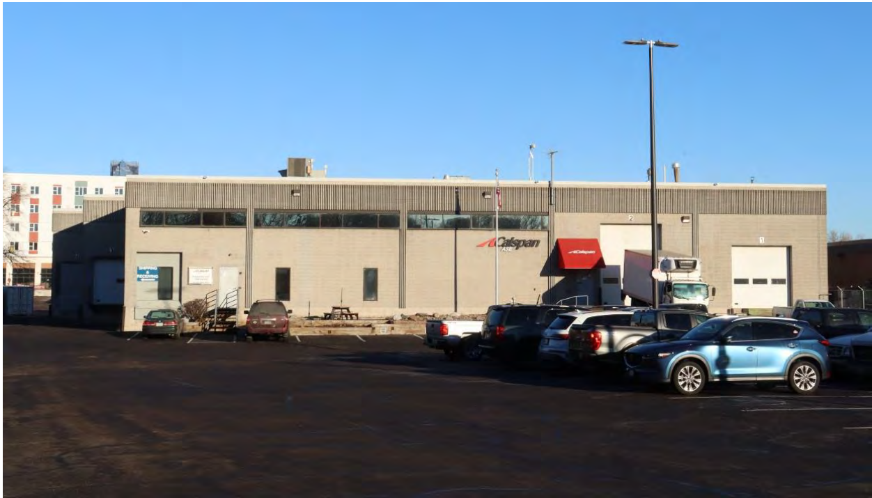
RA-SPC-11928, February 1, 2024, front (south) facade, view facing north.
