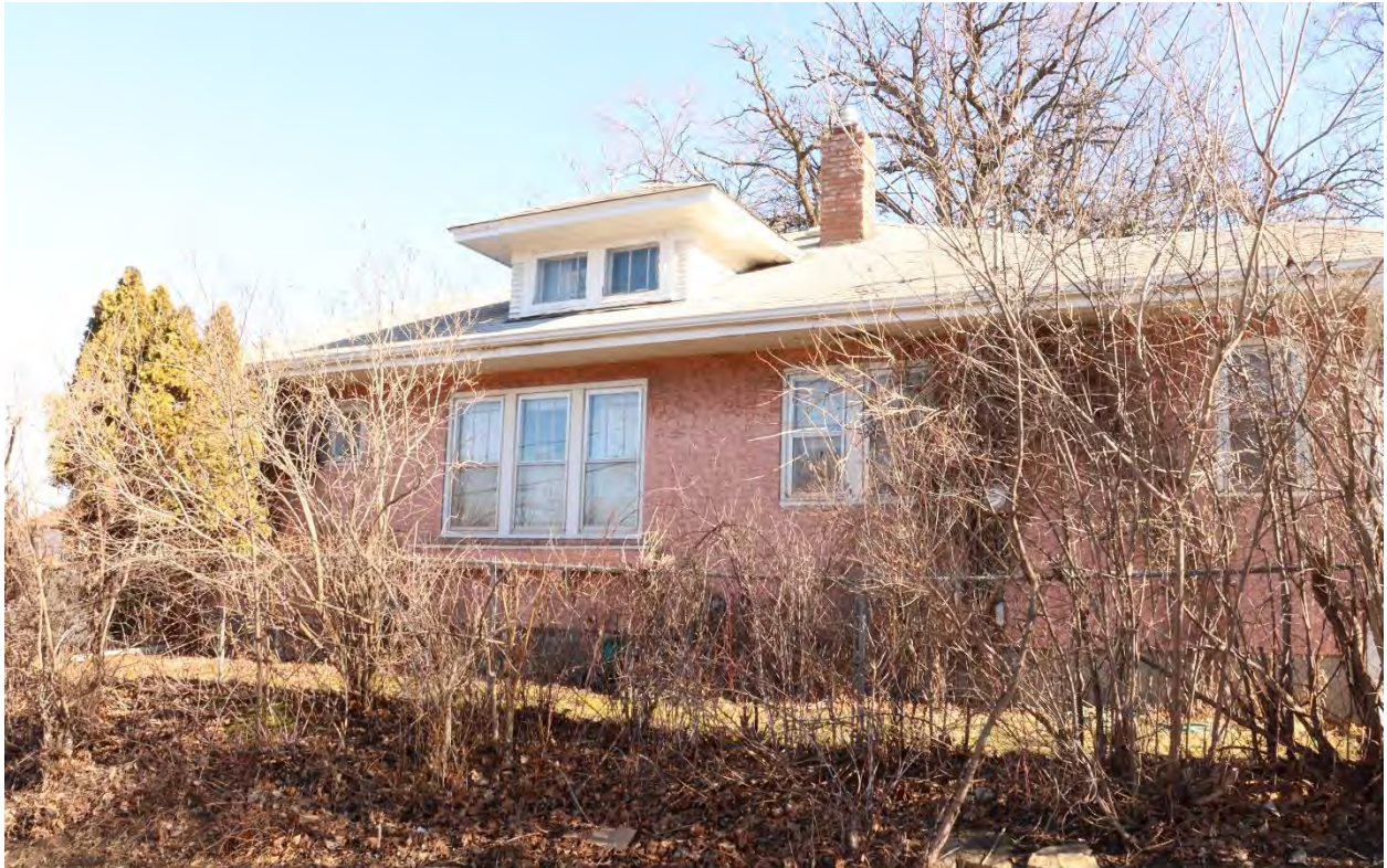
RA-SPC-11908, January 31, 2024, side (west) elevation, view facing northeast.
