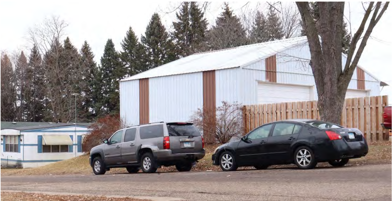
RA-LCC-00083, January 30, 2024, view of large, non-historic-age, metal storage building at Day Avenue and Park Street, view facing southeast.
