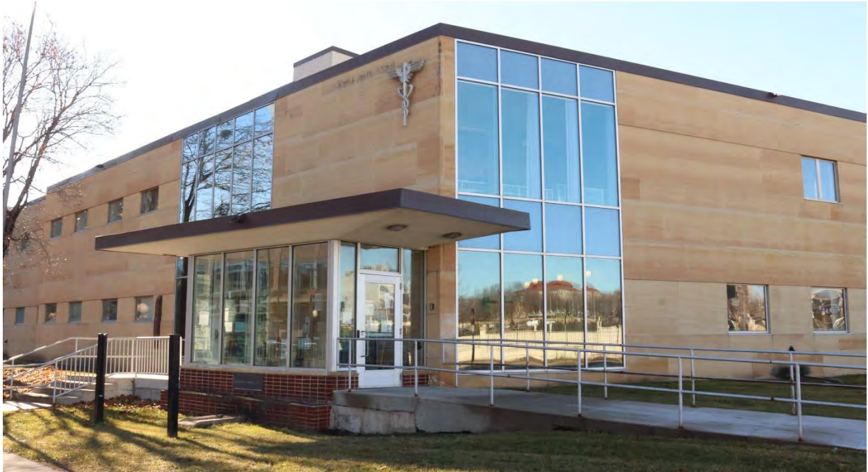
RA-SPC-00556, February 01, 2024, front (northeast) facade and side (northwest) elevation, view facing south.
