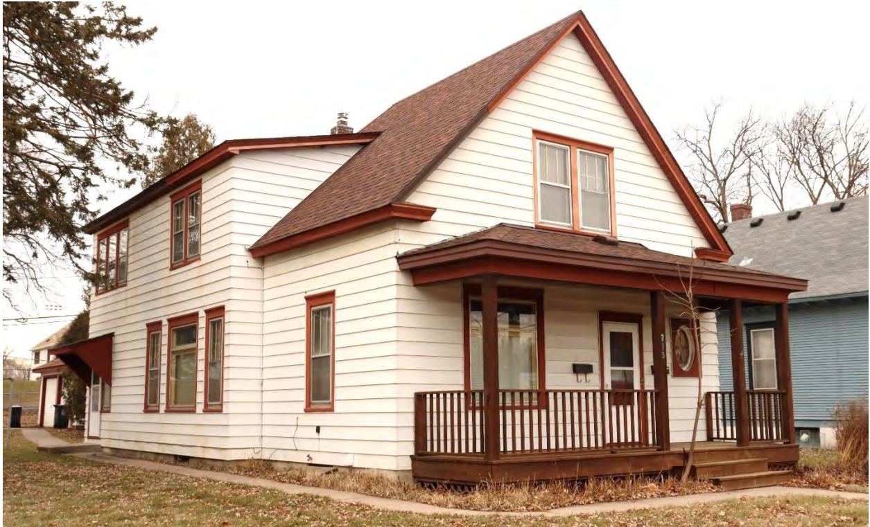
RA-SPC-09004, February 02, 2024, front (east) facade and side (south) elevation, view facing northwest.
