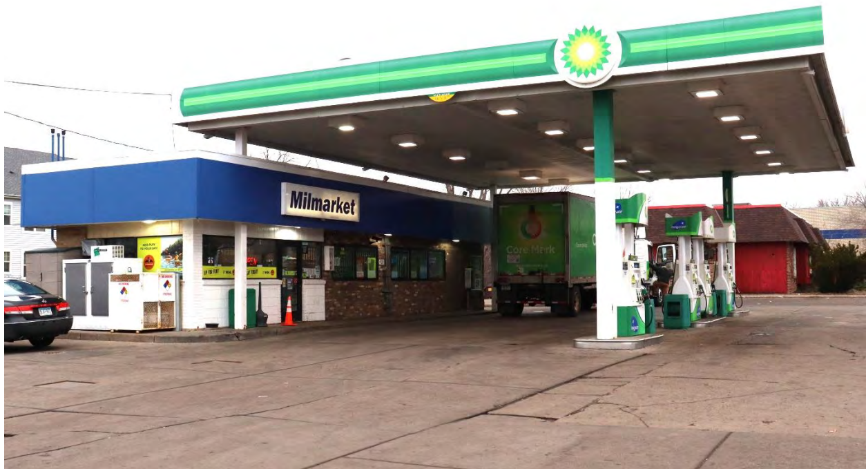
RA-SPC-11917, January 29, 2024, front (west) facade, side (north) elevation, and gas pump canopy, view facing southeast.
