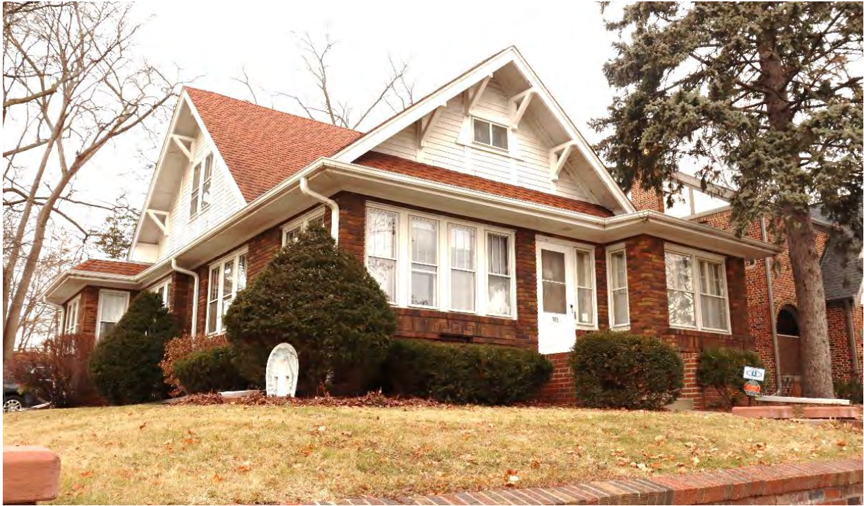
RA-SPC-09000, January 29, 2024, front (north) facade and side (east) elevation, view facing southwest.
