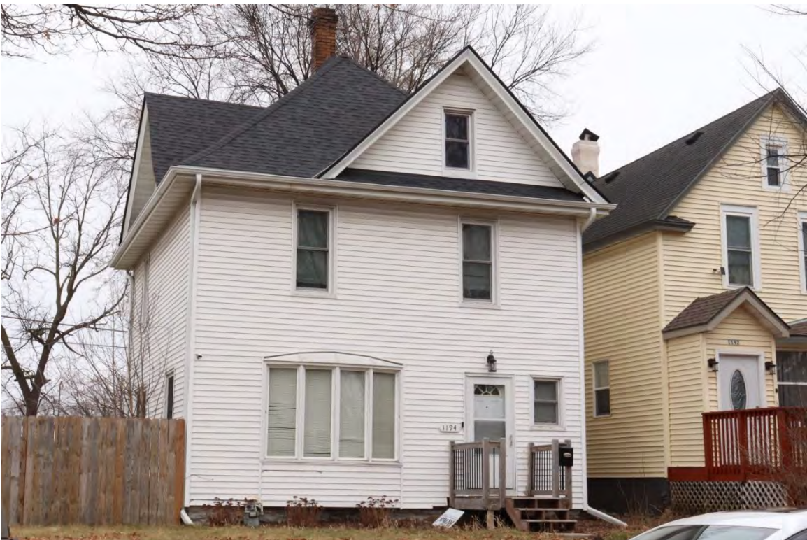
RA-SPC-11901, January 30, 2024, front (west) facade and side (north) elevation, view facing southeast.
