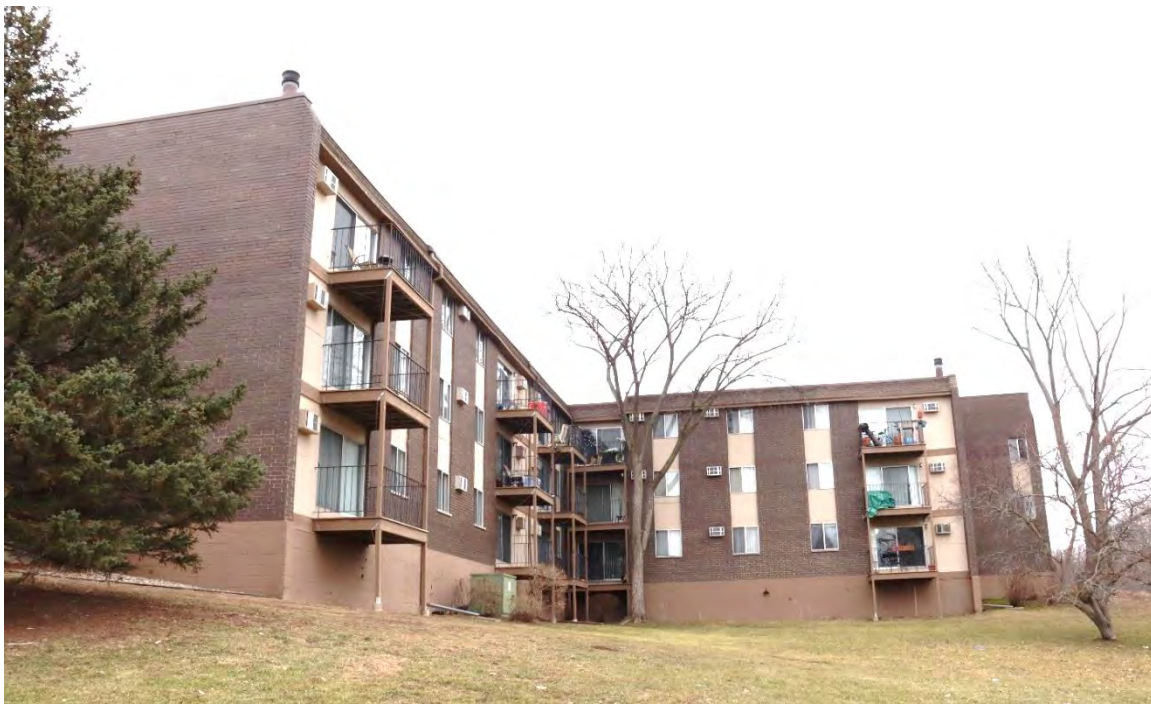
RA-RVC-00065, January 30, 2024, side (east) elevation and side (south) elevations, view facing north.
