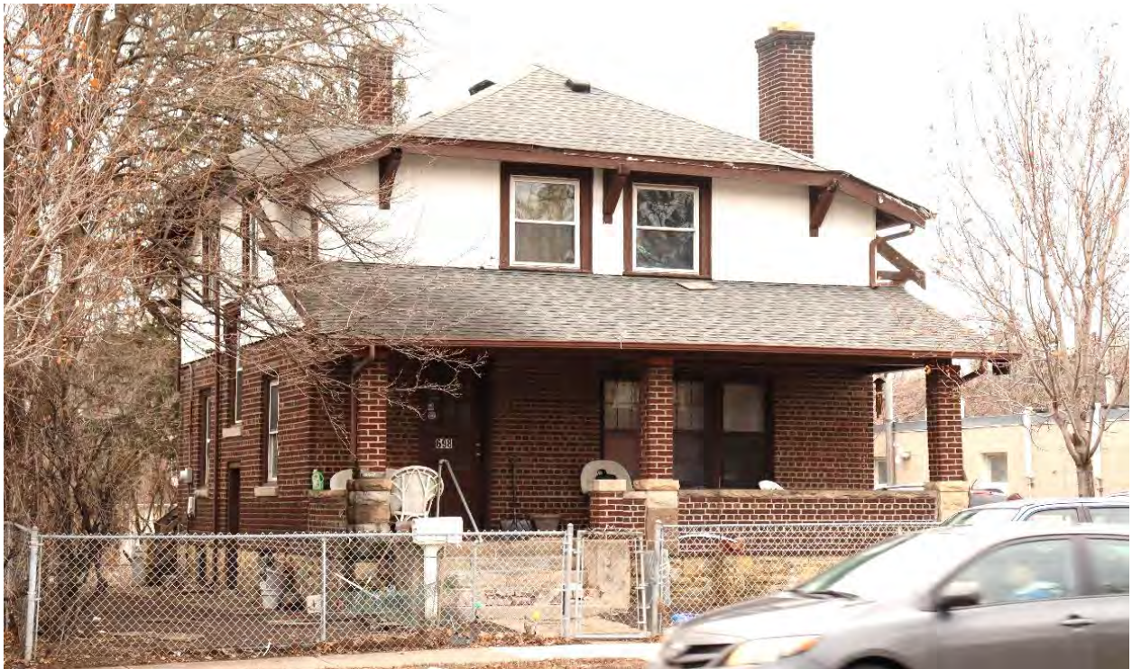
RA-SPC-08998, January 29, 2024, front (west) facade and side (north), view facing southeast.
