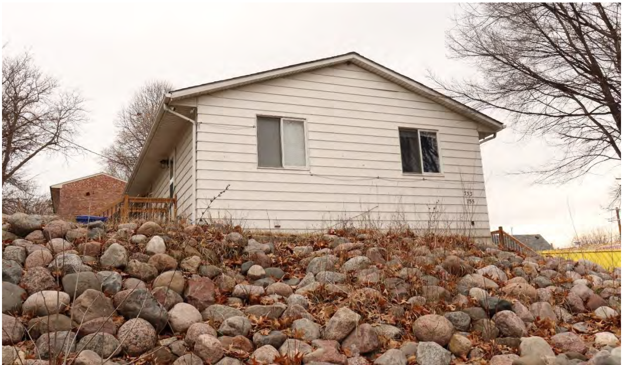
RA-SPC-09014, February 02, 2024, rear (south) and side (east) elevation, view facing northwest.
