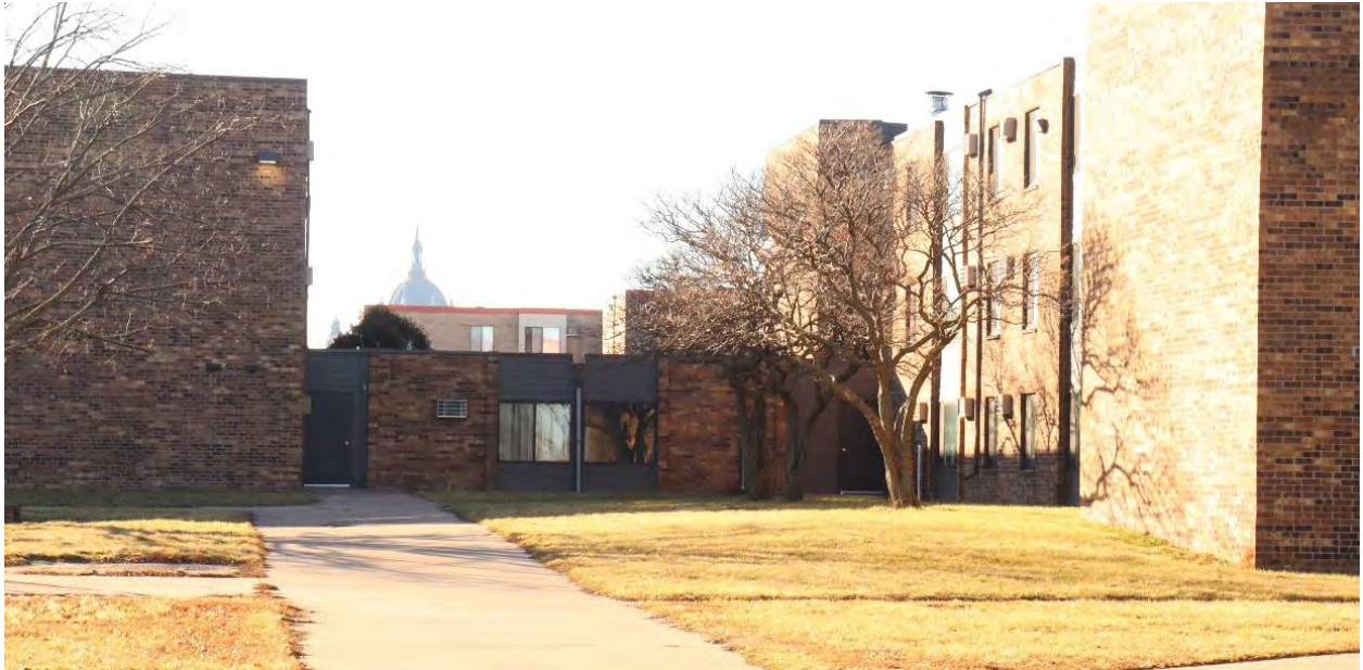
RA-SPC-11929, February 1, 2024, Rear (north) elevation of central administrative office and primary entrance between the building masses, view facing south.
