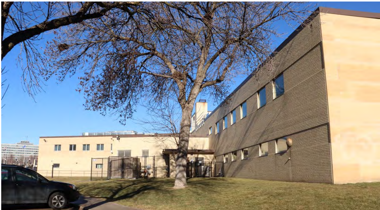
RA-SPC-00556, February 01, 2024, side (southeast) elevation, view facing northwest.
