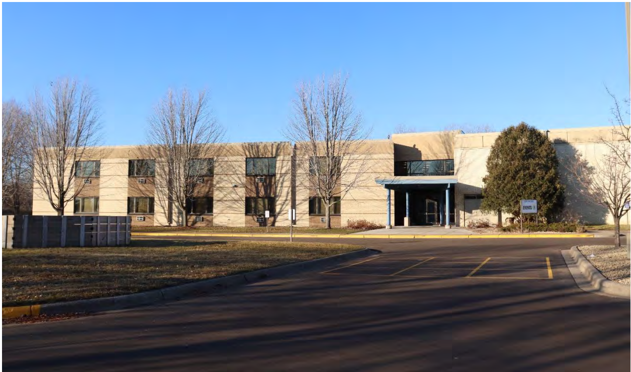
DK-WPC-00081, January 31, 2023, front part of the rear (south) elevation with metal canopy, view facing southwest.
