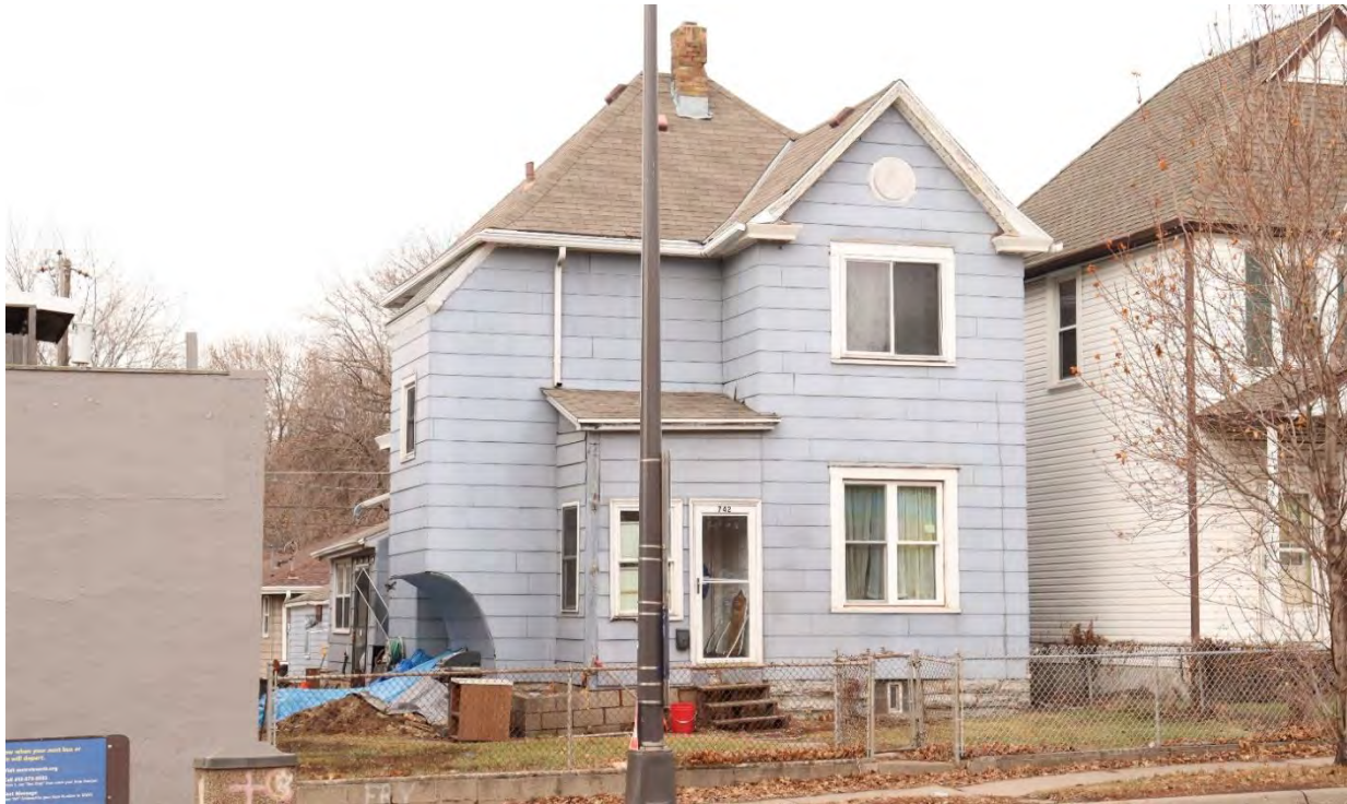
RA-SPC-09009, January 31, 2024, front (west) facade and side (north) elevation, view facing east.
