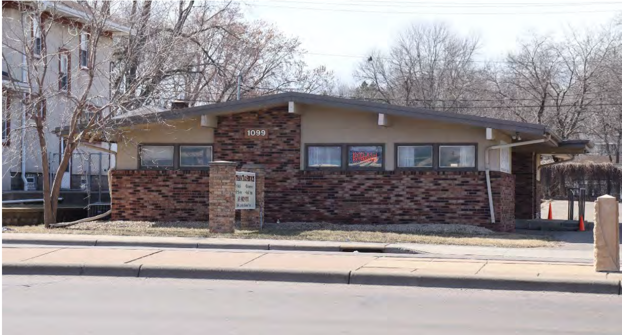
DK-WPC-00085, March 6, 2024, Front (east) facade, view facing west.
