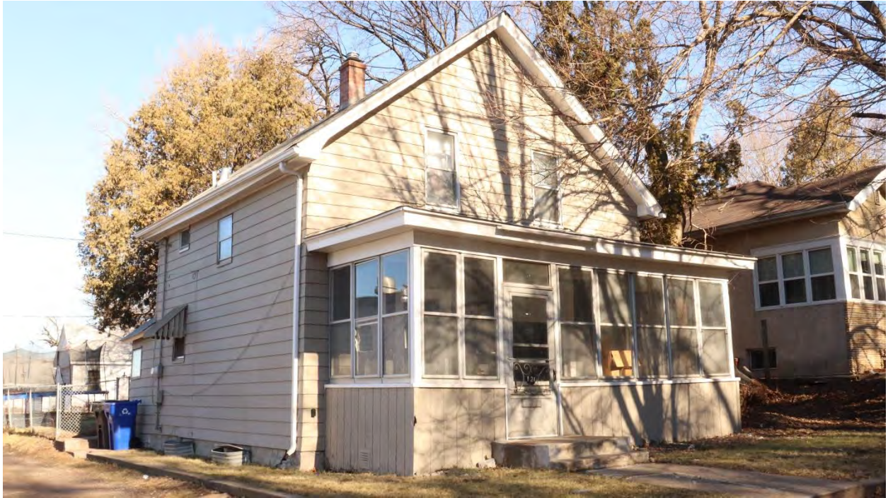
RA-SPC-11905, January 31, 2024, front (south) facade and side (west) elevation, view facing northeast.
