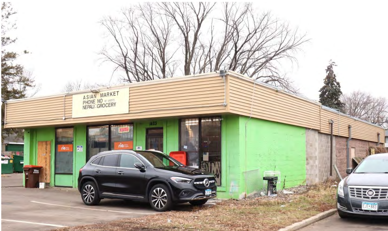
RA-SPC-11914, January 30, 2024, front (east) facade and side (south) elevation, view facing northwest.
