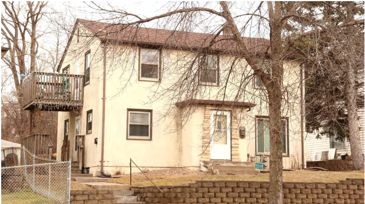
RA-SPC-09021, February 2, 2024, front (west) facade and side (north) elevation, view facing southeast.
