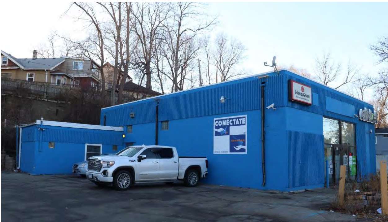
RA-SPC-11920, January 31, 2024, side (southeast) elevation and front (northeast) facade featuring side addition, view facing west.
