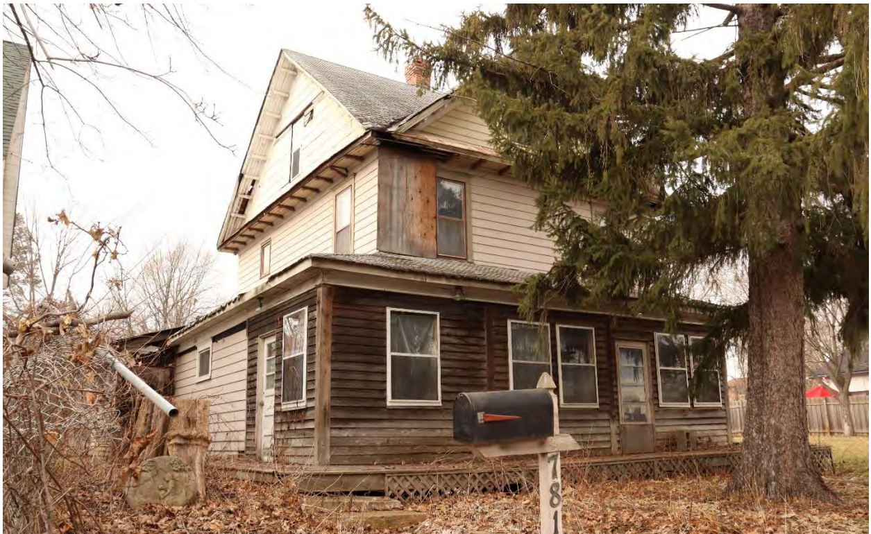
RA-SPC-09022, February 02, 2024, front (east) facade and side (north) elevation, view facing west.
