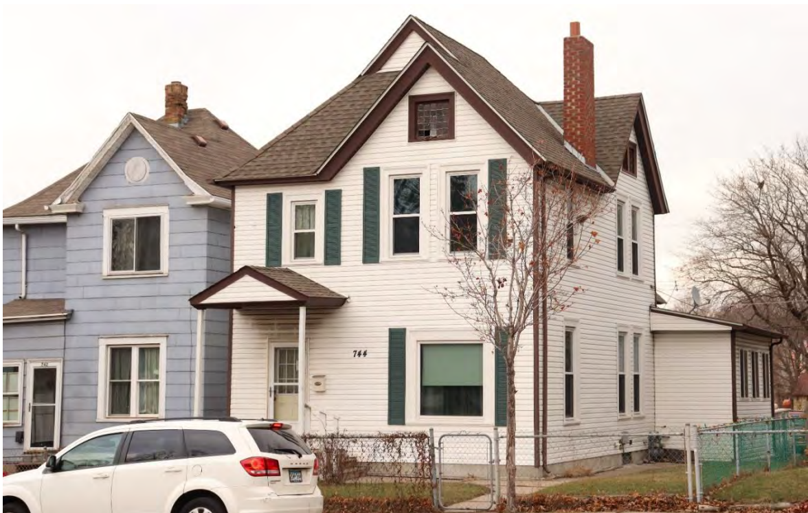
RA-SPC-09010, January 31, 2024, front (west) facade and side (south) elevation, view facing northeast.
