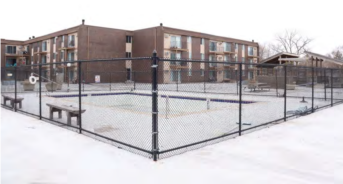
RA-RVC-00065, January 30, 2024, courtyard, showing pool (center), gazebo (right), and part of building 2835's north and east elevations.
