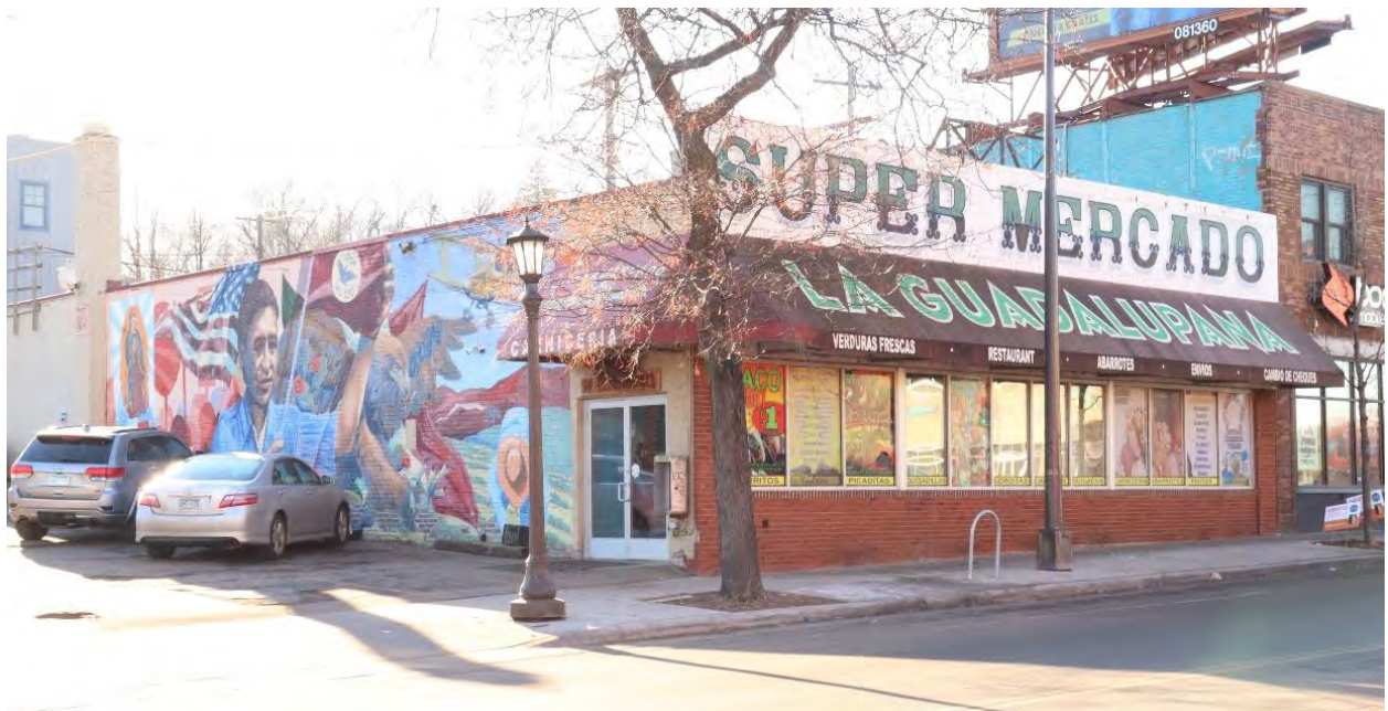
RA-SPC-11927, January 31, 2024, side (east) elevation and front (north) facade, view facing southwest.
