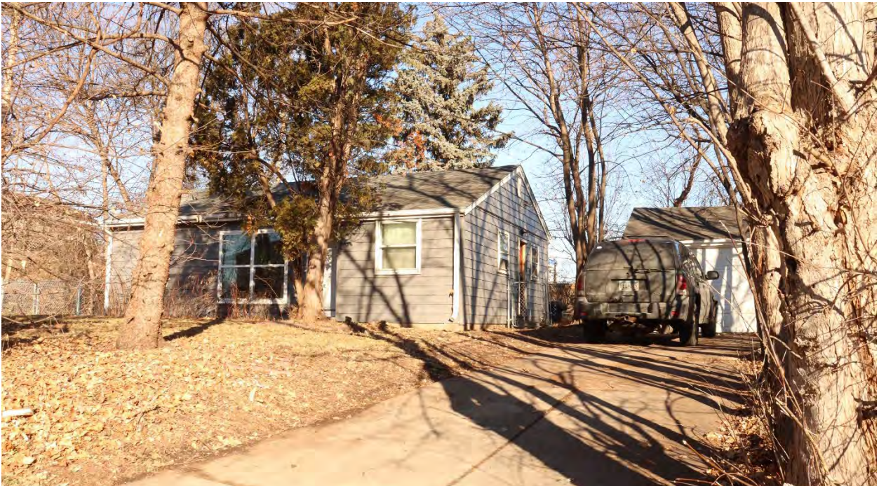
DK-WPC-00095, January 8, 2024, front (south) facade and side (east) elevation, and garage, view facing northwest.
