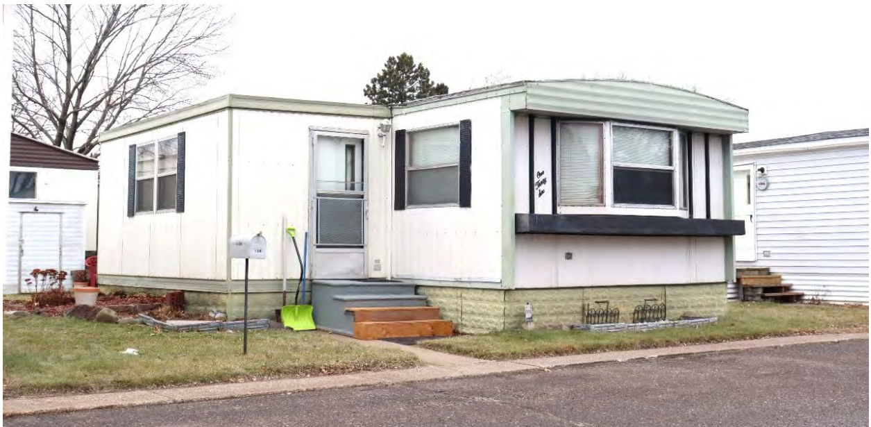
RA-LCC-00083, January 30, 2024, representative example of historic-age mobile home with porch enclosure/addition, view facing northeast.
