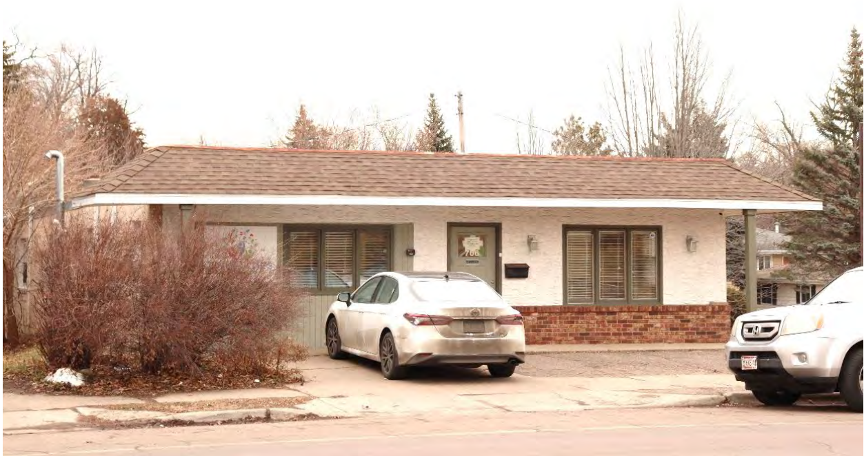
RA-SPC-09001, January 29, 2024, front (west) facade, view facing southeast.
