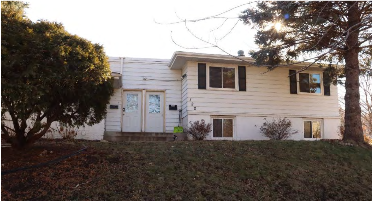
RA-SPC-11904, January 31, 2024, Front (north) facade and detail of connector addition with primary entrances, view facing south.
