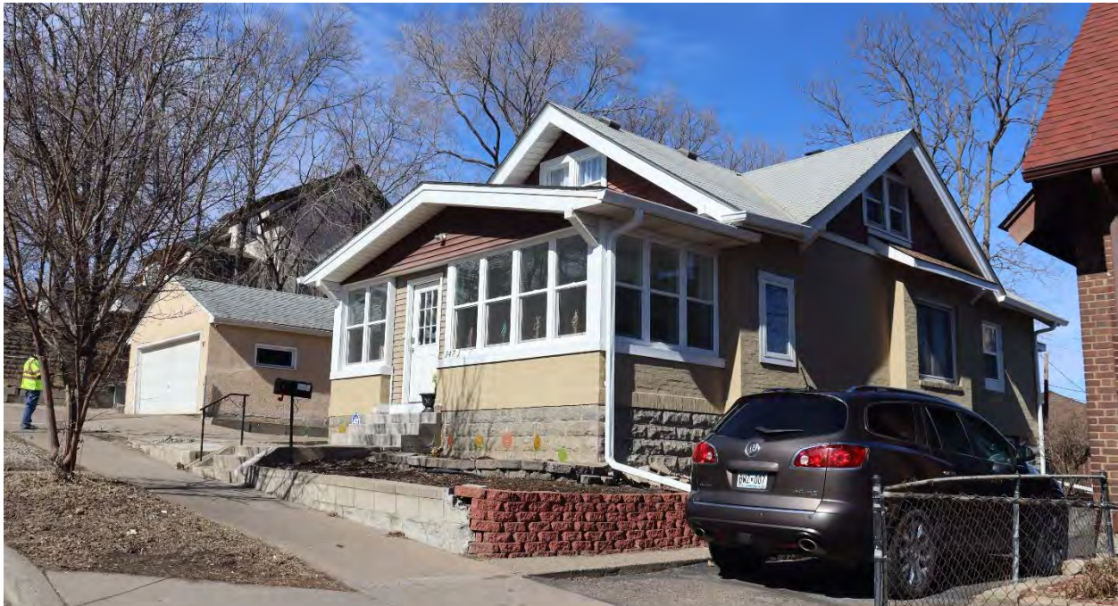
RA-SPC-11918, March 6, 2024, front (south) facade, side (east) elevation, and garage, view facing northwest.
