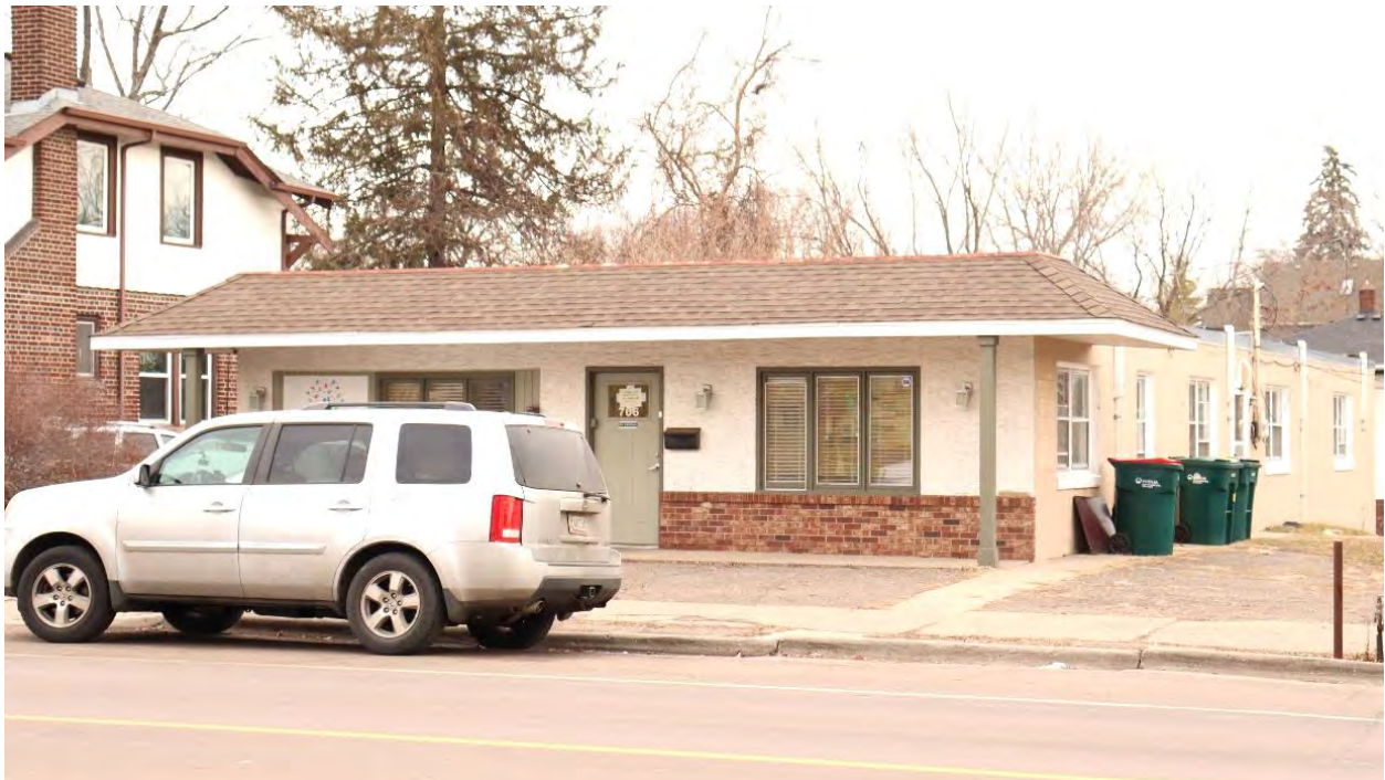
RA-SPC-09001, January 29, 2024, front (west) facade and side (south) elevation, view facing northeast.
