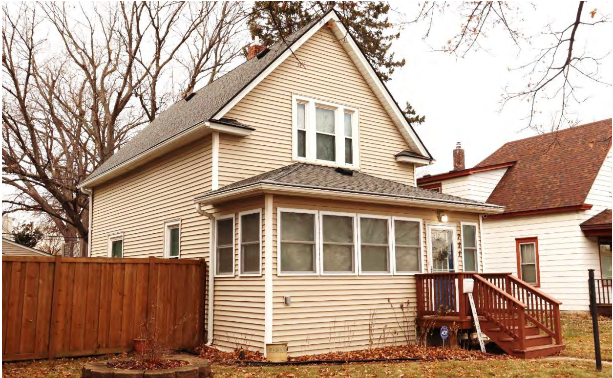
RA-SPC-09005, February 02, 2024, front (east) facade and side (south) elevation, view facing northwest.
