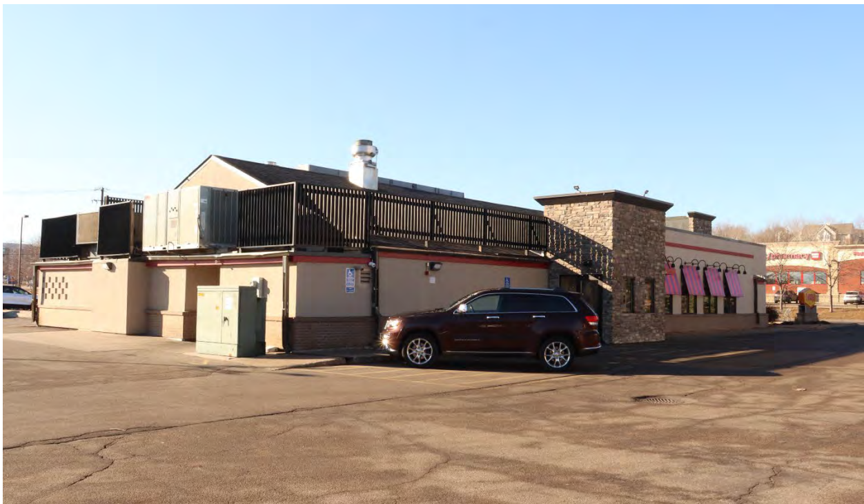
DK-WPC-00098, January 31, 2024, side (north) and rear (east) elevation, view facing southwest.
