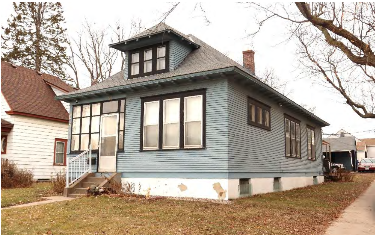
RA-SPC-09003, January 29, 2024, front (east) facade and side (north) elevation, view facing southwest.
