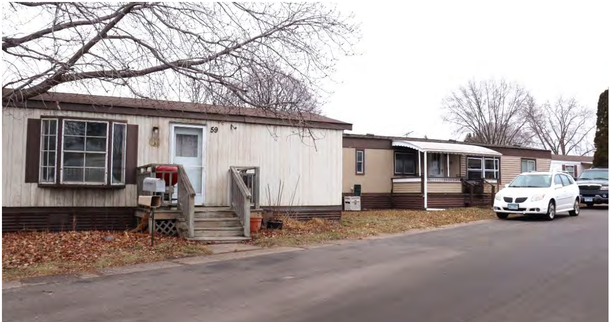
RA-LCC-00083, January 30, 2024, representative examples of historic-age mobile homes with typical alterations including replacement windows, siding, and porch awning, view facing northeast.
