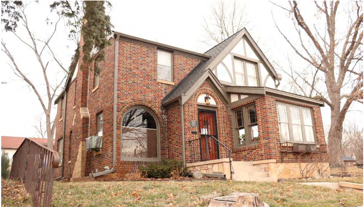
RA-SPC-08999, January 29, 2024, Front (east) facade and side (south) elevation, view facing northwest.
