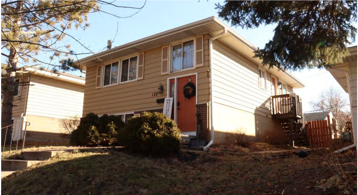
RA-SPC-11912, January 31, 2024, front (north) facade and side (west) elevation, view facing southeast.
