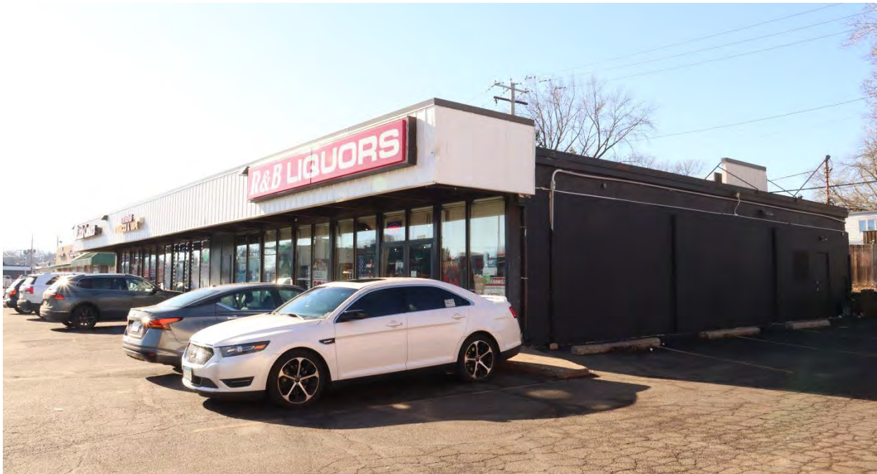
DK-WPC-00089, January 31, 2024, front (east) facade and side (north) elevation, view facing southwest.
