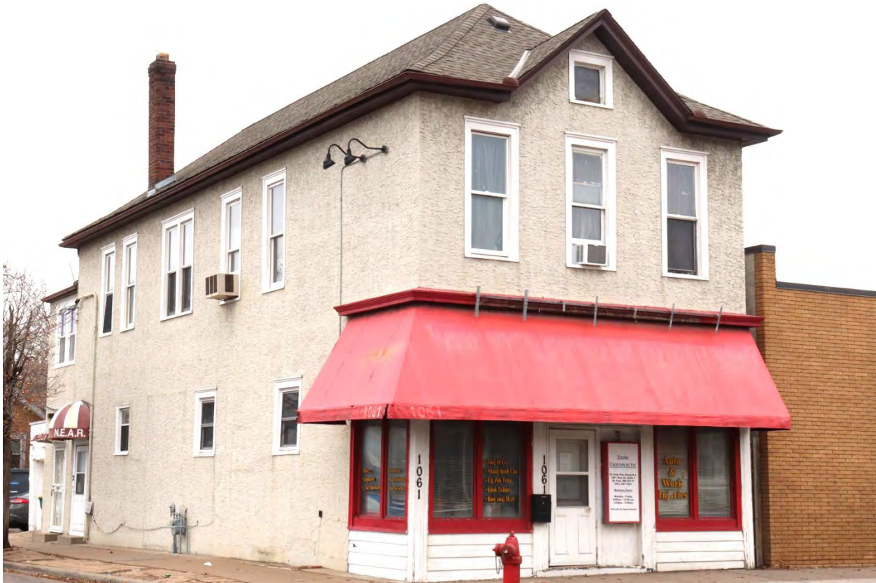
RA-SPC-03088, January 29, 2024, front (east) facade and side (south) elevation, view facing northwest.
