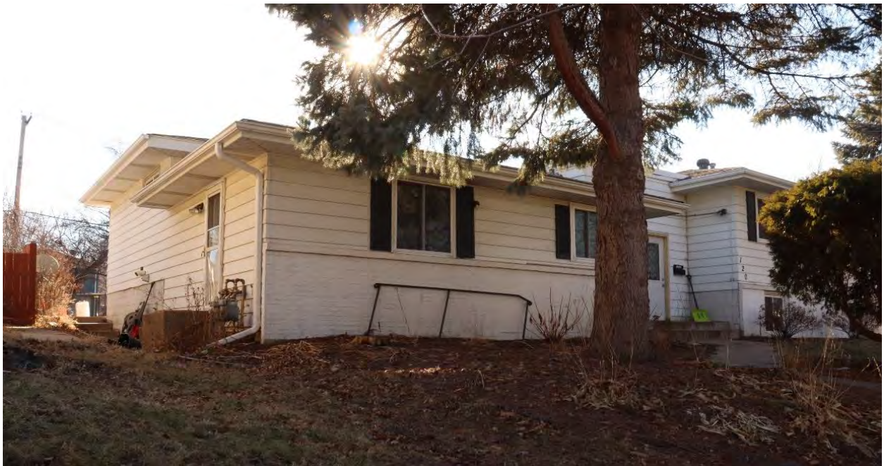
RA-SPC-11904, January 31, 2024, Front (north) facade and side (east) elevation, view facing southwest.
