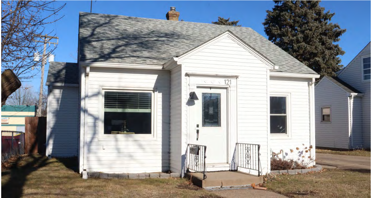
DK-WPC-00094, January 31, 2024, front (south) facade and side (west) elevation, view facing northeast.
