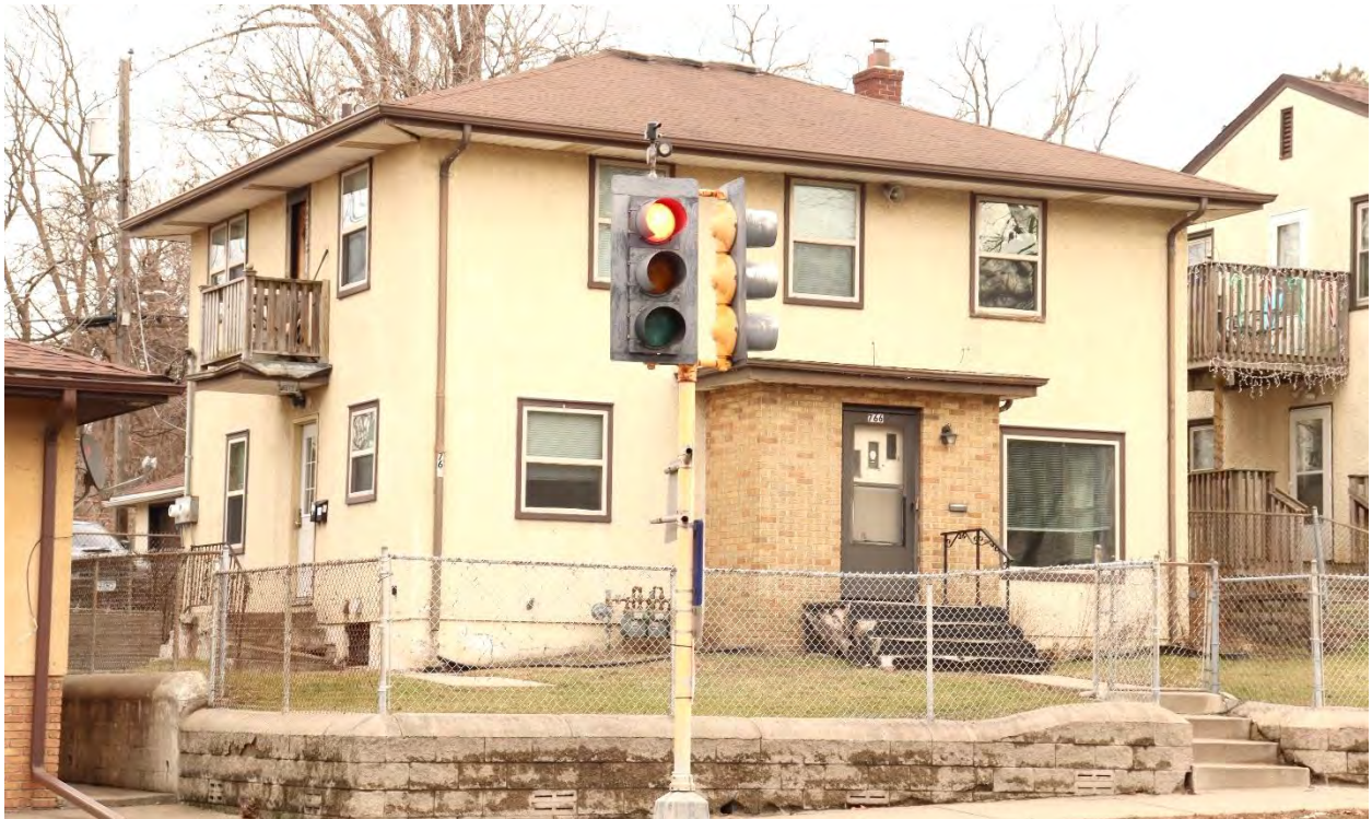
RA-SPC-09019, February 02, 2024, front (west) and side (north) elevation, view facing southeast.
