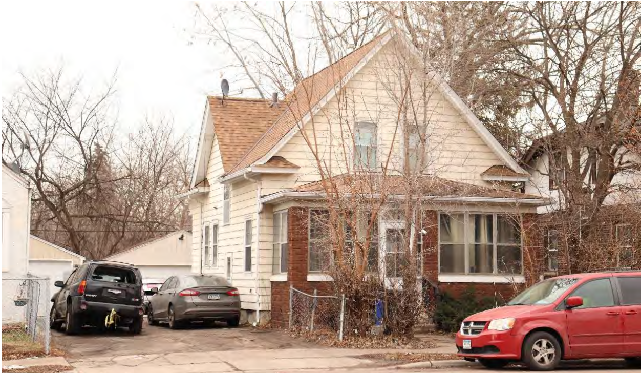
RA-SPC-08997, January 29, 2024, front (west) facade, side (north) elevation, and garage, view facing southeast.
