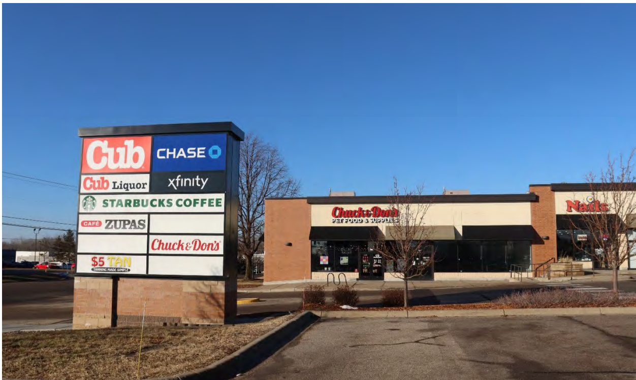
DK-WPC-00100, January 31, 2024, front (east) facade and signage, view facing west.
