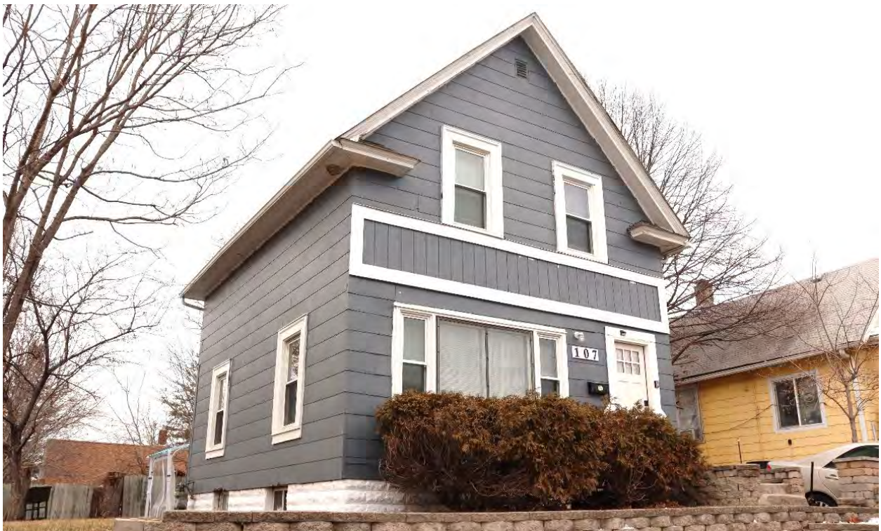
RA-SPC-08953, January 29, 2024, front (south) facade and side (west) elevation, view facing northeast.
