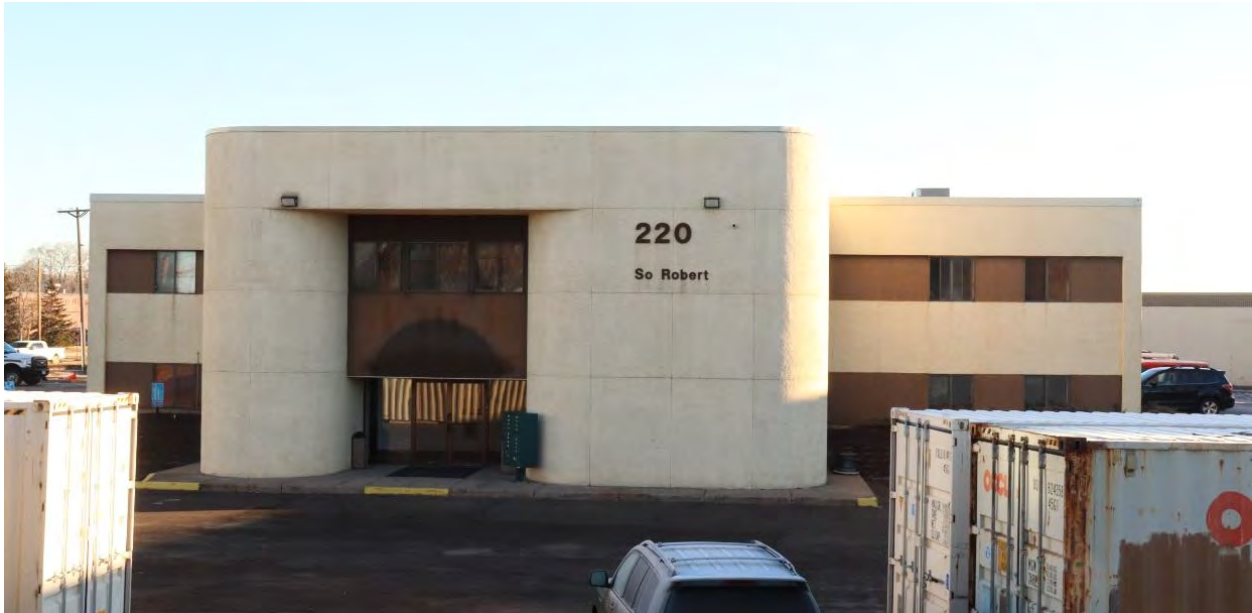
RA-SPC-08966, February 1, 2024, front (west) facade featuring entry addition, view facing east.
