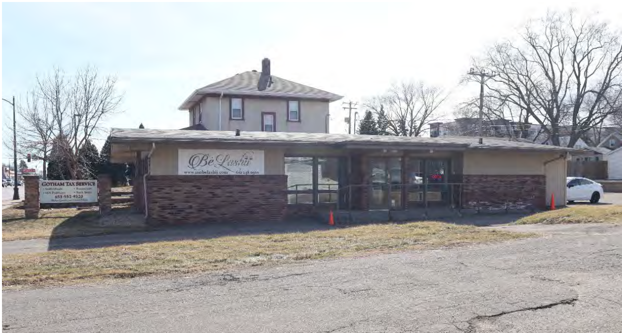
DK-WPC-00085, March 6, 2024, Side (north) elevation featuring primary entrance, view facing southwest.
