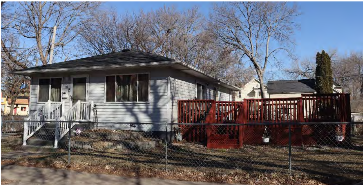
RA-SPC-11896, March 5, 2024, Front (south) facade and side (east) elevation, view facing northwest.
