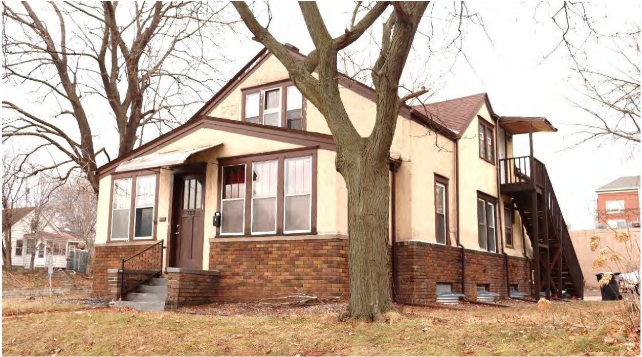
RA-SPC-09042, January 29, 2024, front (north) facade and side (west) elevation, view facing southeast.
