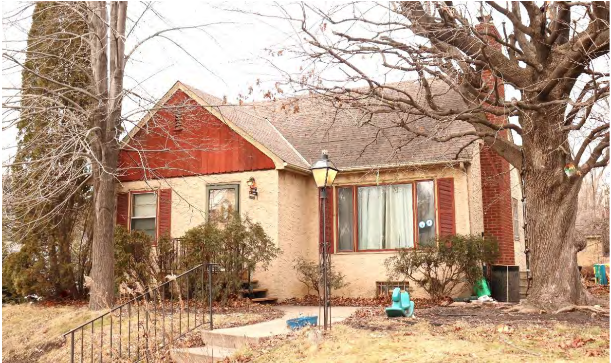
RA-SPC-09039, January 29, 2024, front (west) facade and side (south) elevation, view facing northeast.
