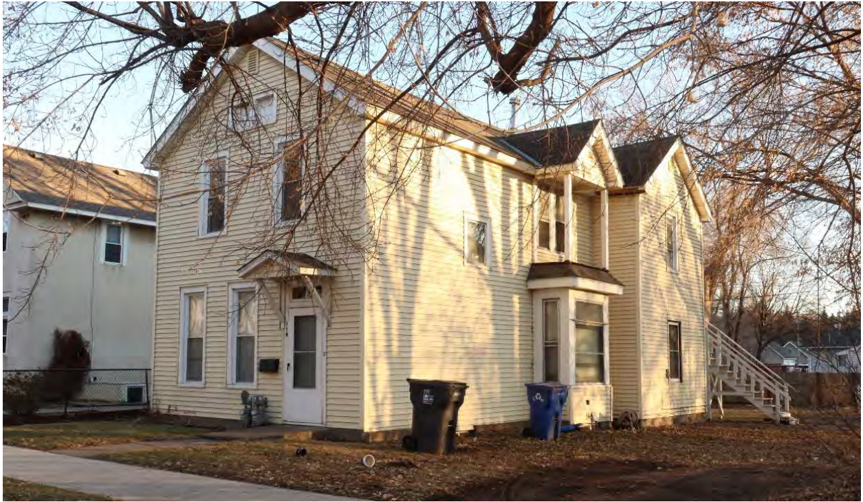
RA-SPC-08959, January 31, 2024, front (north) facade and side (west) elevation, view facing south.
