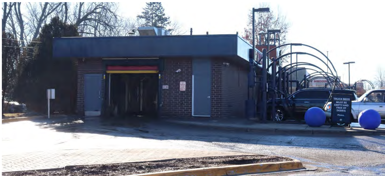
DK-WPC-00086, January 31, 2024, side (north) elevation and front (west) facade, view facing south.
