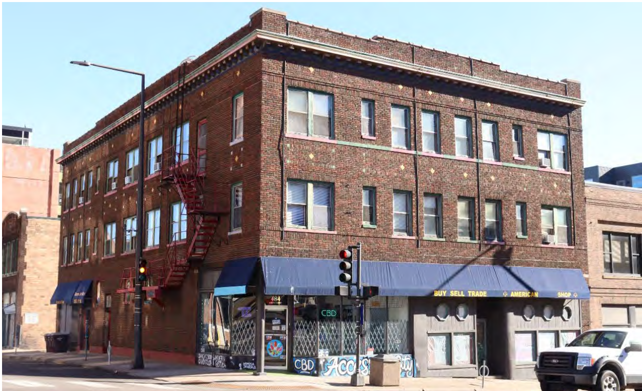
RA-SPC-03173, February 1, 2024, front (west) facade and side (north) elevation, view facing southeast.
