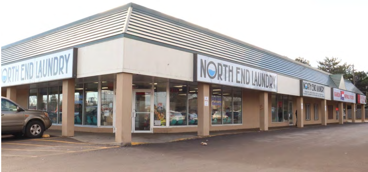
RA-SPC-11892, January 29, 2024, front (east) facade and side (north) elevation, view facing southwest.
