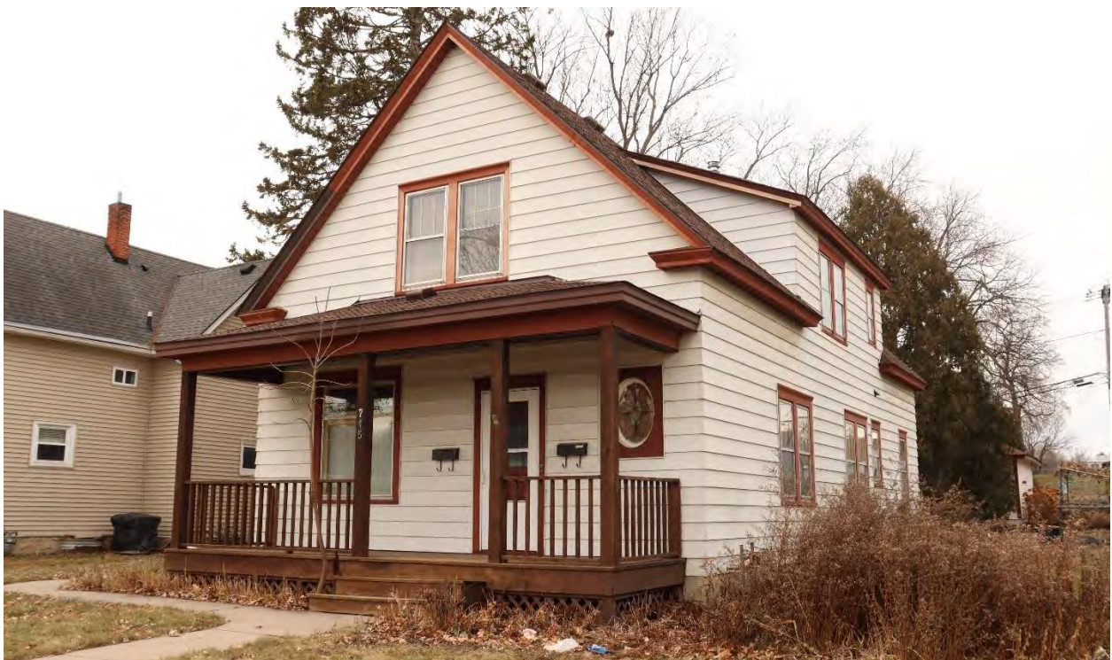
RA-SPC-09004, February 02, 2024, front (east) facade and side (north) elevation, view facing southwest.
