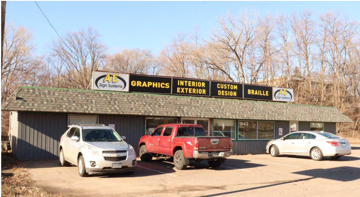
RA-RVC-00060, January 29, 2024, front (east) facade and side (south) elevation, view facing northwest.
