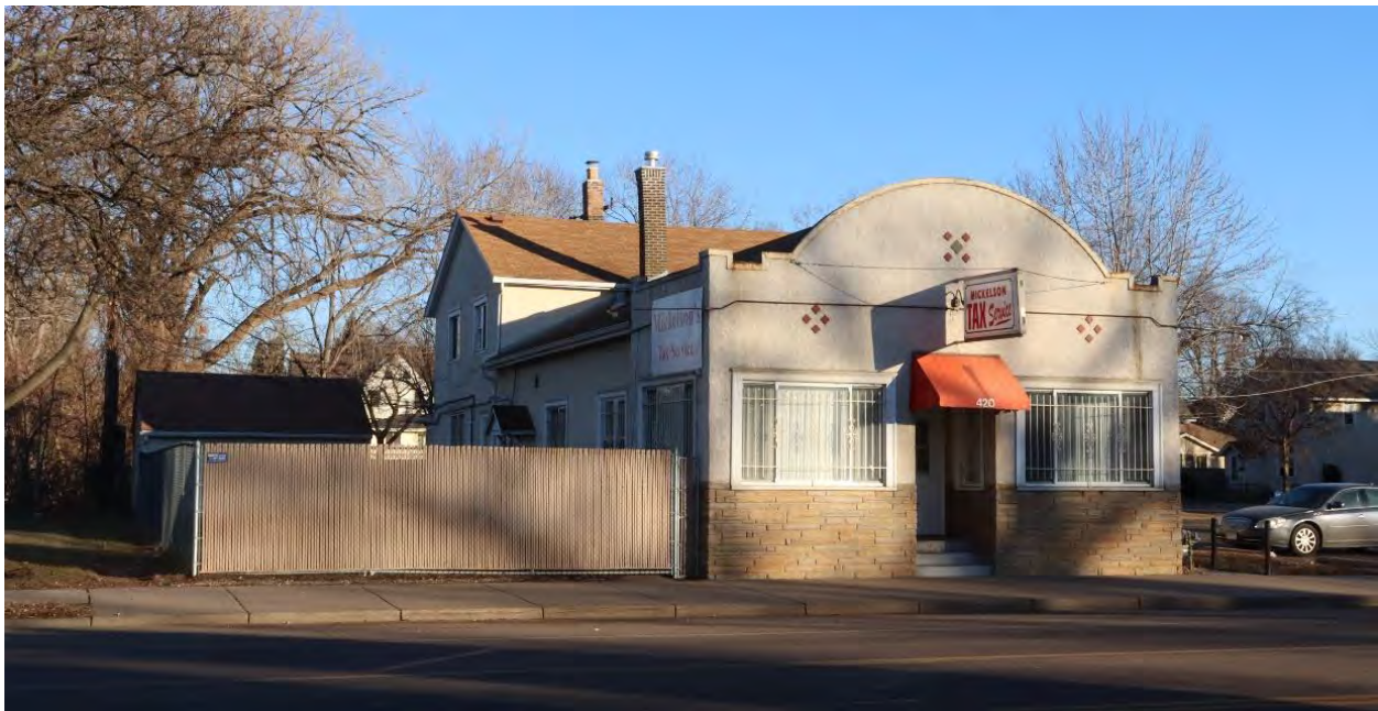
RA-SPC-08968, January 31, 2024, front (west) facade and side (north) elevation, view facing southeast.
