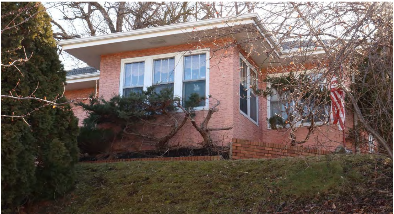
RA-SPC-11908, January 31, 2024, front (north) facade, view facing southeast.
