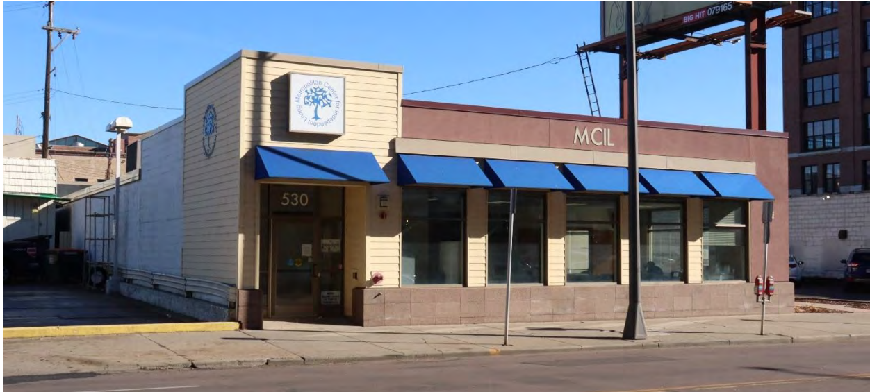
RA-SPC-08962, February 01, 2024, front (southwest) facade and side (northwest) elevation, view facing east.
