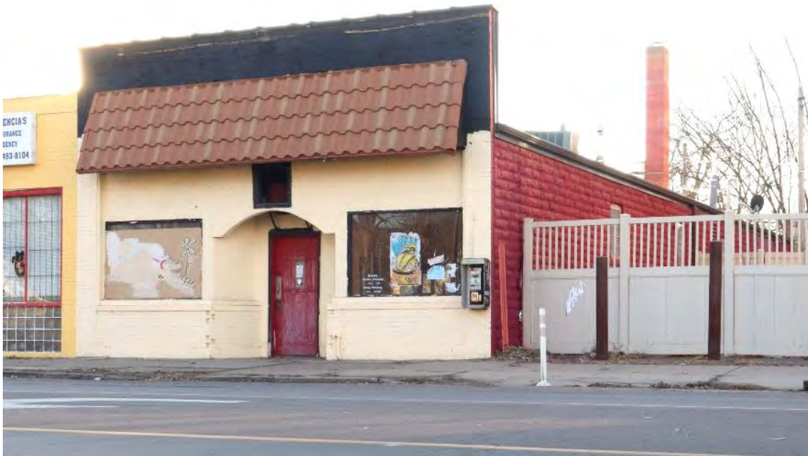
RA-SPC-08969, January 31, 2024, front (east) facade and side (north) elevation, view facing southwest.
