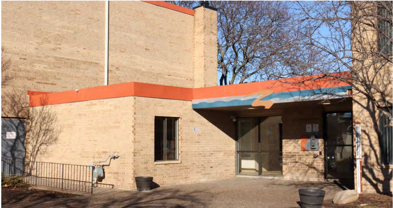
RA-SPC-11925, February 1, 2024, Front (south) facade featuring primary entrance, view facing northwest.
