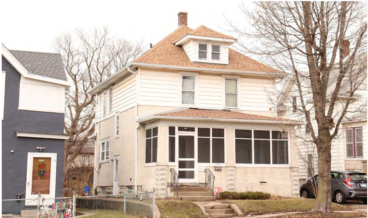
RA-SPC-09013, January 31, 2024, front (west) facade and side (north) elevation, view facing east.
