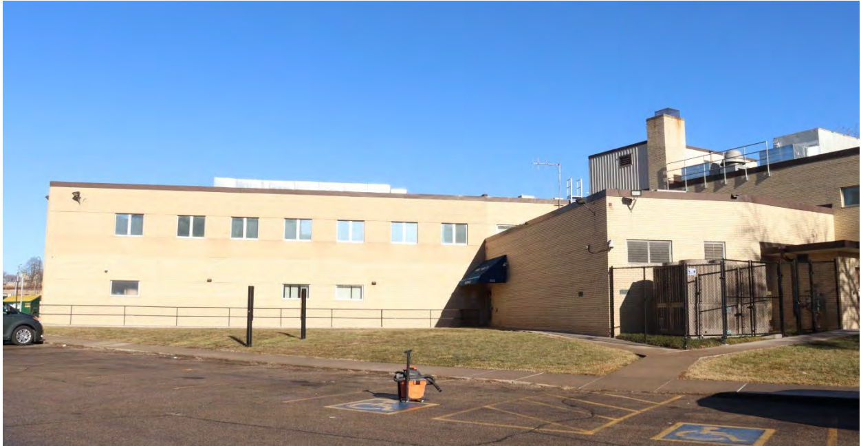
RA-SPC-00556, February 01, 2024, rear (southwest) elevation, view facing north.
