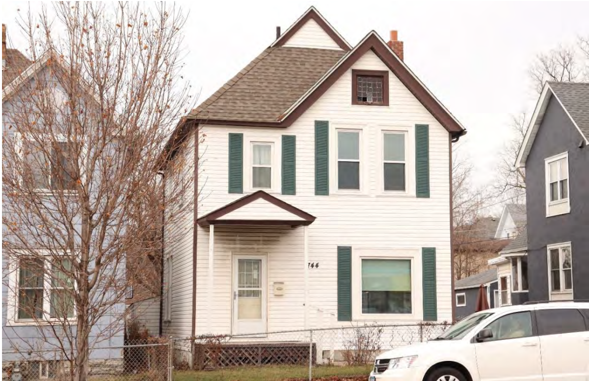
RA-SPC-09010, January 31, 2024, front (west) facade and side (north) elevation, view facing east.
