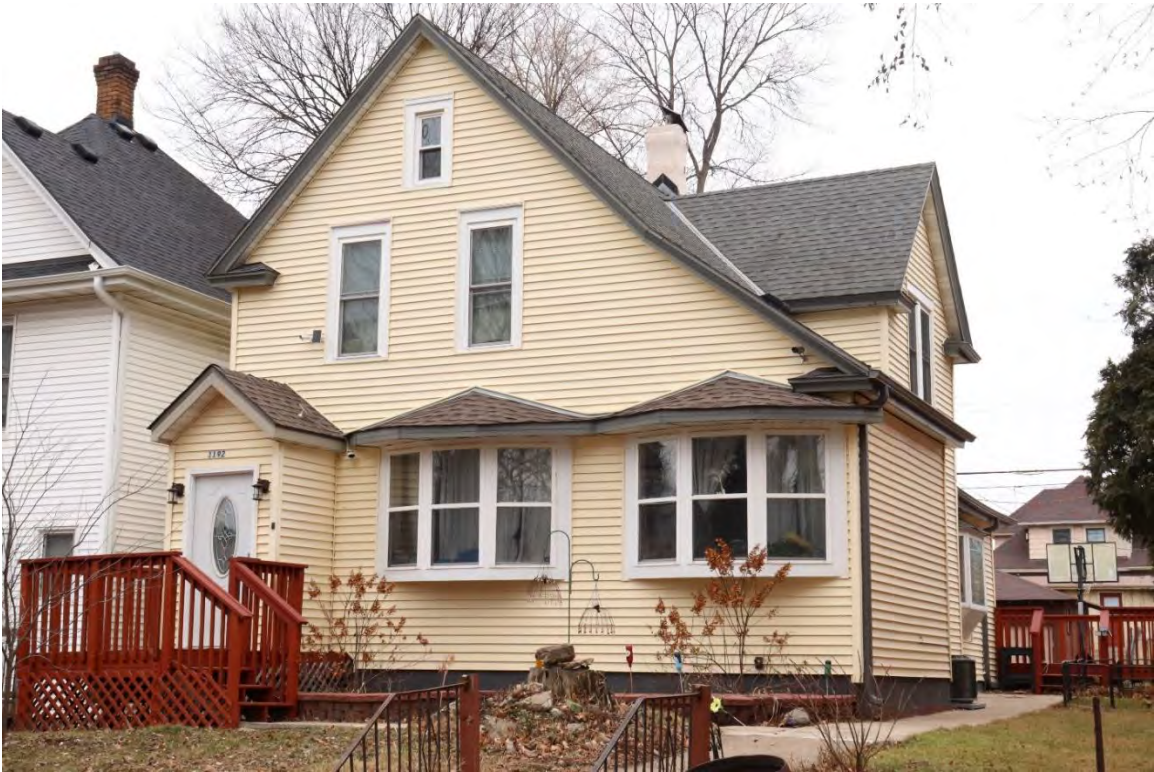
RA-SPC-11900, January 29, 2024, front (west) facade and side (south) elevation, view facing northeast.
