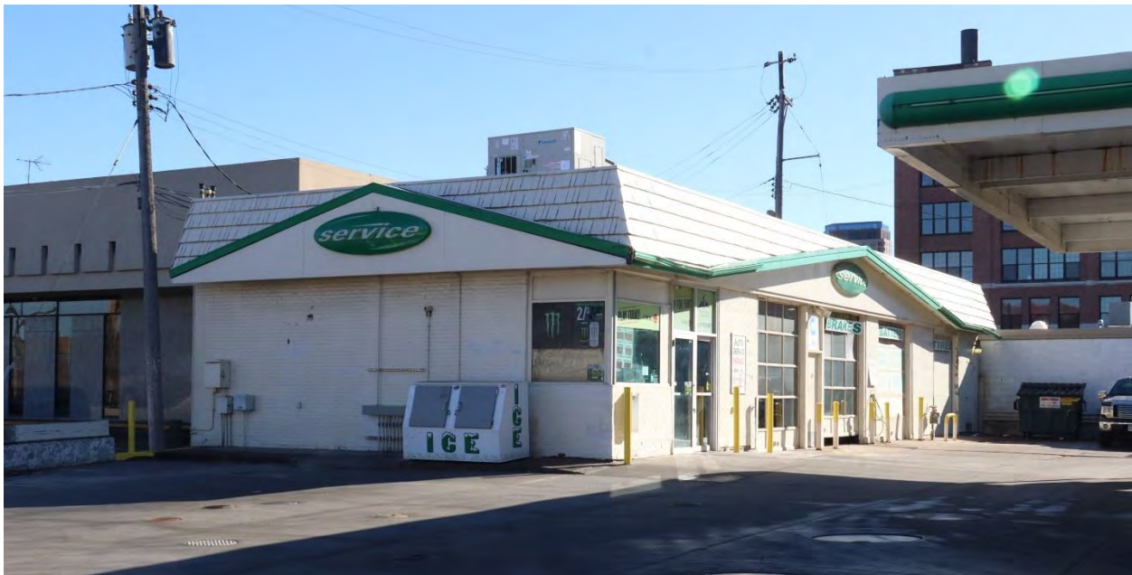
RA-SPC-08963, February 01, 2024, front (southwest) elevation and side (northwest), view facing east.
