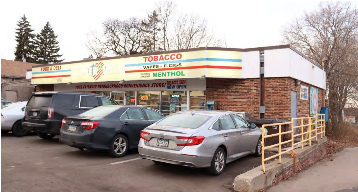
RA-SPC-11941, January 29, 2024, Front (south) facade and side (east) elevation, view facing northeast.
