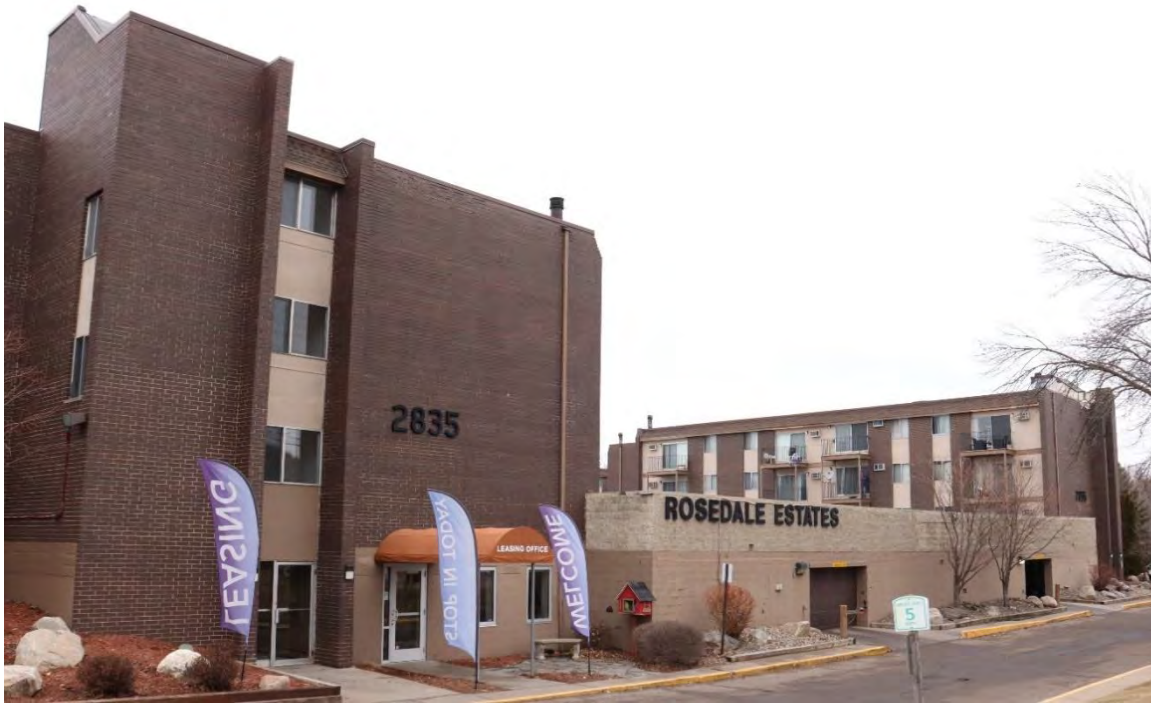
RA-RVC-00065, January 30, 2024, front (east) façade and side (south) elevation, view facing northwest.
