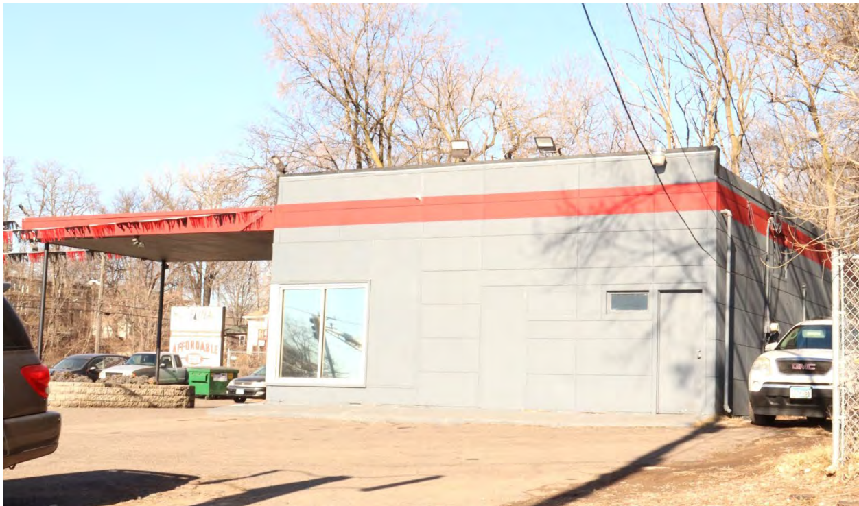
RA-MWC-00358, January 29, 2024, side (south) elevation and rear (east) elevation, view facing northwest.
