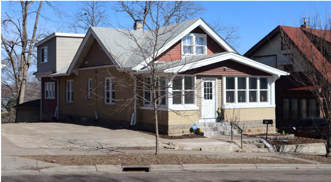
RA-SPC-11918, March 6, 2024, front (south) facade and side (west) elevation, view facing northeast.
