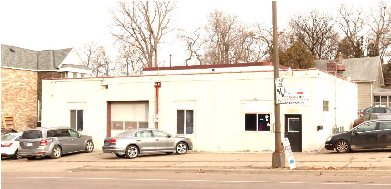
RA-SPEC-09024, February 02, 2024, front (west) facade and side (south) elevation, view facing northeast.
