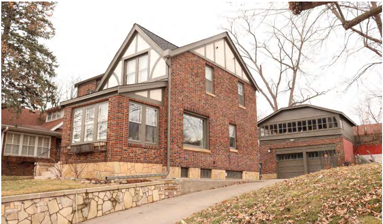
RA-SPC-08999, January 29, 2024, front (east) facade, side (north) elevation, and garage, view facing southwest.
