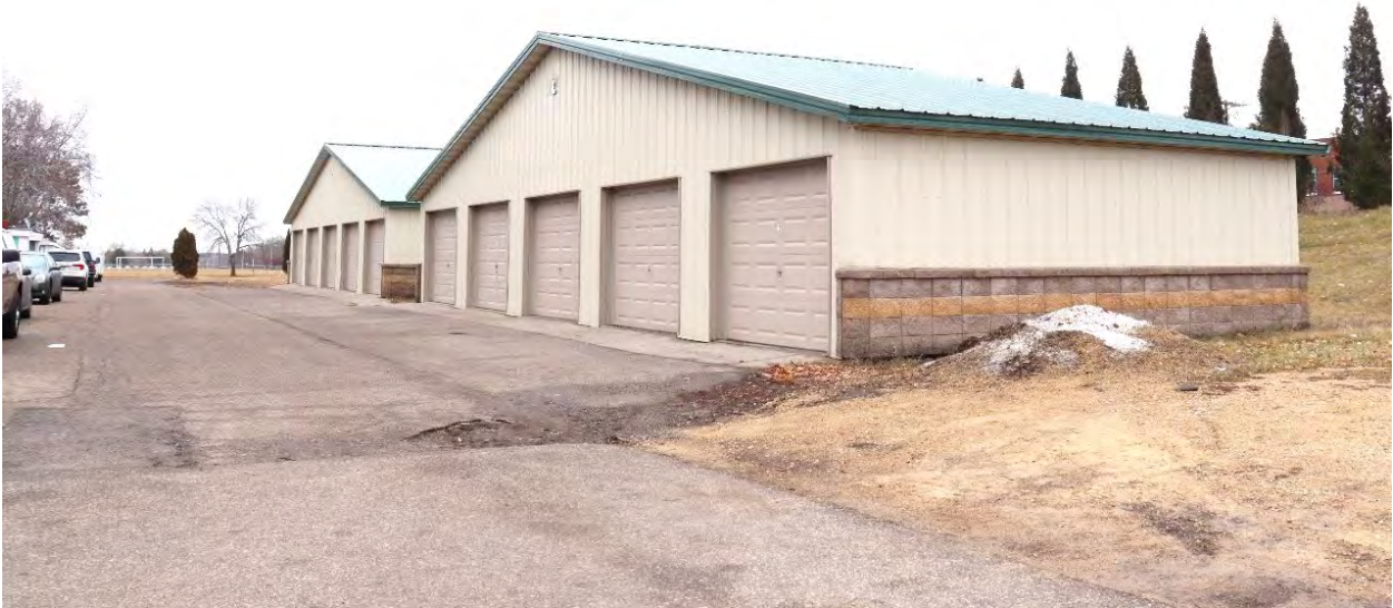
RA-LCC-00083, January 30, 2024, view from Rice Street of two additional non-historic-age, multi-bay garages near southern end of mobile home park, view facing southeast.
