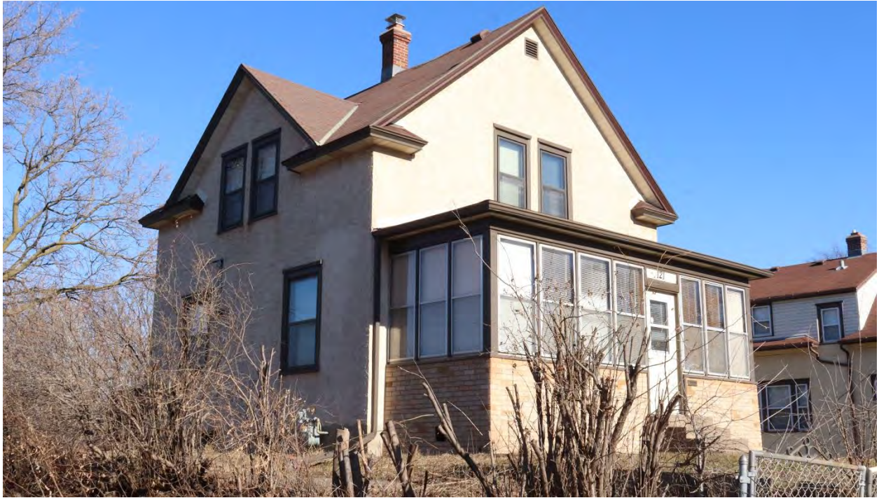
RA-SPC-11906, January 31, 2024, front (south) facade and side (west) elevation, view facing northeast.
