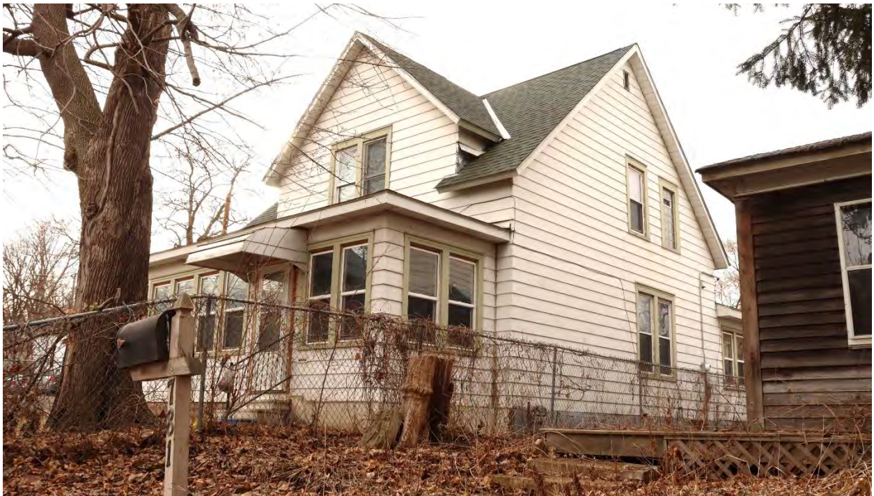
RA-SPC-09025, February 02, 2024, front (east) facade and side (north) elevation, view facing southwest.
