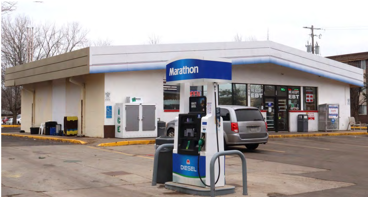
RA-RVC-00064, January 30, 2024, front (west) facade, side (north) elevation, and diesel pump, view facing southeast.
