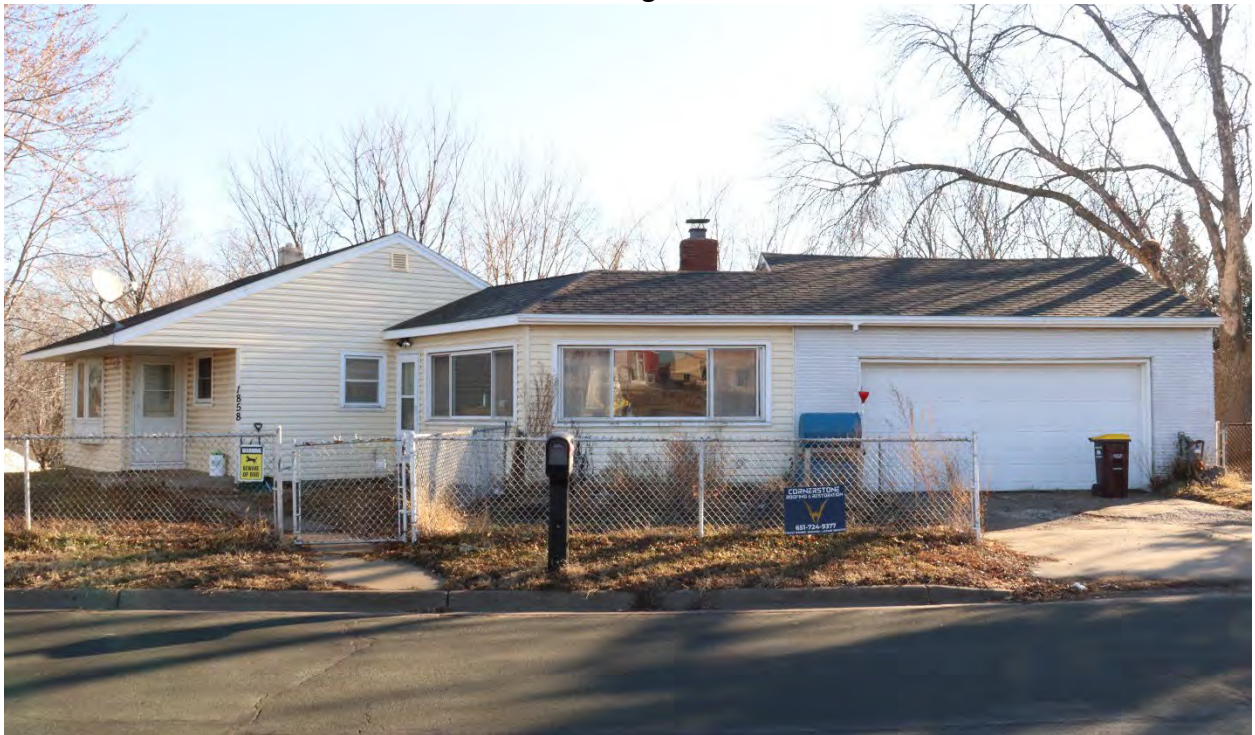
DK-WPC-00083, January 31, 2024, front (southwest) elevation and side (southeast) elevation, and garage attachment, view facing east.
