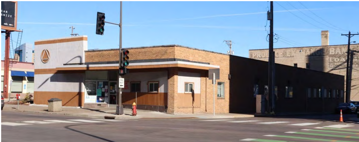
RA-SPC-08961, February 01, 2024, front (southwest) and side (southeast) elevation, view facing north.
