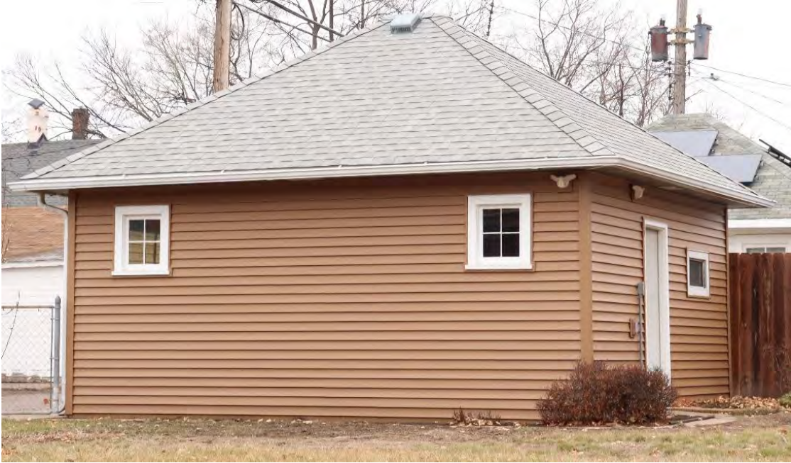
RA-SPC-11898, January 29, 2024, detached garage to the rear (west) of the home, view facing southwest.
