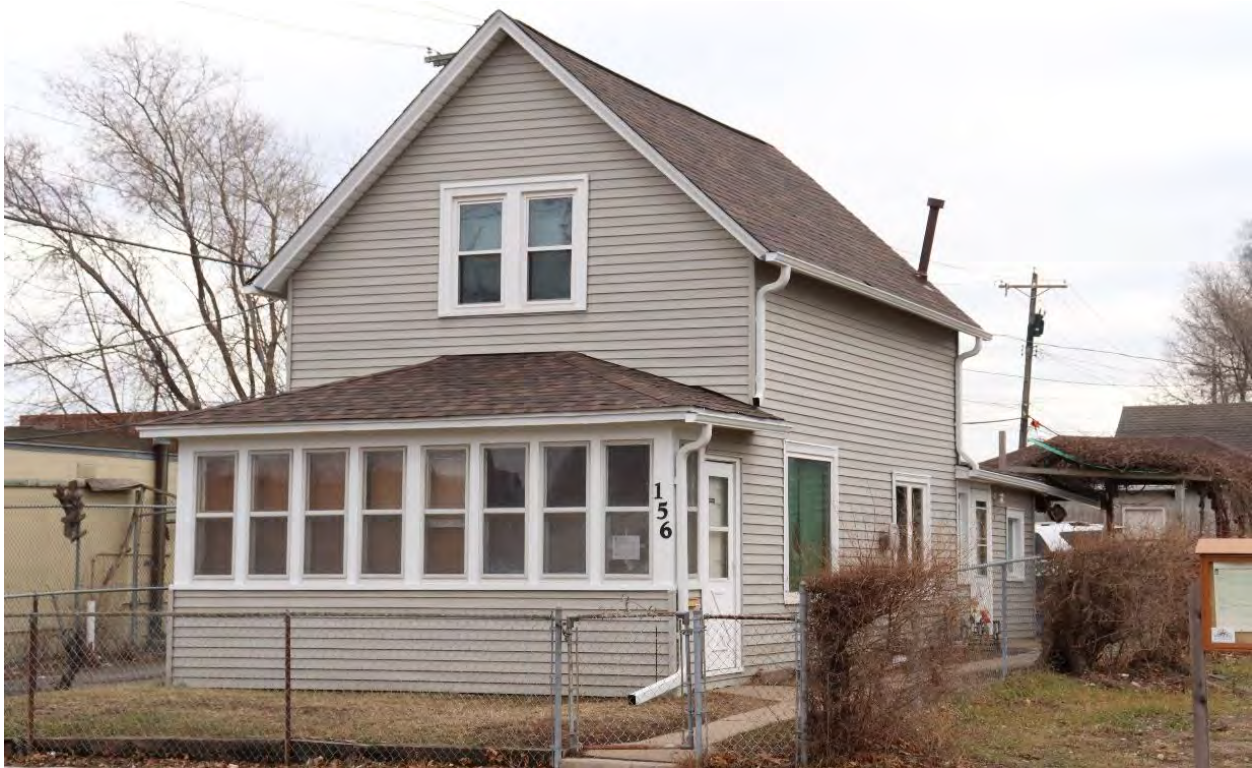
RA-SPC-11923, January 30, 2024, Front (north) facade and side (west) elevation, view facing southeast.
