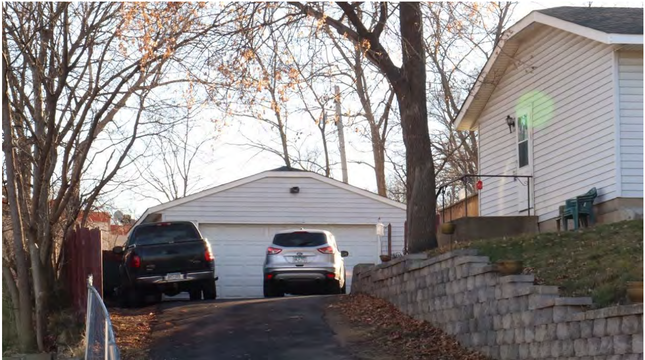
RA-SPC-11922, January 31, 2024, Garage and side (east) elevation of house, view facing southwest.
