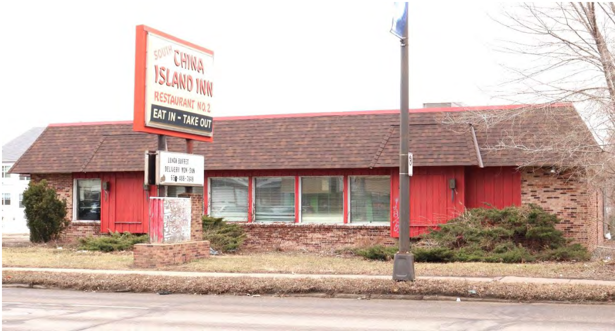
RA-SPC-11915, January 29, 2024, front (west) facade, side (south) elevation, and sign to the west of the building, view facing northeast.
