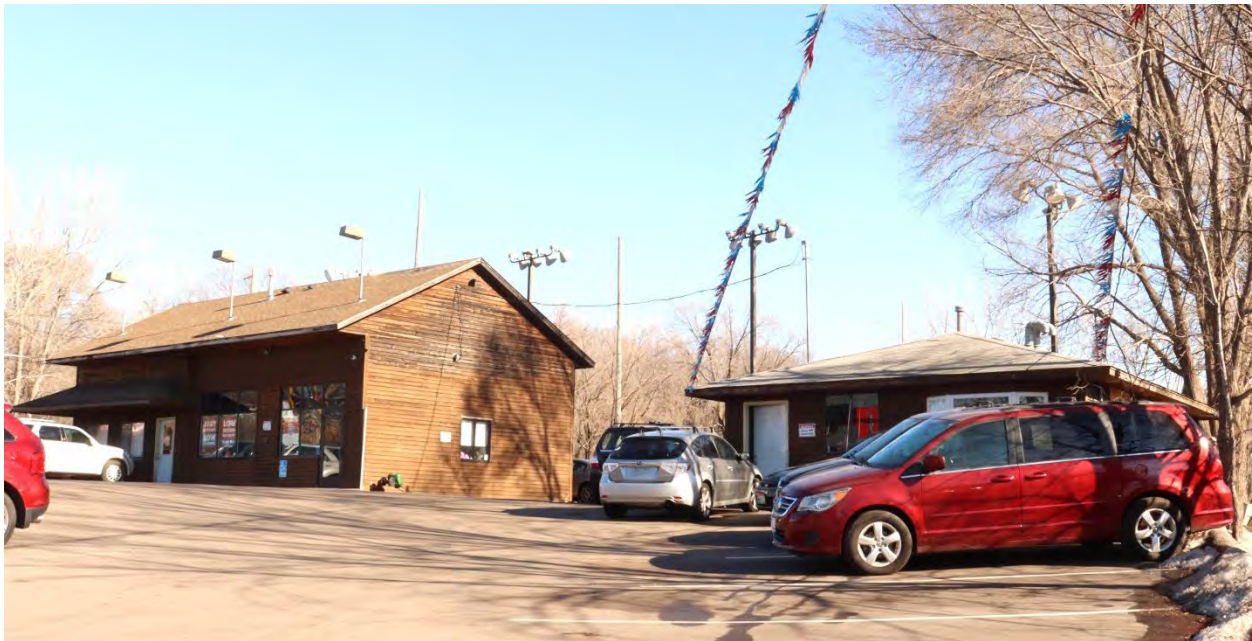
RA-MWC-00357, January 29, 2024, front (west) and side (south) elevation of the primary building (left) and front (west) facade of the non-historic-age secondary building (right) view facing northeast.
