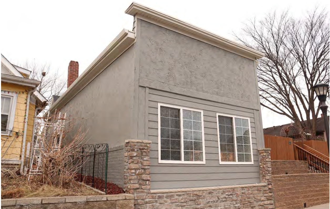
RA-SPC-11897, January 31, 2024, front (south) facade of the former storefront addition and side (west) elevation, view facing northeast.
