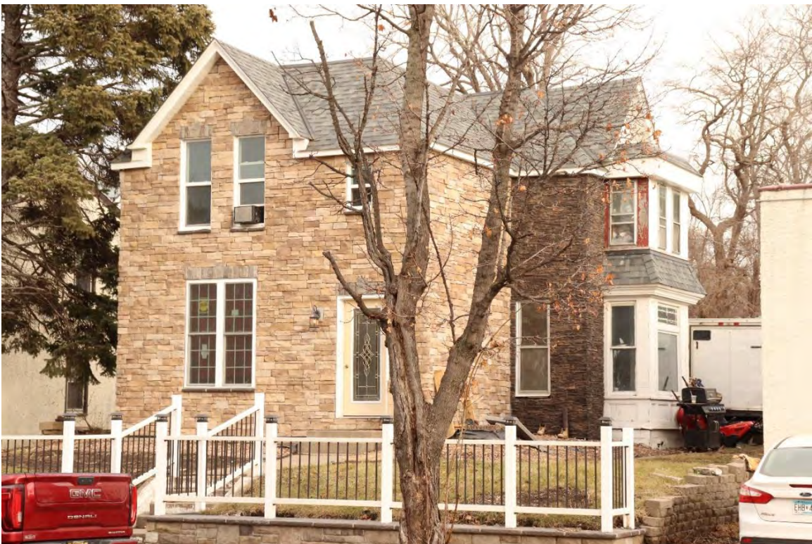
RA-SPC-09023, February 02, 2024, front (west) facade and side (south) elevation, view facing northeast.
