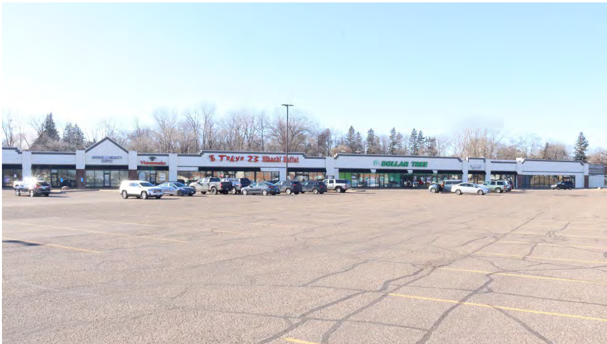
DK-WPC-00082, January 31, 2024, Front (northeast) facade of northwest ell, view facing west.
