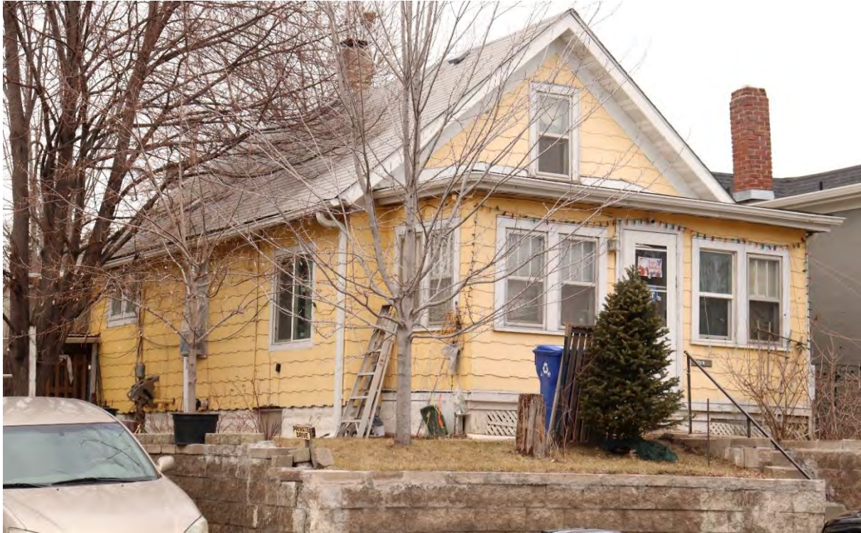
RA-SPC-11895, January 31, 2024, front (south) facade and side (west) elevation, view facing northeast.
