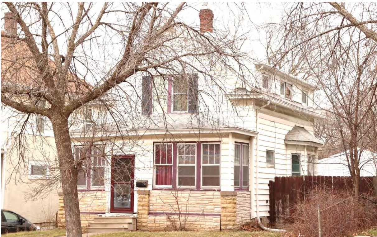
RA-SPC-09015, January 31, 2024, front (west) facade and side (south) elevation, view facing northeast.
