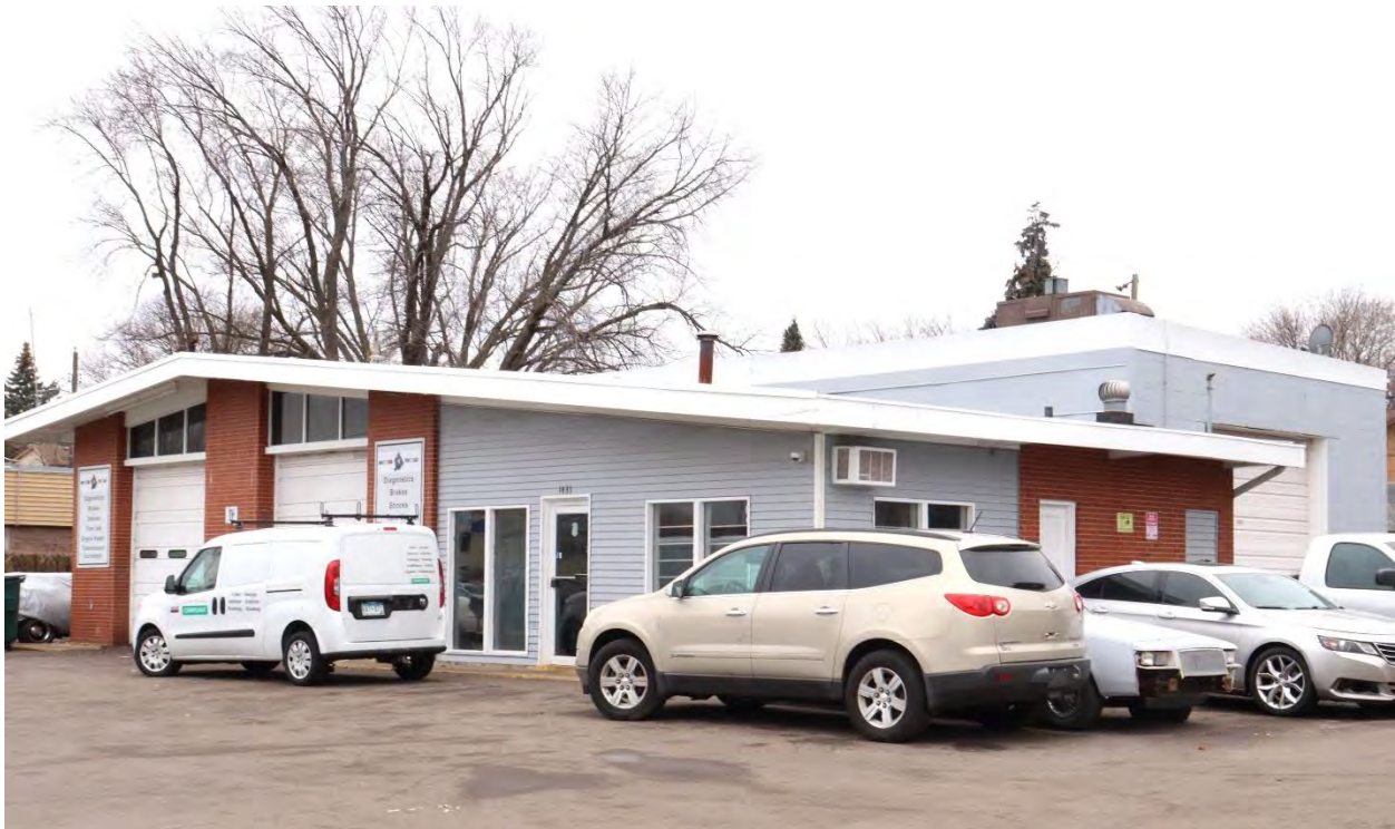
RA-SPC-11916, January 30, 2024, front (east) facade, side (north) elevation, and rear (west) addition, view facing southwest.
