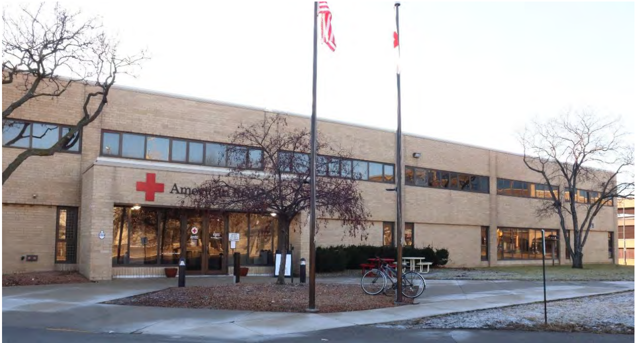
RA-SPC-11893, February 1, 2024, front (northwest) facade with primary entrance, view facing southeast.
