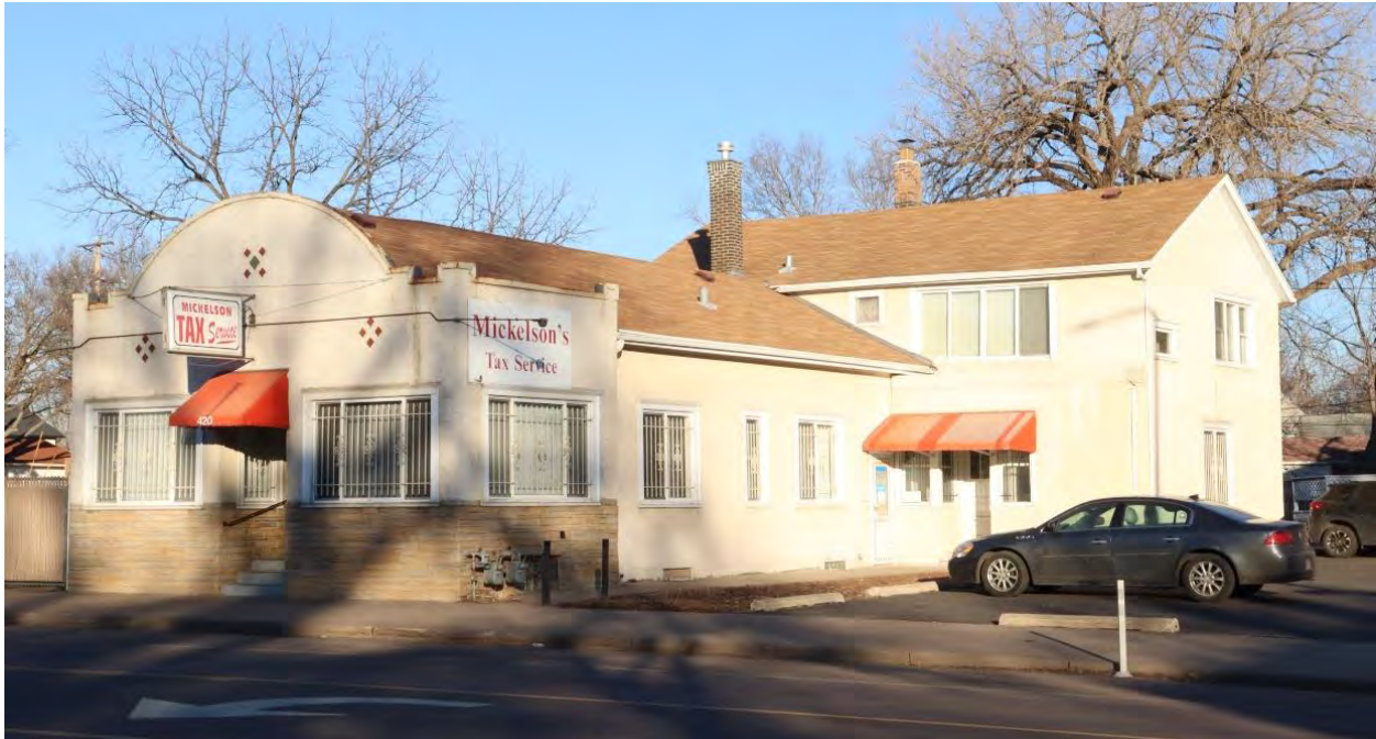
RA-SPC-08968, January 31, 2024, front (west) facade and side (south) elevation, view facing northeast.
