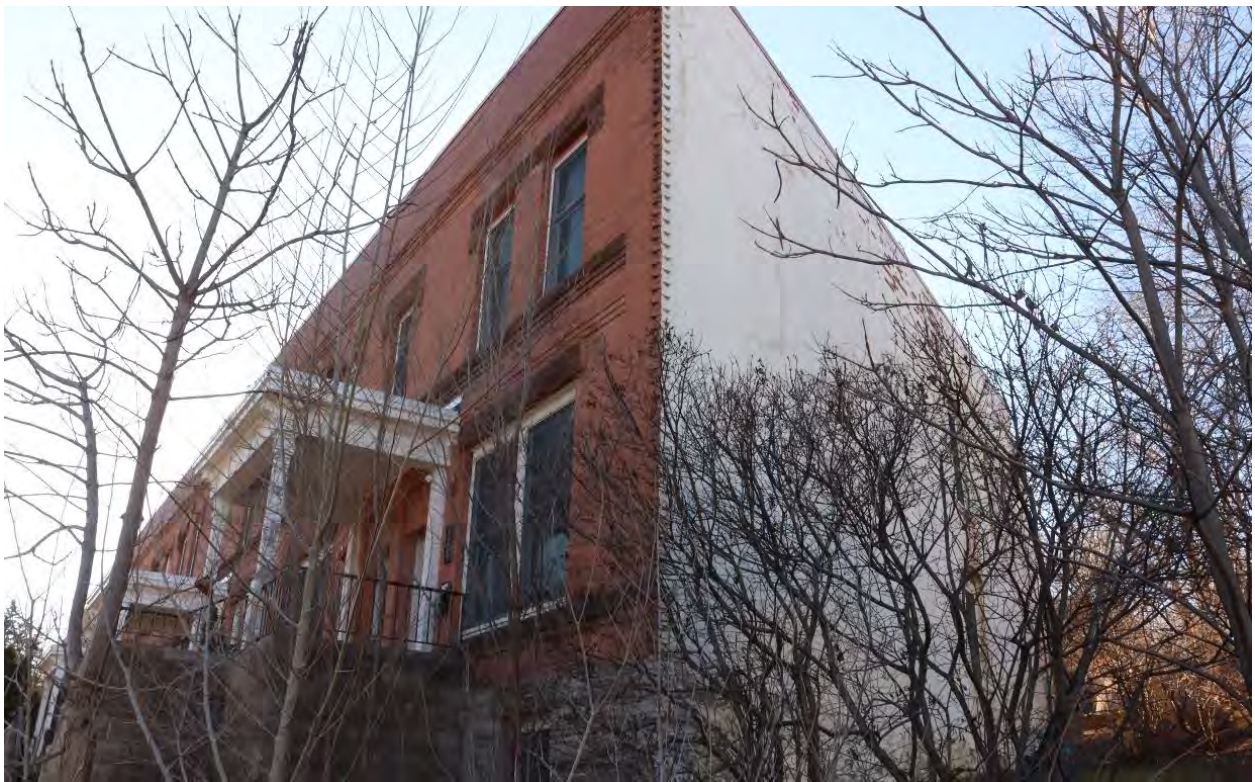
RA-SPC-03525, January 31, 2024, front (east) facade and side (north) elevation, featuring acute northeast corner of the building, view facing southwest.
