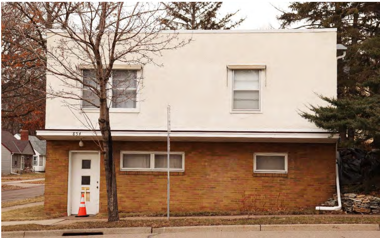
RA-SPC-09037, January 29, 2024, front (west) facade, view facing east.
