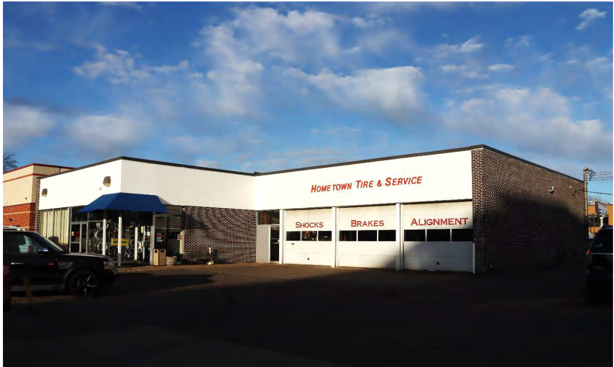
DK-WPC-00091, March 5, 2024, front (west) facade and side (south) elevation, view facing northeast.
