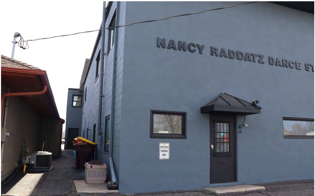
DK-WPC-00093, March 6, 2024, Front (north) facade and side (east) elevation featuring addition, view facing southwest.
