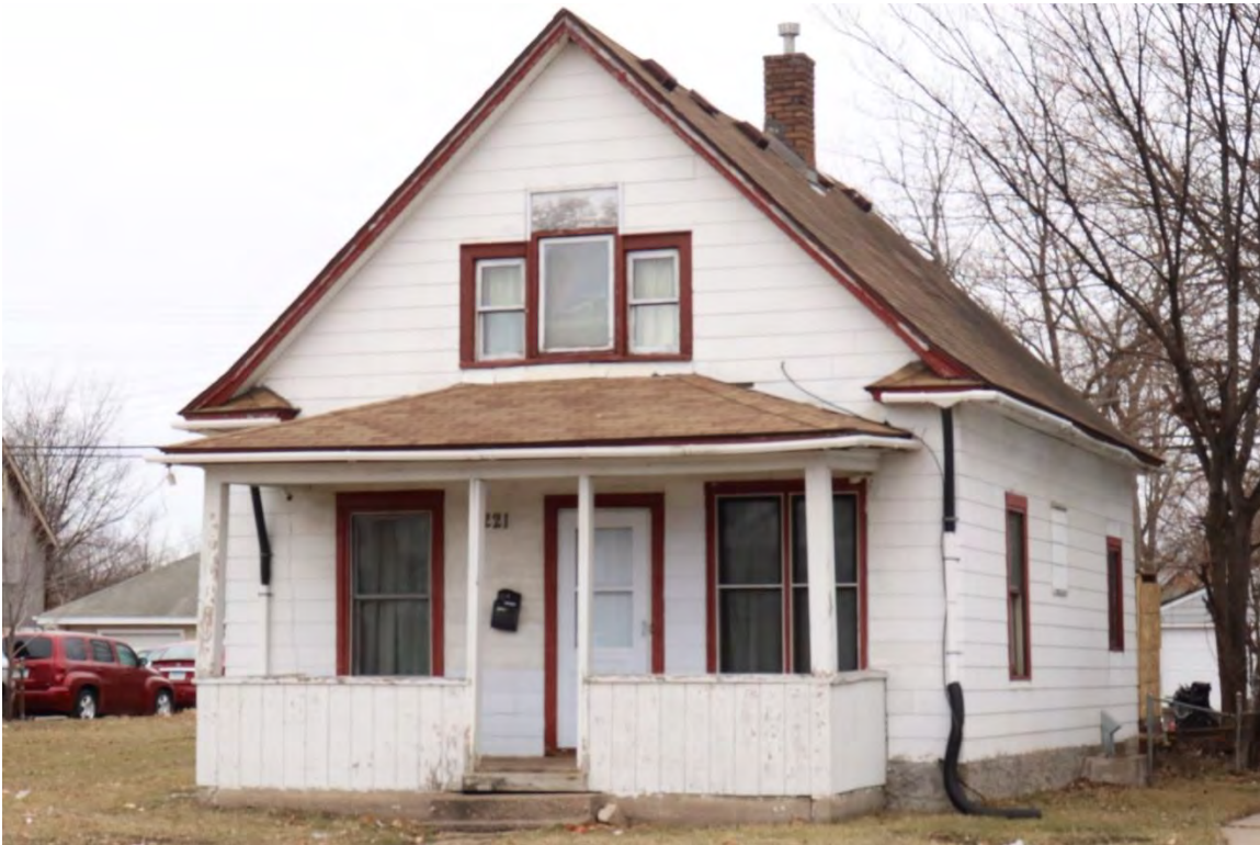
RA-SPC-11909, January 30, 2024, front (east) facade and side (south) elevation, view facing northwest.
