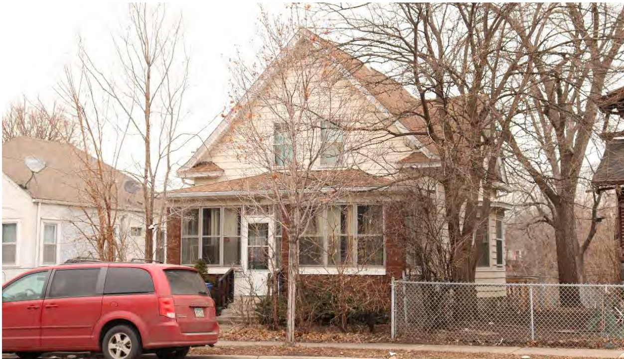
RA-SPC-08997, January 29, 2024, front (west) facade and side (south), view facing northeast.
