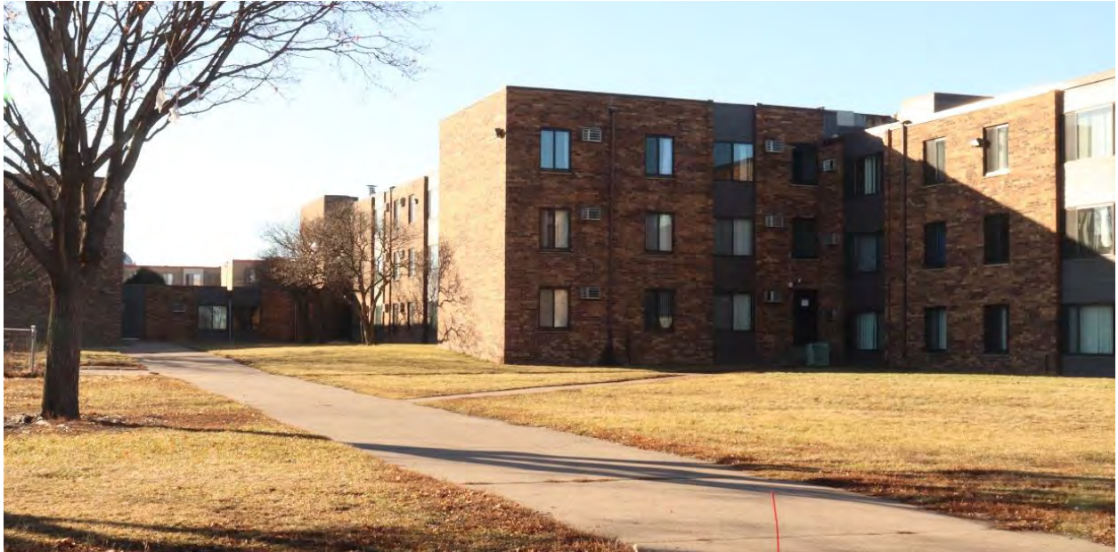
RA-SPC-11929, February 1, 2024, Side (east) elevation of northernmost building mass, featuring one-story portion with administration offices, view facing southwest.
