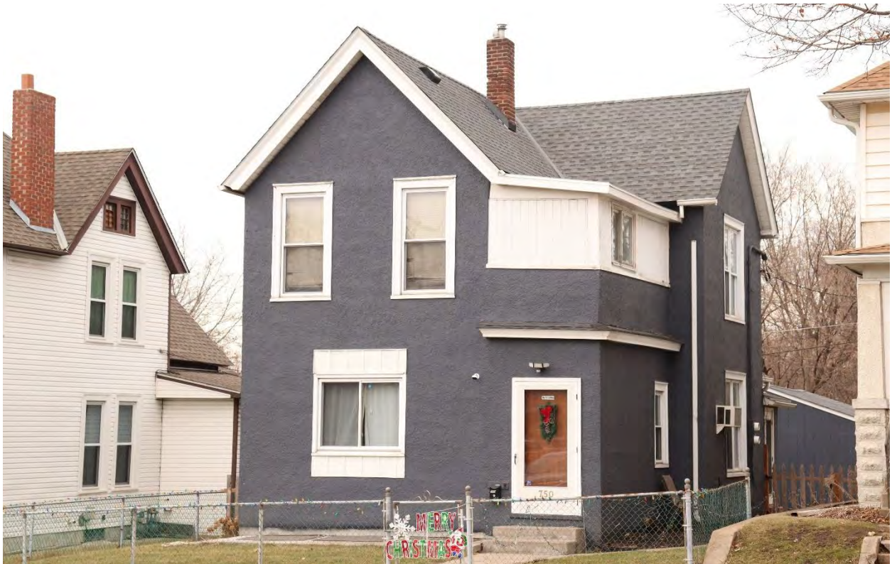
RA-SPC-09012, January 31, 2024, front (west) facade and side (south) elevation, view facing northeast.
