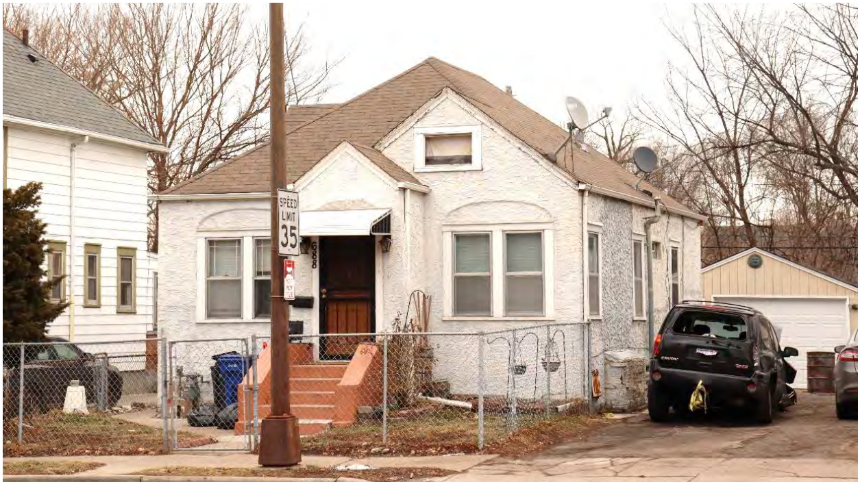
RA-SPC-08996, January 29, 2024, front (west) facade and side (south) elevation featuring garage, view facing northwest.
