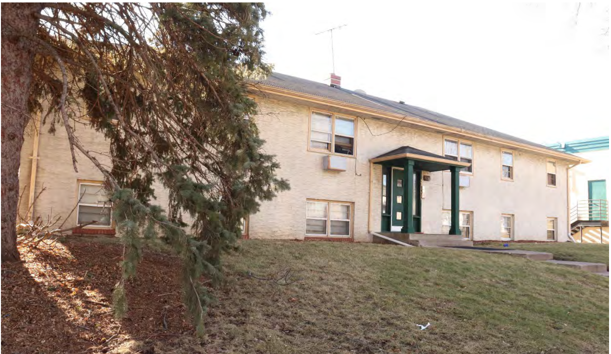
DK-WPC-00096, January 31, 2024, front (north) facade and side (east) elevation, view facing southwest.
