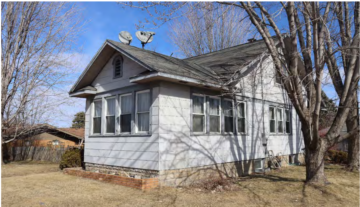
DK-WPC-00084, March 6, 2024, Front (west) facade and side (south) elevation, view facing northeast.
