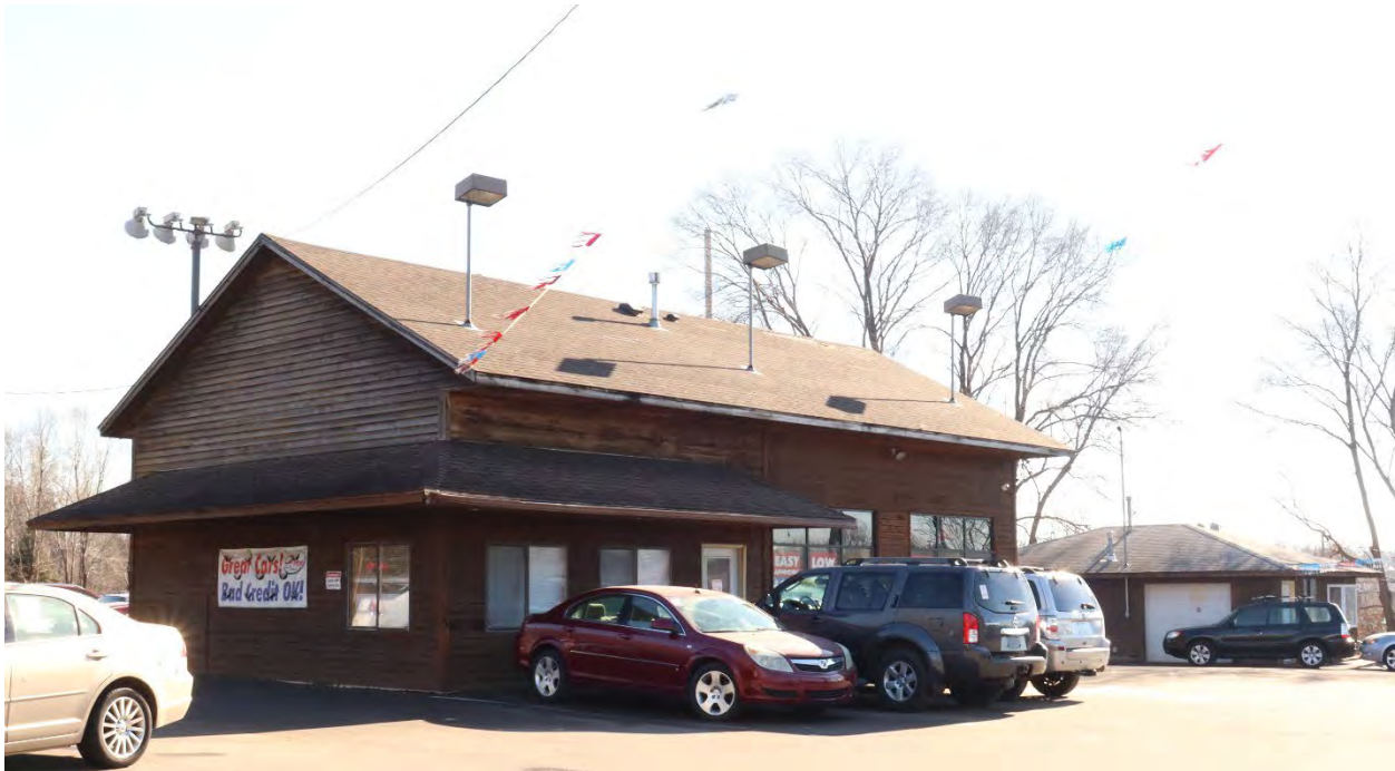
RA-MWC-00357, January 29, 2024, front (west) facade and side (north) elevation of the primary building (left), and front (west) facade and side (north) elevation of the non-historic-age secondary building (right), view facing southeast.
