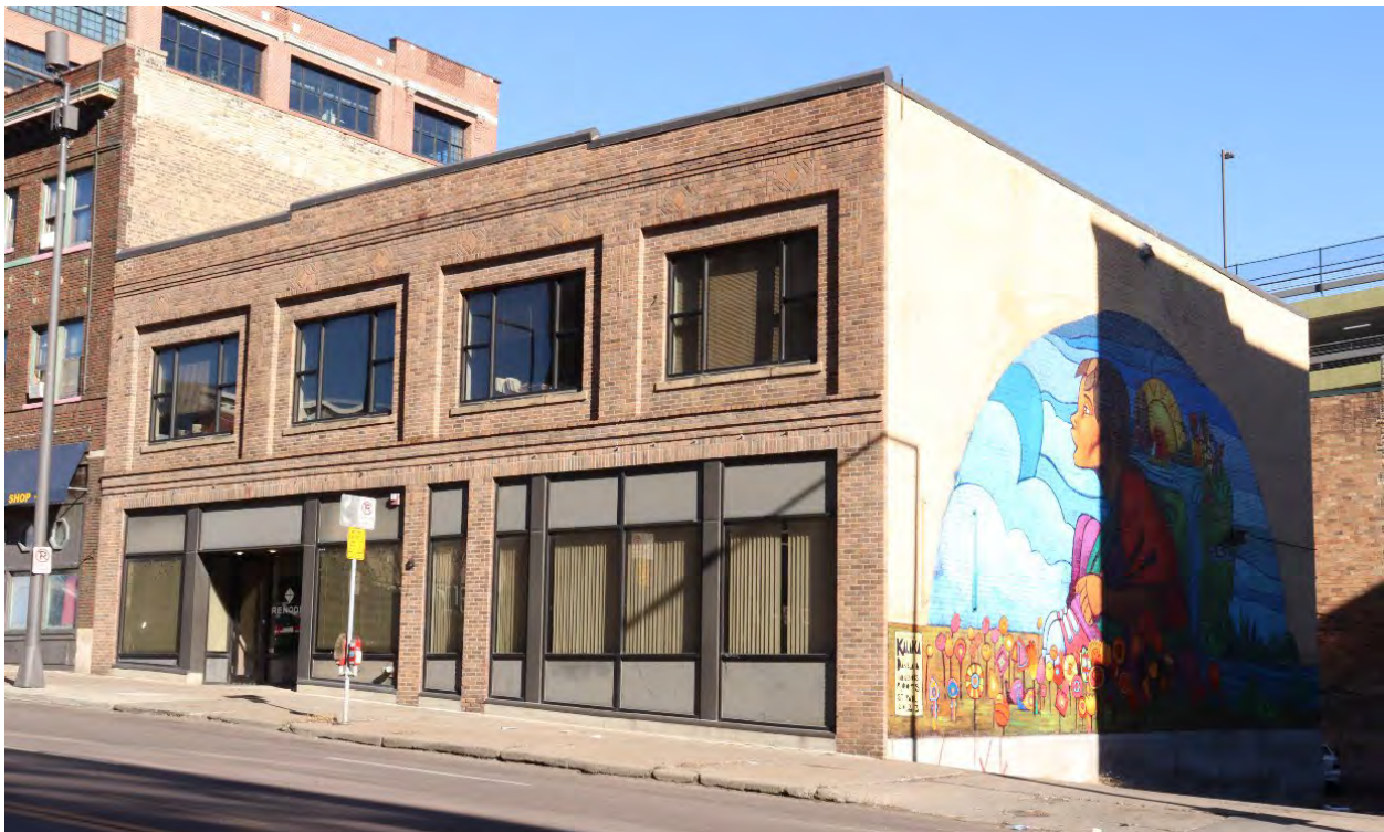
RA-SPC-03172, February 1, 2024, front (west) facade and side (south) elevation with ca. 2024 mural, view facing northeast.
