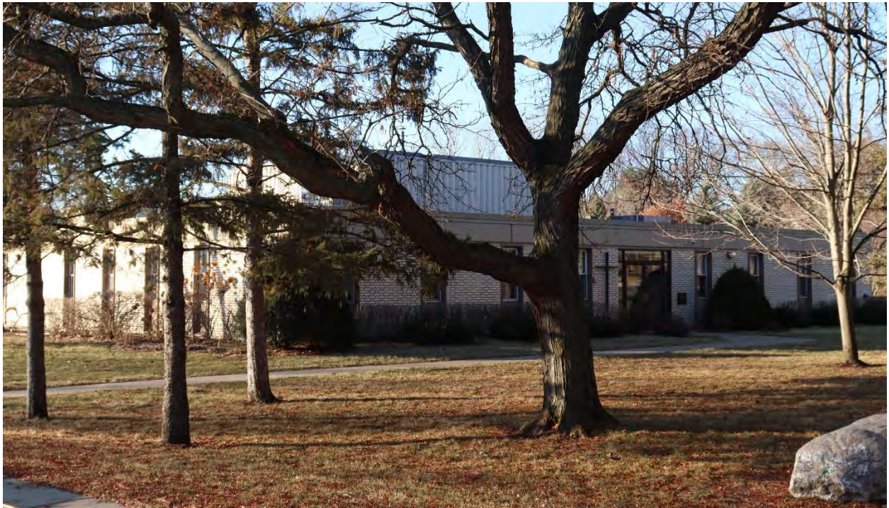
DK-WPC-00081, January 31, 2023, front (north) facade of main block, view facing southwest.
