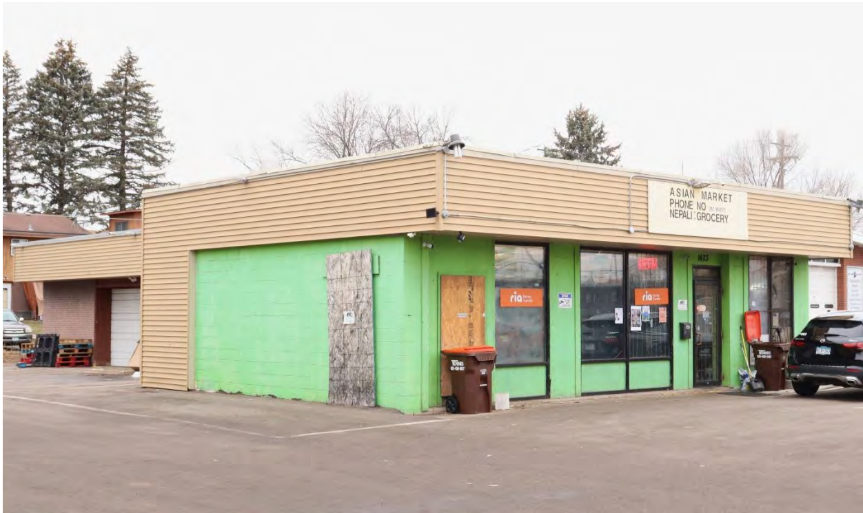
RA-SPC-11914, January 30, 2024, front (east) facade and side (north) elevation, view facing southwest.
