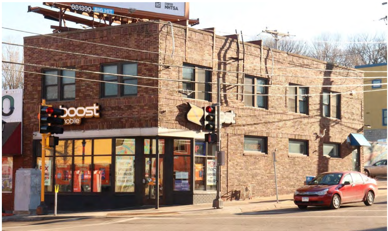
RA-SPC-11926, January 31, 2024, side (west) elevation and front (north) facade, view facing southeast.
