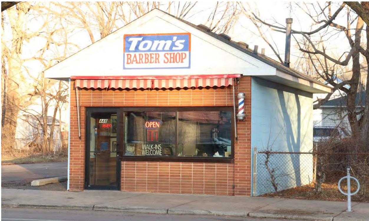
RA-SPC-08971, January 31, 2024, front (west) facade and side (south) elevation, view facing northeast.
