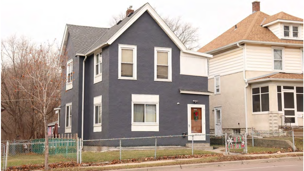
RA-SPC-09012, January 31, 2024, front (west) facade and side (north) elevation, view facing east.
