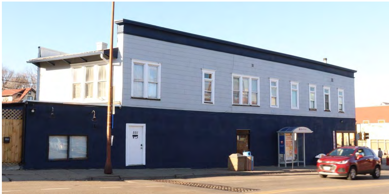
RA-SPC-03524, January 31, 2024, side (east) elevation and rear addition, view facing northwest.
