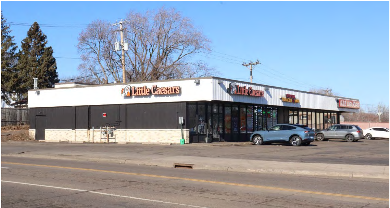
DK-WPC-00089, January 31, 2024, front (east) facade and side (south) elevation, view facing northwest.
