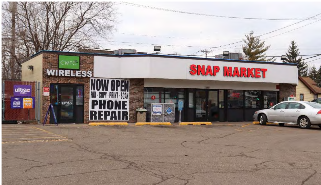
RA-SPC-11938, January 30, 2024, Front (east) facade and side (south) elevation, view facing northwest.
