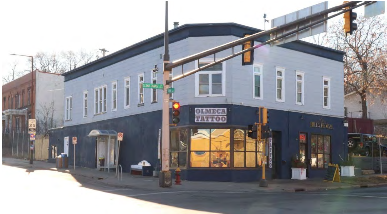
RA-SPC-03524, January 31, 2024, front (north) facade and side (east) elevation featuring canted corner, view facing southwest.
