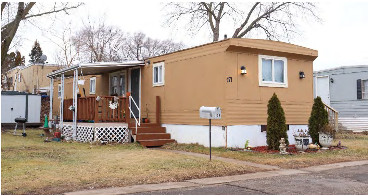
RA-LCC-00083, January 30, 2024, representative example of historic-age mobile home with replacement vinyl windows, porch addition, and awning, view facing northwest.
