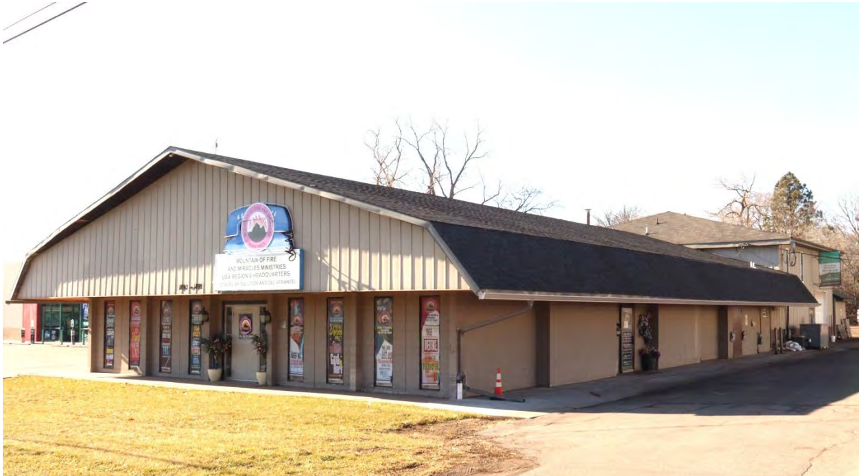
RA-RVC-00058, January 29, 2024, front (east) facade and side (north) elevation, view facing southwest.
