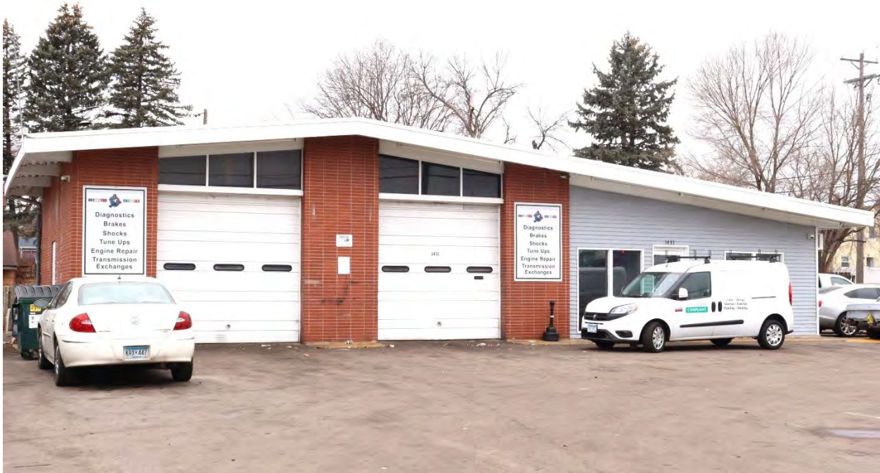
RA-SPC-11916, January 30, 2024, front (east) facade and side (south) elevation, view facing northwest.
