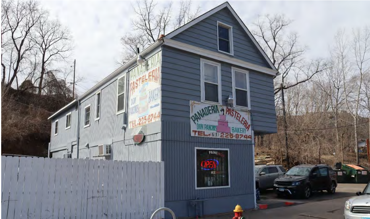
RA-SPC-11913, March 06, 2024, front (northeast) facade and side (southeast) elevation, view facing west.
