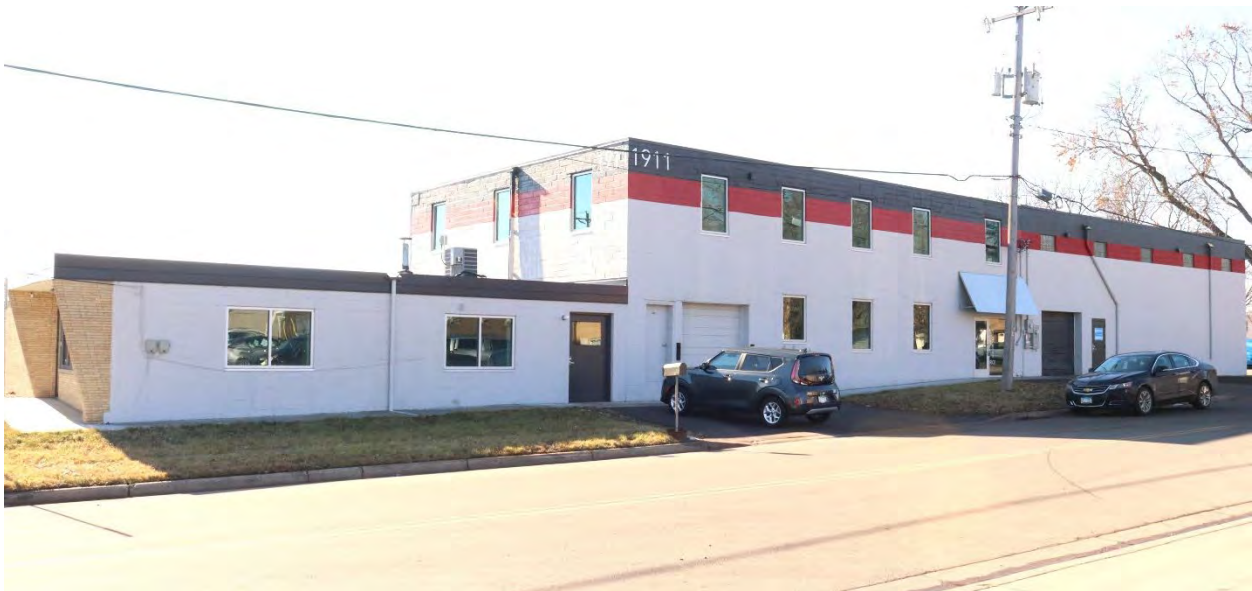
RA-RVC-00016, January 29, 2024, front (north) facade and side (west) elevation, view facing southeast.
