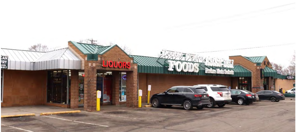
RA-SPC-11568, January 30, 2024, front (south) facade of the eastern portion, view facing northeast.
