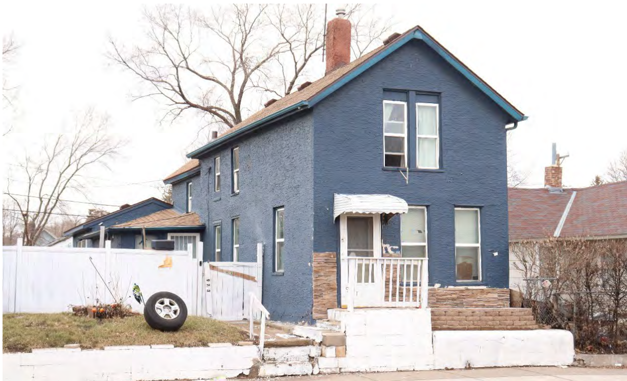
RA-SPC-03083, January 30, 2024, front (east) facade and side (south) elevation, view facing northwest.
