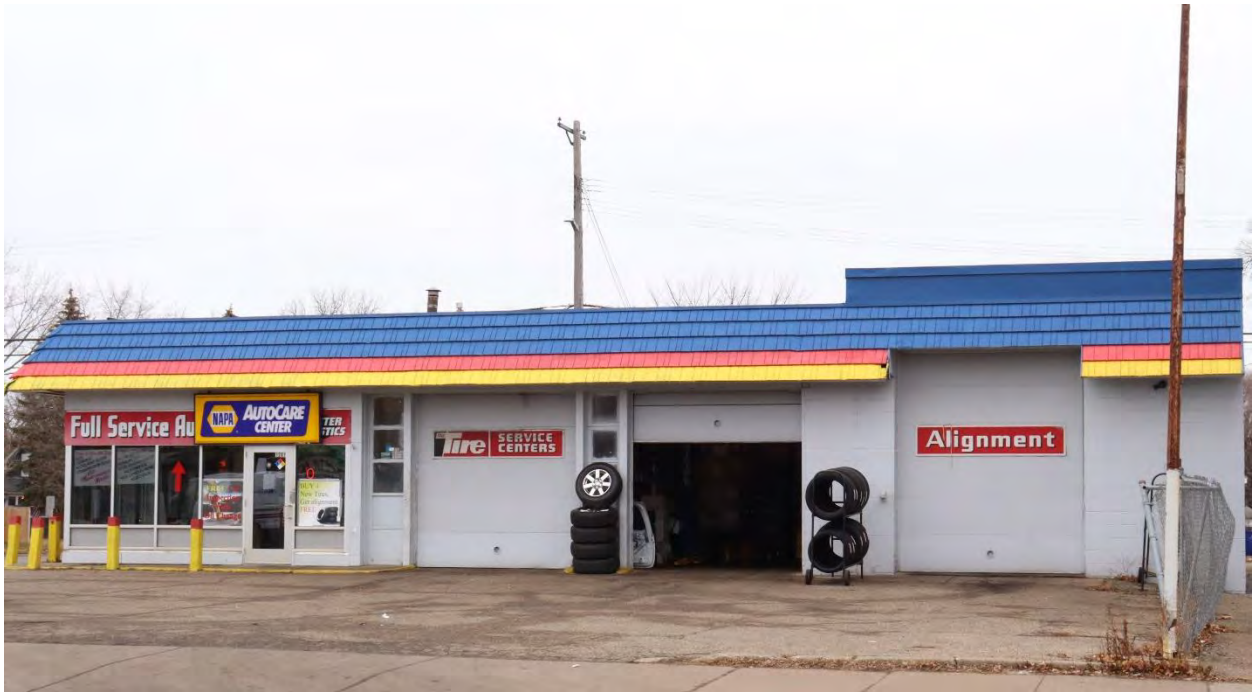
RA-SPC-11903, January 30, 2024, front (east) facade, view facing southwest.
