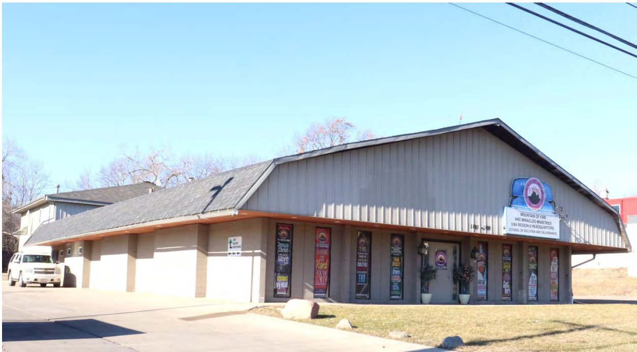
RA-RVC-00058, January 29, 2024, front (east) facade and side (south) elevation, view facing northwest.
