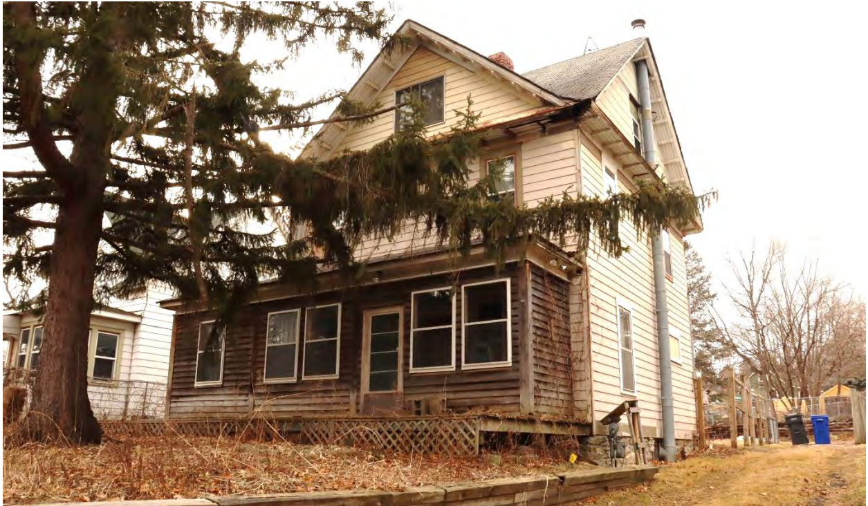
RA-SPC-09022, February 02, 2024, front (east) facade and side (south) elevation, view facing northwest.
