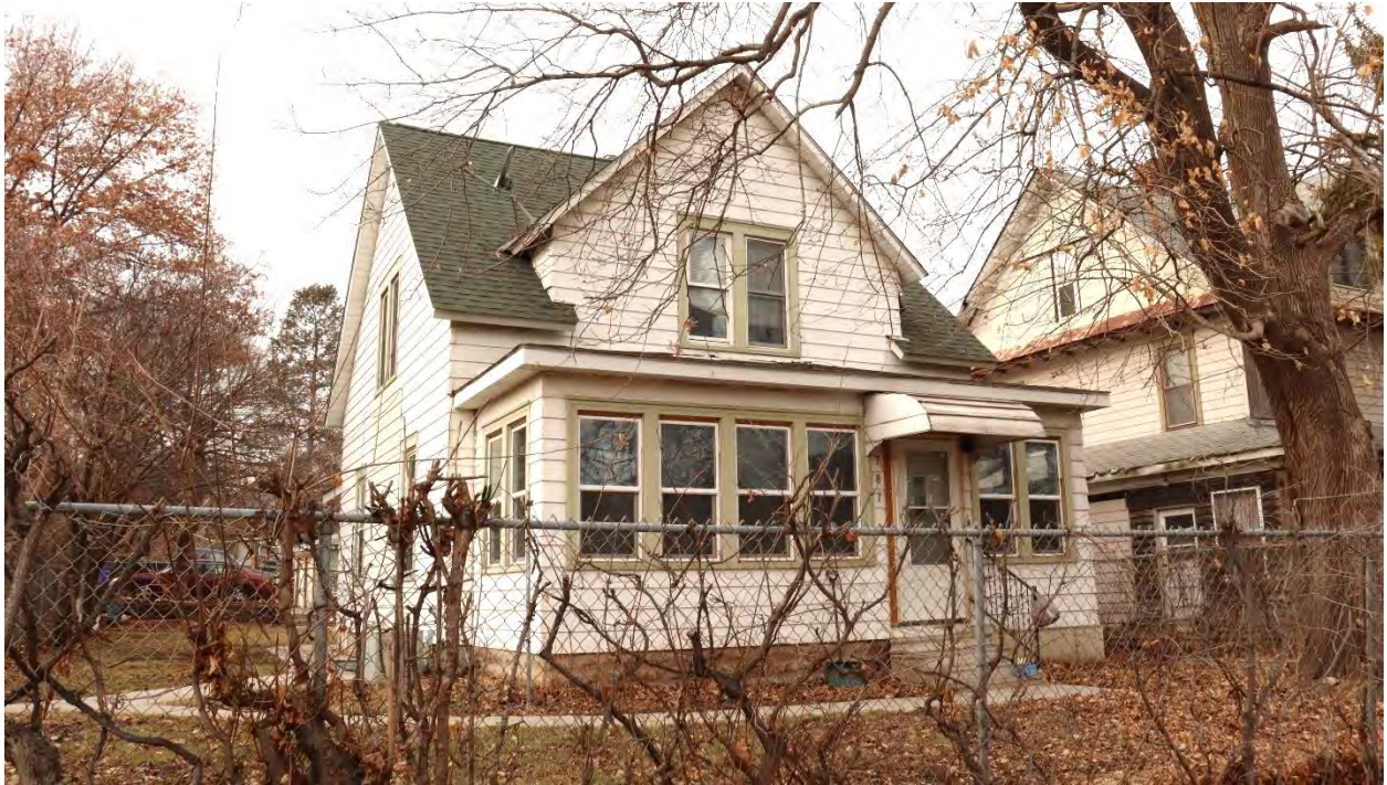
RA-SPC-09025, February 02, 2024, front (east) facade and side (south) elevation, view facing northwest.
