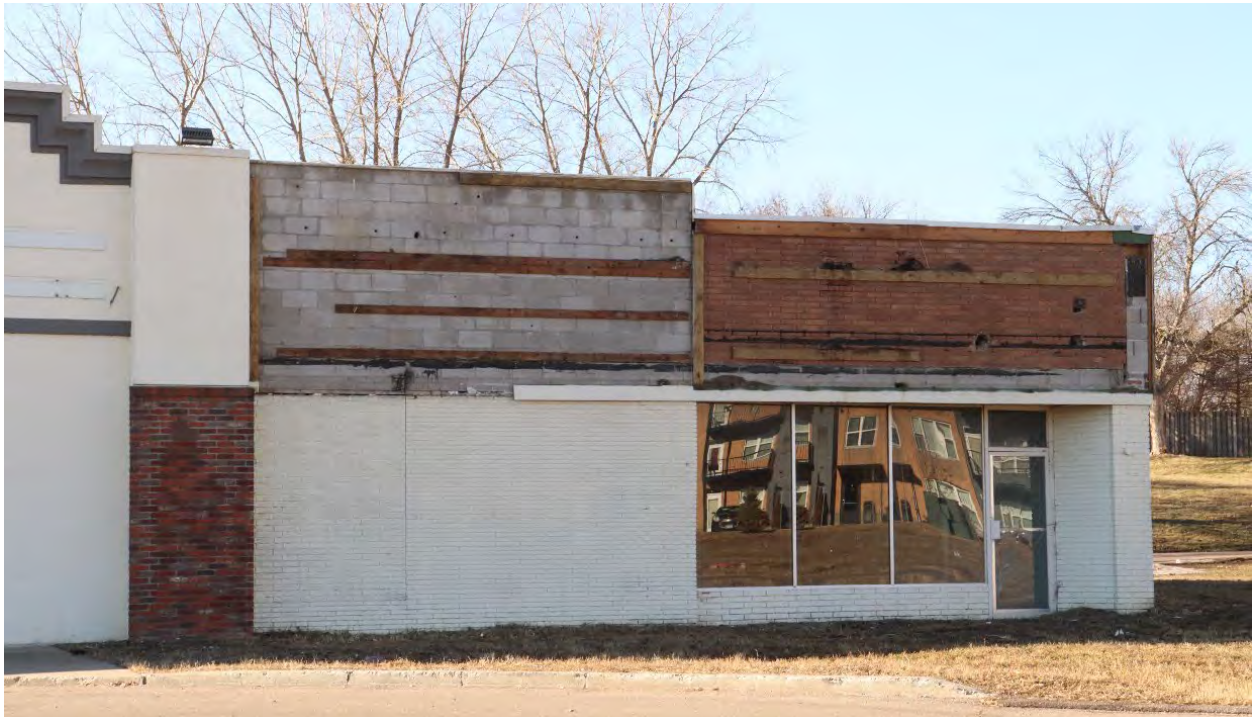
DK-WPC-00082, January 31, 2024, Front (northeast) facade of northwest ell featuring exposed original construction, view facing west.
