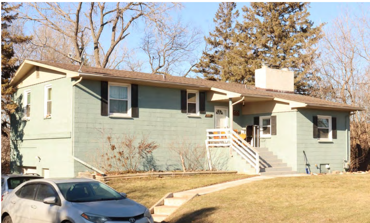
RA-RVC-00061, January 29, 2024, front (east) facade and side (south) elevation, view facing northwest.
