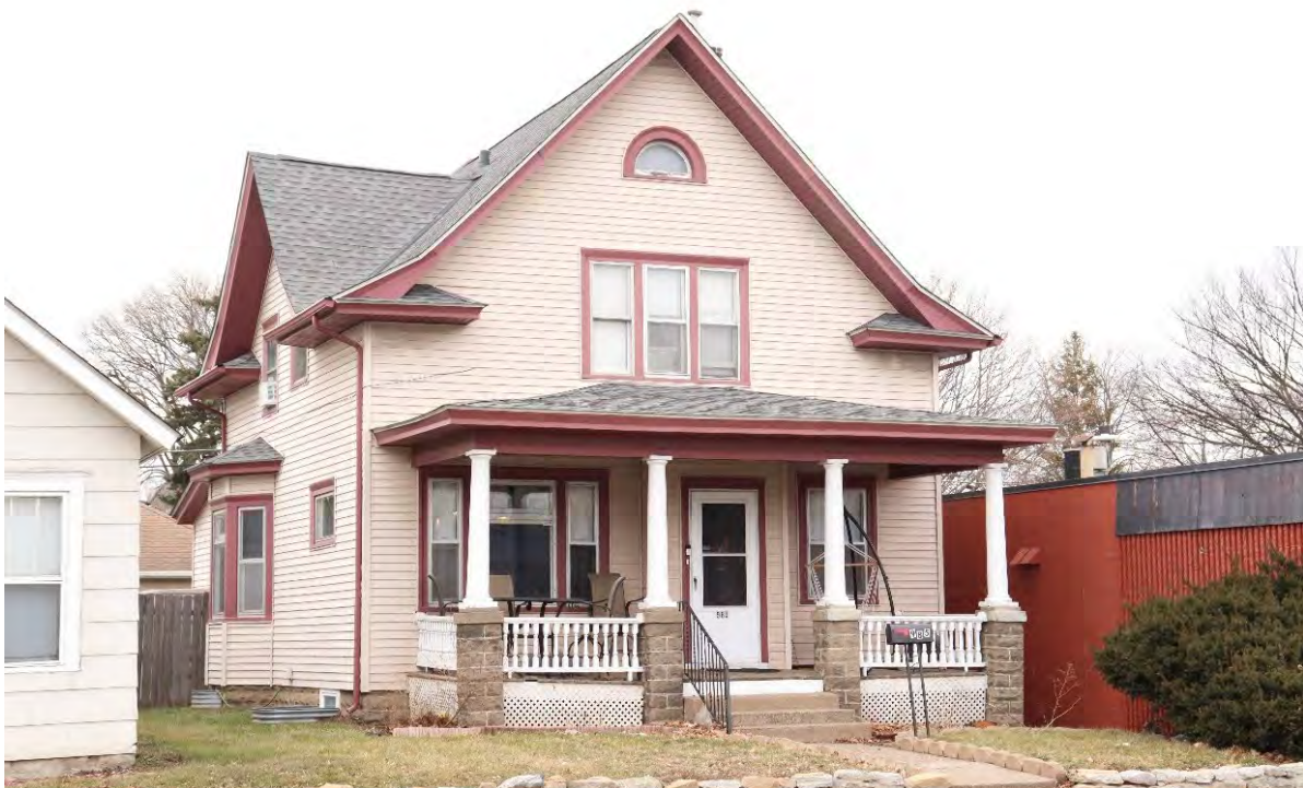
RA-SPC-03086, January 30, 2024, front (east) facade and side (south) elevation, view facing northwest.
