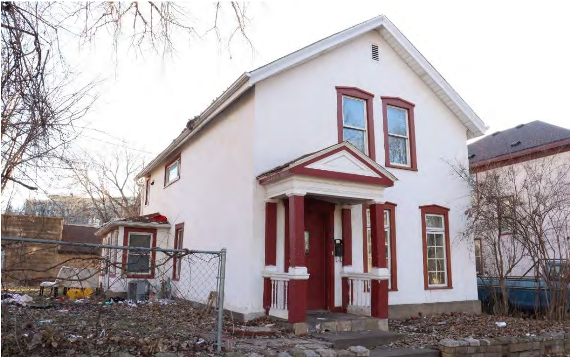
RA-SPC-11936, January 31, 2024, front (north) facade and side (east) elevation, view facing southwest.
