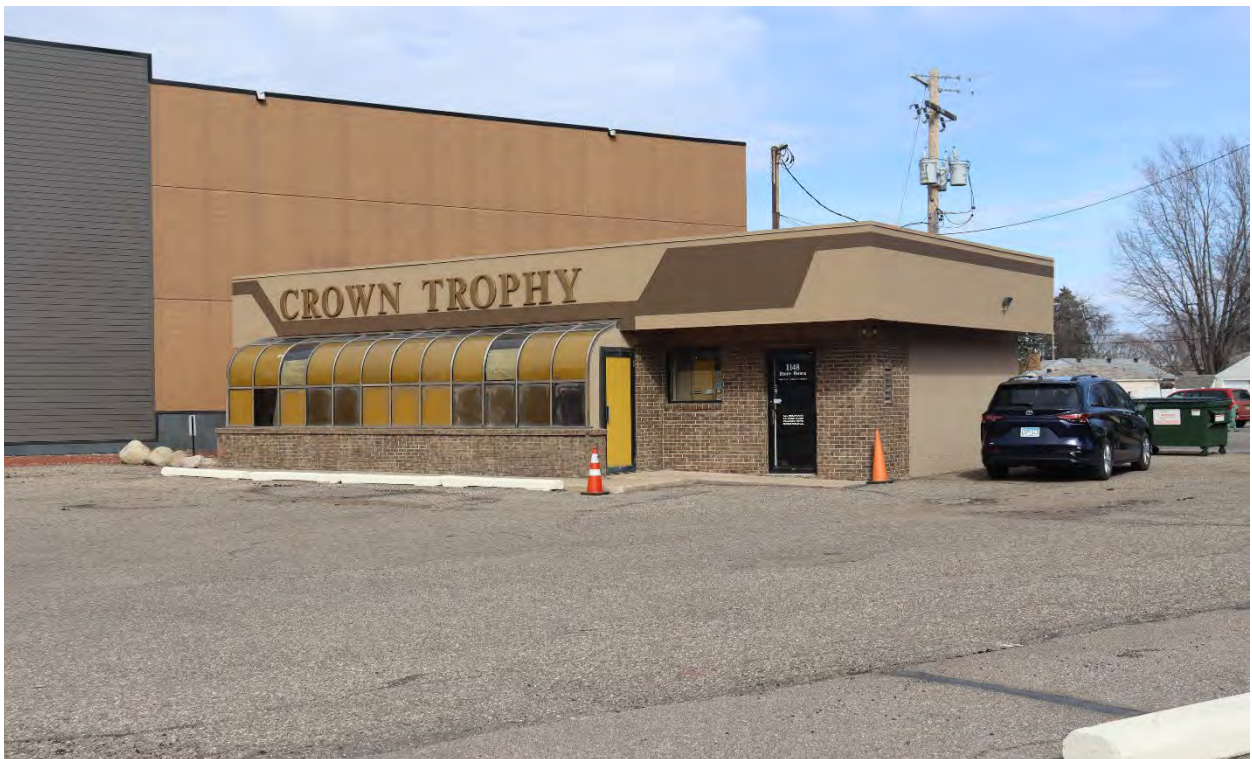
DK-WPC-00092, March 06, 2024, front (west) facade and side (south) elevation, view northeast.
