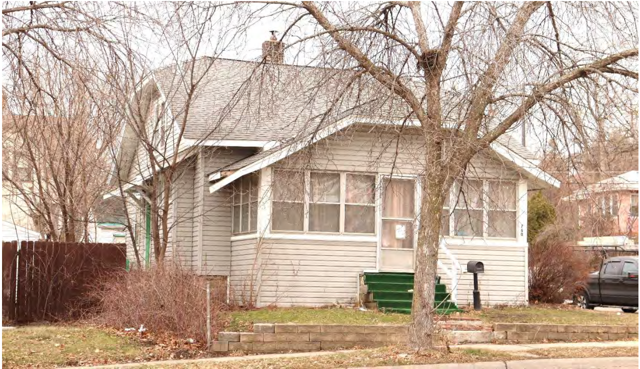
RA-SPC-09016, February 02, 2024, front (west) facade and side (north) elevation, view facing southeast.
