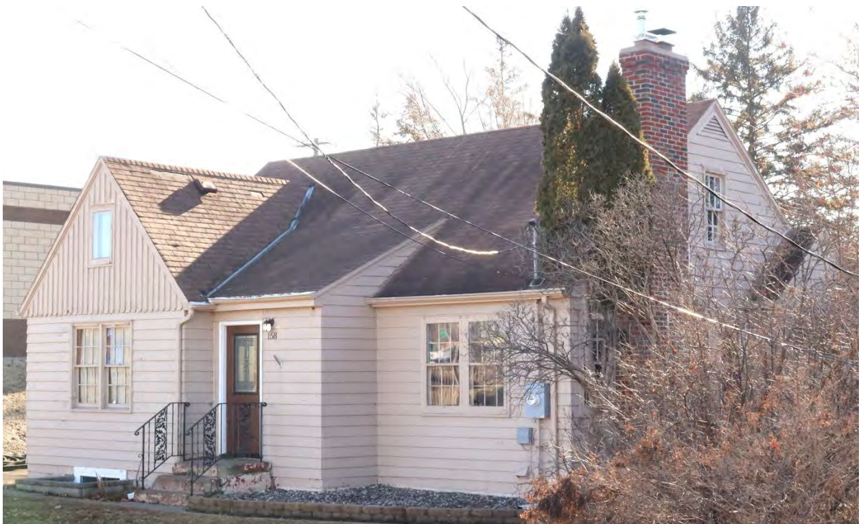
RA-RVC-00055, January 29, 2024, front (north) façade and side (west) elevation, view facing southeast.
