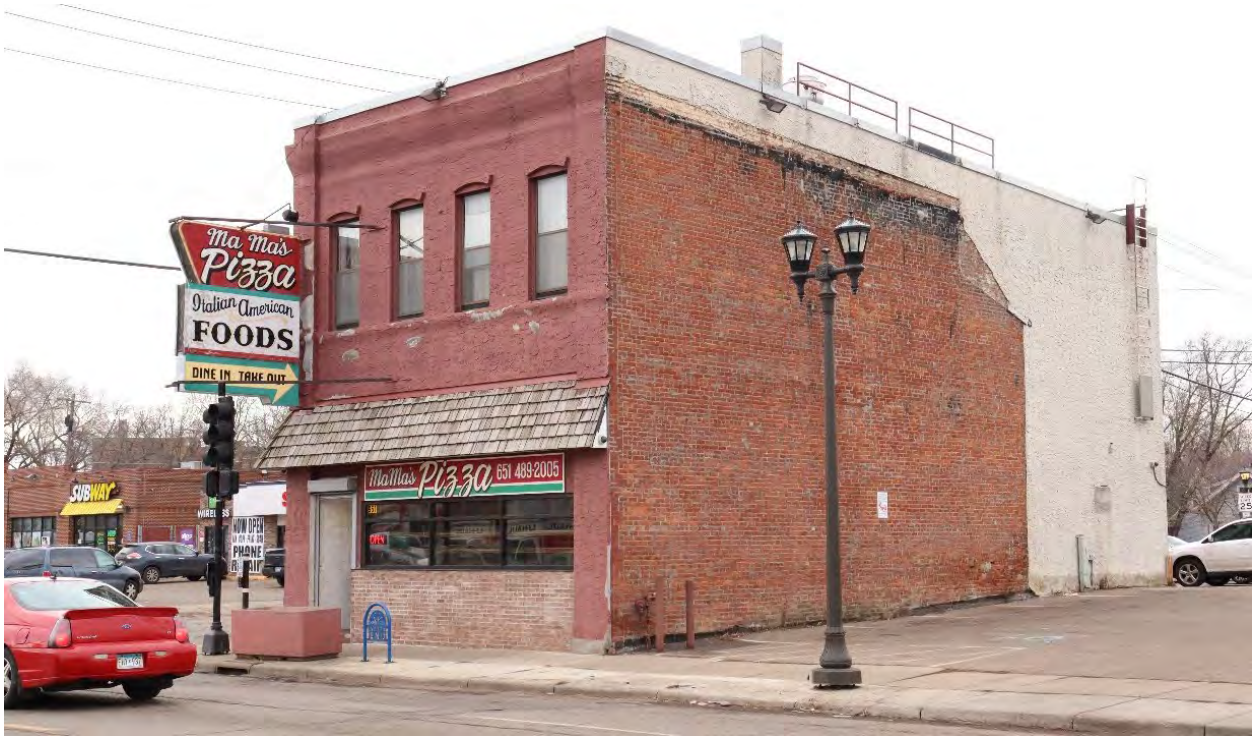
RA-SPC-03082, January 30, 2024, front (east) facade and side (north) elevation, view facing southwest.
