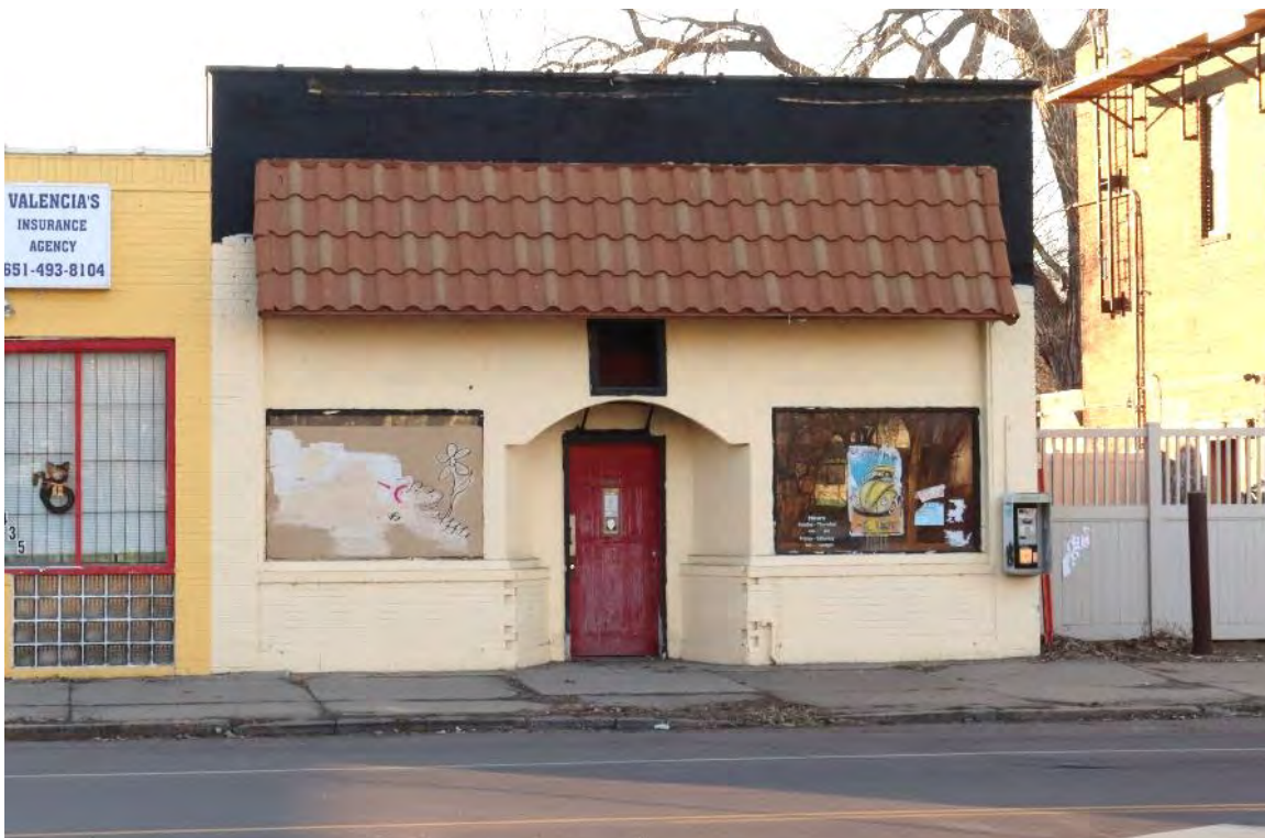
RA-SPC-08969, January 31, 2024, front (east) facade, view facing west.
