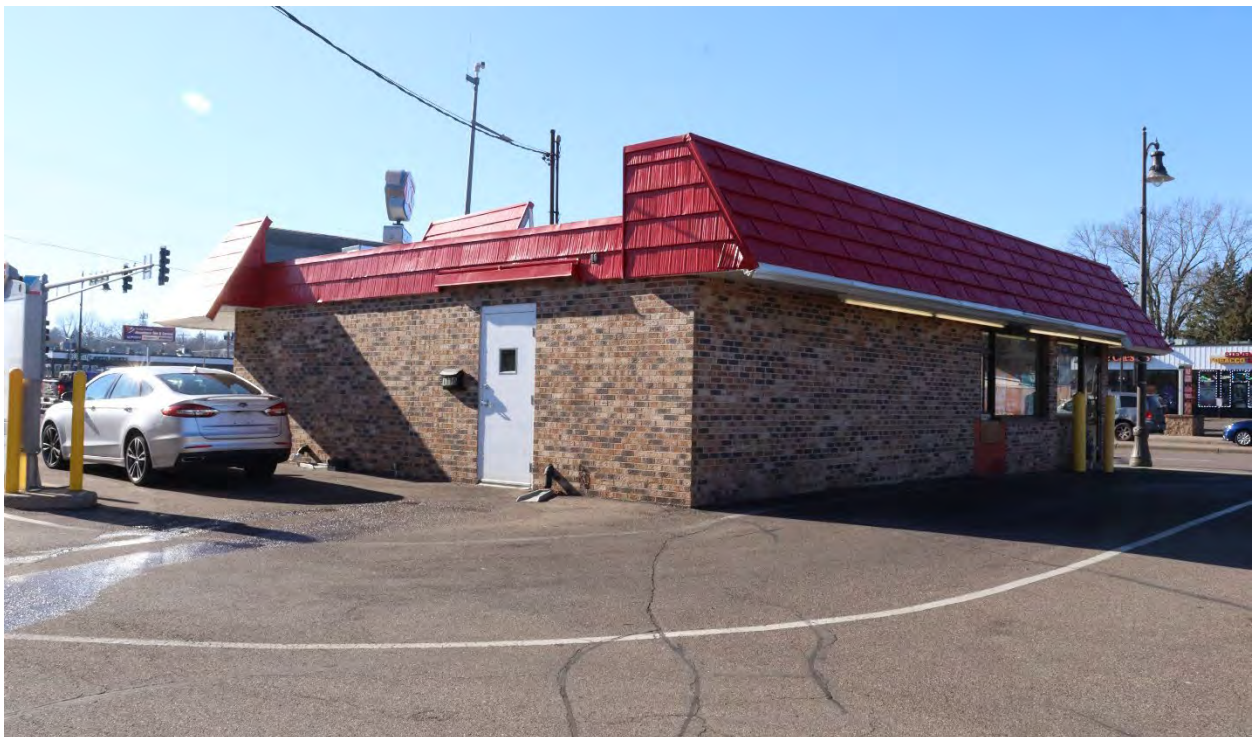
DK-WPC-00088, January 31, 2024, rear (north) facade and side (east) elevation with drive-through menu board (left) and signage (in background), view facing southwest.
