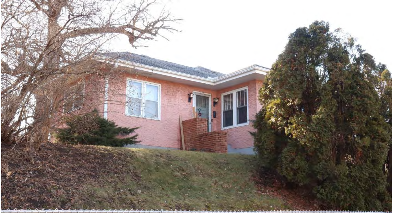
RA-SPC-11908, January 31, 2024, front (north) facade and side (east) elevation, view facing southwest.
