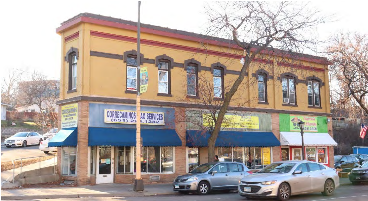
RA-SPC-00785, January 31, 2024, front (northeast) facade, view facing west.
