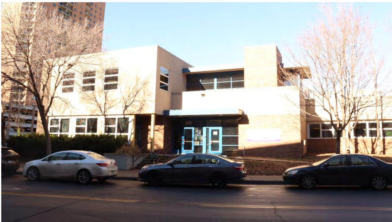
RA-SPC-08952, February 1, 2024, front (south) facade addition, view facing northwest.
