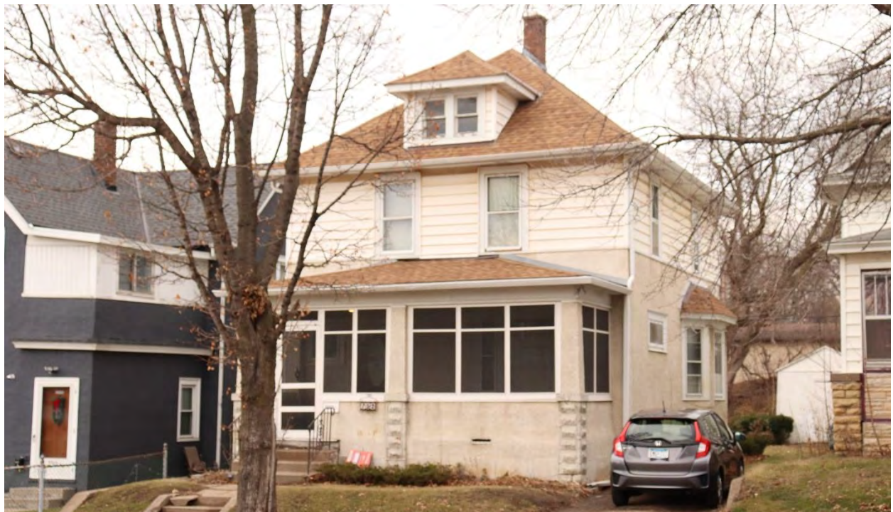
RA-SPC-09013, January 31, 2024, front (west) facade, side (south) elevation, and shed, view facing northeast.
