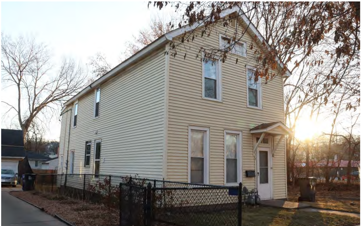
RA-SPC-08959, January 31, 2024, front (north) facade and side (east) elevation, view facing southwest.
