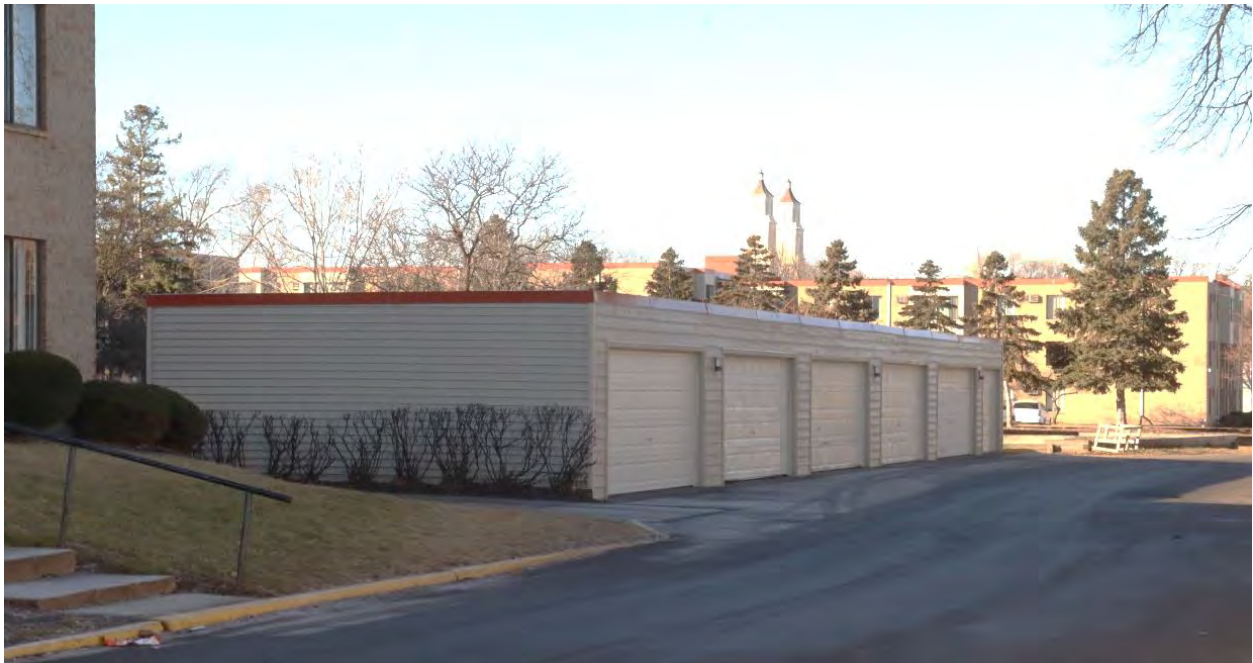
RA-SPC-11925, February 1, 2024, Front (north) facade of garage building, view facing southwest.
