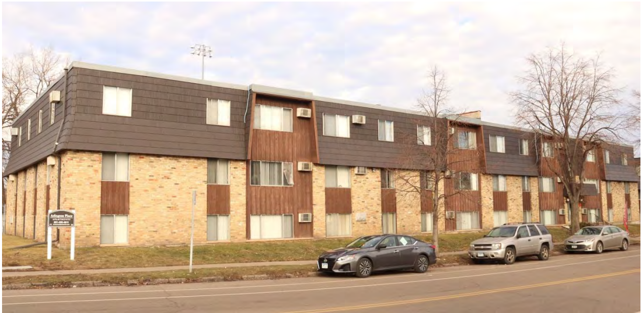
RA-SPC-11899, January 29, 2024, front (south) facade and side (west) elevation, view facing northeast.
