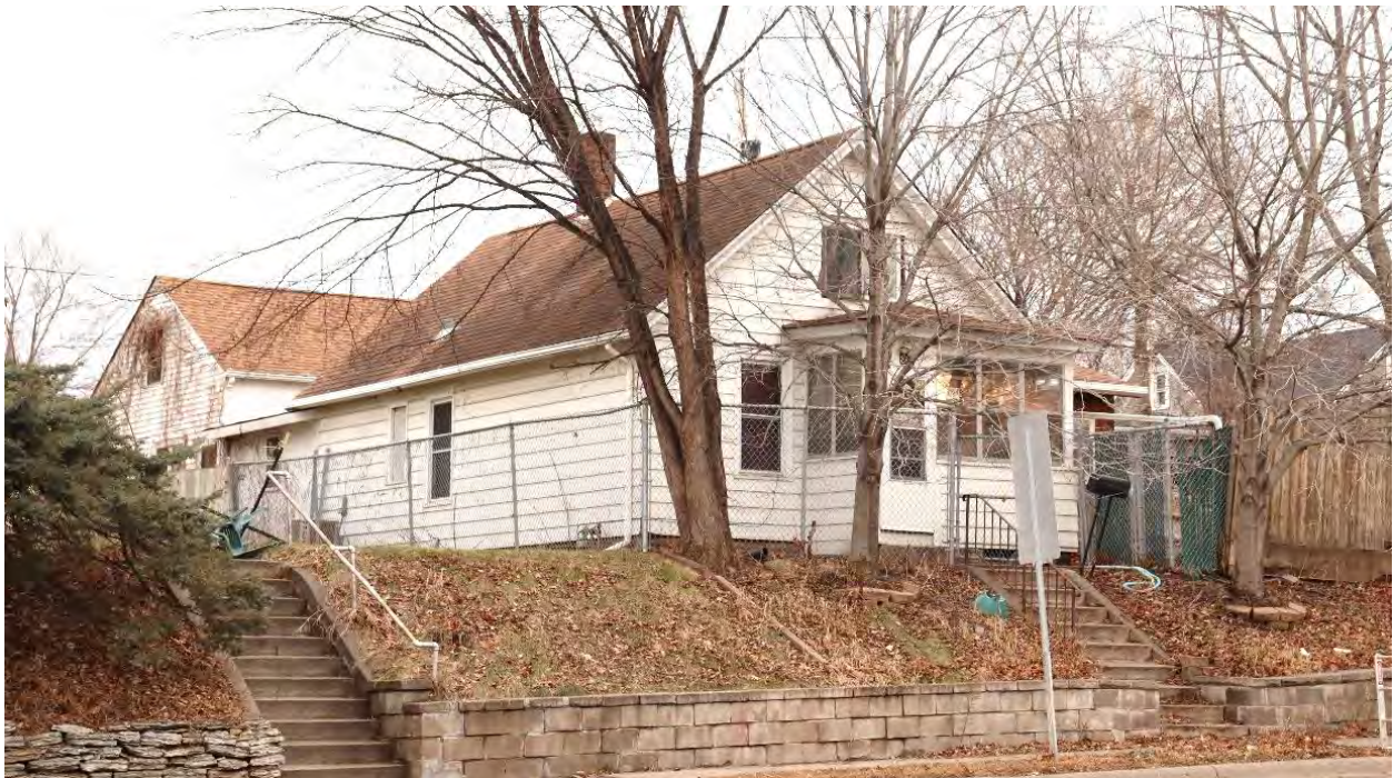
RA-SPC-09038, January 29, 2024, front (west) facade and side (north) elevation featuring breezeway and garage, view facing southeast.
