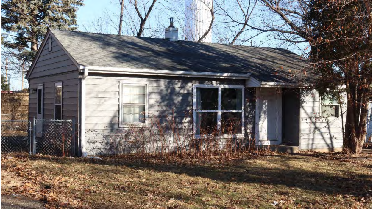
DK-WPC-00095, January 8, 2024, front (south) facade and side (west) elevation, view facing northeast.
