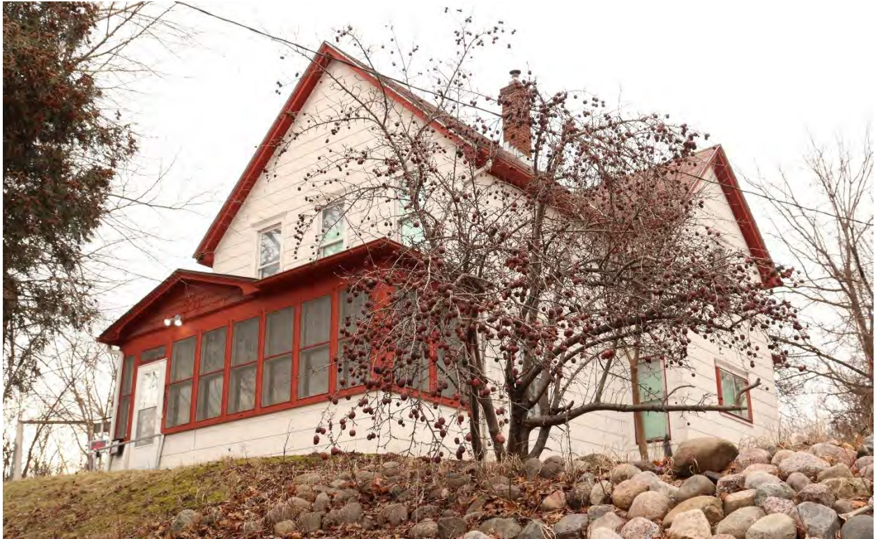
RA-SPC-09017, February 02, 2024, front (east) facade and side (north) elevation, view facing southwest.
