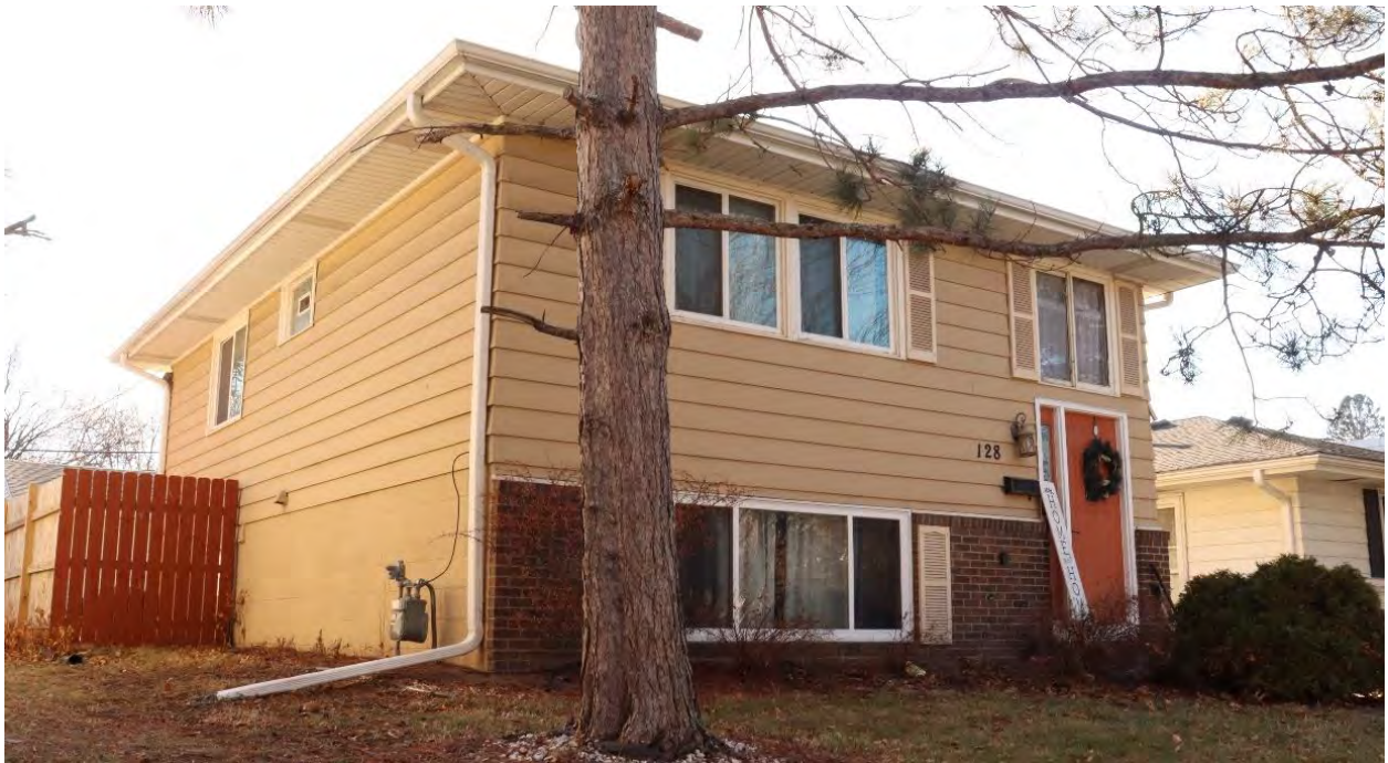
RA-SPC-11912, January 31, 2024, Front (north) facade and side (east) elevation, view facing southwest.
