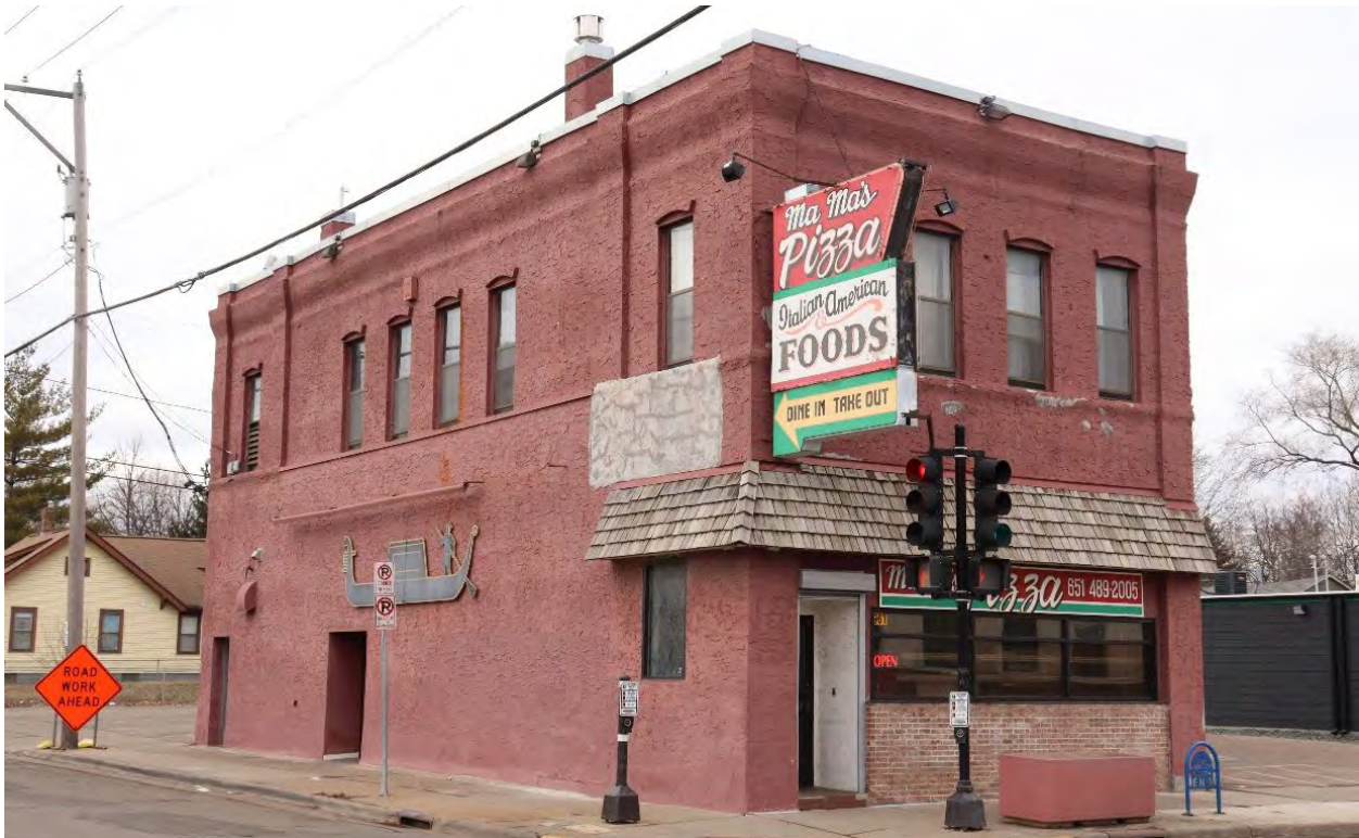
RA-SPC-03082, January 30, 2024, front (east) facade and side (south) elevation, view facing northwest.
