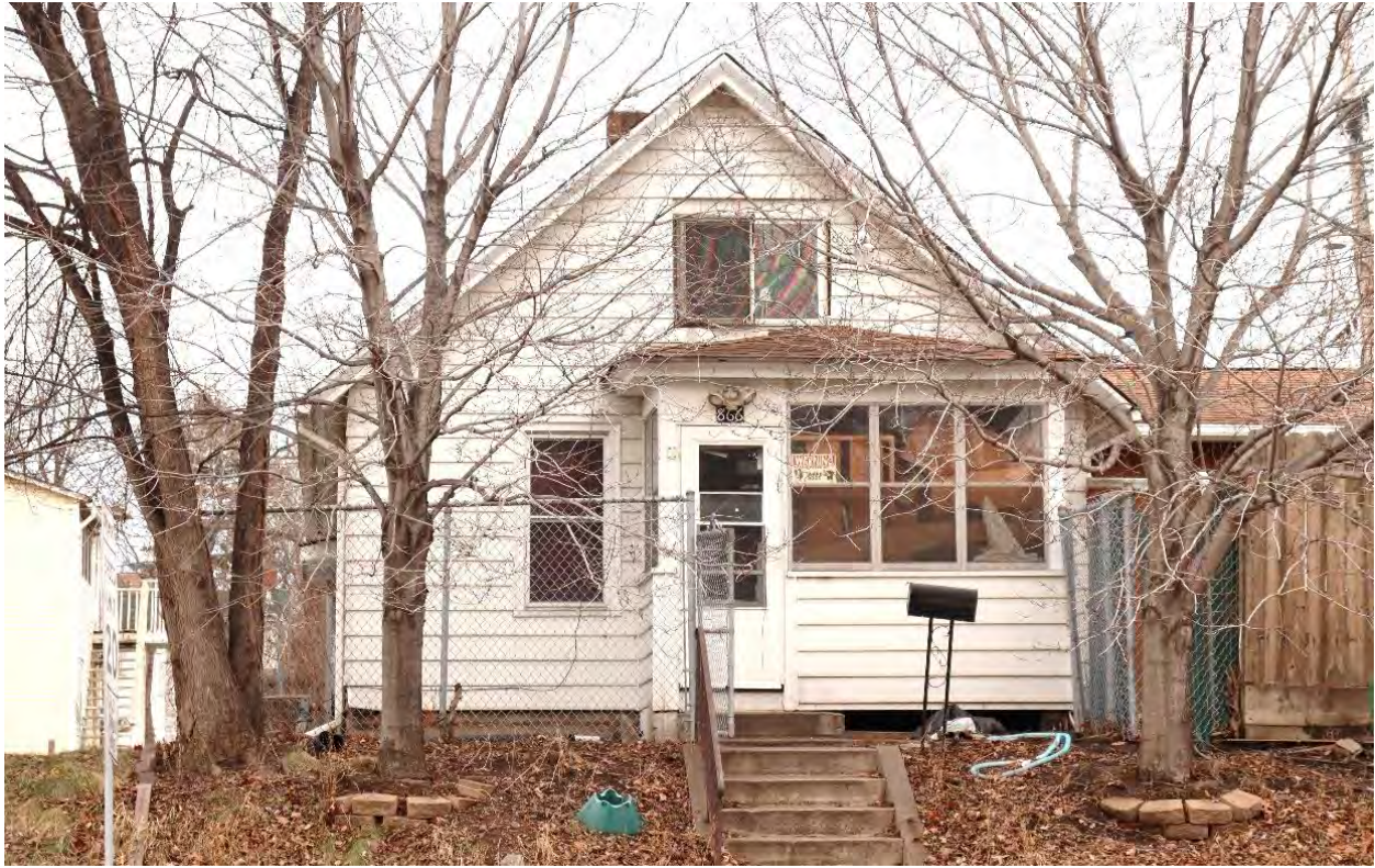
RA-SPC-09038, January 29, 2024, front (west) facade, view facing east.
