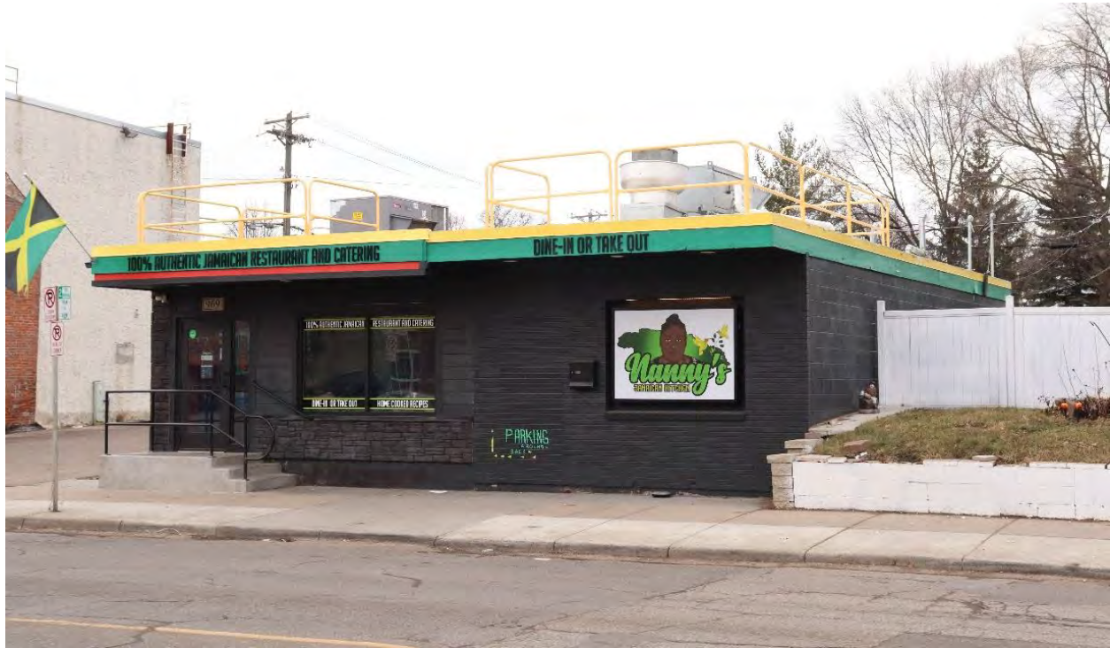
RA-SPC-11940, January 30, 2024, Front (east) facade and side (north) elevation, view facing southwest.
