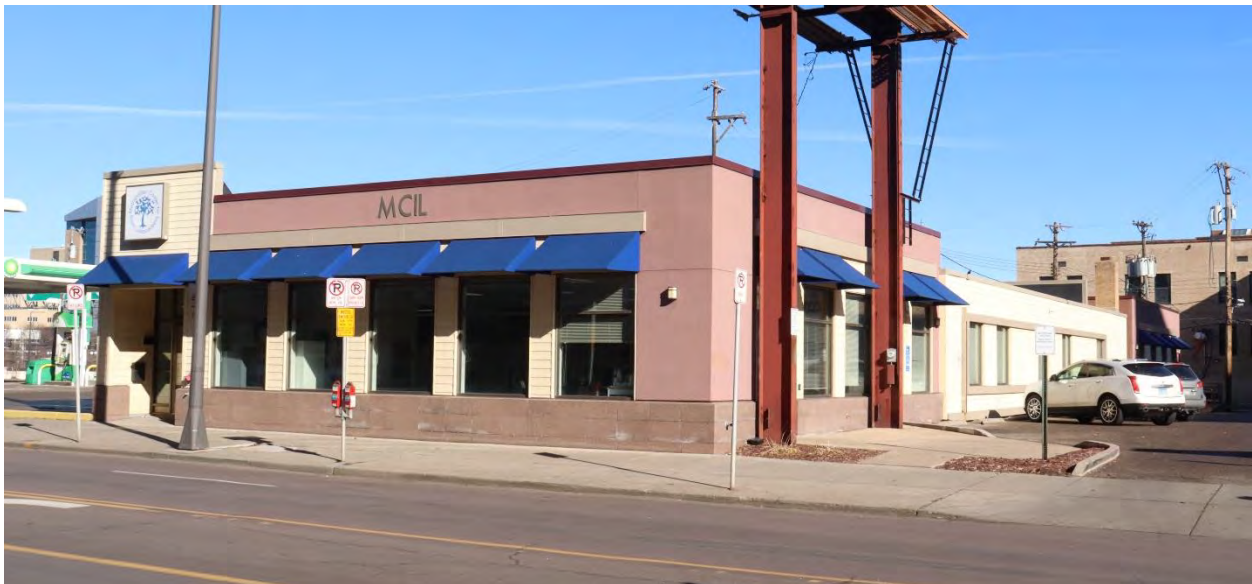
RA-SPC-08962, February 01, 2024, front (southwest) facade and side (southeast) elevation, view facing north.
