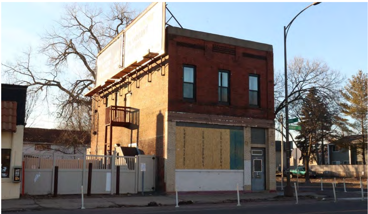
RA-SPC-03185, January 31, 2024, front (west) facade and side (south) elevation, view facing northwest.
