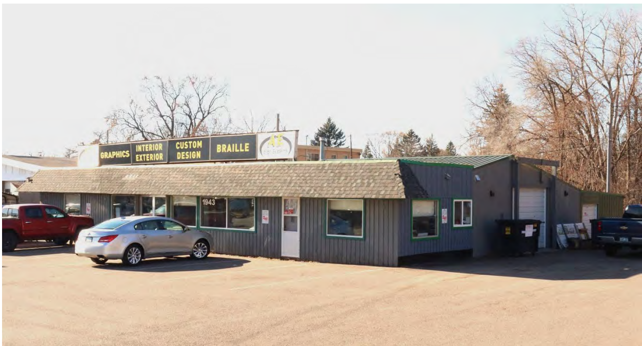
RA-RVC-00060, January 29, 2024, front (east) facade and side (north) elevation, view facing southwest.
