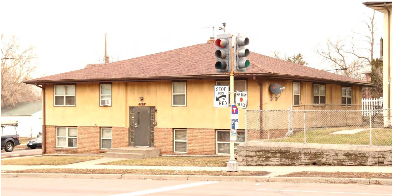
RA-SPC-09018, February 02, 2024, front (west) facade and side (south) elevation, view facing northeast.
