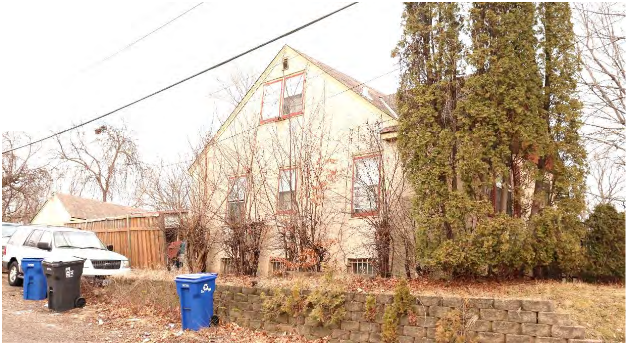
RA-SPC-09039, January 29, 2024, side (north) elevation featuring garage, view facing southeast.
