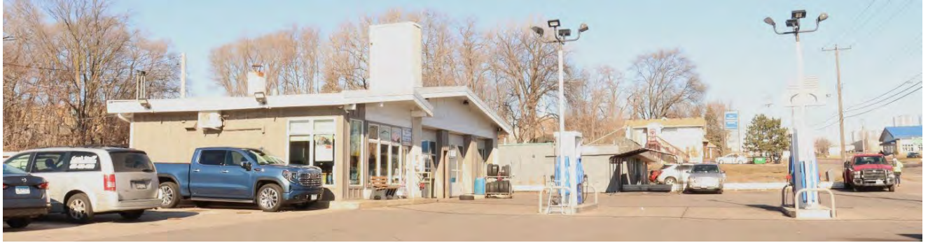
RA-RVC-00059, January 29, 2024, front (east) facade, side (south) elevation and gas pumps, view facing northwest.
