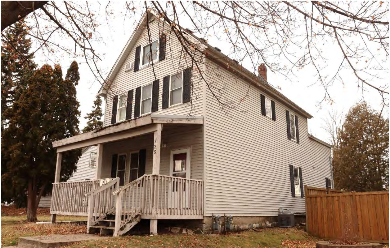
RA-SPC-09006, February 02, 2024, front (east) facade and side (north) elevation, view facing southwest.
