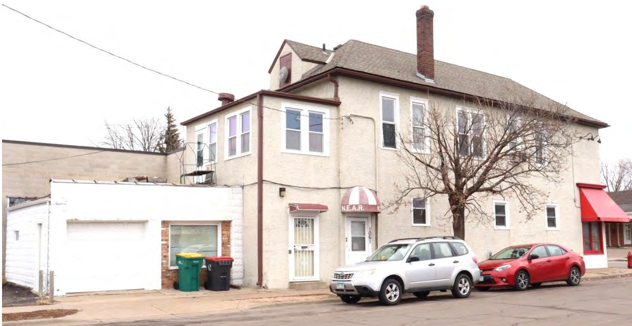
RA-SPC-03088, January 29, 2024, side (south) elevation and rear (west) elevation, view facing northeast.
