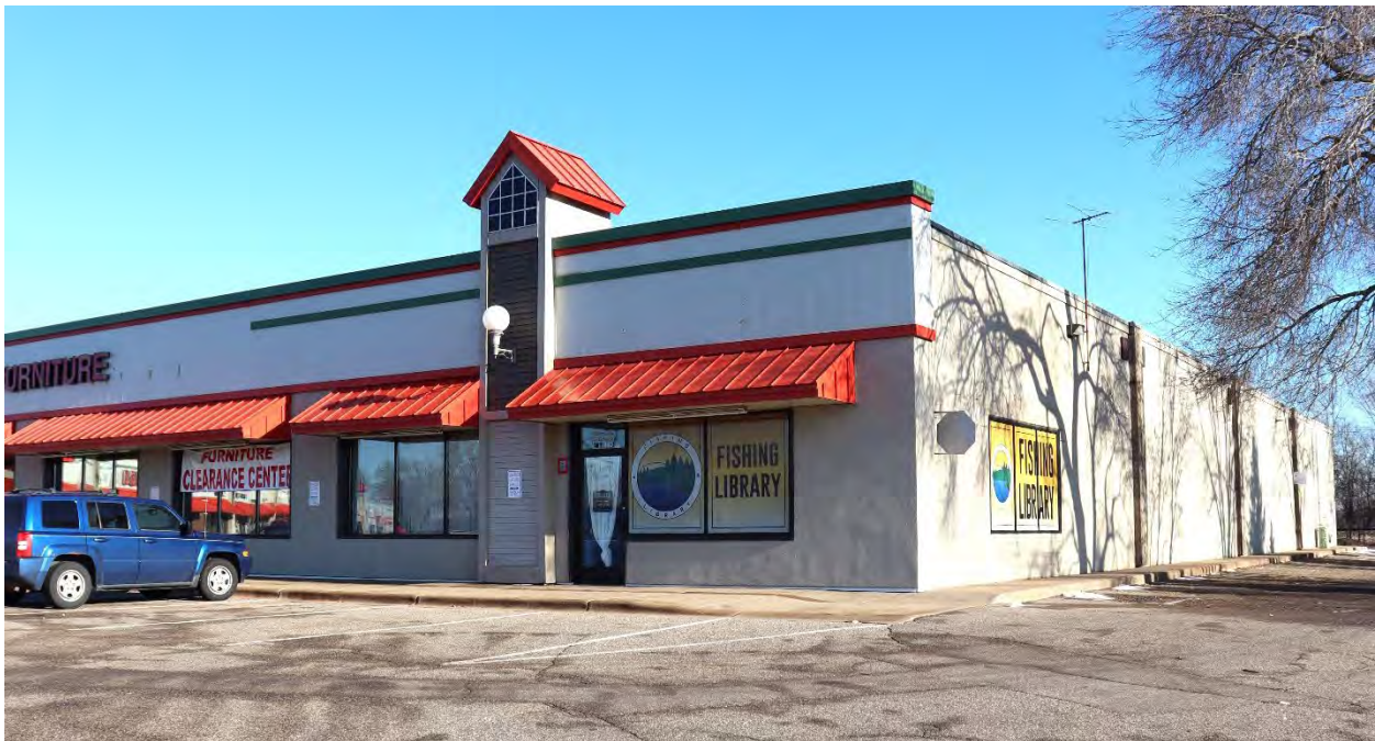
RA-LCC-00084, January 29, 2024, front (south) facade and side (west) elevation, view facing northeast.
