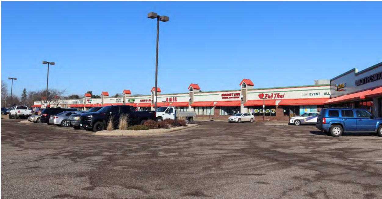
RA-LCC-00084, January 29, 2024, front (south) elevation, view facing northeast.
