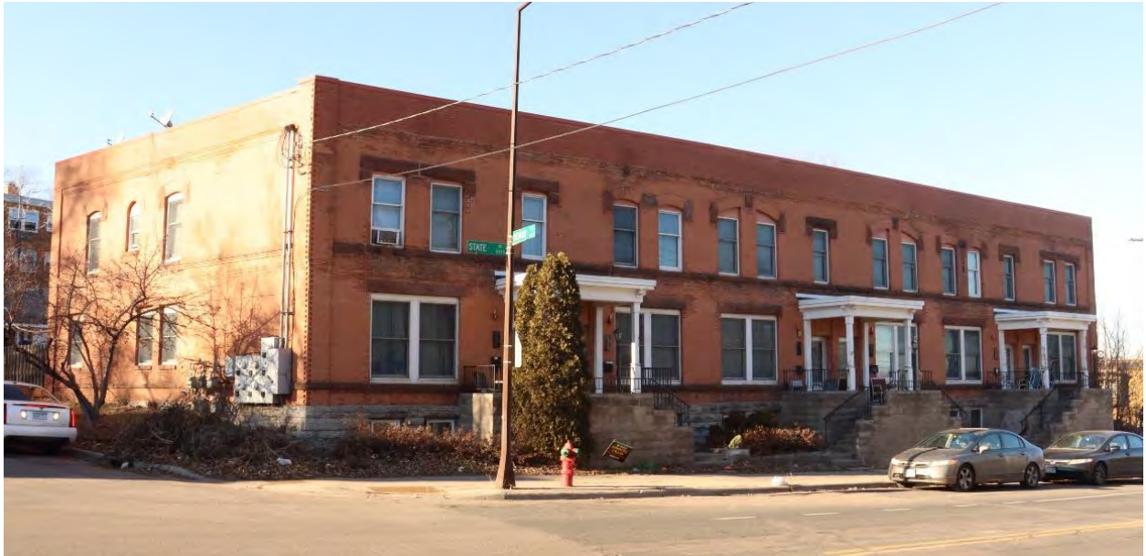
RA-SPC-03525, January 31, 2024, front (east) facade and side (south) elevation, view facing northwest.
