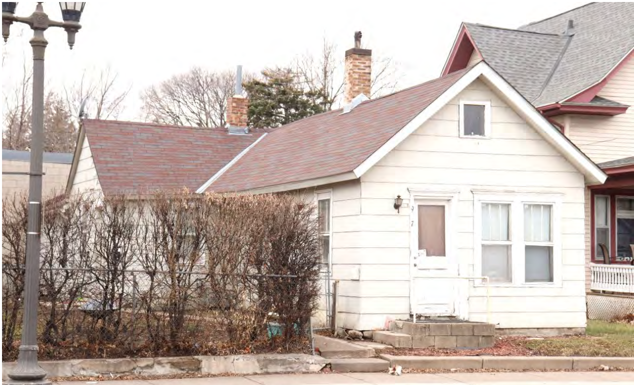
RA-SPC-03084, January 30, 2024, front (east) facade and side (south) elevation, view facing northwest.
