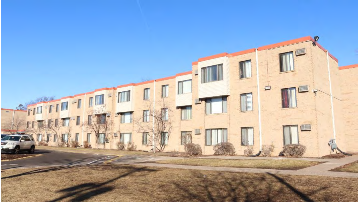
RA-SPC-11925, February 1, 2024, Side (south) elevation of easternmost building, view facing northwest.
