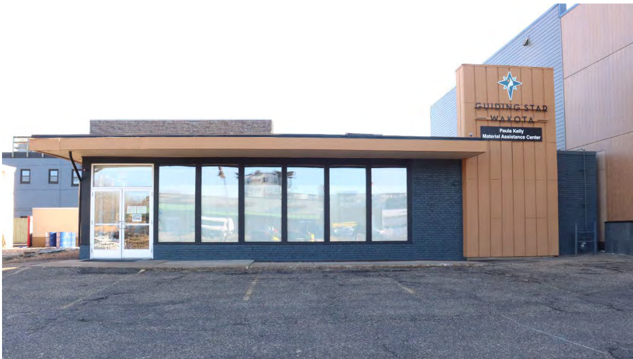
DK-WPC-00090, January 31, 2024, front (west) facade, view facing east.
