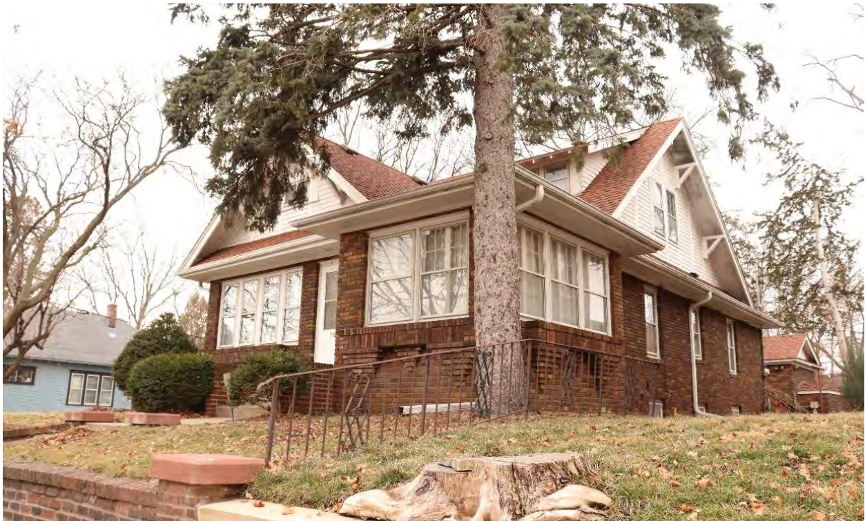
RA-SPC-09000, January 29, 2024, front (north) facade and side (west) elevation, view facing southeast.
