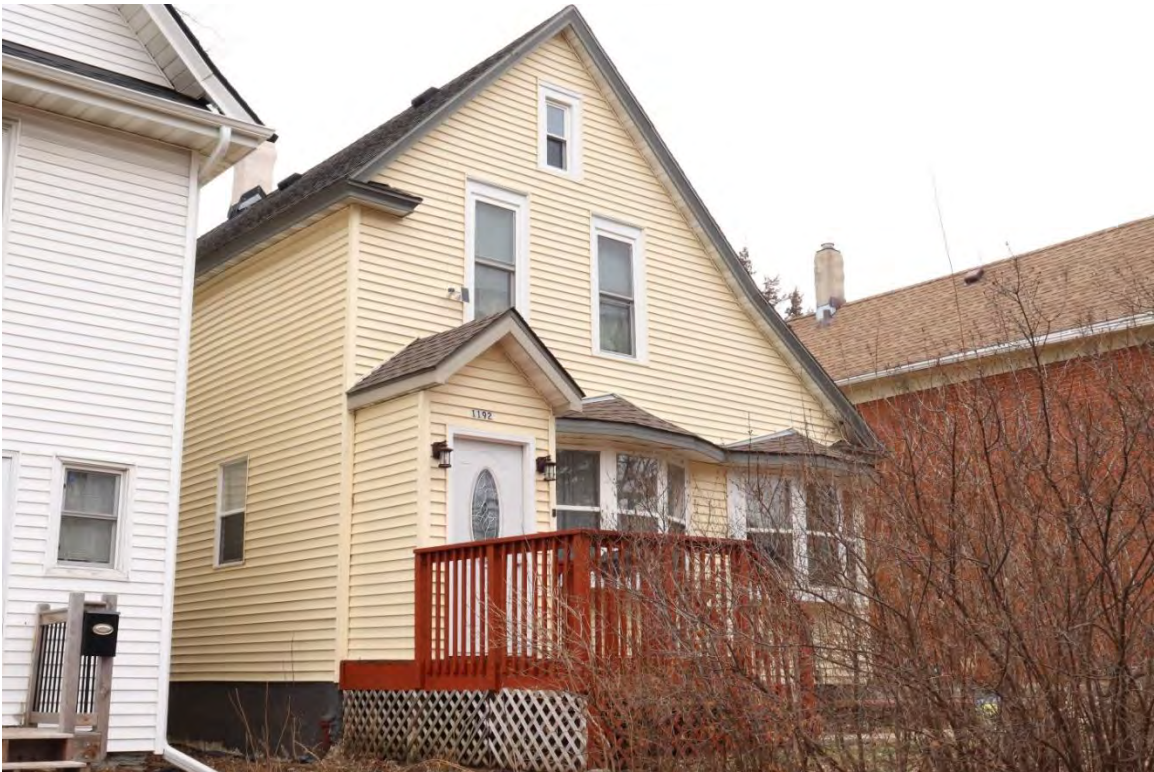
RA-SPC-11900, January 29, 2024, front (west) facade and side (north) elevation, view facing southeast.
