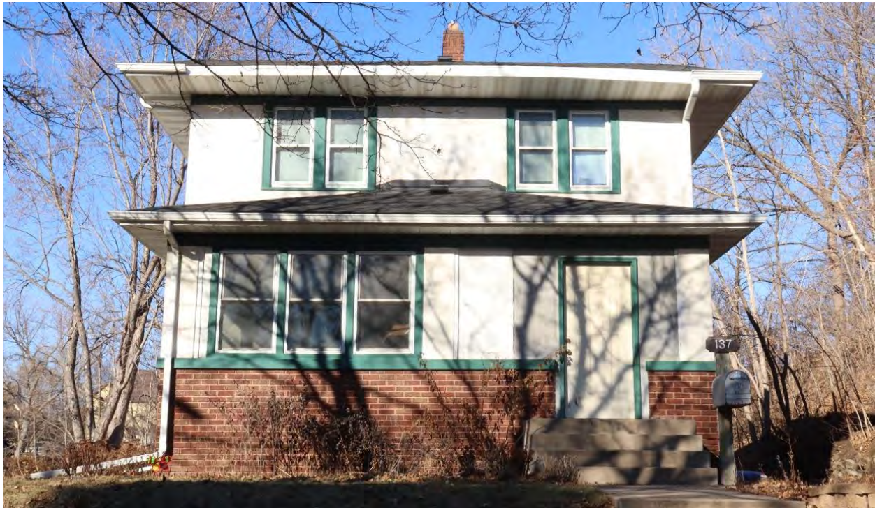
RA-SPC-11891, January 31, 2024, Front (south) facade, view facing north.
