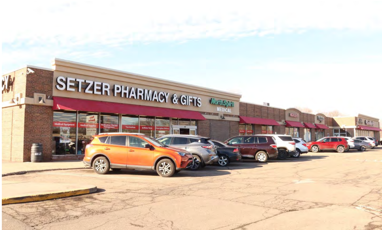
RA-RVC-00057, January 29, 2024, front (east) facade and side (south) elevation, view facing northwest.
