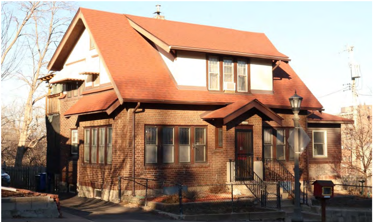
RA-SPC-11921, January 31, 2024, Side (west) elevation and front (south) facade, view facing northeast.
