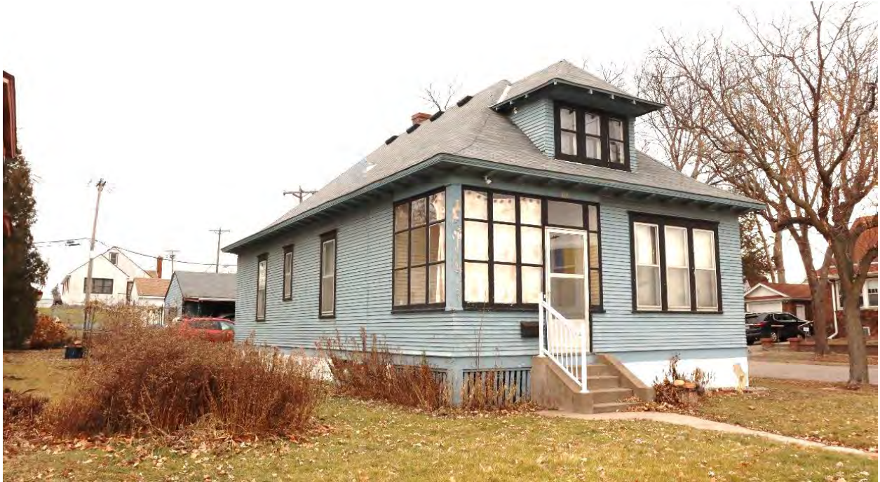
RA-SPC-09003, January 29, 2024, front (east) facade and side (south) elevation, view facing northwest.
