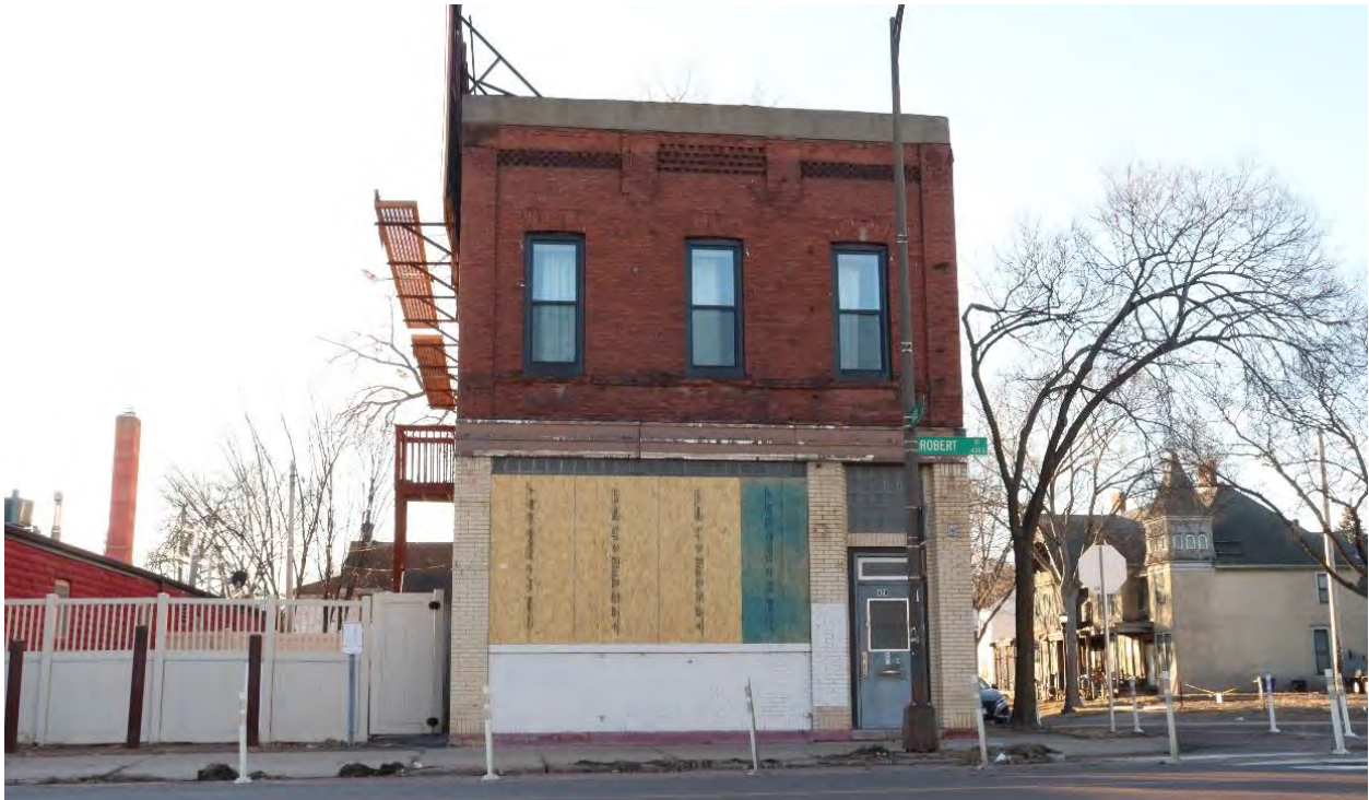
RA-SPC-03185, January 31, 2024, front (east) facade, view facing west.
