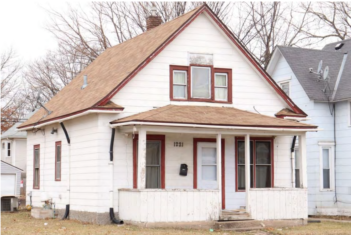
RA-SPC-11909, January 30, 2024, front (east) facade and side (north) elevation, view facing southwest.
