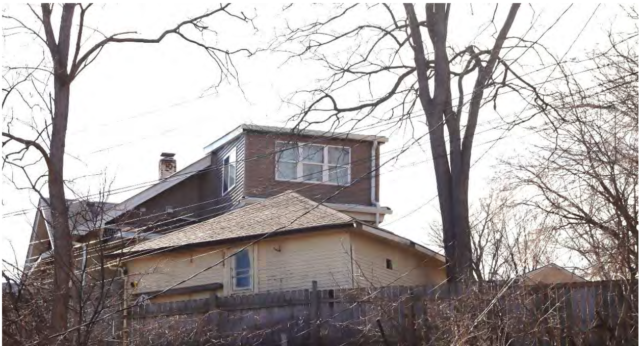
RA-SPC-11921, January 31, 2024, Rear (northeast) elevation of detached garage, view facing southwest.
