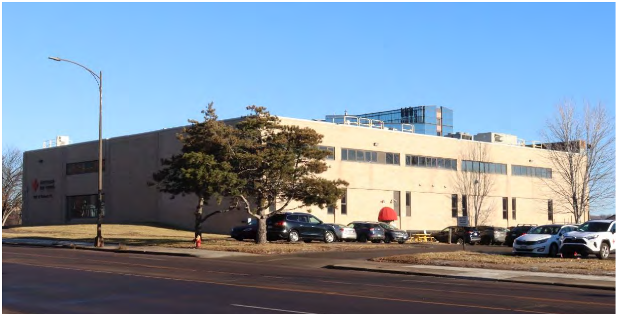
RA-SPC-11893, February 1, 2024, side (southwest) and rear (southeast) elevations with secondary entrance, view facing northeast.
