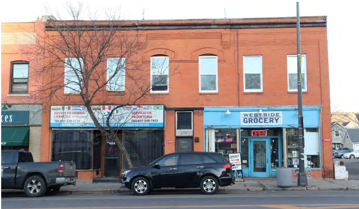
RA-SPC-03188, January 31, 2024, front (west) facade, view facing east.
