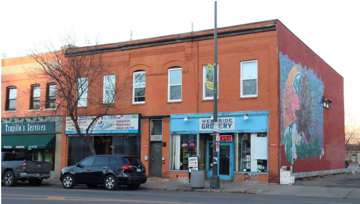
RA-SPC-03188, January 31, 2024, front (west) facade and side (south) elevation, view facing northeast.
