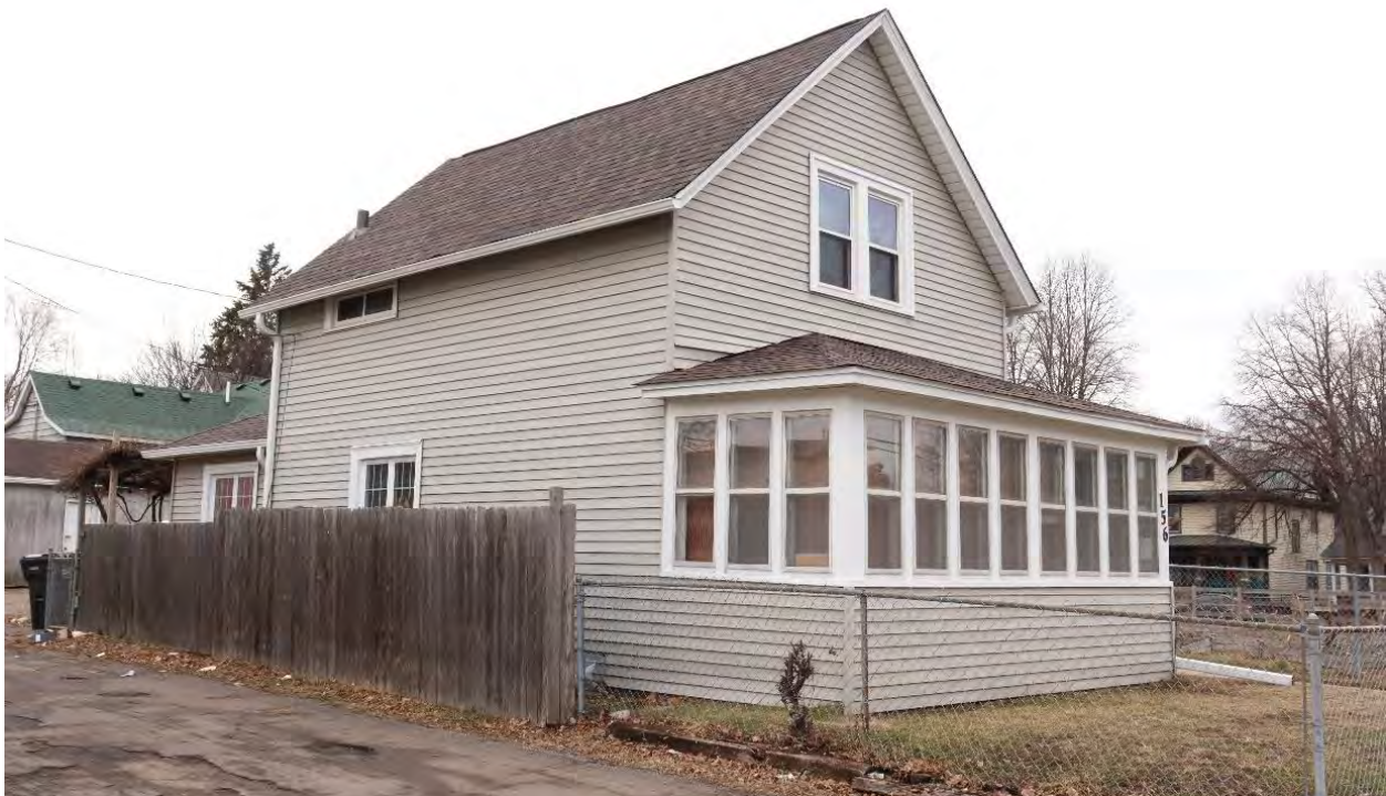
RA-SPC-11923, January 30, 2024, Front (north) facade and side (east) elevation, view facing southwest.
