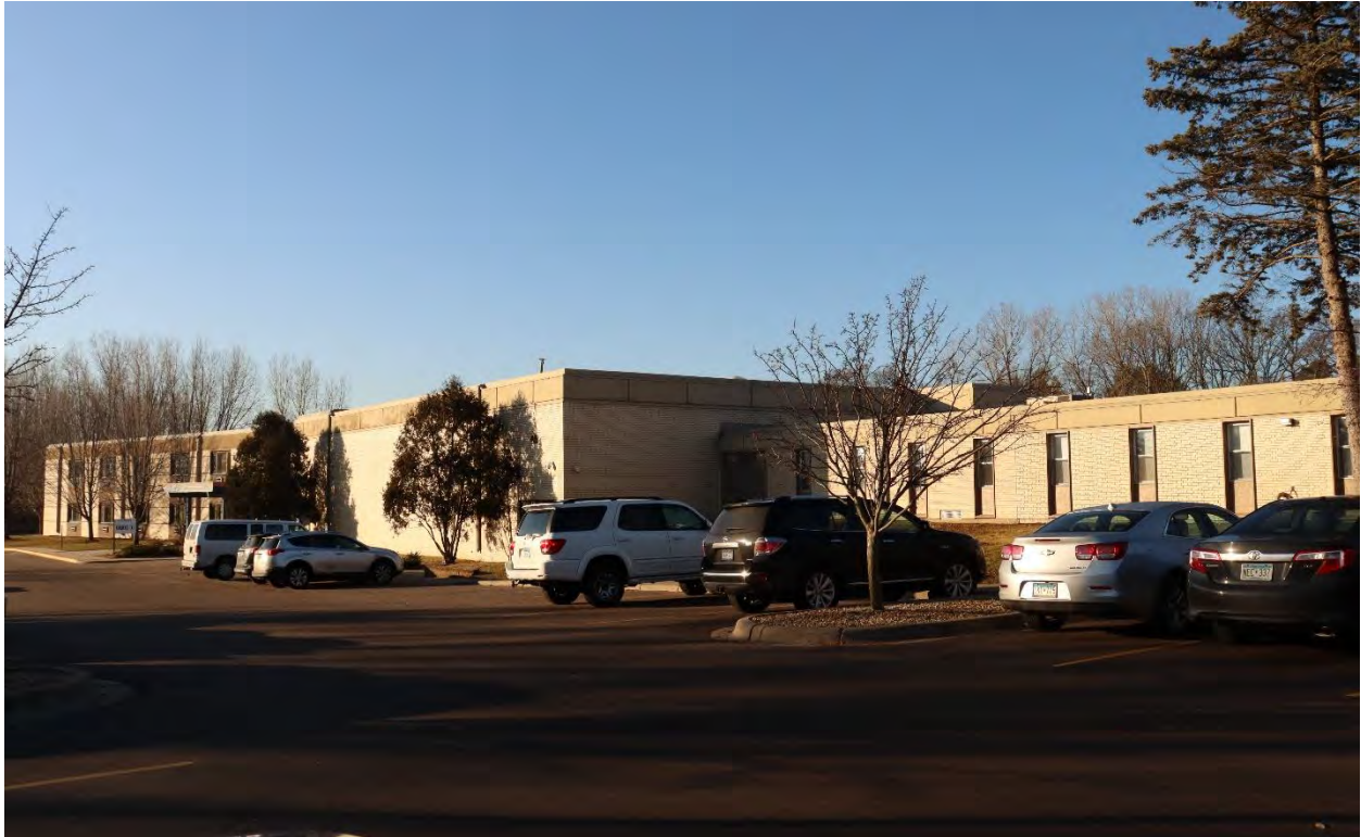
DK-WPC-00081, January 31, 2023, side (east) elevation, view facing northeast.
