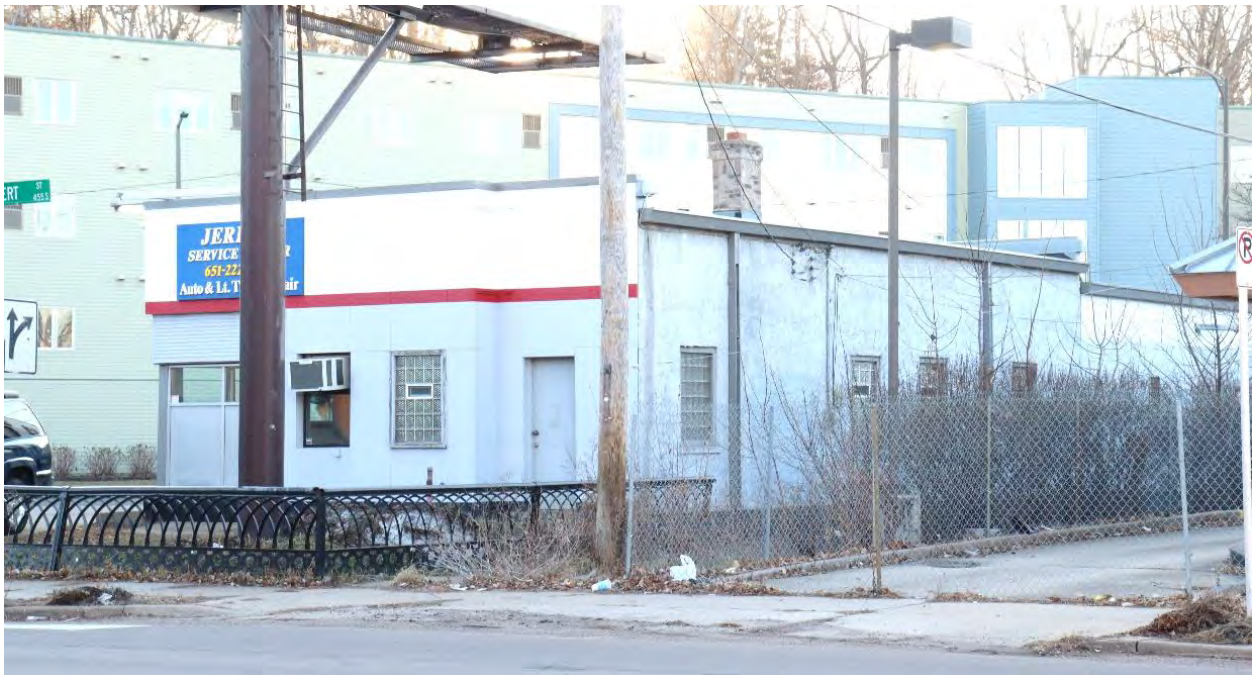
RA-SPC-08972, January 31, 2024, side (east) elevation and rear (north) elevation, view facing southwest.
