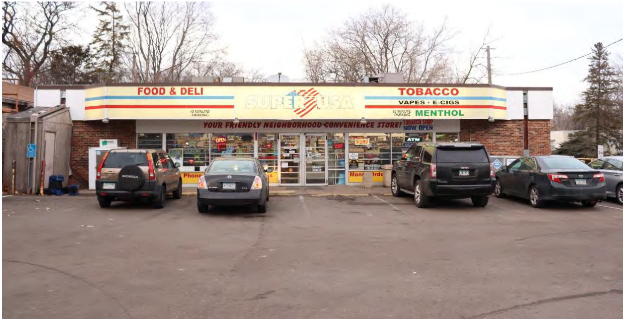
RA-SPC-11941, January 29, 2024, Front (south) facade, view facing north.
