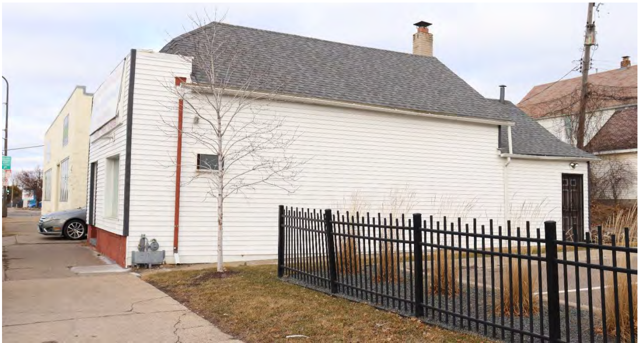
RA-SPC-11934, January 30, 2024, front (west) facade and side (south) elevation, view facing northeast.
