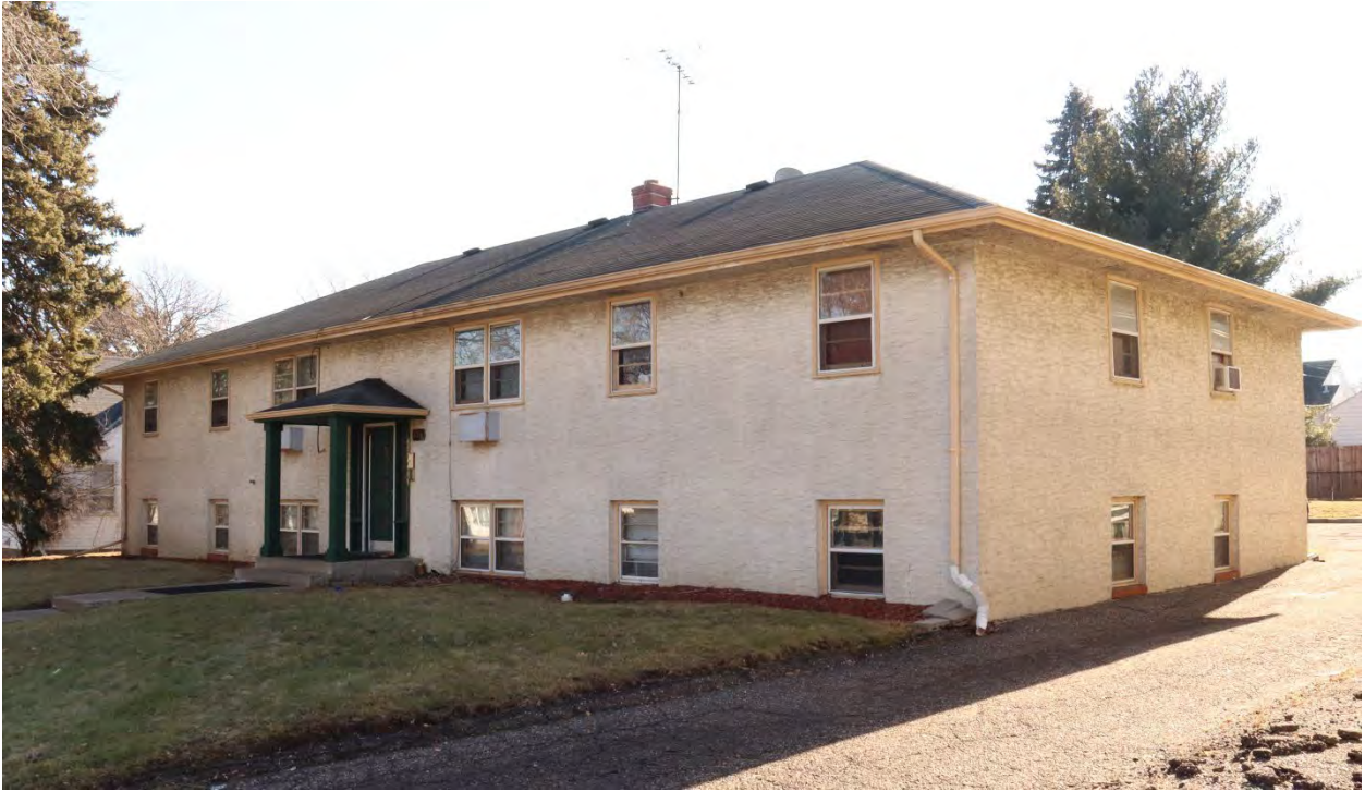
DK-WPC-00096, January 31, 2024, front (north) facade and side (west) elevation, view facing southeast.
