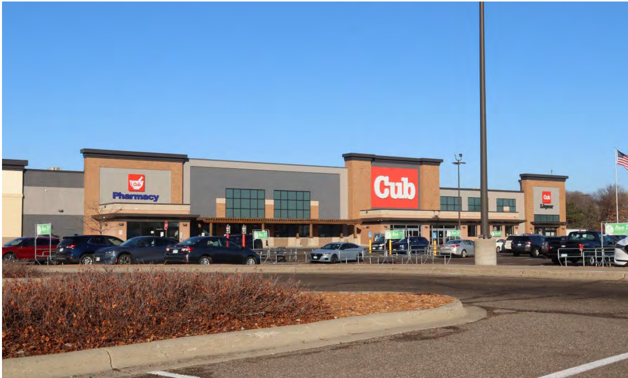
DK-WPC-00100, January 31, 2024, front (east) facade, view facing northwest.
