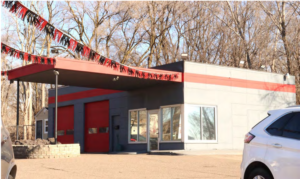
RA-MWC-00358, January 29, 2024, front (west) facade, side (south) elevation, and non-historic-age shed to the northeast of the building, view facing northeast.
