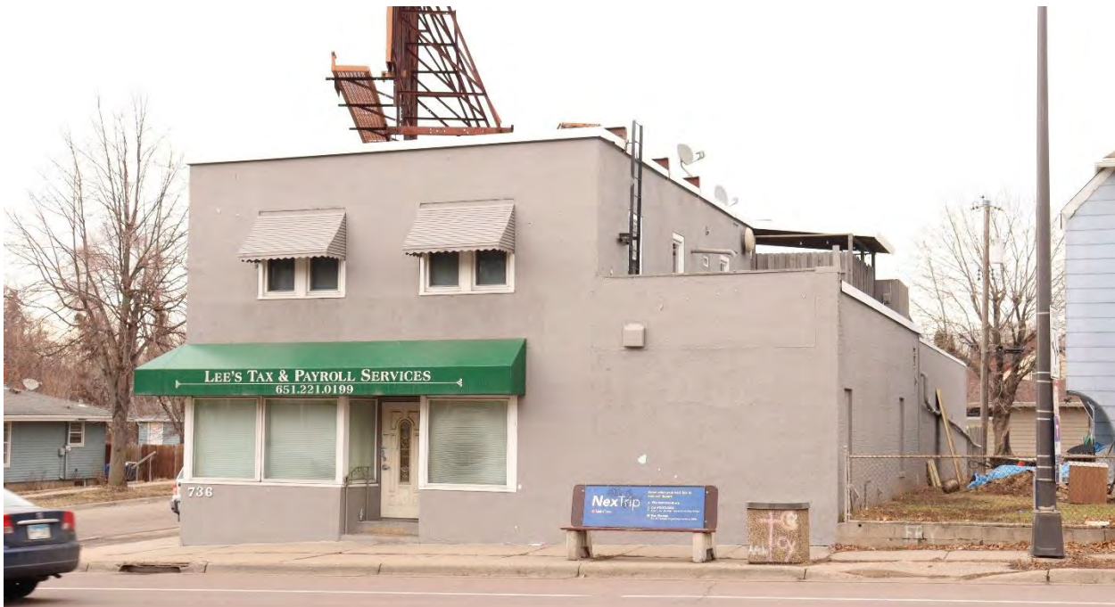
RA-SPC-05754, January 31, 2024, front (west) facade and side (south) elevation, view facing northeast.
