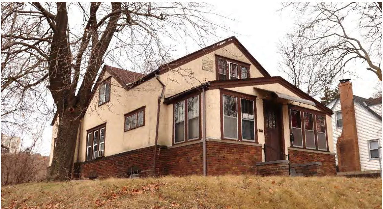
RA-SPC-09042, January 29, 2024, front (north) facade and side (east) elevation, view facing southwest.
