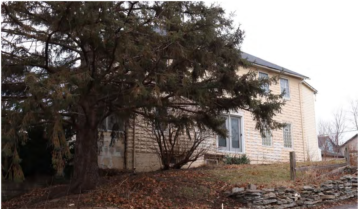
RA-SPC-11902, January 29, 2024, side (west) elevation, view facing southeast.
