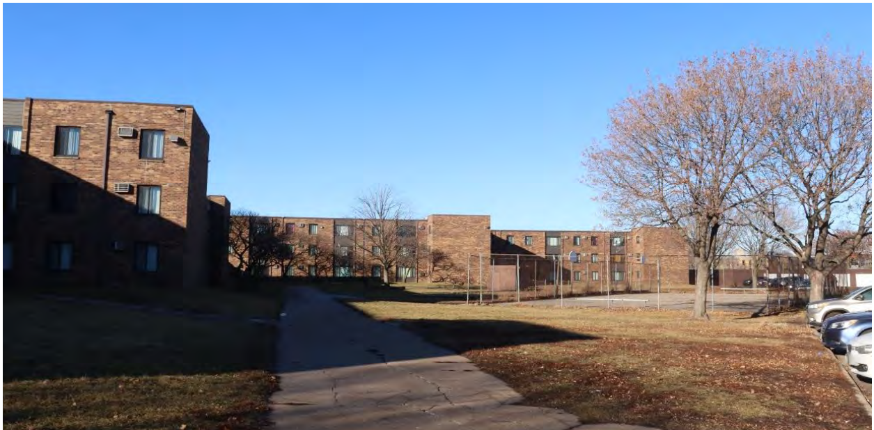
RA-SPC-11929, February 1, 2024, Side (east) elevation of westernmost building mass with basketball court at right, view facing west.
