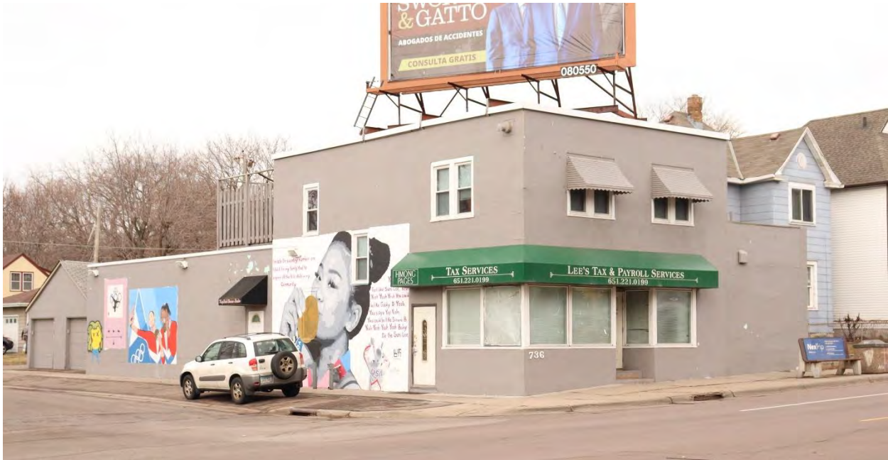
RA-SPC-05754, January 31, 2024, front (west) facade and side (north) elevation, and garage, view facing southeast.
