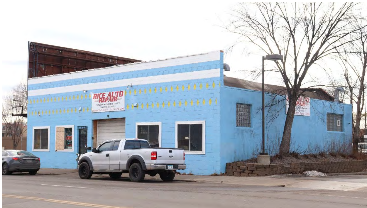
RA-SPC-11933, January 30, 2024, front (east) facade and side (north) elevation, view facing southwest.
