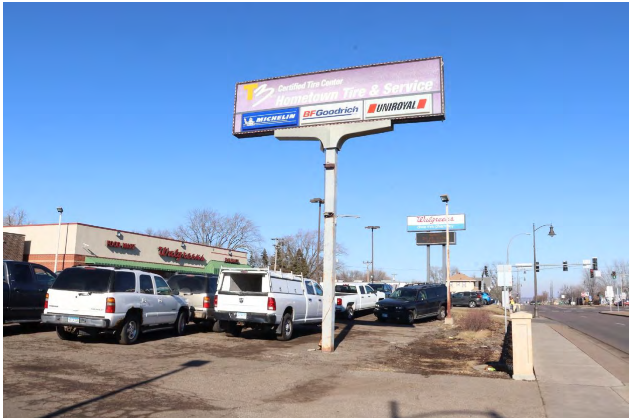
DK-WPC-00091, January 31, 2024, free standing sign, view facing north.
