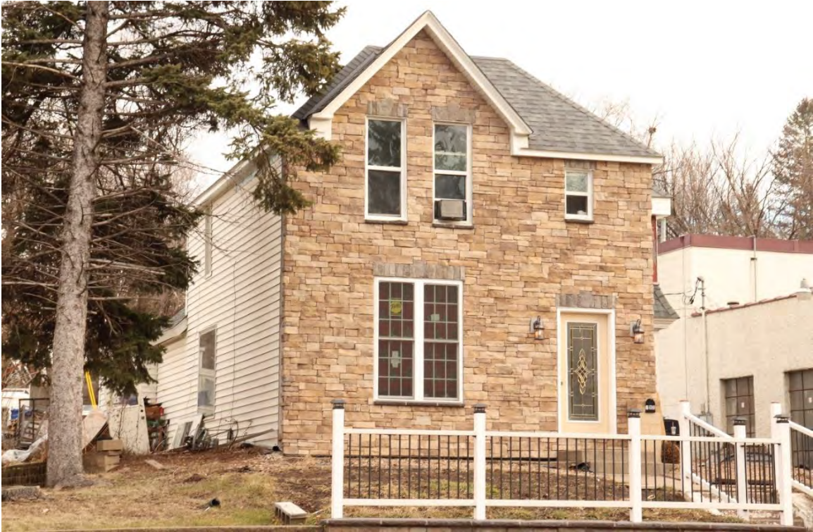
RA-SPC-09023, February 02, 2024, front (west) facade and side (north) elevation, view facing southeast.
