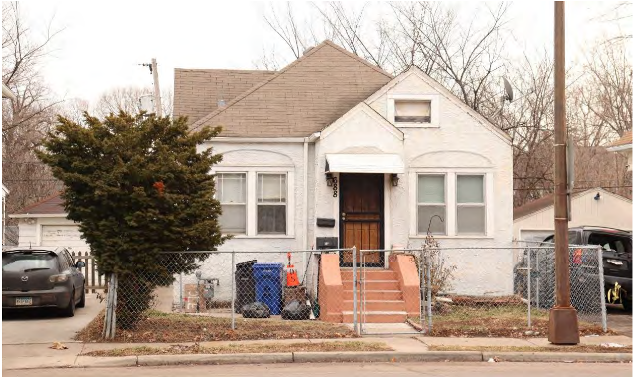
RA-SPC-08996, January 29, 2024, front (west) facade, view facing east.
