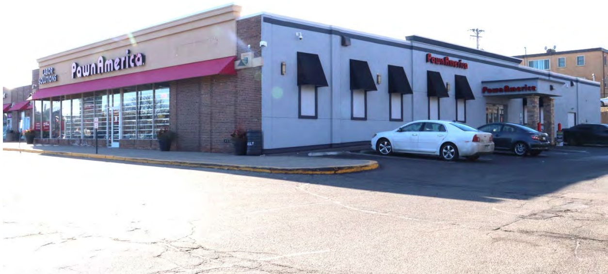
RA-RVC-00057, January 29, 2024, front (east) facade and side (north) elevation, view facing northwest.
