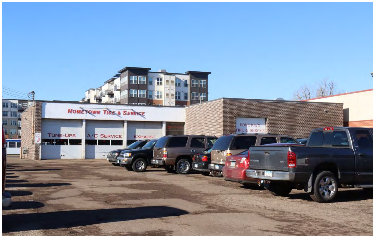
DK-WPC-00091, January 31, 2024, side (south) and rear (east) elevation, view facing northwest.
