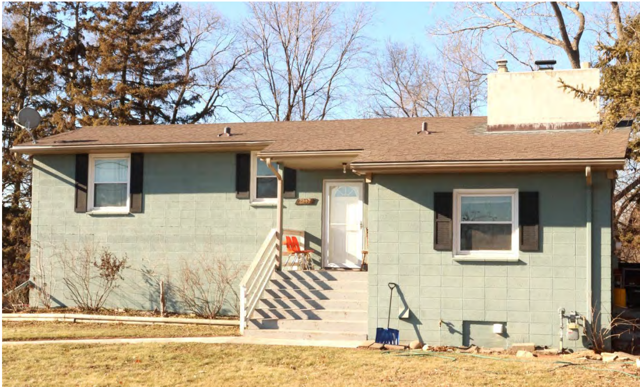
RA-RVC-00061, January 29, 2024, front (east) facade and side (north) elevation, view facing southwest.
