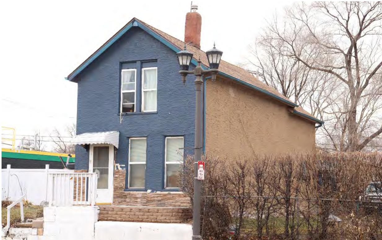
RA-SPC-03083, January 30, 2024, front (east) facade and side (north) elevation, view facing southwest.
