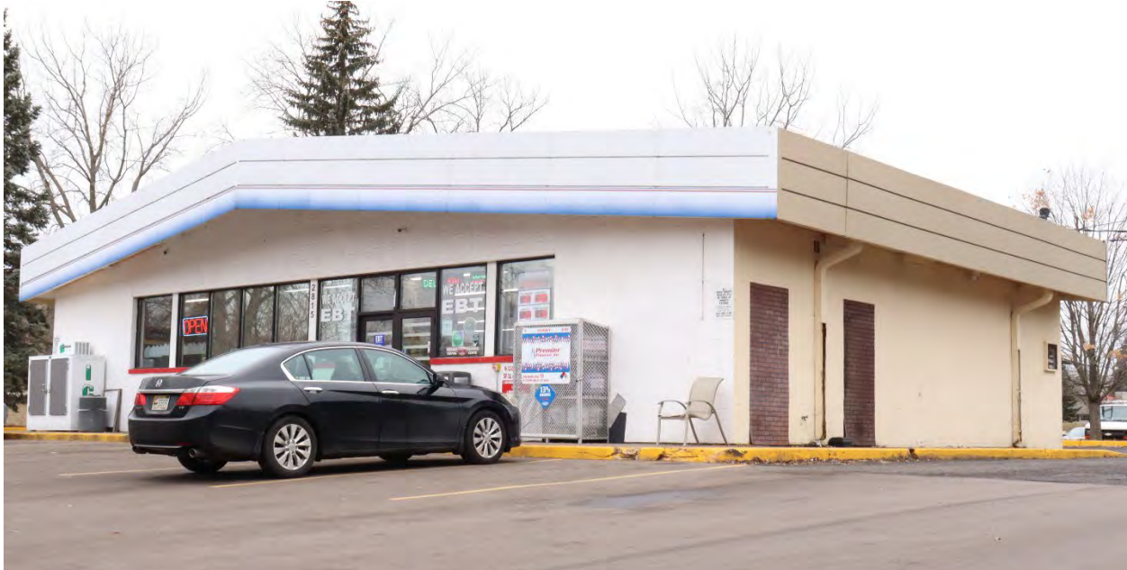
RA-RVC-00064, January 30, 2024, front (west) facade and side (south) elevation, view facing northeast.
