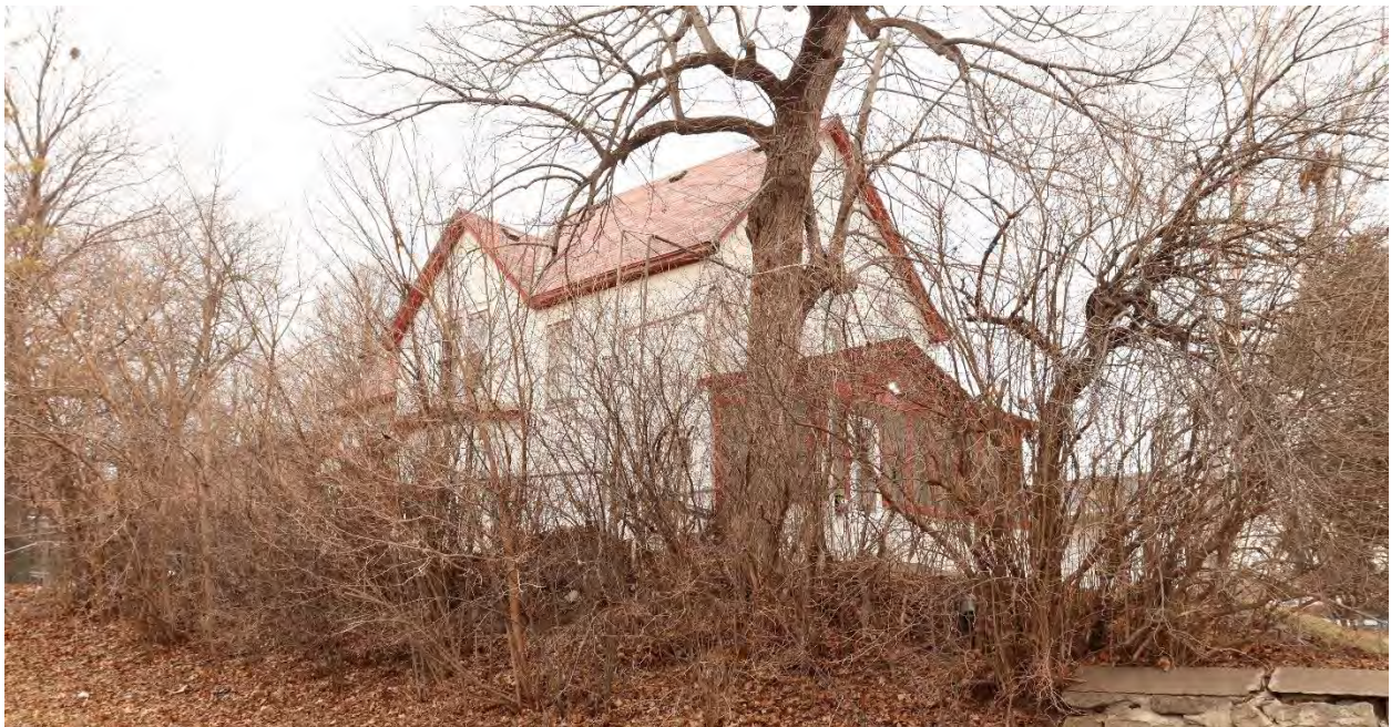
RA-SPC-09017, February 02, 2024, front (east) facade and side (south) elevation, view facing northwest.
