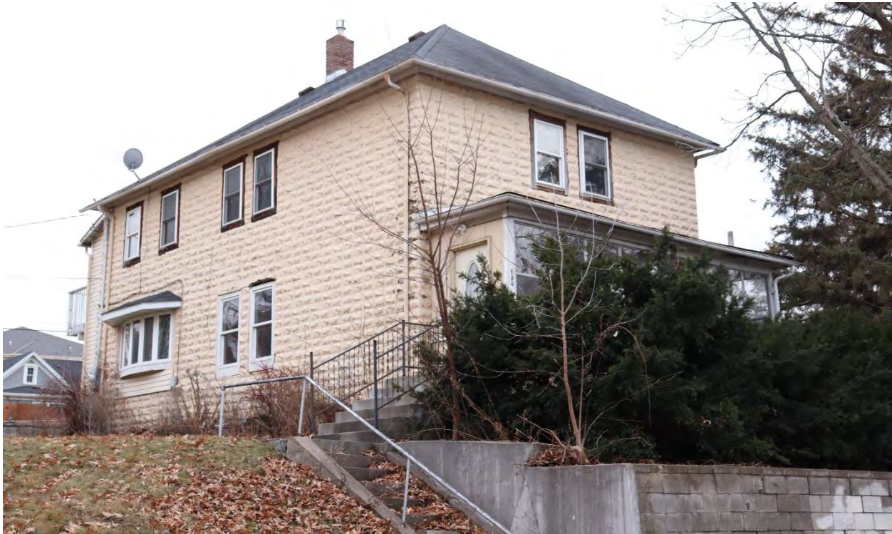
RA-SPC-11902, January 29, 2024, front (north) facade and side (east) elevation, view facing southwest.
