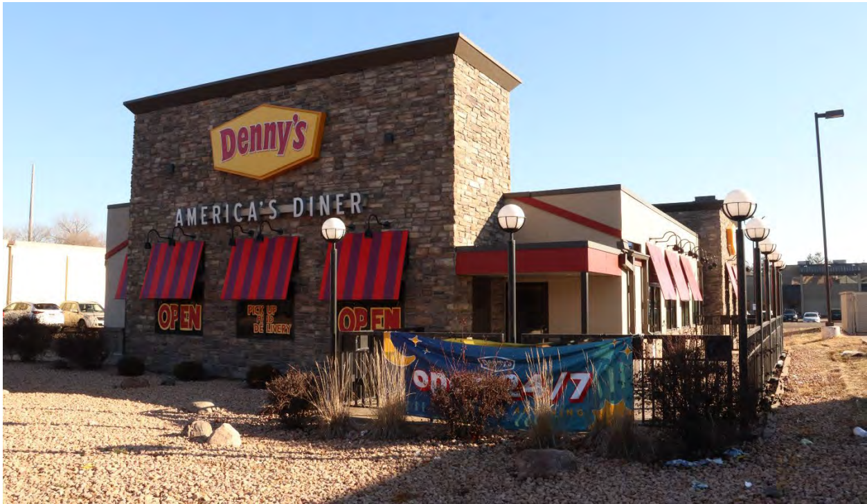
DK-WPC-00098, January 31, 2024, front (west) facade and side (south) elevation, view facing northeast.
