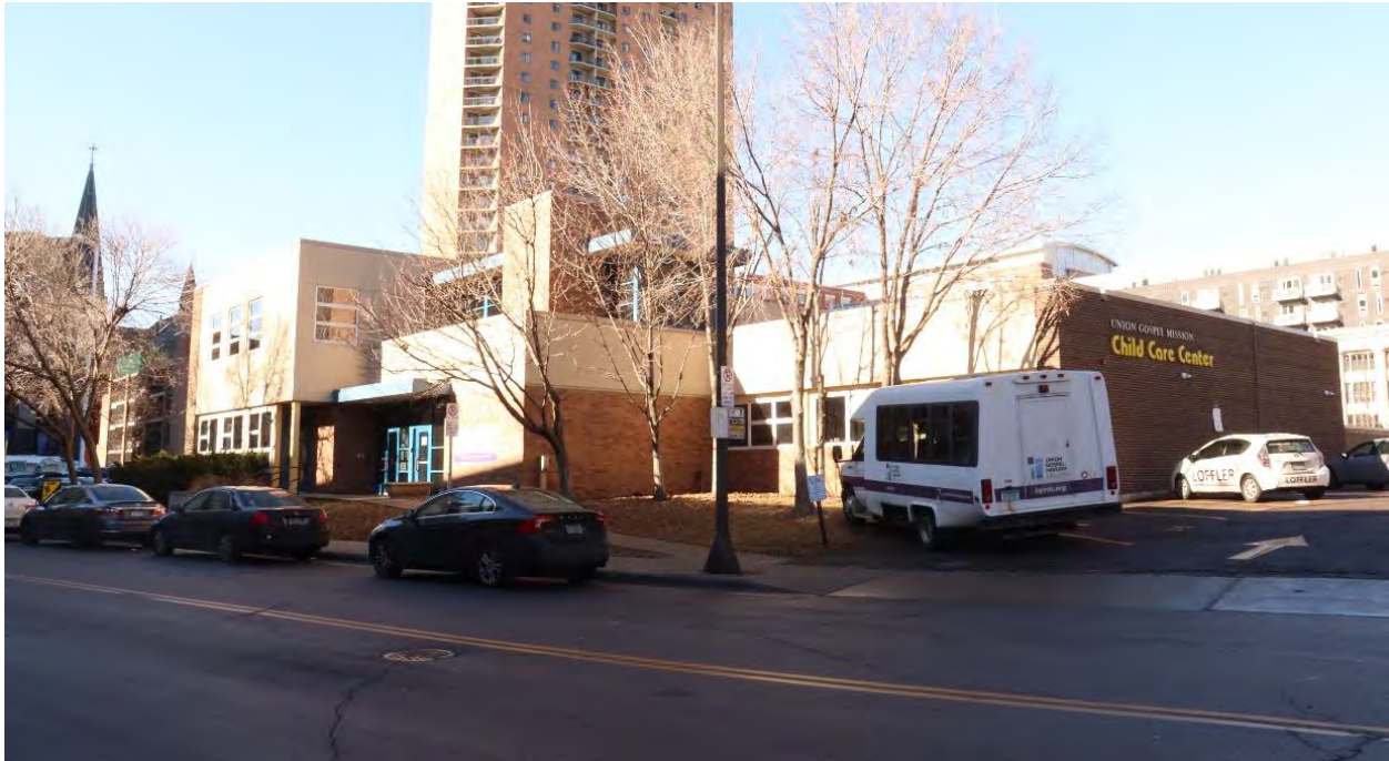
RA-SPC-08952, February 1, 2024, side (northeast) elevation, view facing west.
