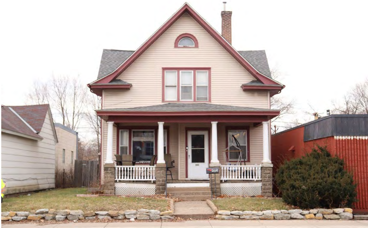
RA-SPC-03086, January 30, 2024, front (east) facade, view facing west.
