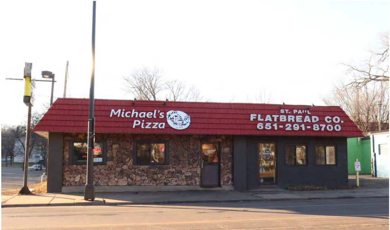
RA-SPC-11932, January 31, 2024, front (east) facade, view facing west.
