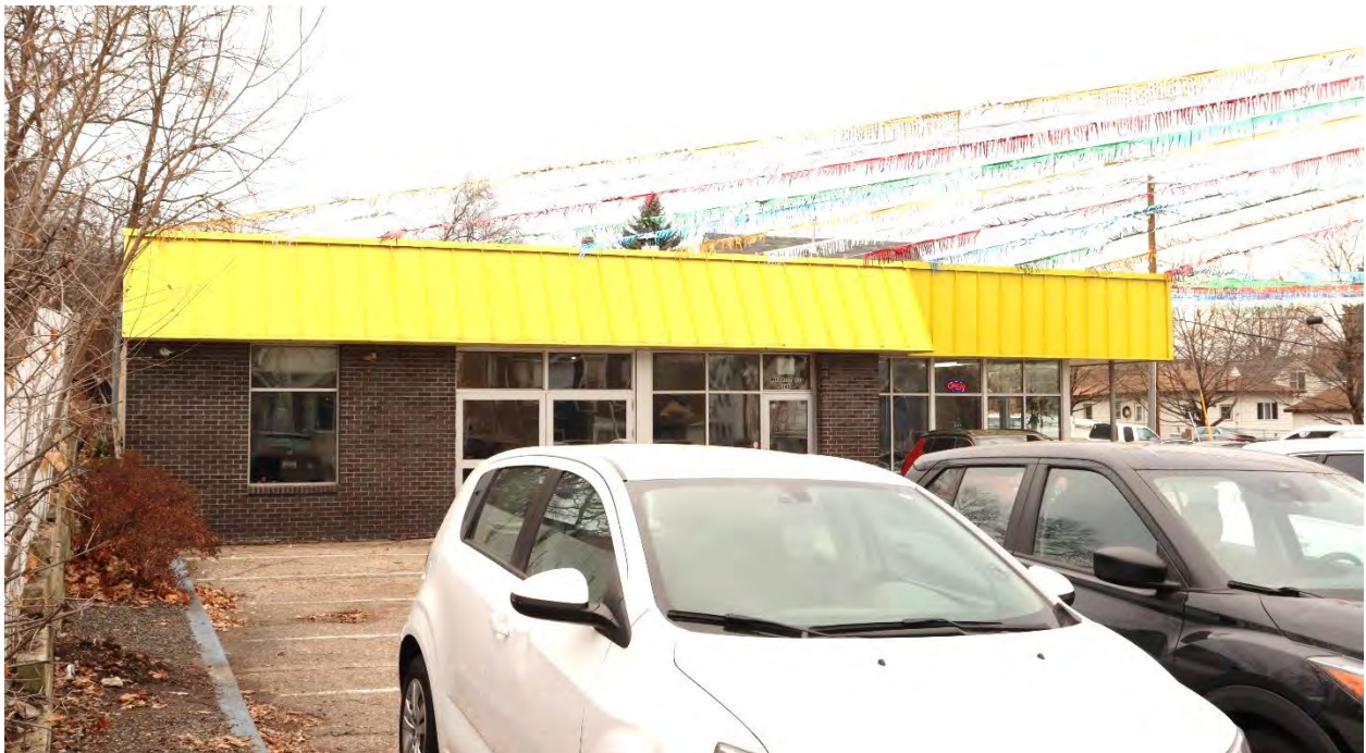
RA-SPC-09011, February 02, 2024, front (east) facade, view facing northwest.
