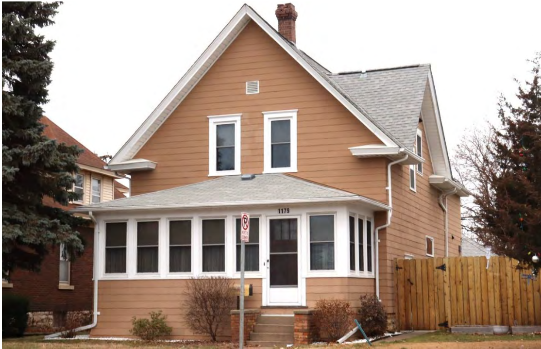
RA-SPC-11898, January 29, 2024, front (east) facade and side (north) elevation, view facing southwest.
