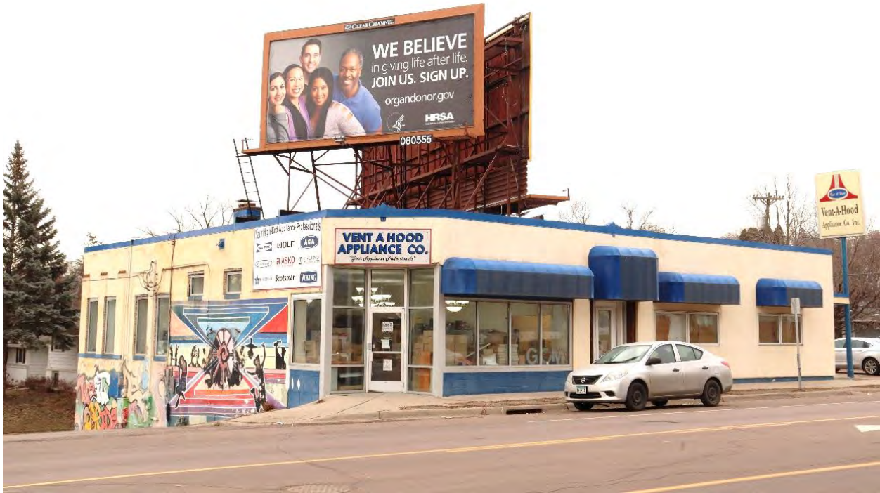
RA-SPC-09002, January 29, 2024, front (west) facade and side (north) elevation, view facing southeast.
