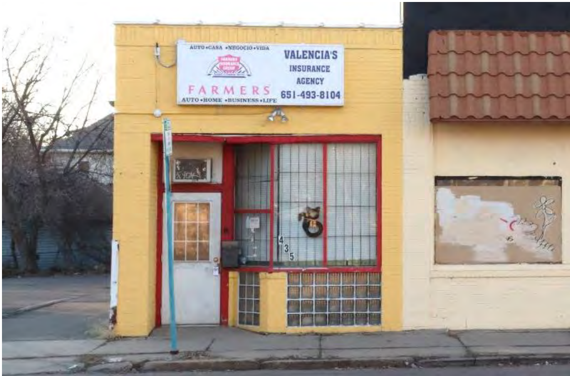
RA-SPC-08970, January 31, 2024, front (east) facade, view facing west.
