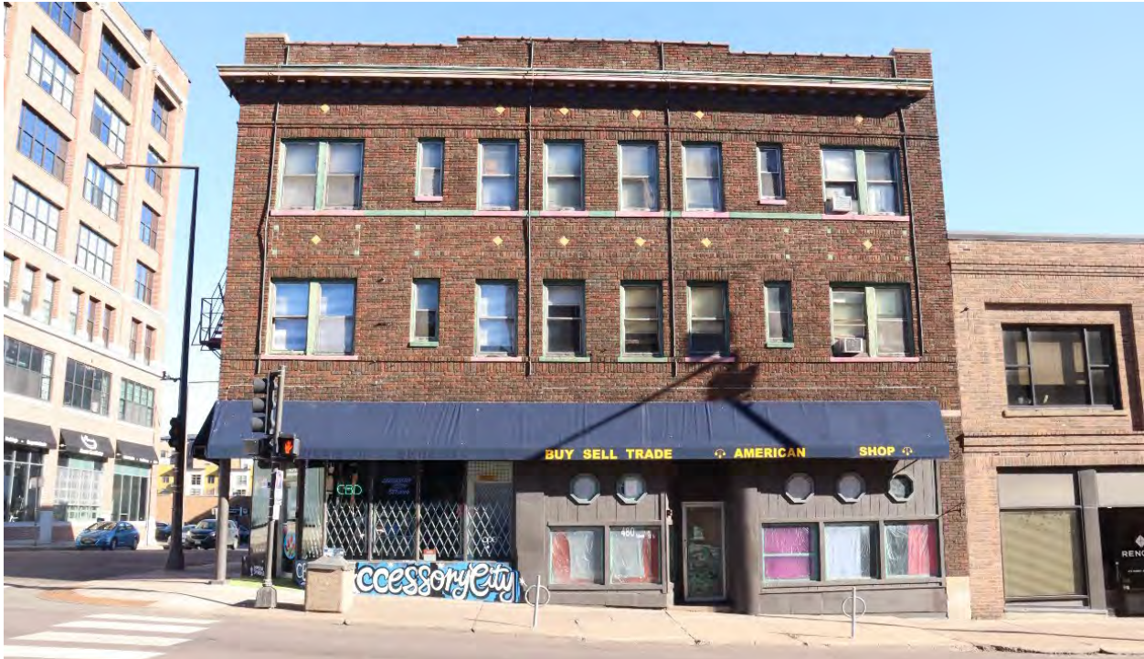
RA-SPC-03173, February 1, 2024, front (west) facade, view facing north.
