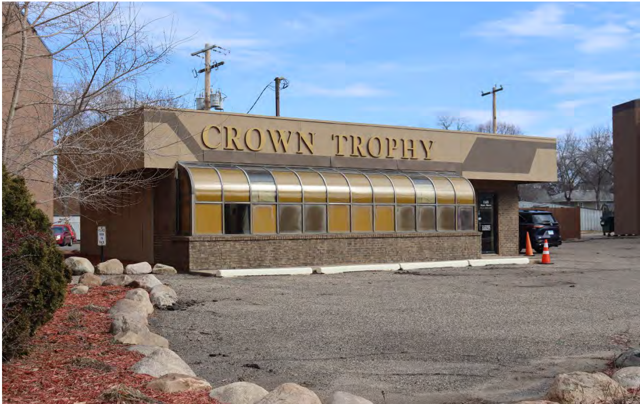
DK-WPC-00092, March 06, 2024, front (west) facade and side (north) elevation, view southeast.
