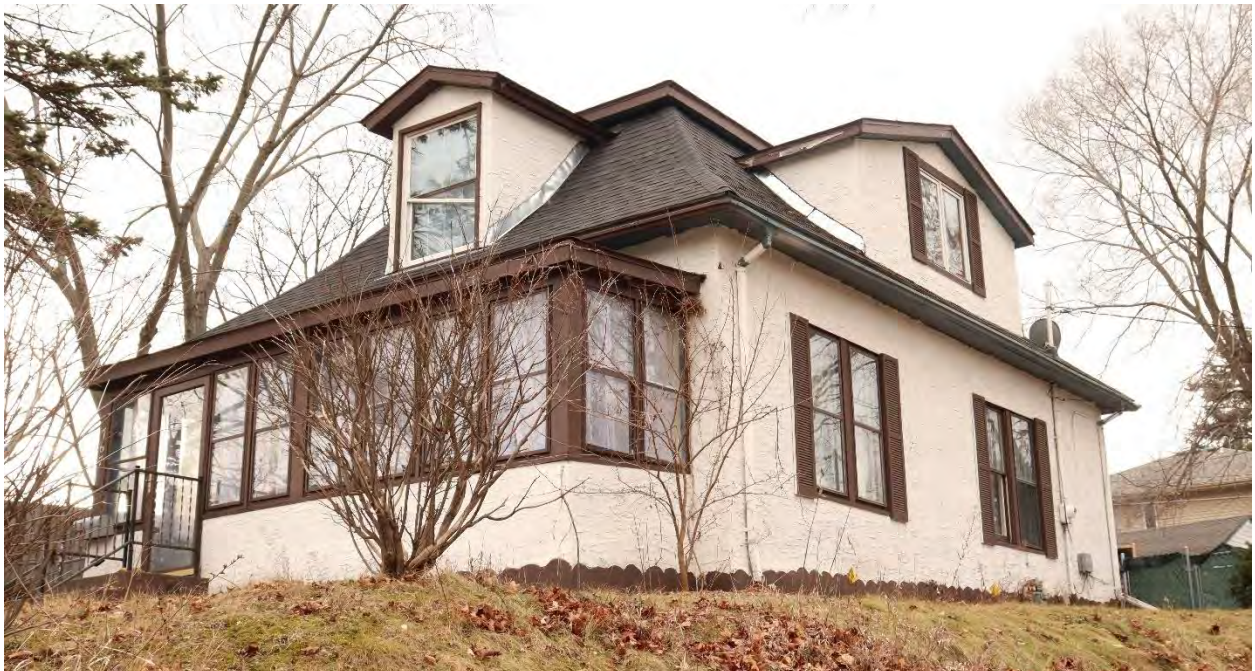
RA-SPC-09020, February 02, 2024, front (east) facade and side (north) elevation, view facing southwest.
