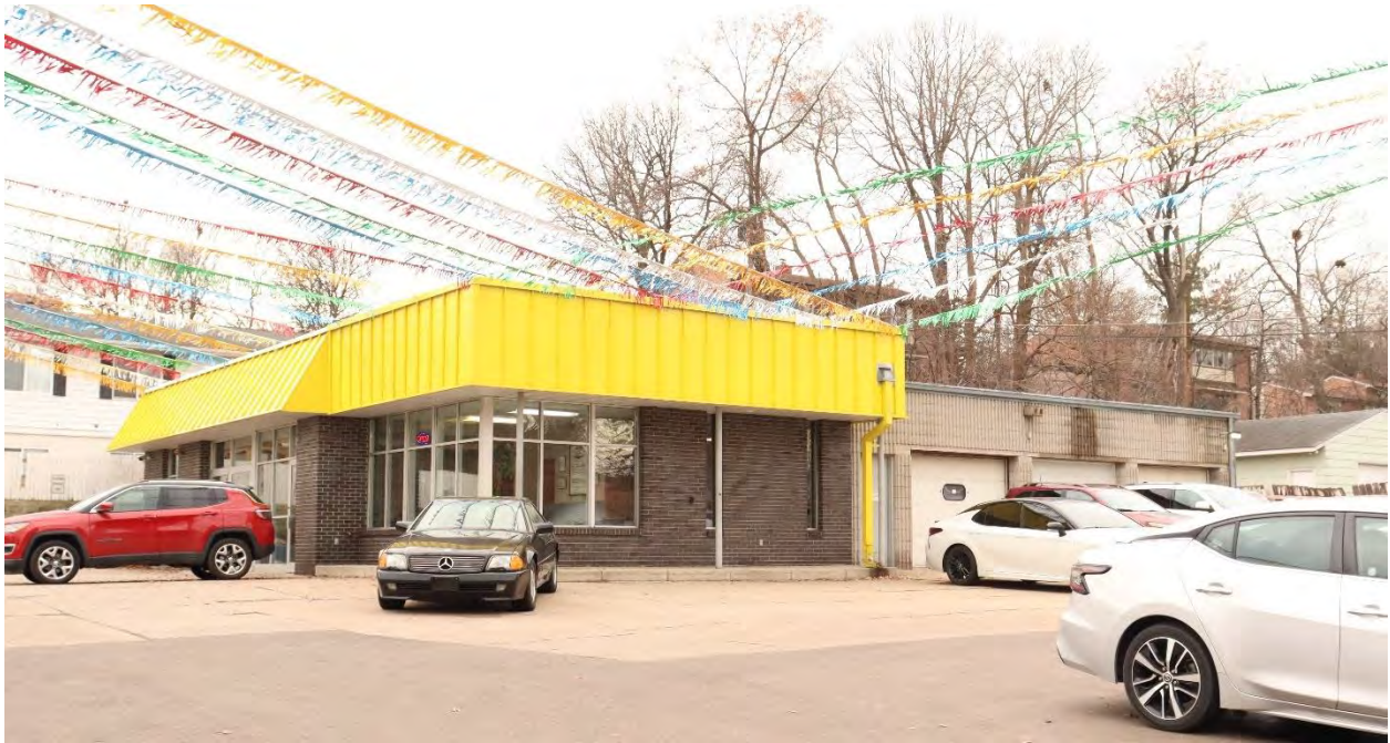
RA-SPC-09011, February 02, 2024, front (east) facade and side (north) elevation, view facing southwest.
