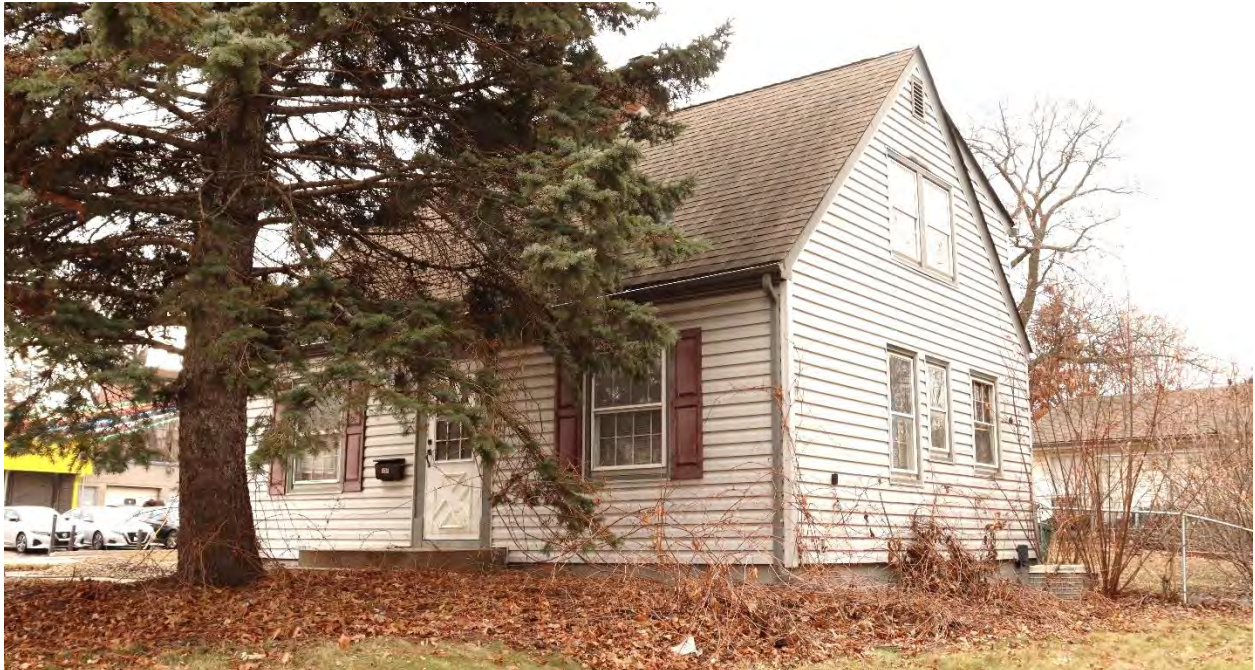
RA-SPC-09007, February 02, 2024, front (east) facade and side (north) elevation, view facing southwest.
