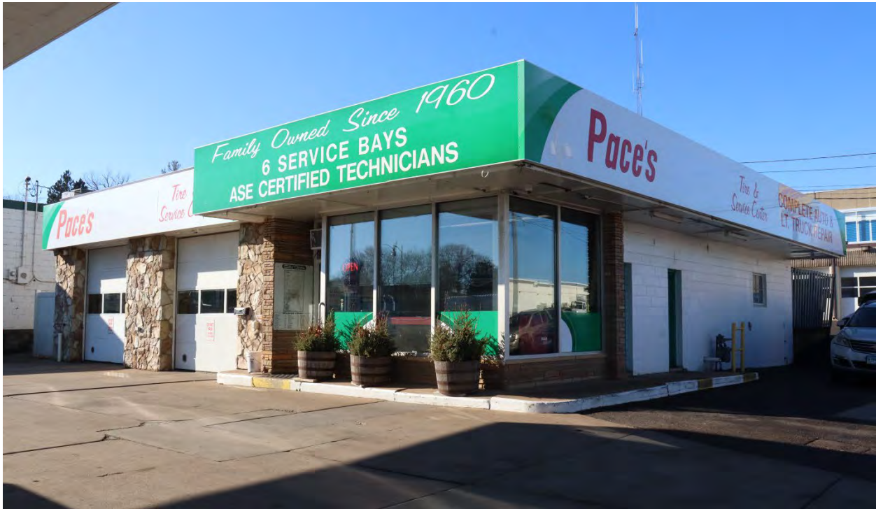
DK-WPC-00097, January 31, 2024, front (east) facade and side (north) elevation, view facing southwest.
