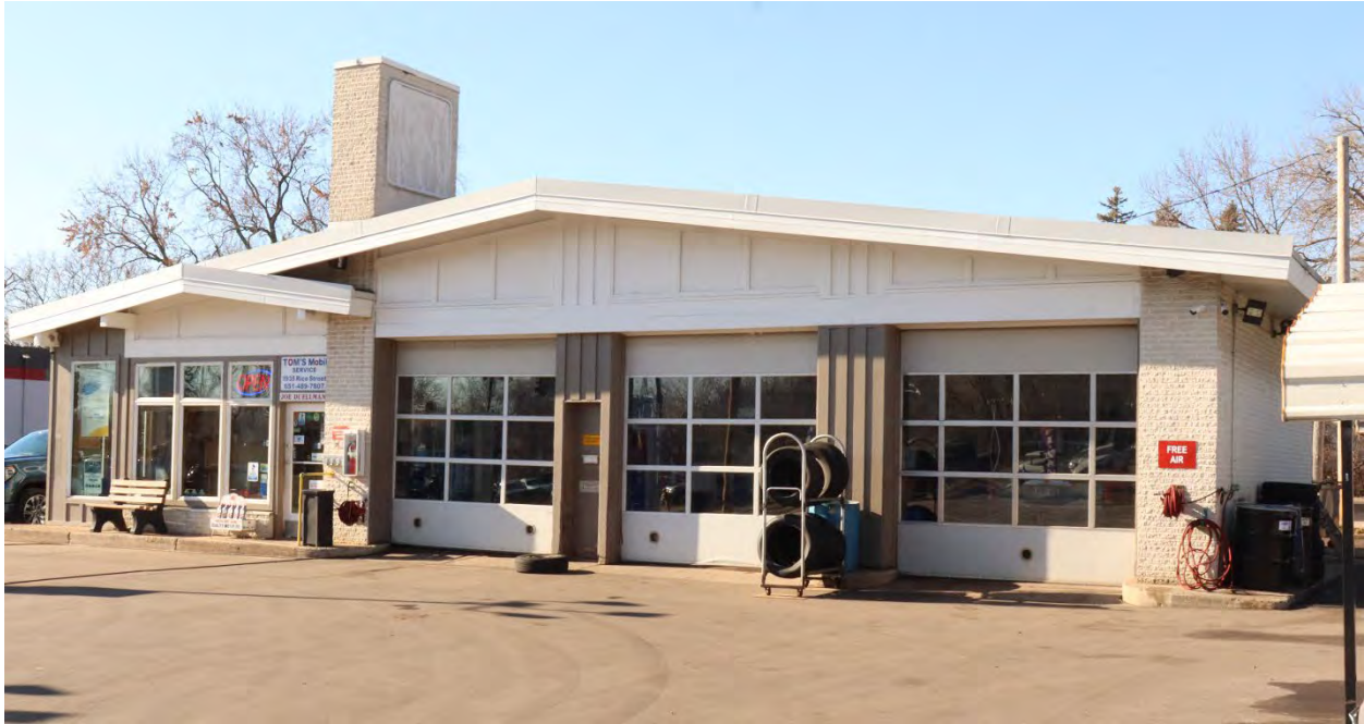
RA-RVC-00059, January 29, 2024, front (east) facade and side (north) elevation, view facing southwest.
