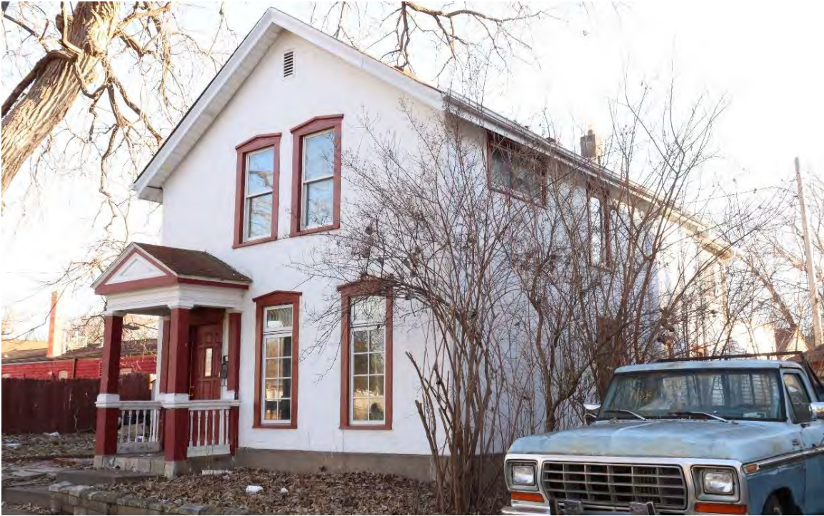
RA-SPC-11936, January 31, 2024, front (north) facade and side (west) elevation, view facing southeast.
