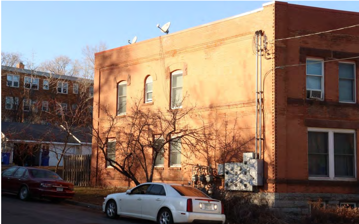
RA-SPC-03525, January 31, 2024, side (south) elevation featuring garage to the west of the building, view facing northwest.
