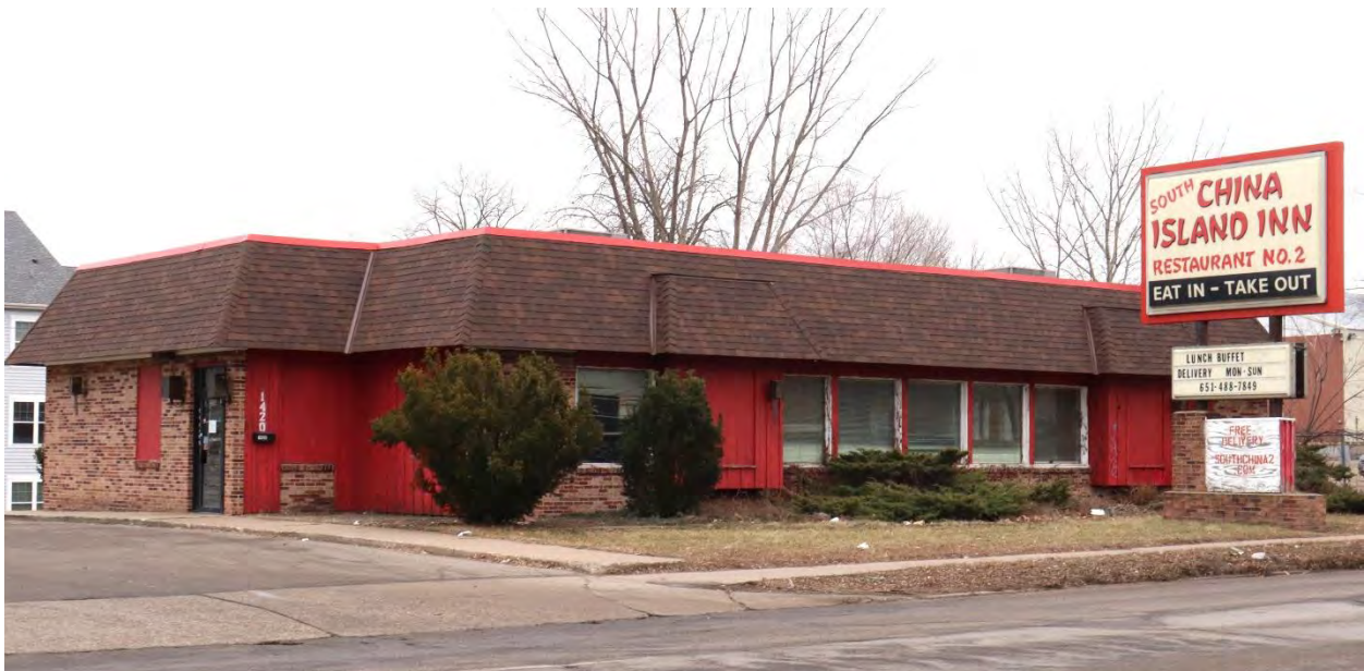
RA-SPC-11915, January 29, 2024, front (west) facade, side (north) elevation, and sign to the west of the building, view facing southeast.
