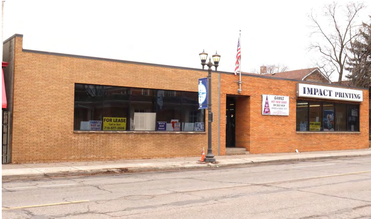
RA-SPC-11894, January 30, 2024, front (east) facade and side (south) elevation, view facing northwest.
