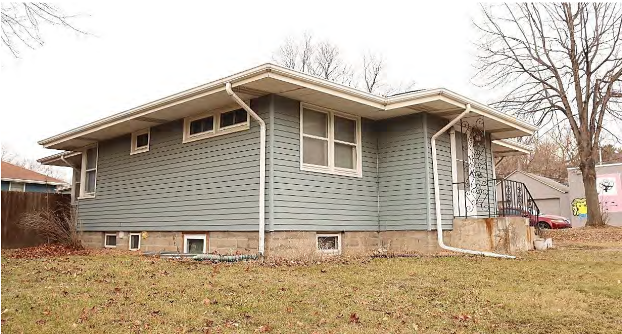
RA-SPC-09040, January 29, 2024, side (north) elevation and front (west) facade, view facing southeast.
