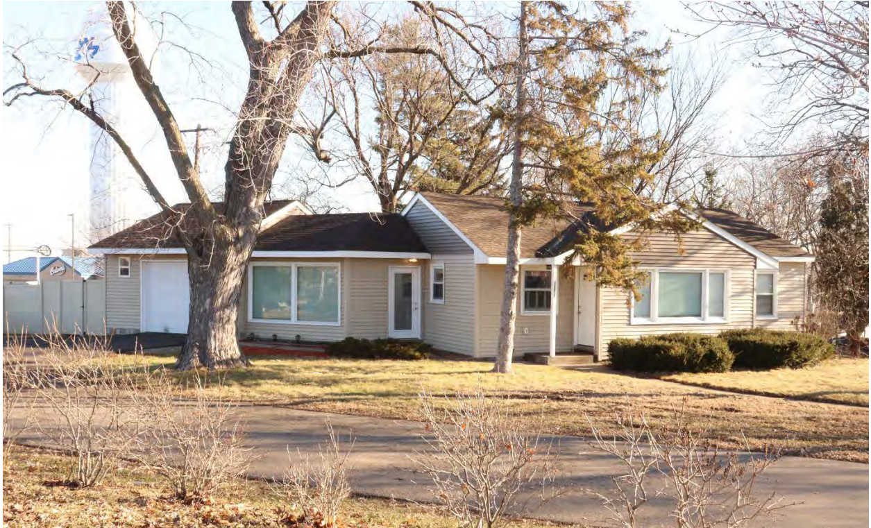
DK-WPC-00099, January 31, 2024, front (southwest) facade and side (northwest) elevation, view facing east.
