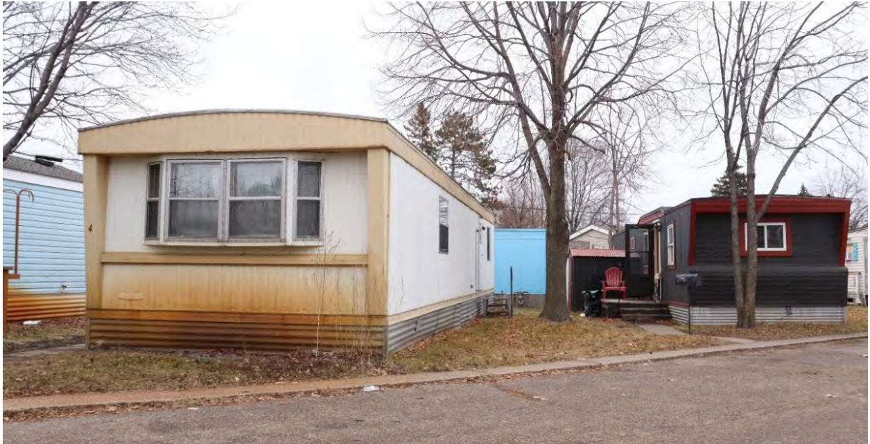
RA-LCC-00083, January 30, 2024, representative examples of ca. 1950s-1960s mobile homes on diagonal lots at southern end of mobile home park, view facing northeast.
