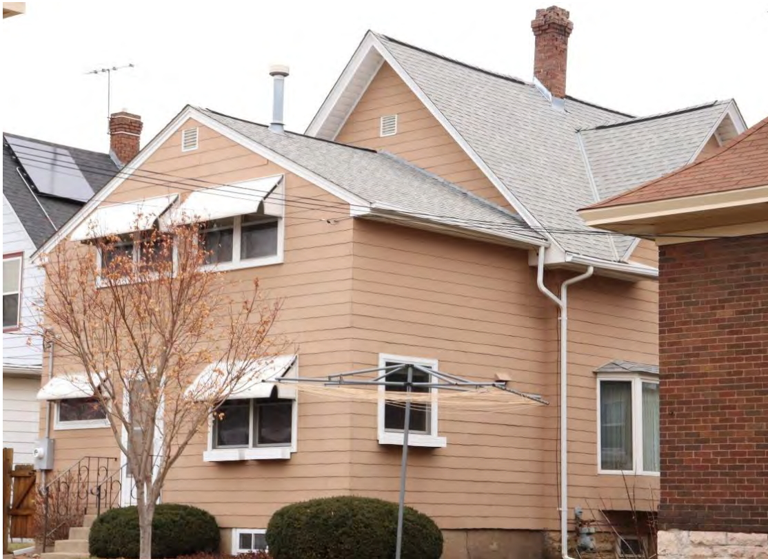
RA-SPC-11898, January 29, 2024, rear (west) elevation and side (south) elevation, view facing northeast.
