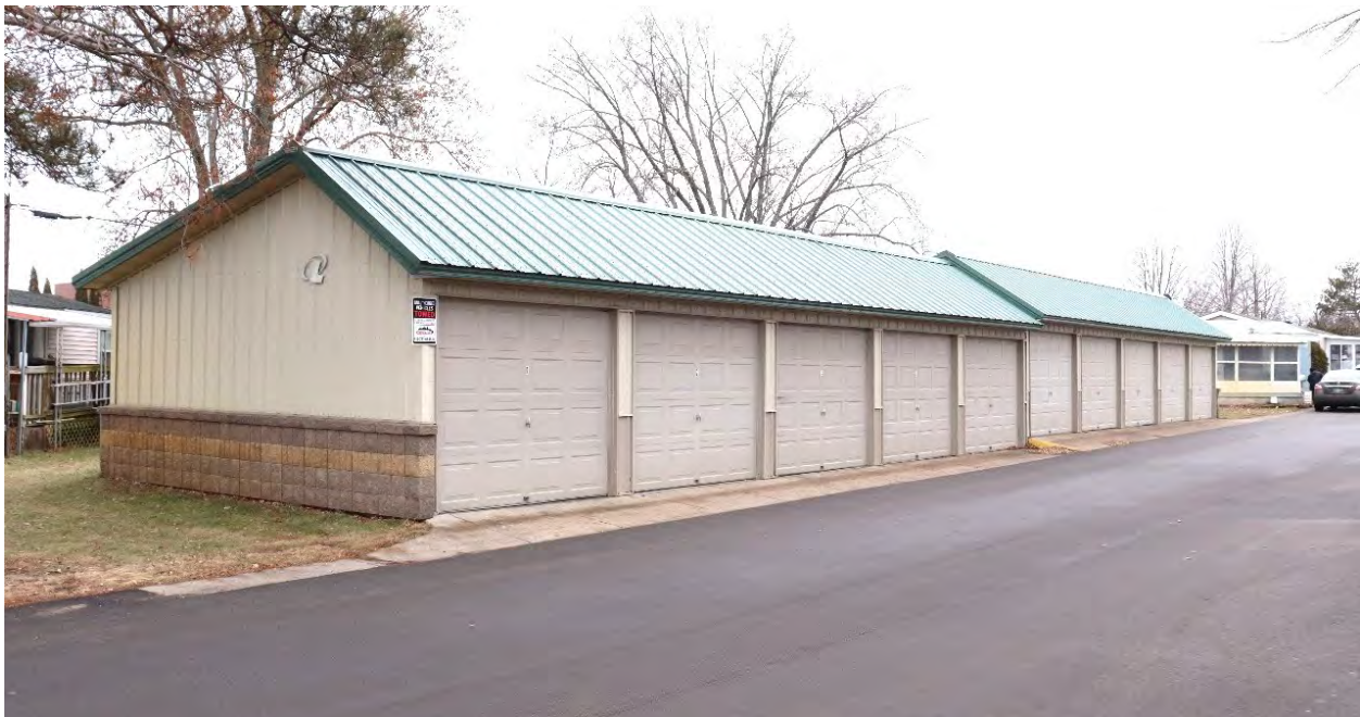
RA-LCC-00083, January 30, 2024, non-historic-age, multi-bay garages near southern end of mobile home park, view facing southwest.
