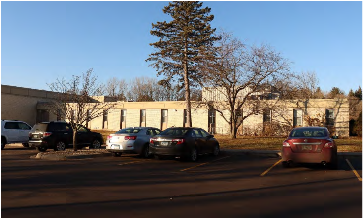
DK-WPC-00081, January 31, 2023, side (east) elevation of main block, view facing west.
