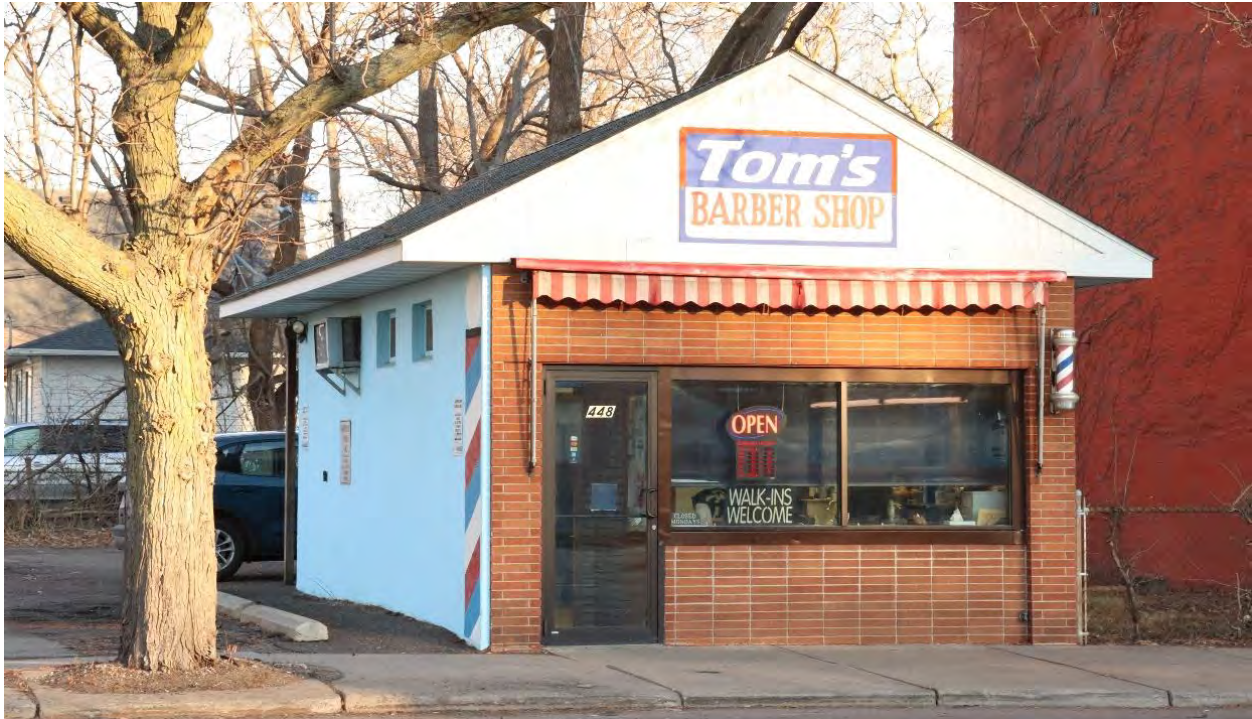
RA-SPC-08971, January 31, 2024, front (west) facade and side (north) elevation, view facing southeast.
