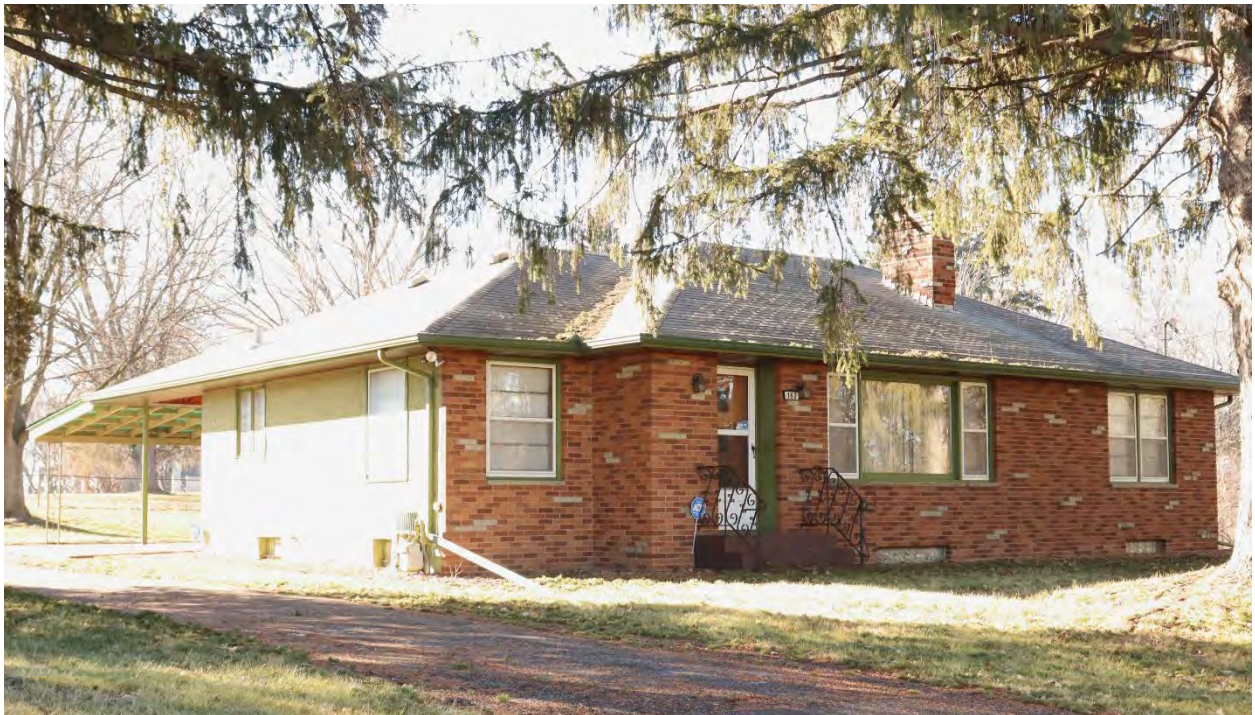
RA-RVC-00056, January 29, 2024, front (north) facade and side (east) elevation of home, view facing southwest.
