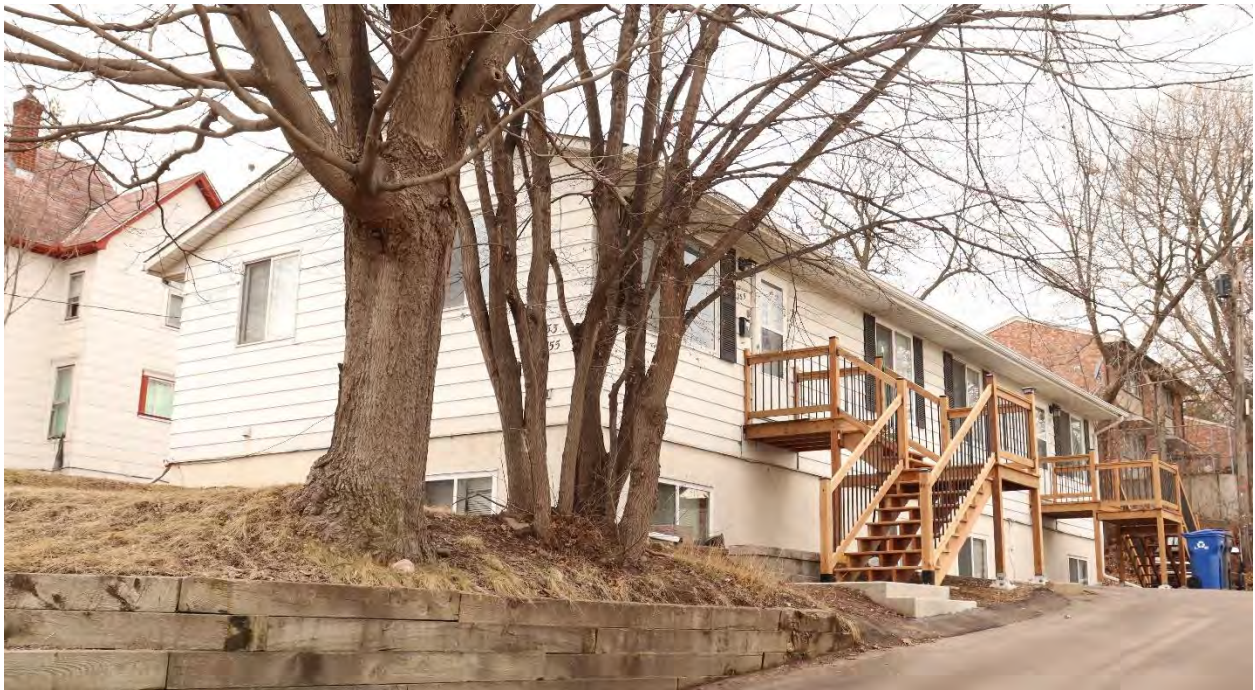
RA-SPC-09014, February 02, 2024, front (north) facade and side (east) elevation, view facing southwest.
