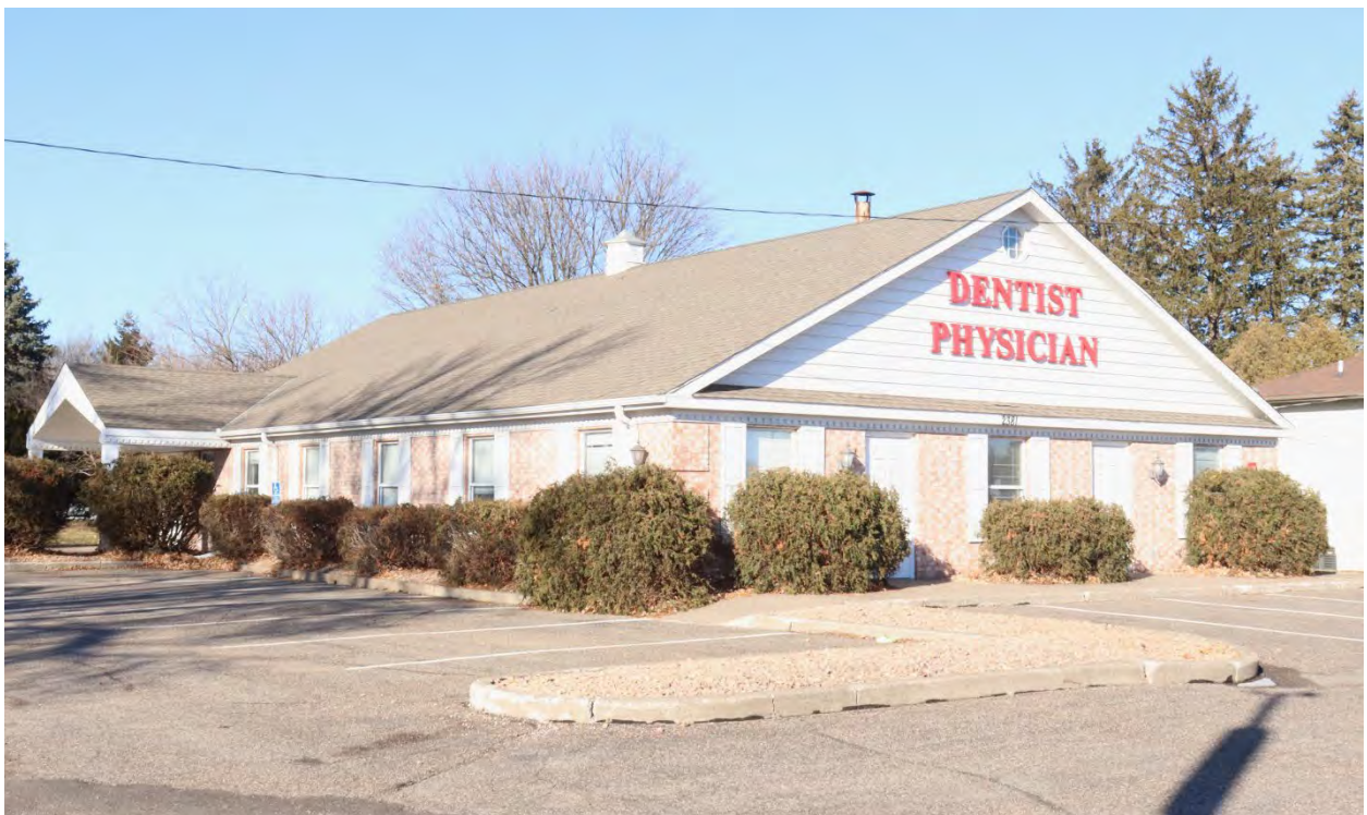
RA-RVC-00062, January 29, 2024, front (south) facade and side (east) elevation, view facing northwest.
