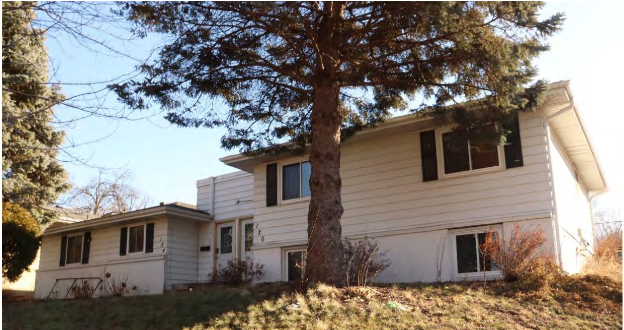
RA-SPC-11904, January 31, 2024, front (north) facade, view facing southeast.
