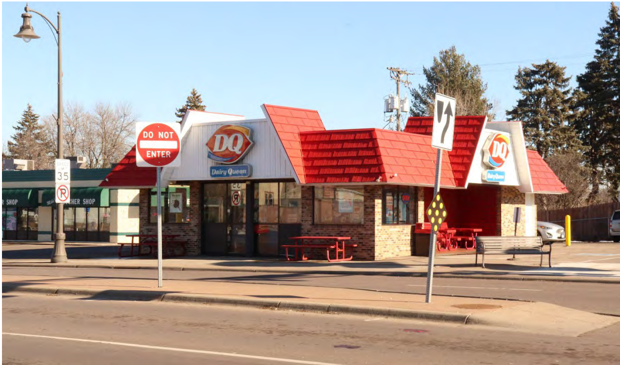
DK-WPC-00088, January 31, 2024, front (south) facade and side (west) elevation, view facing northeast.
