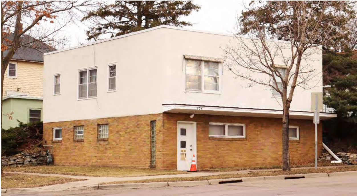
RA-SPC-09037, January 29, 2024, front (west) facade and side (north) elevation, view facing southeast.
