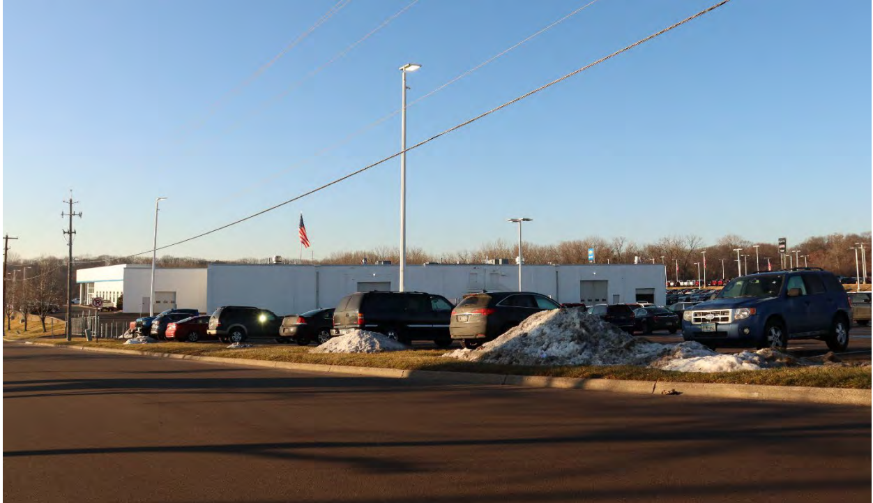
DK-IVG-00063, January 31, 2024, rear (southwest) facade and side (southeast) elevation, view facing northwest.
