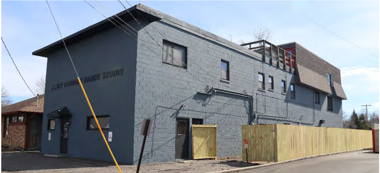
DK-WPC-00093, March 6, 2024, Front (north) facade and side (west) elevation featuring three-story, neo-mansard roofed portion, view facing southeast.
