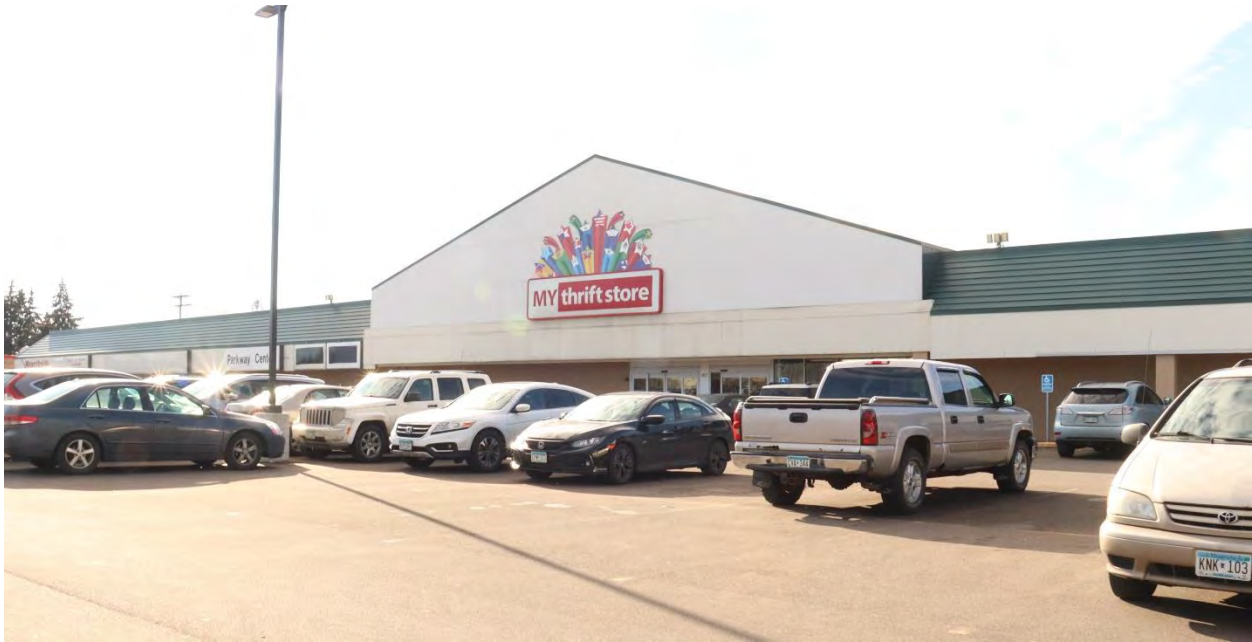
RA-SPC-11892, January 29, 2024, front (east) facade, view facing southwest.
