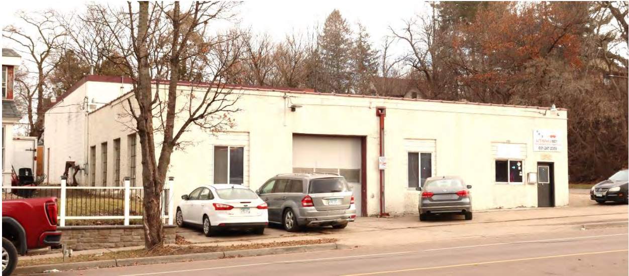
RA-SPEC-09024, February 02, 2024, front (west) facade, side (north) elevation, and rear (east) addition, view facing southeast.
