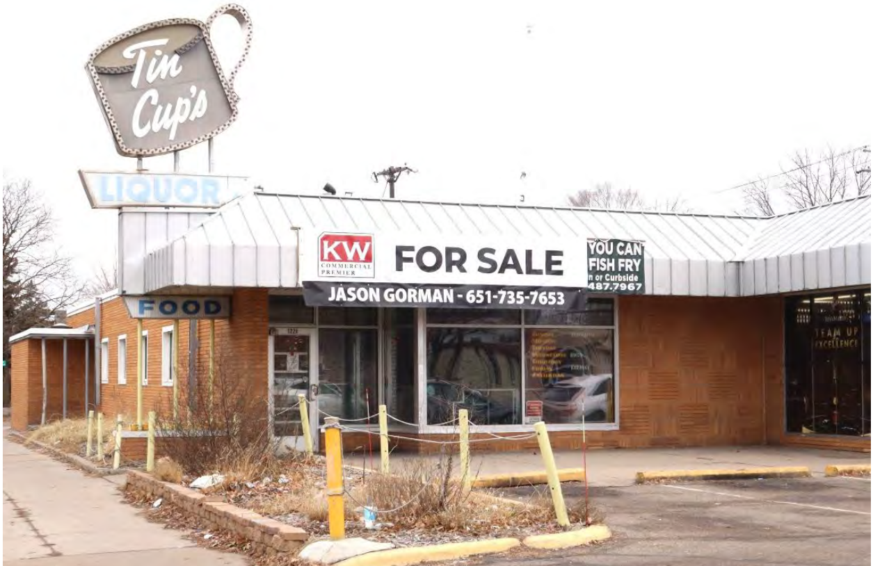
RA-SPC-11568, January 29, 2024, front (south) facade and side (west) elevation of the western portion, view facing north.
