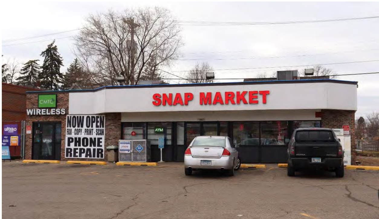
RA-SPC-11938, January 30, 2024, Front (east) facade, view facing west.
