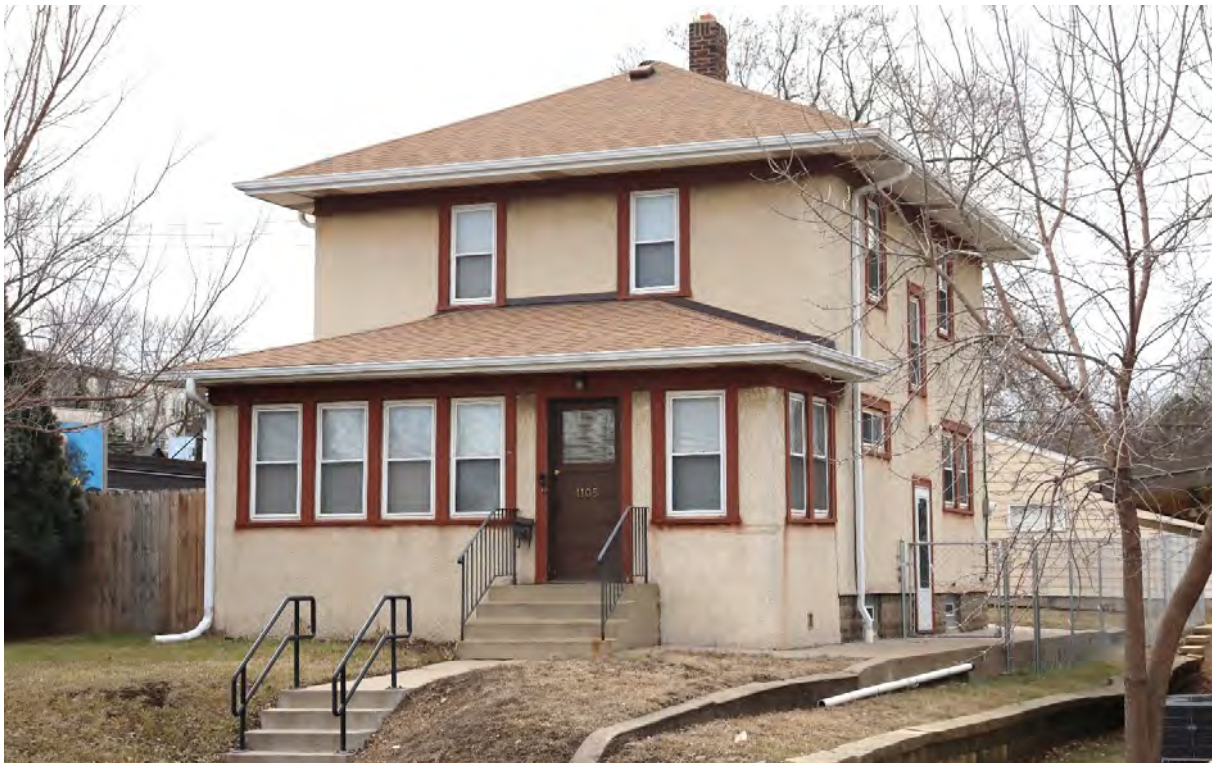
DK-WPC-00087, March 06, 2024, front (east) facade, side (north) elevation, and garage in rear, view facing southwest.
