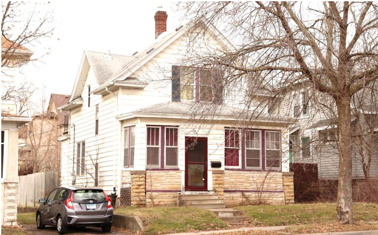
RA-SPC-09015, January 31, 2024, front (west) facade and side (north) elevation, view facing southeast.
