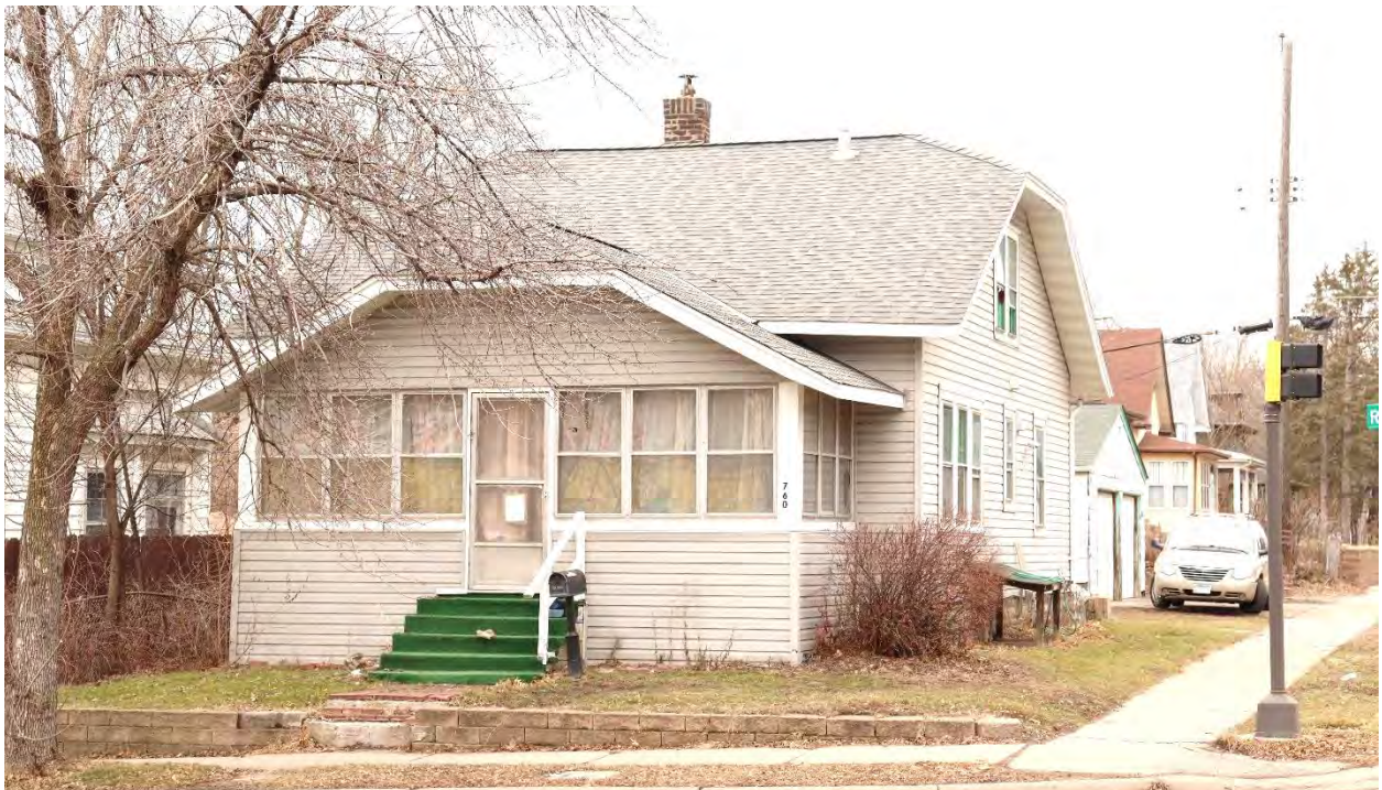
RA-SPC-09016, February 02, 2024, front (west) facade, side (south) elevation, and garage, view facing northeast.
