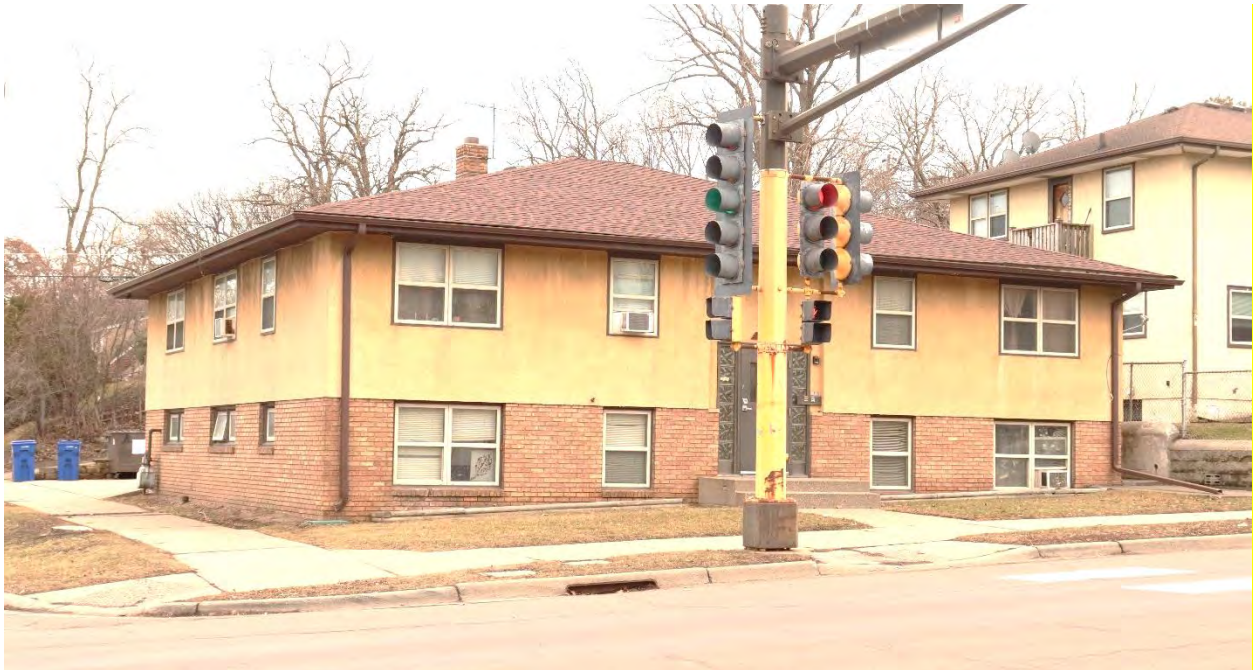
RA-SPC-09018, February 02, 2024, front (west) facade and side (north) elevation, view facing southeast.
