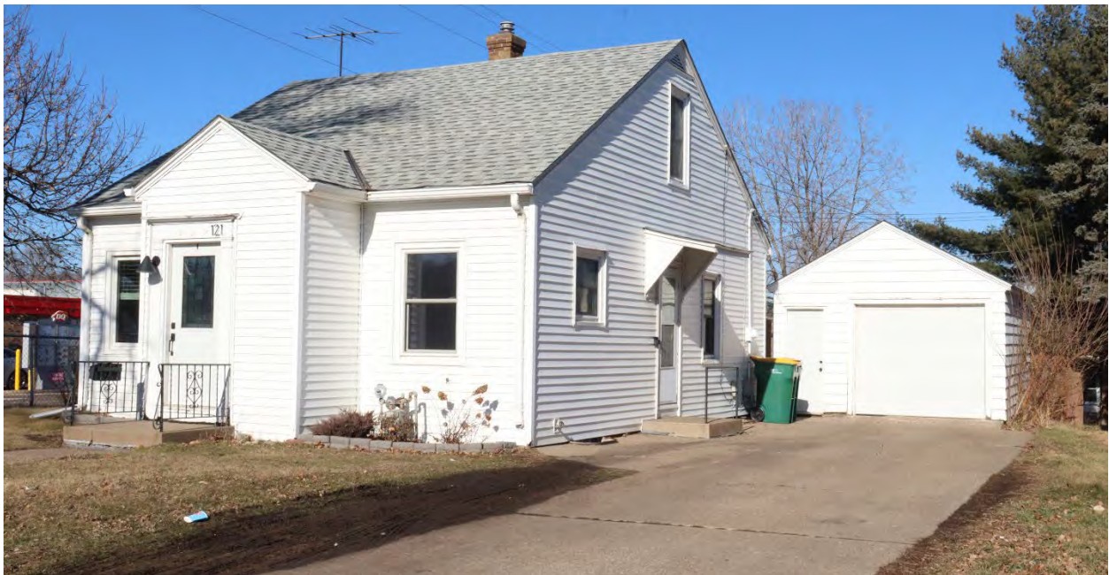
DK-WPC-00094, January 31, 2024, front (south) facade and side (east) elevation with garage, view facing northwest.
