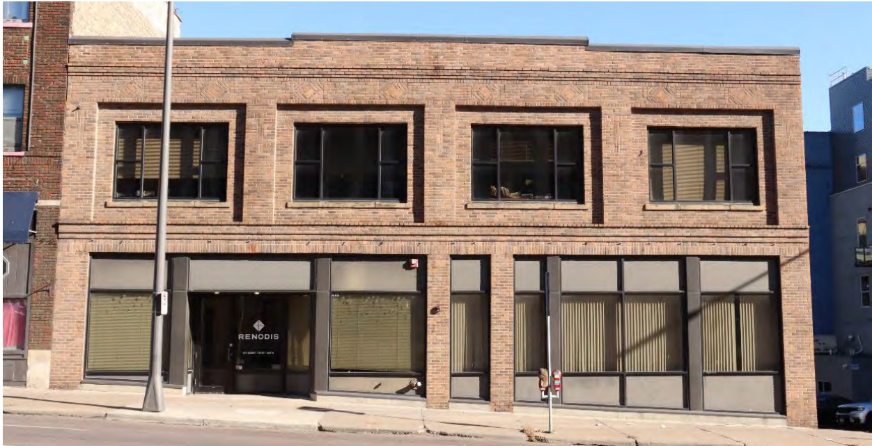
RA-SPC-03172, February 1, 2024, front (west) facade, view facing east.
