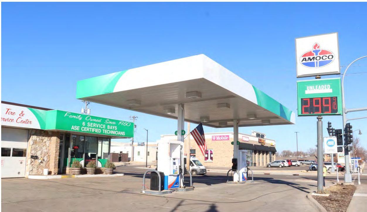
DK-WPC-00097, January 31, 2024, free-standing canopy, view facing southwest.
