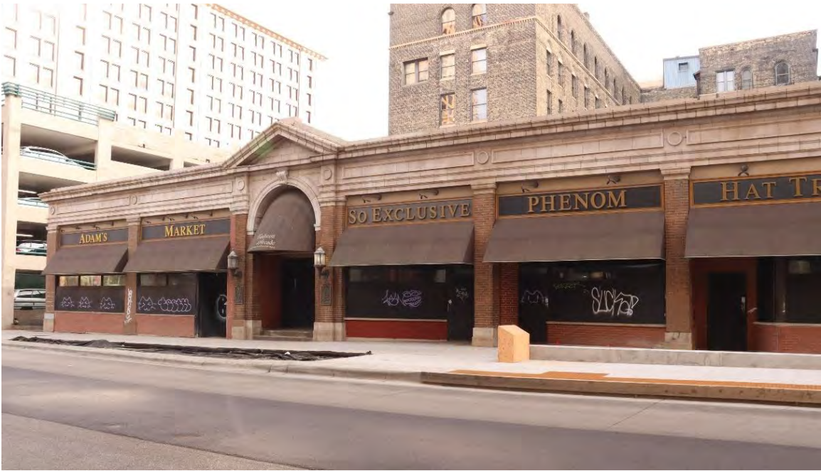
Figure 50. National Register-listed Endicott Arcade Addition, facing northeast from 5th Street East.
