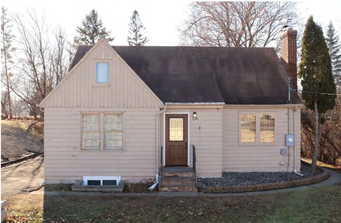
Figure 13. Minimal Traditional House, facing south from County Road B West.
