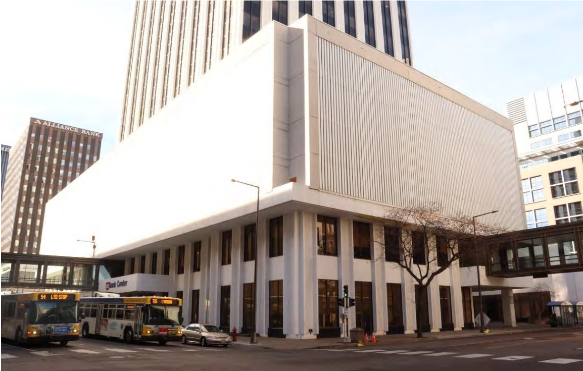
Figure 48. American National Bank (now US Bank Center), facing west from the Robert Street North and 5th Street East intersection.
