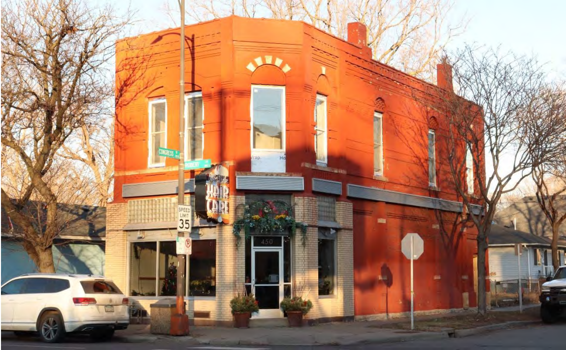
Figure 63. West (front) facade and south (side elevation) of Schulz Building, facing northeast from the intersection of Robert Street South and Congress Street East.
