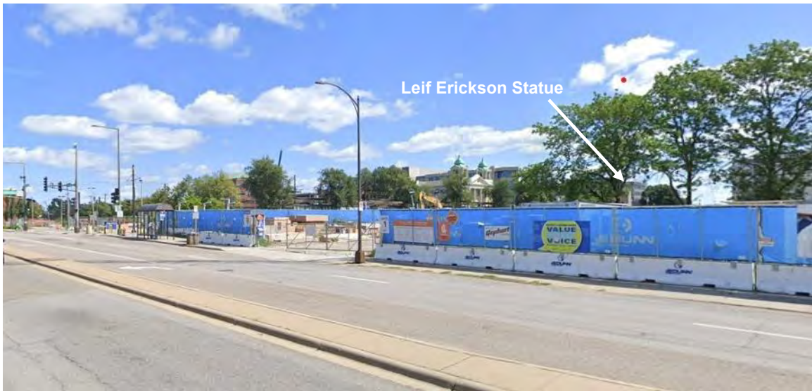
Figure 28. Google Street View imagery (August 2024) showing general location of Leif Erickson Lawn and Statue currently under construction, facing northeast from Rice Street toward University Avenue.
