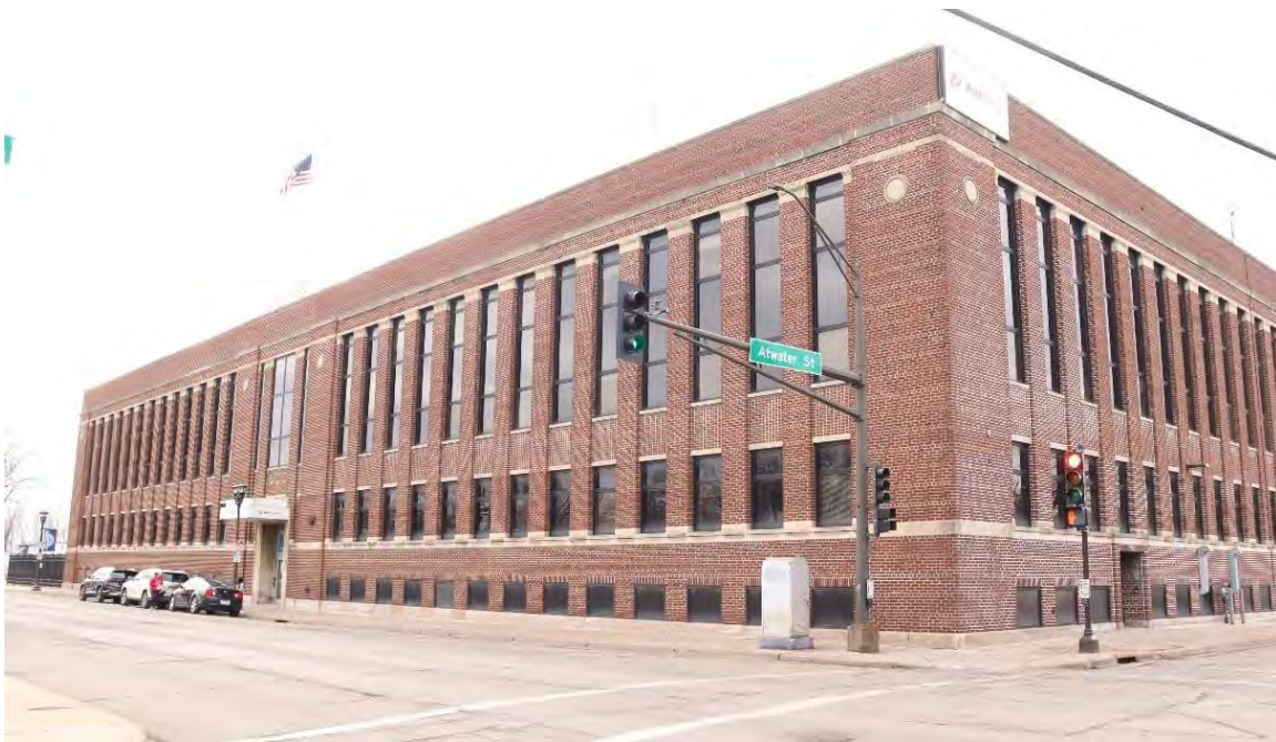
Figure 17. Front (east) facade and side (north) elevation of the Saint Paul Gas Light Company Service Station building in area of proposed station location, facing southwest from Rice Street.
