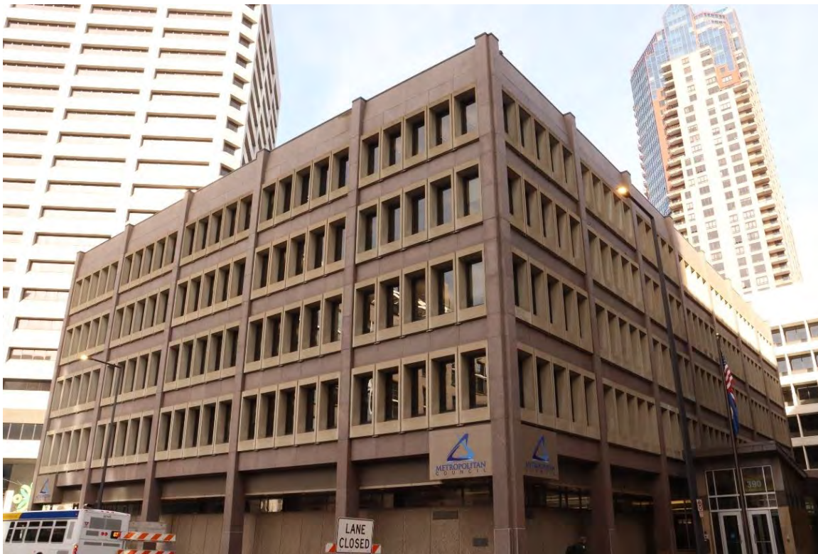
Figure 47. Minnesota Department of Economic Security Building (currently Metropolitan Council), facing north from Robert Street North.
