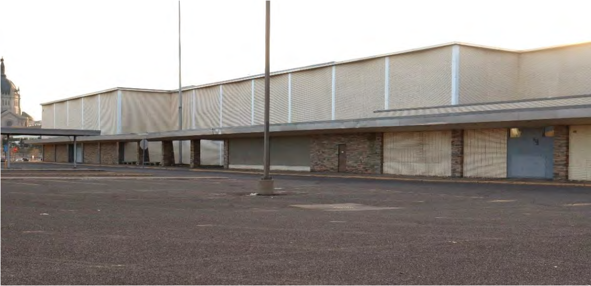
Figure 38. Side (east) elevation of Sears Retail Store, facing southwest from the parking lot adjacent to the west side of Rice Street.
