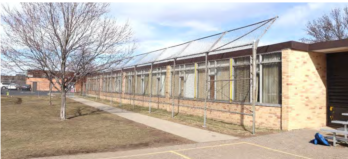
Figure 22. Rear (west) elevation of 1961 linear classroom addition, view facing northeast.
