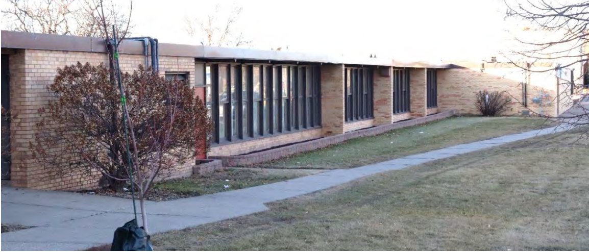
Figure 16. Facade of 1953 addition (left) and 1958 addition (center and right), view facing northwest.
