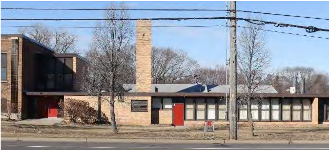
Figure 10. Front (east) facade of 1953 addition at north end of original 1935 school building, view facing west.
