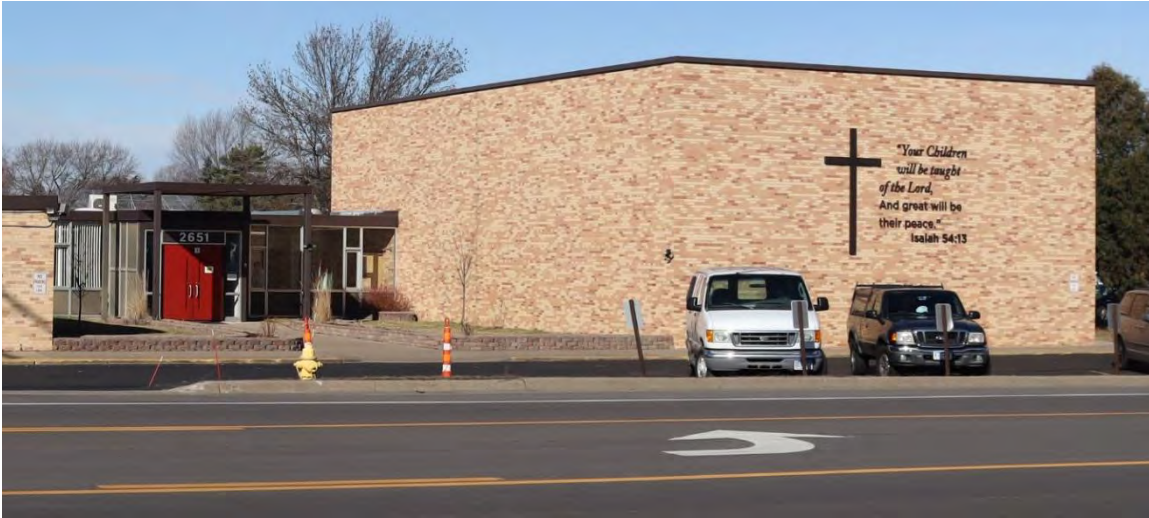
Figure 27. Side (south) elevation and front (east) facade of 1975 gymnasium addition (right) immediately north of 1961 addition and entrance (left), view facing northwest.
