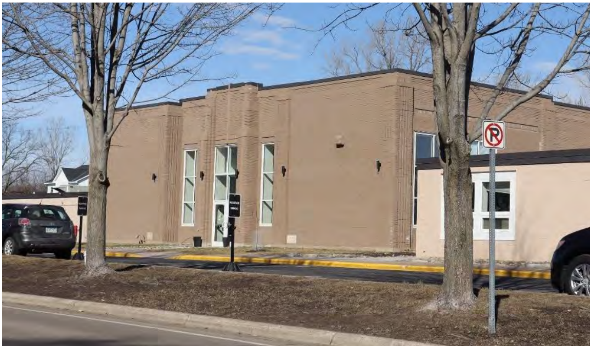
Figure 37. McCarrons Lake School (Hand in Hand Christian Montessori School) with recent facade alterations, view facing northwest.
