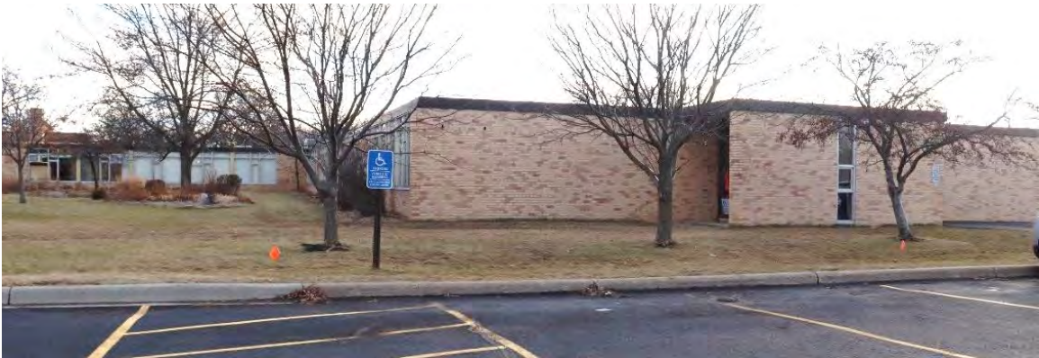
Figure 24. Side (north) elevation of 1961 linear classroom addition (right) and library hyphen addition (background left), view facing south.
