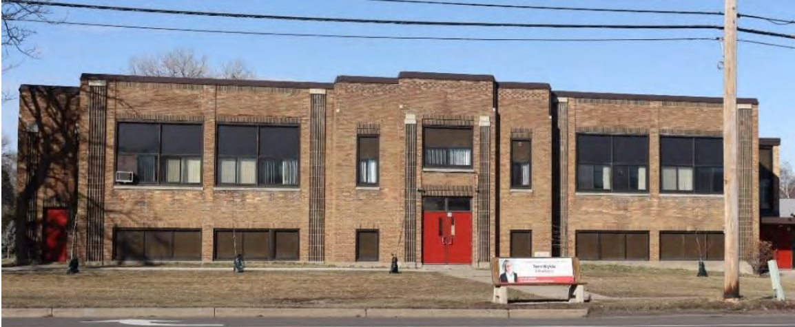
Figure 4. Facade of original 1935 North Heights School, view facing west.
