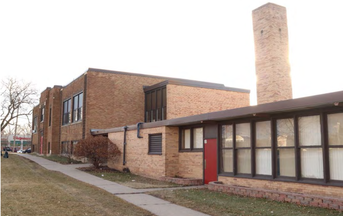
Figure 13. Facade of 1953 addition with original 1935 school building (left), view facing southwest.
