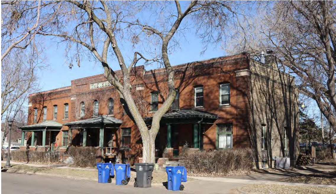
Figure 41. Front (south) facade and side (east) elevation, view toward northwest.
