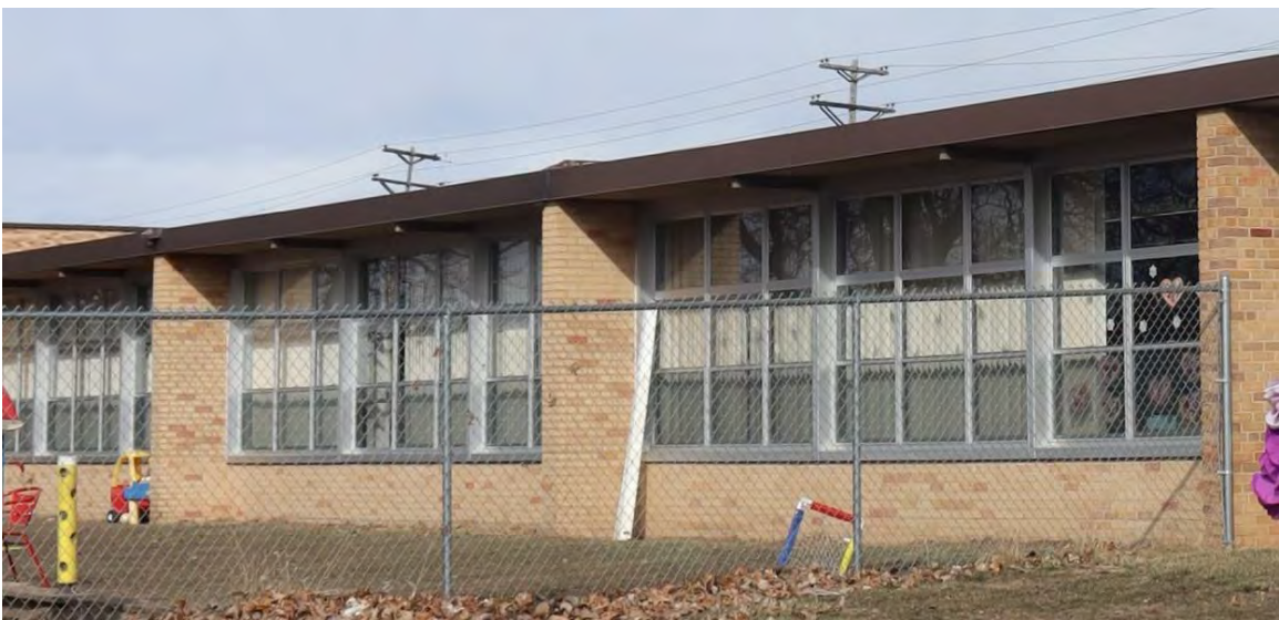
Figure 18. Rear (west) elevation of 1958 addition with replacement windows, view facing northeast.
