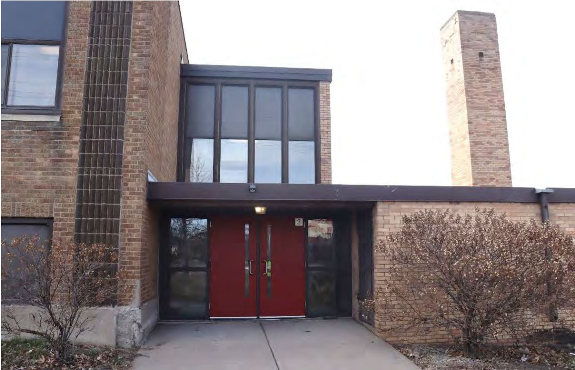
Figure 12. Facade of 1953 addition and entrance at north end of original 1935 school building, view facing west.
