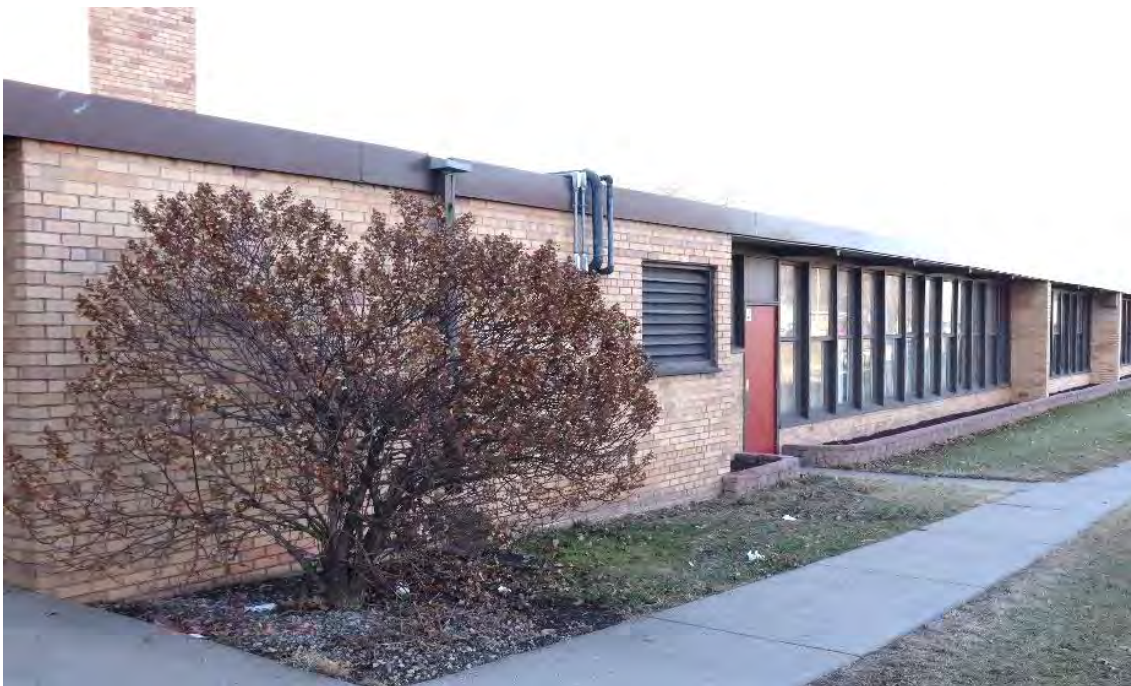
Figure 11. Facade of 1953 addition, view facing northwest.
