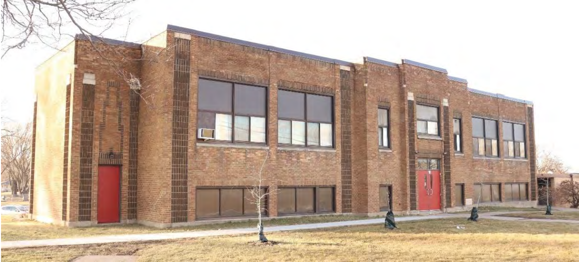
Figure 6. Front (east) facade of original 1935 North Heights School, view facing northwest.
