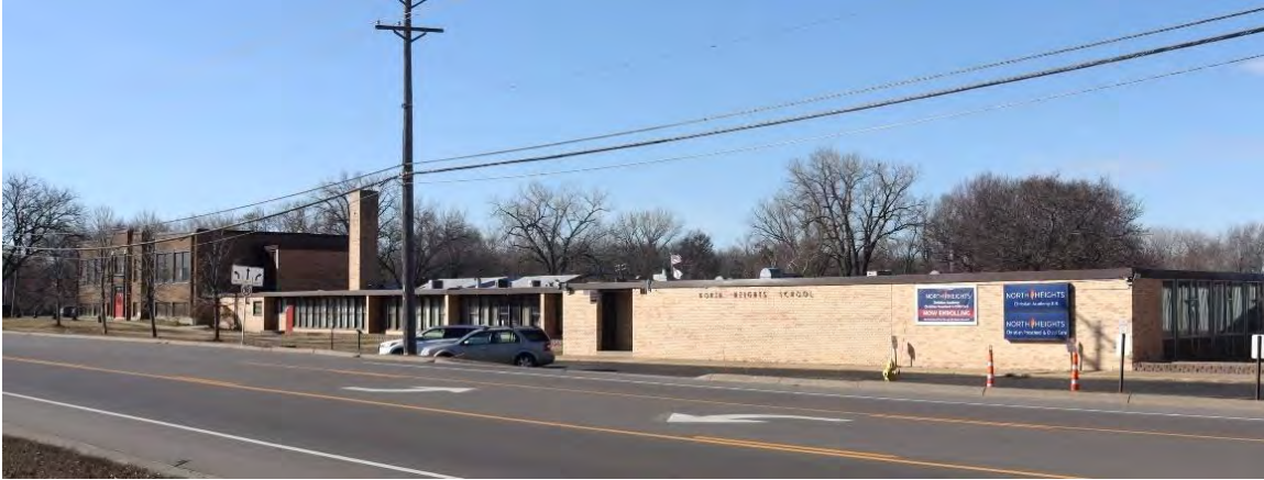
Figure 31. Original 1935 building (far left), 1953 addition (left), 1958 addition (center), and part of 1961 addition (right), view facing southwest.
