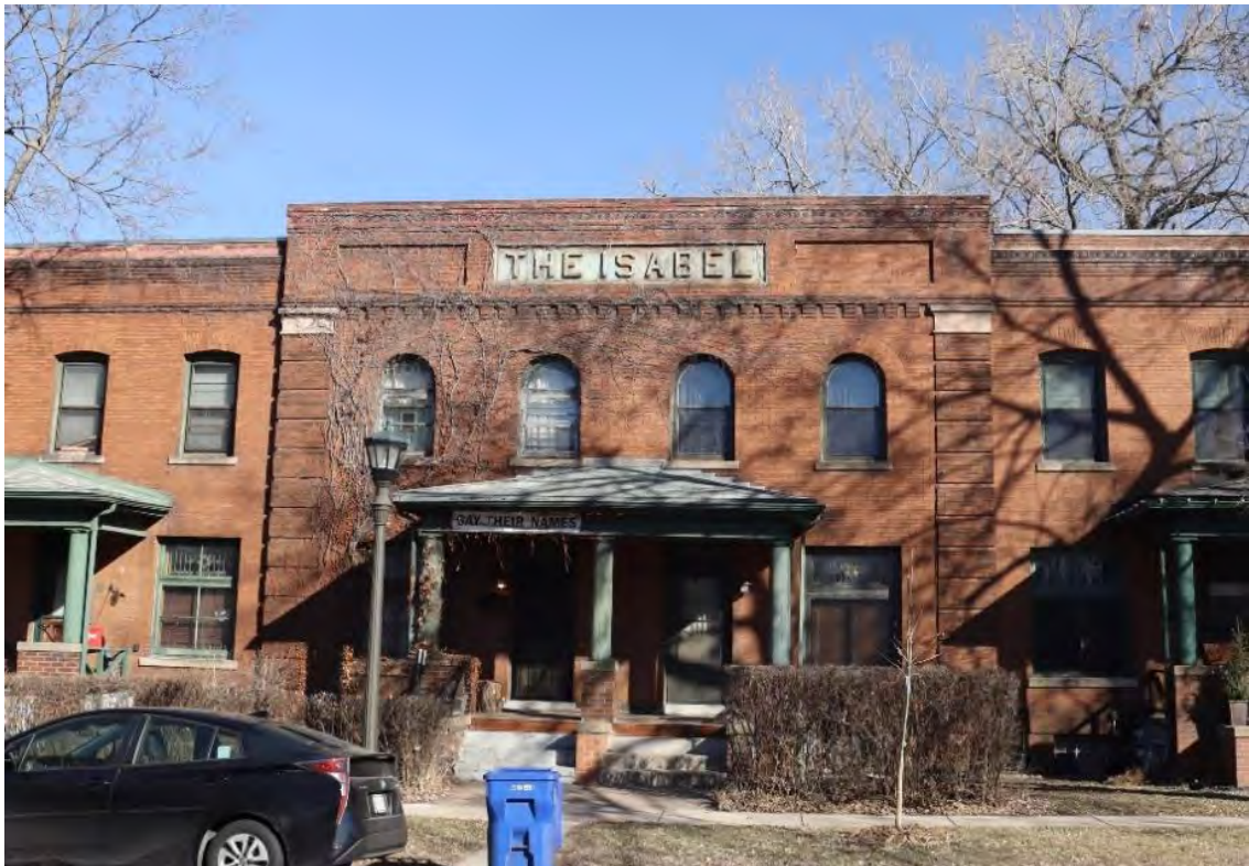
Figure 43. Front (south) facade, view toward north.
