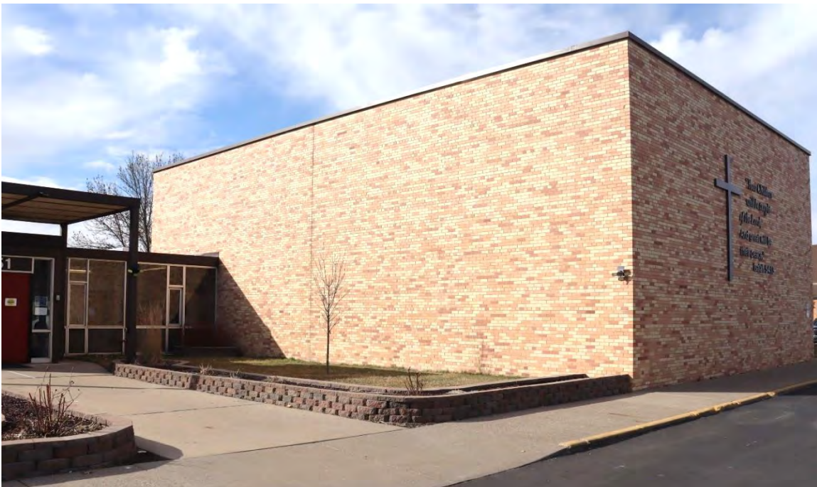
Figure 28. Side (south) elevation and front (east) facade of 1975 gymnasium addition, view facing northwest.
