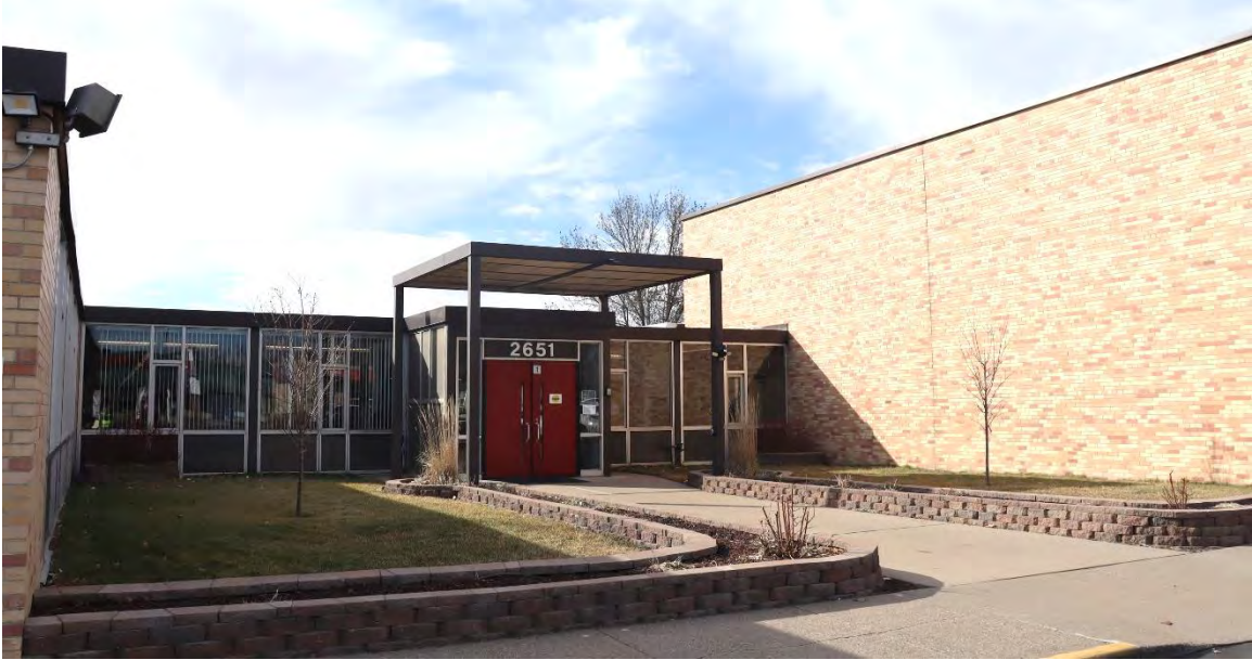
Figure 20. Facade of 1961 addition with new primary entrance, view facing west-northwest.
