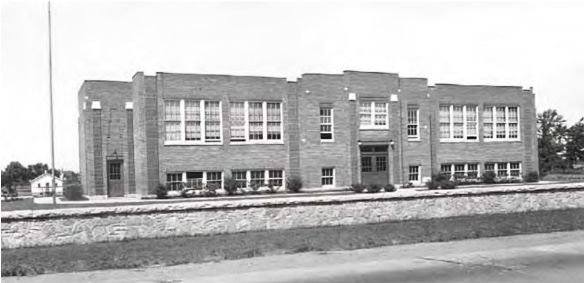
Figure 33. Undated photograph of the school shortly after completion in 1935. 59
