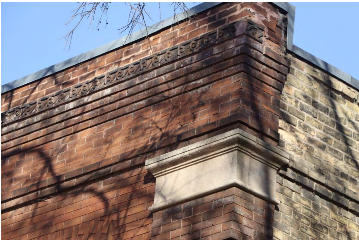
Figure 45. Detail view of molded band motif, stone capital, and brick work, view toward northwest.
