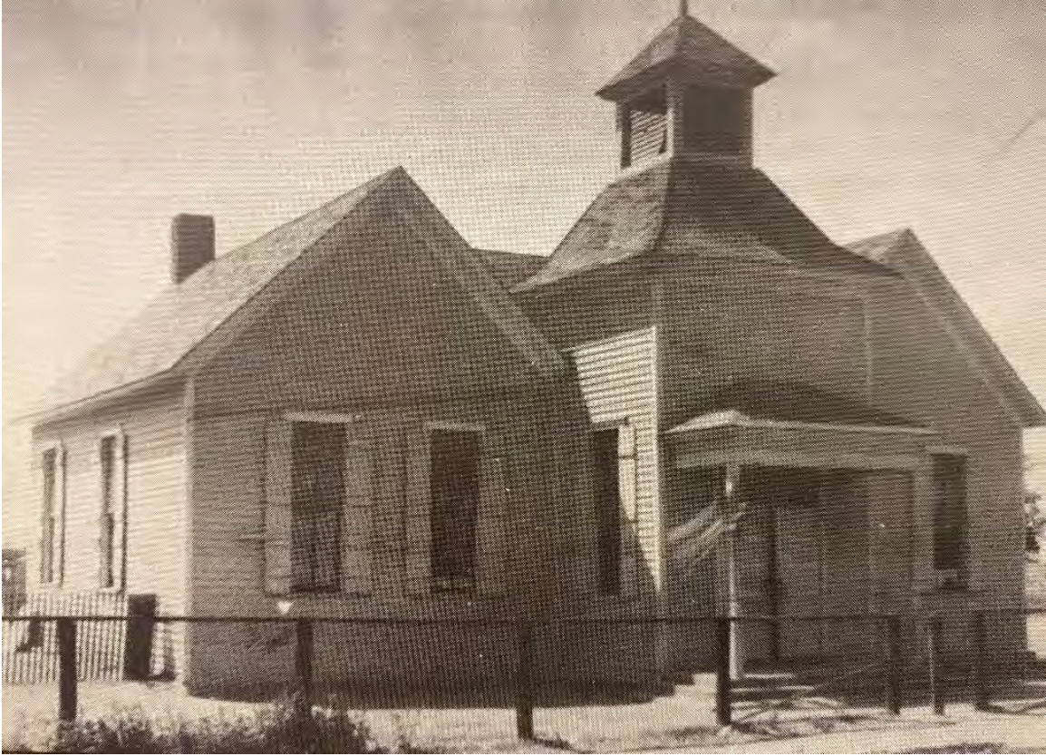
Figure 32. Undated photograph of original 1886 school (nonextant). 50
