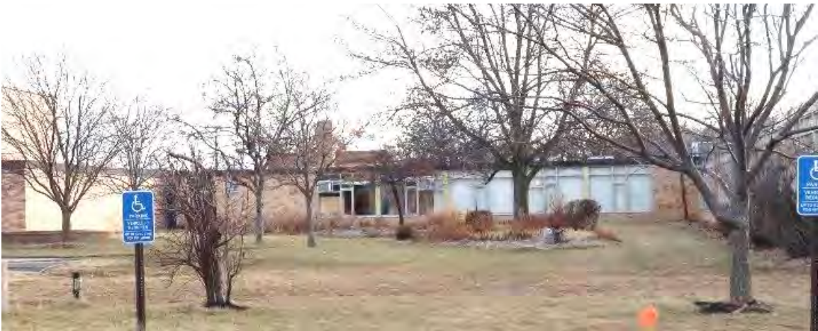
Figure 25. Side (north) elevation of 1961 library hyphen addition, view facing south.
