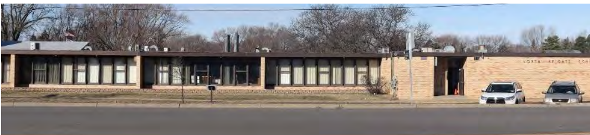
Figure 15. Facade of 1958 addition at north end of 1953 addition, view facing west.
