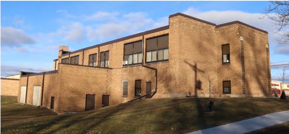
Figure 8. Rear (west) and side (south) elevations of original 1935 North Heights School, view facing northeast.
