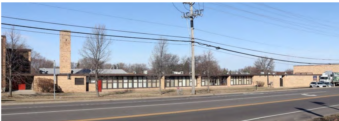
Figure 30. Facade of 1953 addition (left) and 1958 addition (right), view facing northwest.
