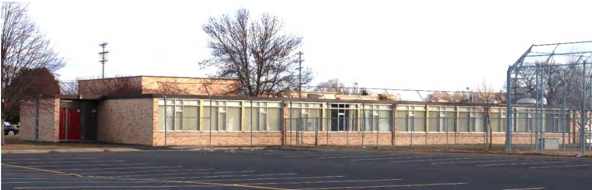
Figure 21. Side (north) and rear (west) elevations of 1961 linear classroom addition, view facing southeast.
