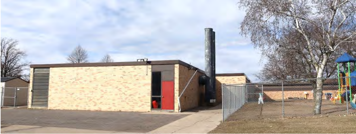
Figure 23. Side (south) elevations of 1961 linear classroom addition (left) and library hyphen addition (right), view facing north.
