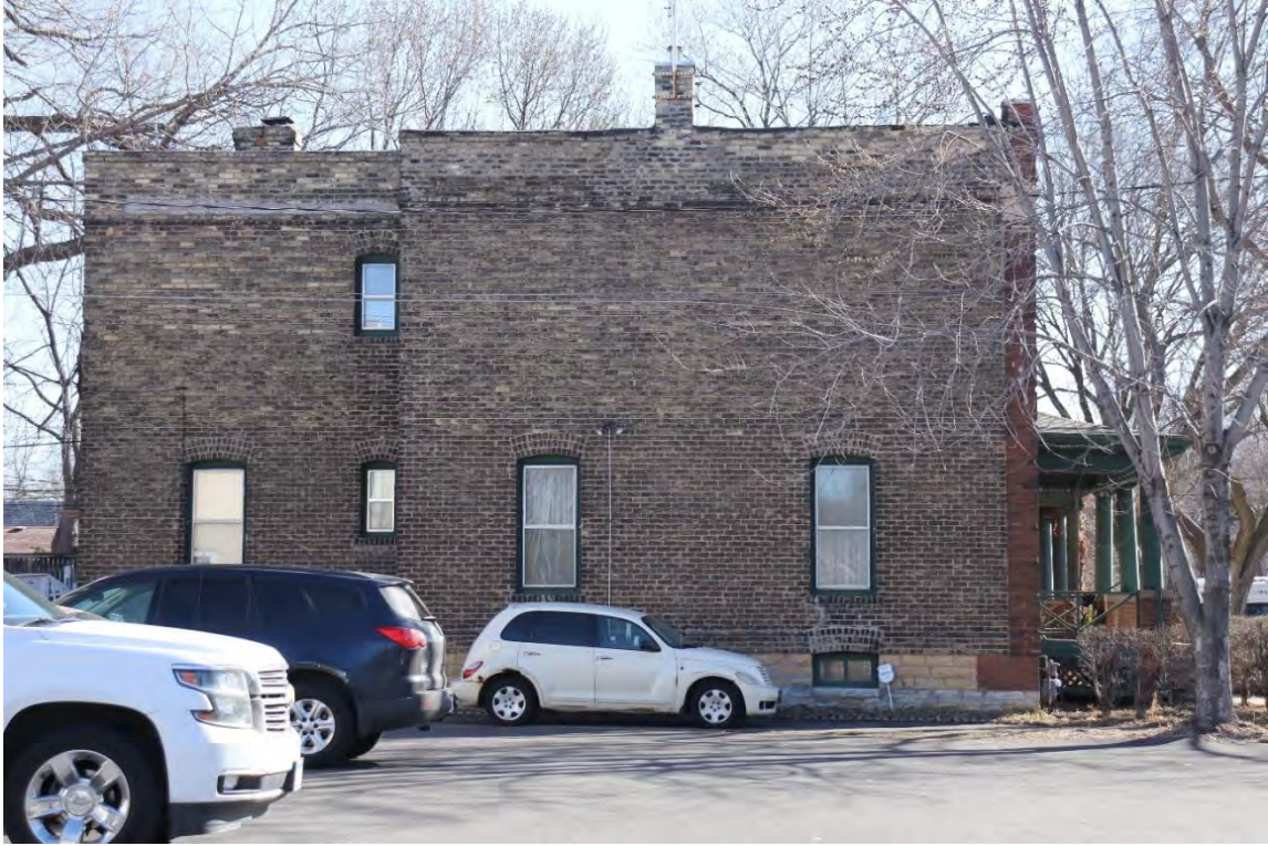
Figure 46. Side (west) elevation, view toward east.
