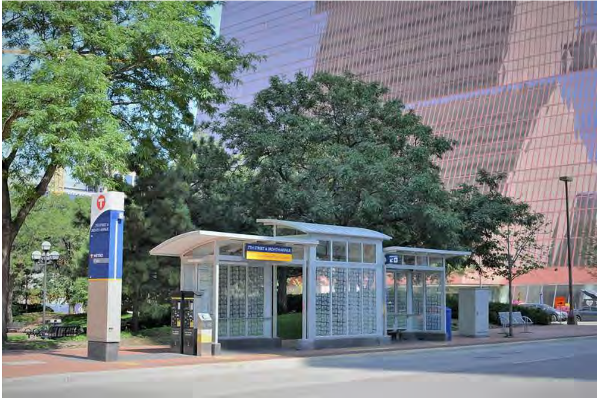
Typical BRT large shelter.
