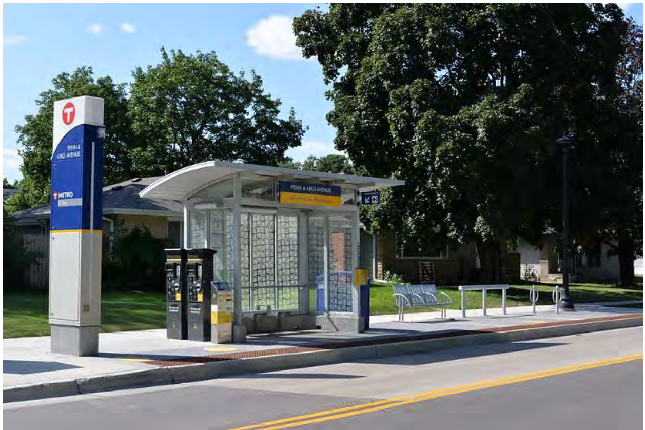
Typical BRT small shelter.
