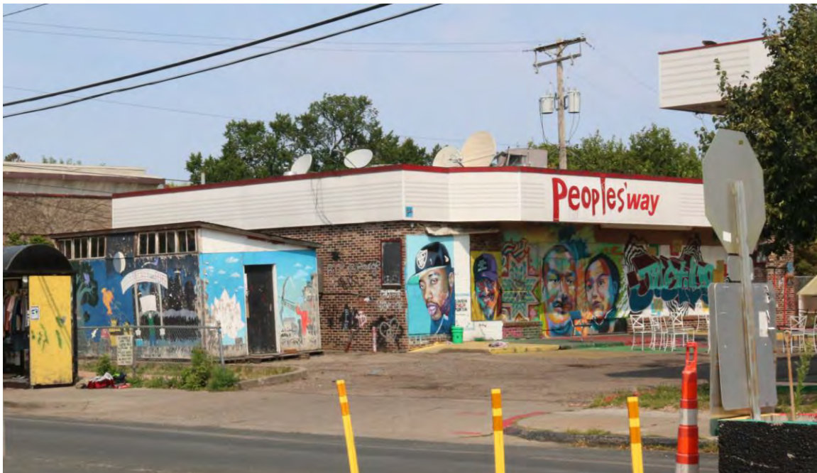
Figure 3. The People's Way, located at the northwest corner of Chicago Avenue and 38th Street, includes a now vacant former Speedway store and a plywood storage structure (at the far left), view facing northwest.
