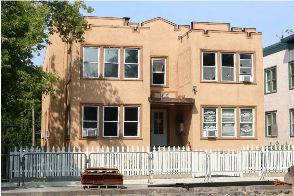
HE-MPC-22757, August 6, 2026, front (east) facade and side (south) elevation, view facing northwest.
