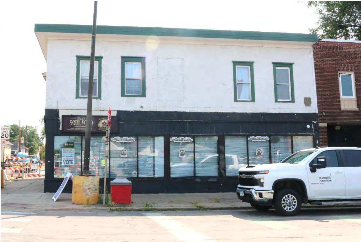
HE-MPC-18028, August 6, 2026, front (west) facade, view facing east.
