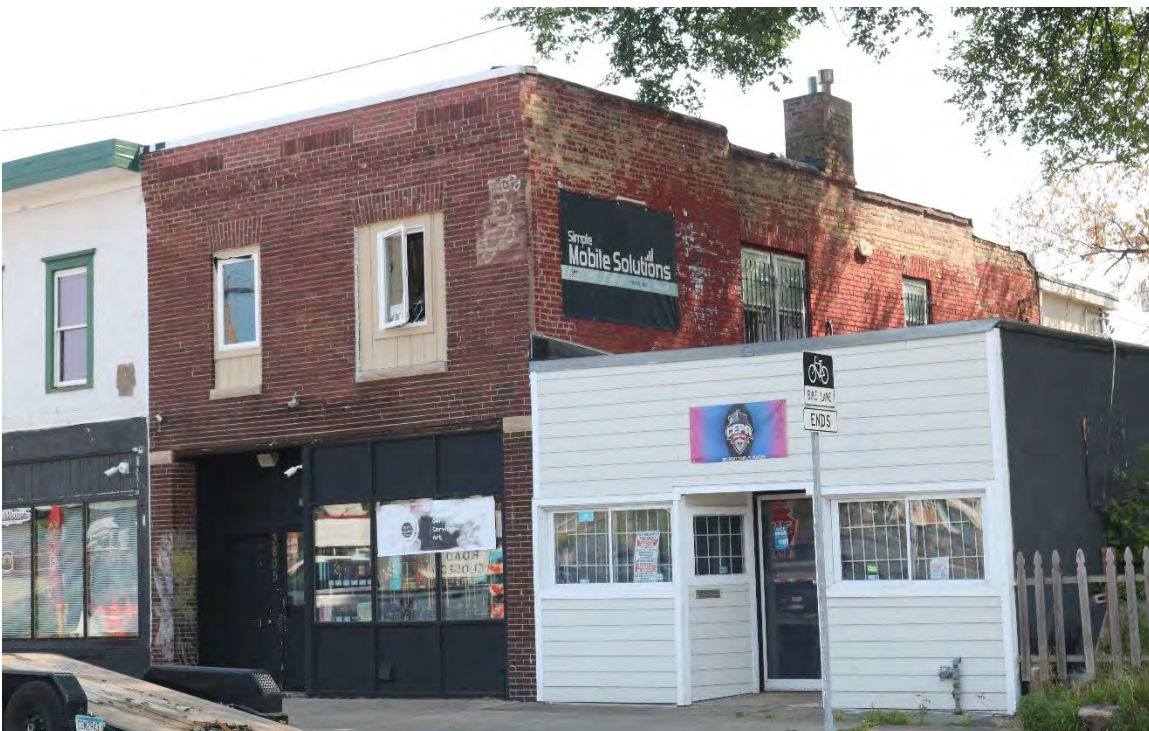
HE-MPC-18016, August 6, 2026, front (west) facade and side (south) elevation, view facing northeast. HE-MPC-18017 is visible in the foreground.
