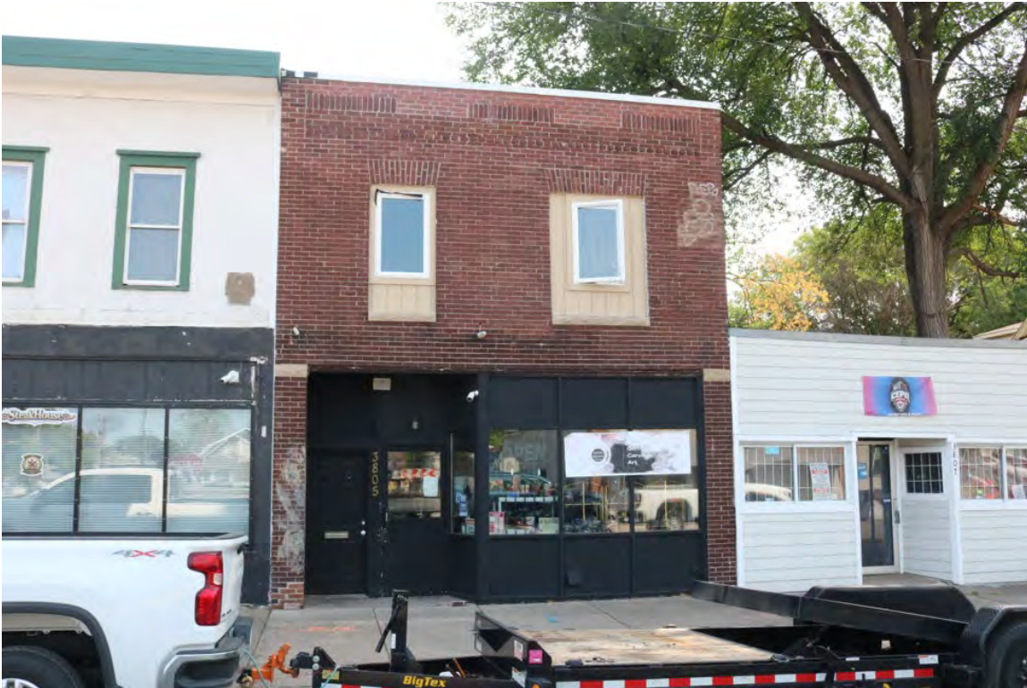
HE-MPC-18016, August 6, 2026, front (west) facade, view facing east.
