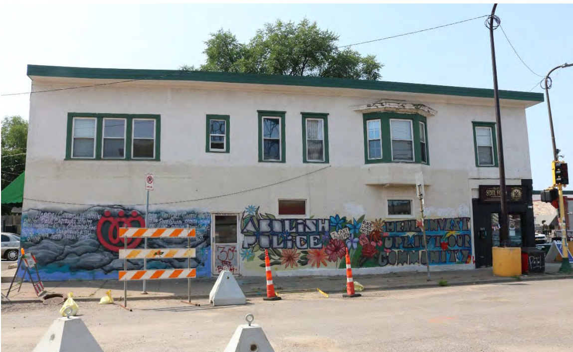
HE-MPC-18028, August 6, 2026, side (north) elevation, view facing south.
