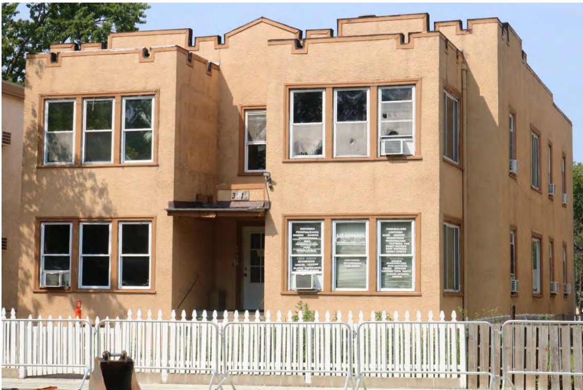
HE-MPC-22757, August 6, 2026, front (east) facade and side (north) elevation, view facing southwest.
