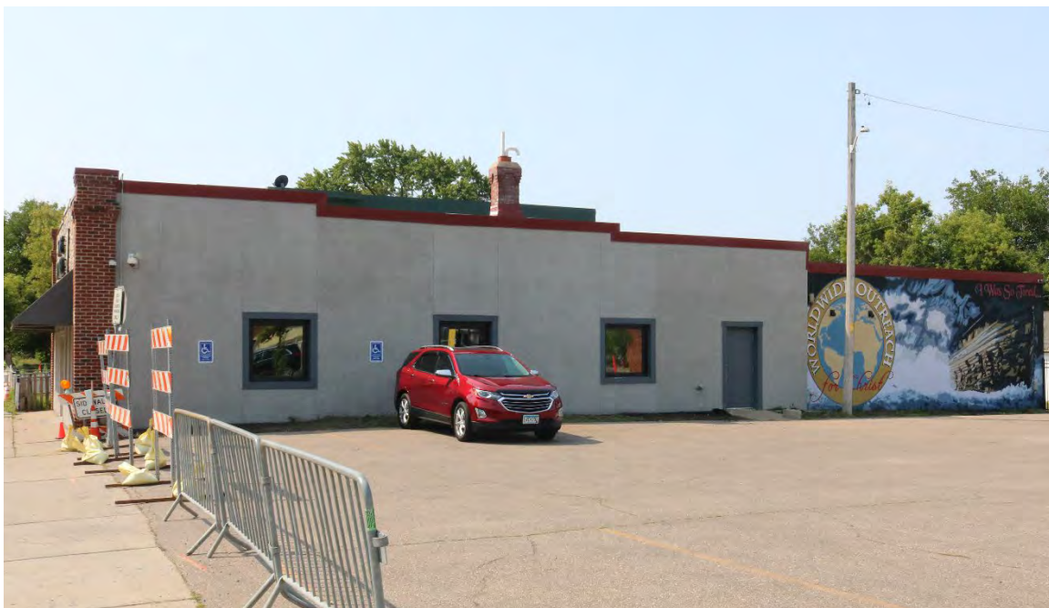
HE-MPC-19254, August 6, 2026, side (north) elevation, view facing south.
