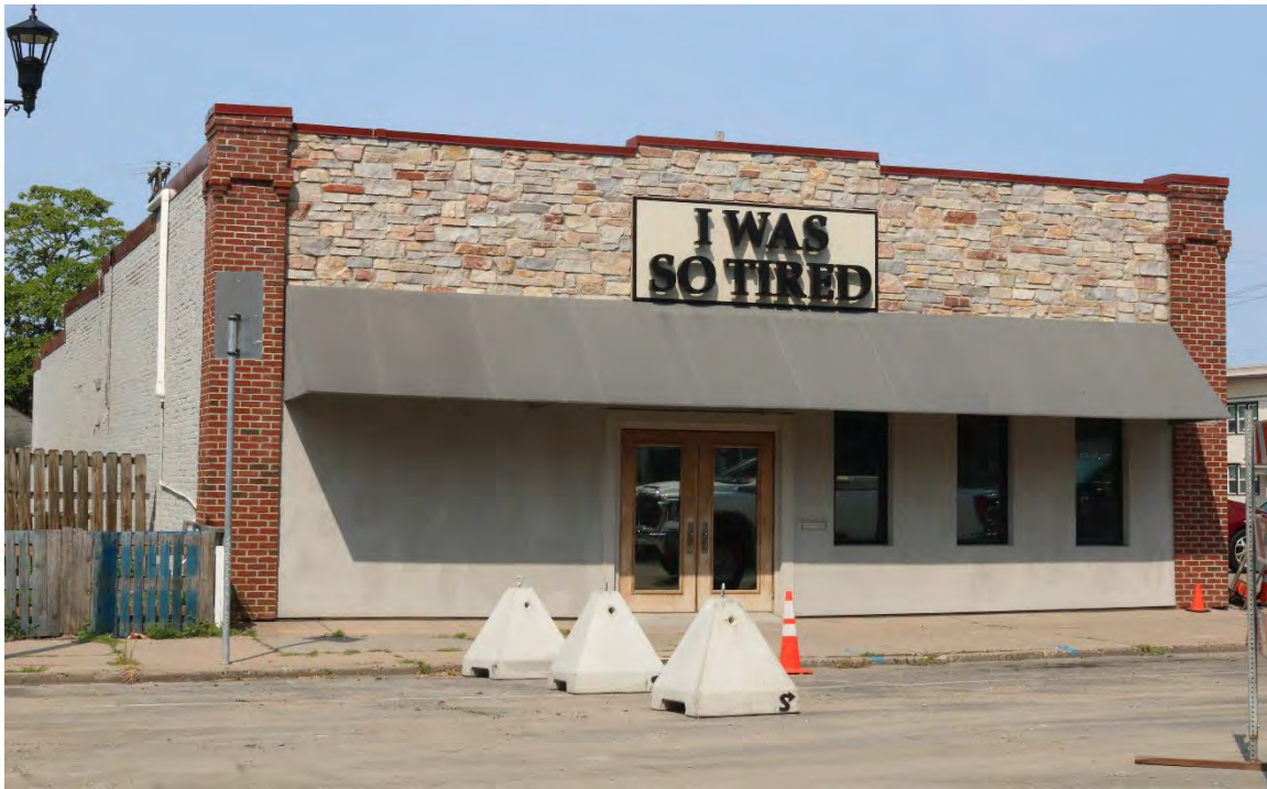
HE-MPC-19254, August 6, 2026, front (east) facade and side (south) elevation, view facing northwest.
