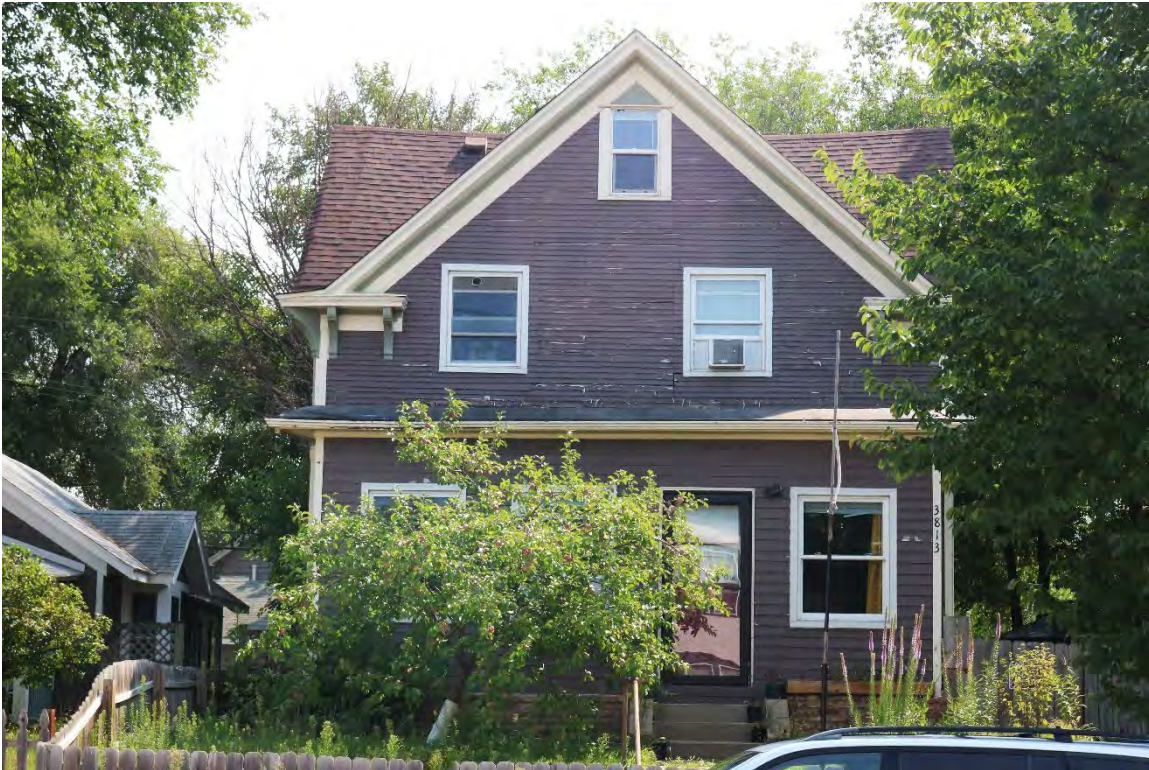
HE-MPC-19256, August 6, 2026, front (west) facade, view facing east.
