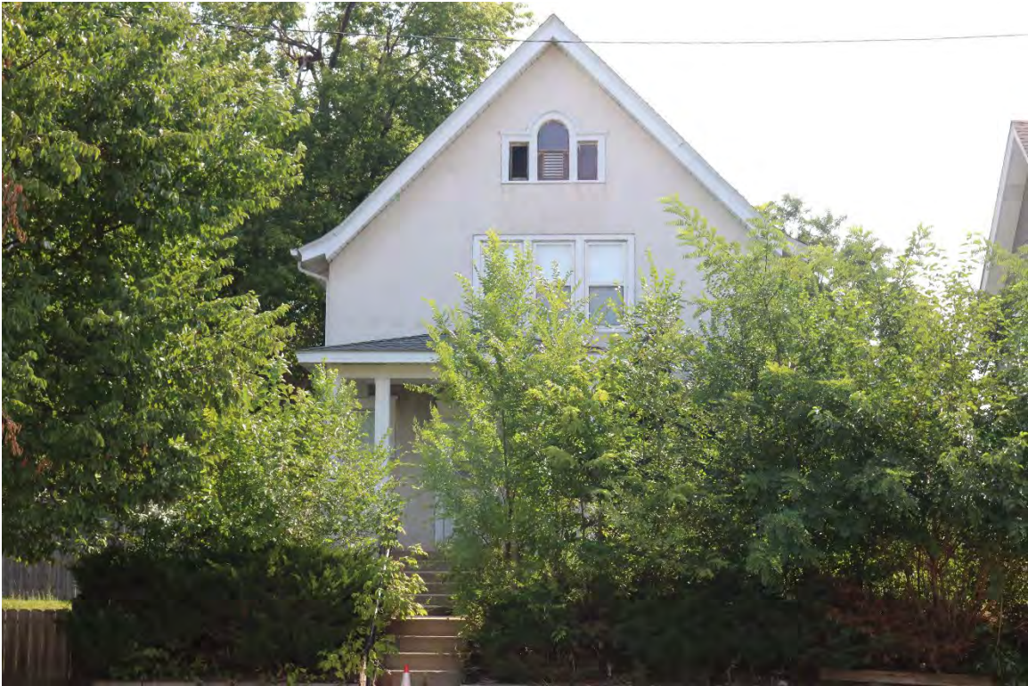
HE-MPC-22758, August 6, 2026, front (west) facade, view facing east.
