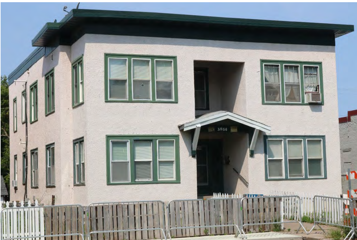
HE-MPC-19257, August 6, 2026, front (east) facade and side (south) elevation, view facing northwest.
