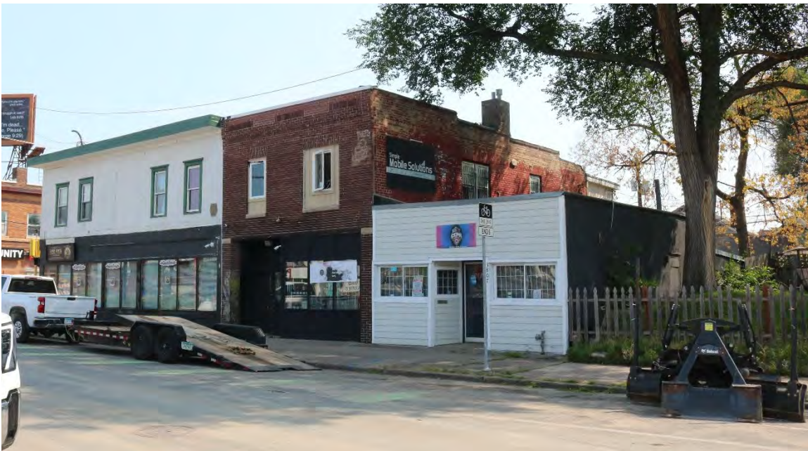
HE-MPC-18017, August 6, 2026, front (west) facade and side (south) elevation, and adjacent commercial properties, view facing northeast.
