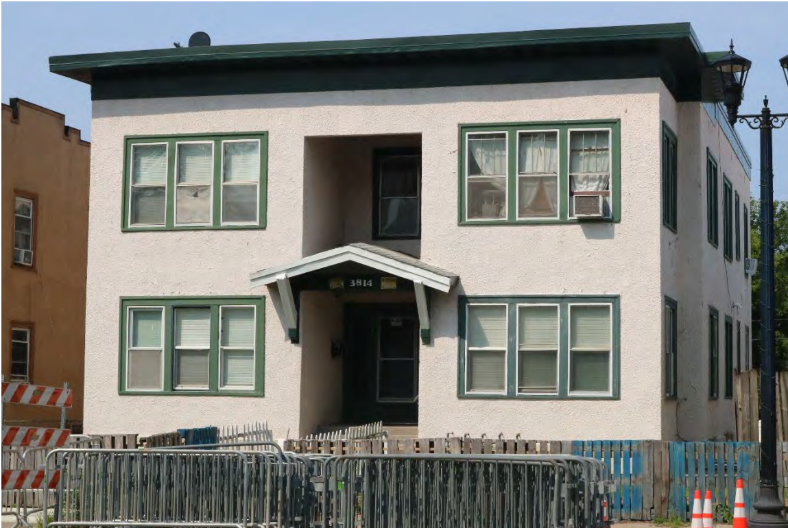
HE-MPC-19257, August 6, 2026, front (east) facade and side (north) elevation, view facing southwest.
