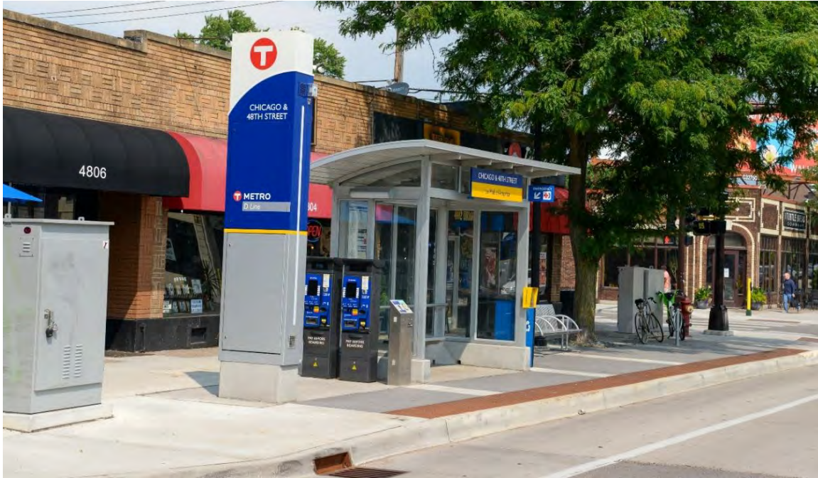
Figure 4. Existing D Line platform at Chicago Avenue and 48th Street. The proposed platforms at Chicago Avenue and 38th Street will be the same with the exception of the trash can placement, which will be adjacent to the bench rather than along the shelter.
