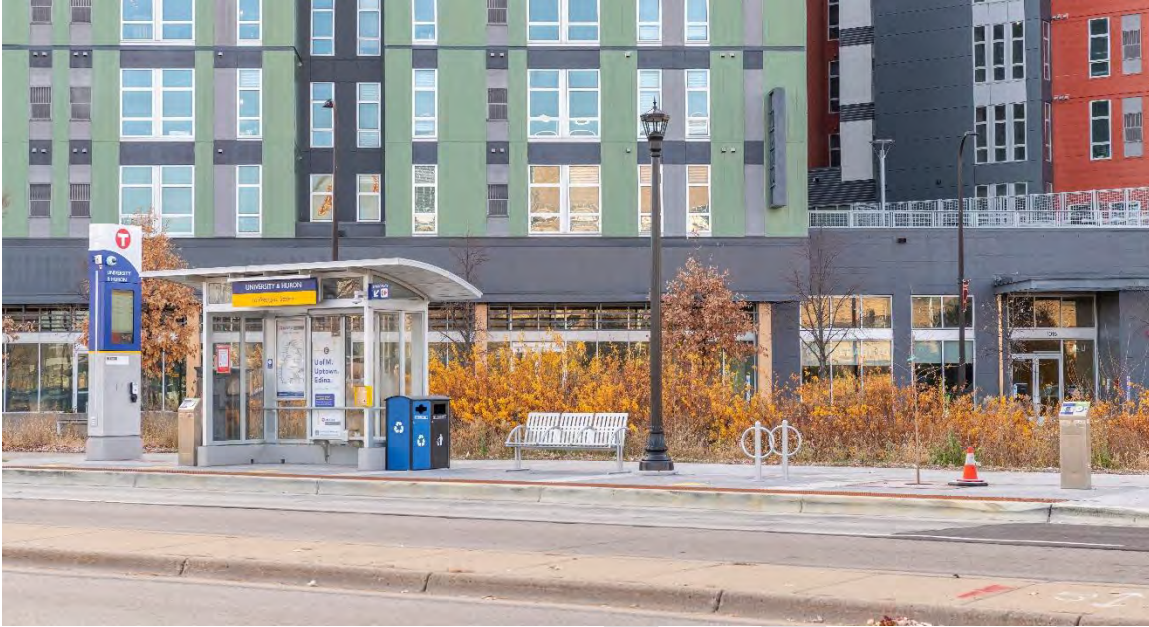
Figure 1. The E Line BRT platform at University Avenue and Huron includes the standard features implemented at platforms throughout the metro area (from left to right): the free-standing pylon with the station information, fare machines, metal-frame shelter with clear glass panels, trash can, bench, and bike rack.
