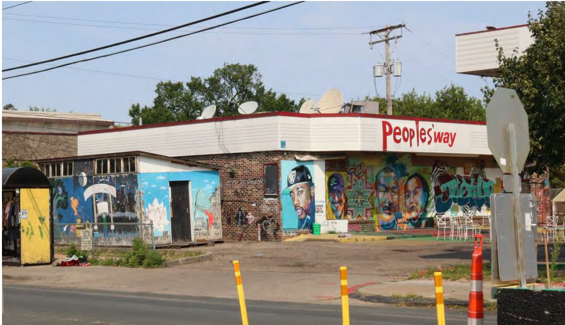
Figure 4. The People's Way, located at the northwest corner of Chicago Avenue and 38th Street, includes a now vacant former Speedway store and a plywood storage structure (at the far left), view facing northwest.
