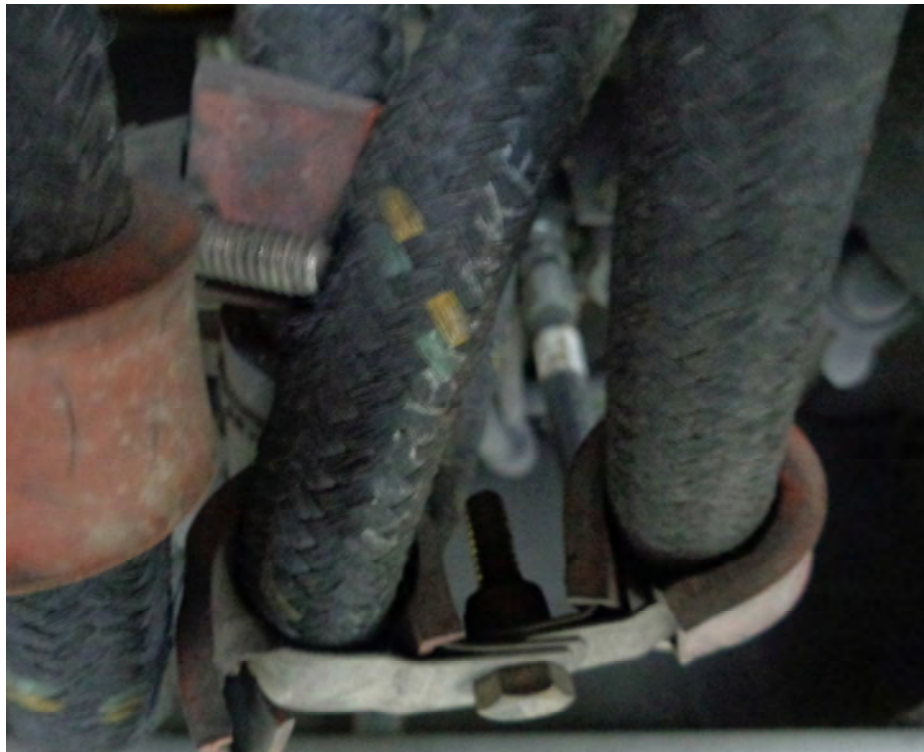
Bus 1205: Bolt Rubbing Hole in Brake Hose
