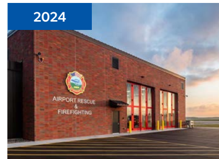
2024 Aircraft Rescue and Fire Fighting (ARFF) Facility and Snow Removal Equipment (SRE) Facility Project Minnesota/North Dakota Associated Builders and Contractors Excellence in Construction Award
