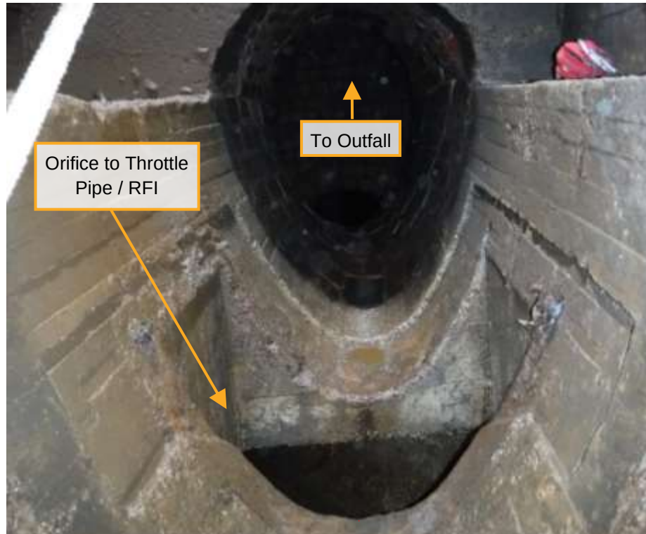
Figure 8 | Sanger – Washington East Regulator, Facing Downstream Toward Outfall
