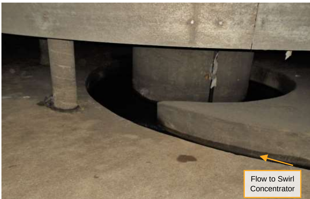
Figure 33 | Fayette Swirl Concentrator Dry Weather Flow Channel
