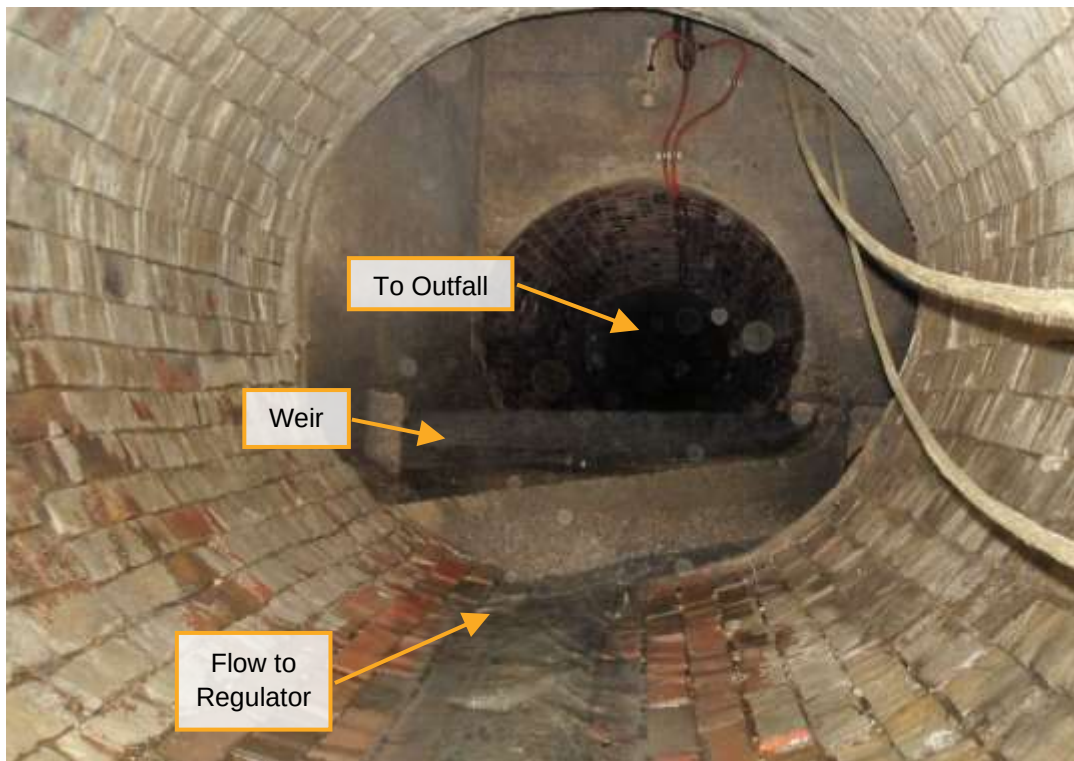
Figure 12 | South Regulator, Facing Downstream Toward Outfall
