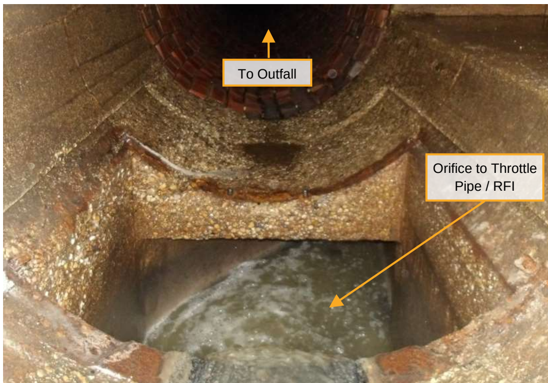
Figure 5 | Sanger North Regulator, Facing Downstream Toward Outfall
