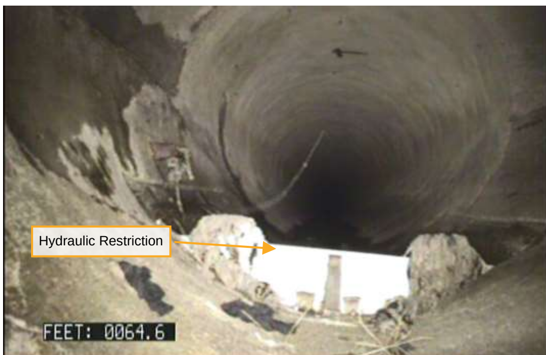
Figure 14 | Cedar Hydraulic Restriction from Outfall Pipe, Facing Upstream Toward Regulator
