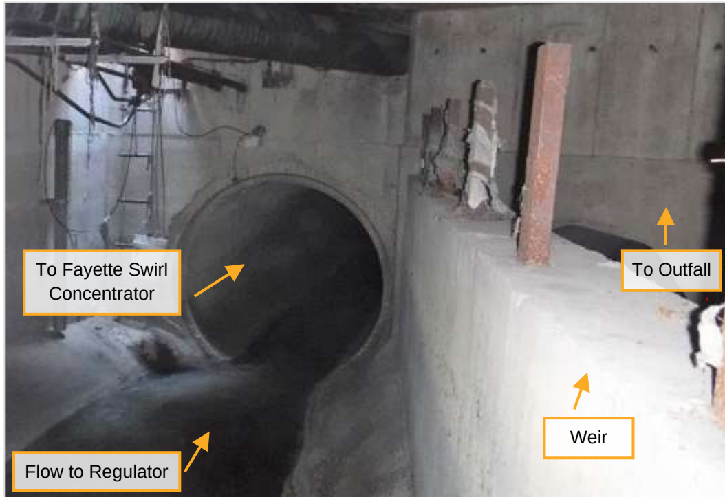
Figure 30 | Fayette Regulator, from Upstream Facing Downstream
