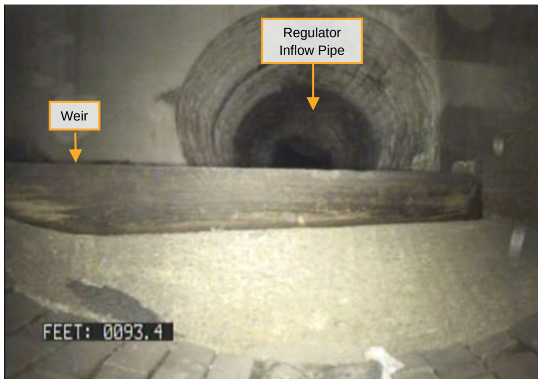
Figure 11 | South Weir from Outfall Pipe, Facing Upstream Toward Regulator
