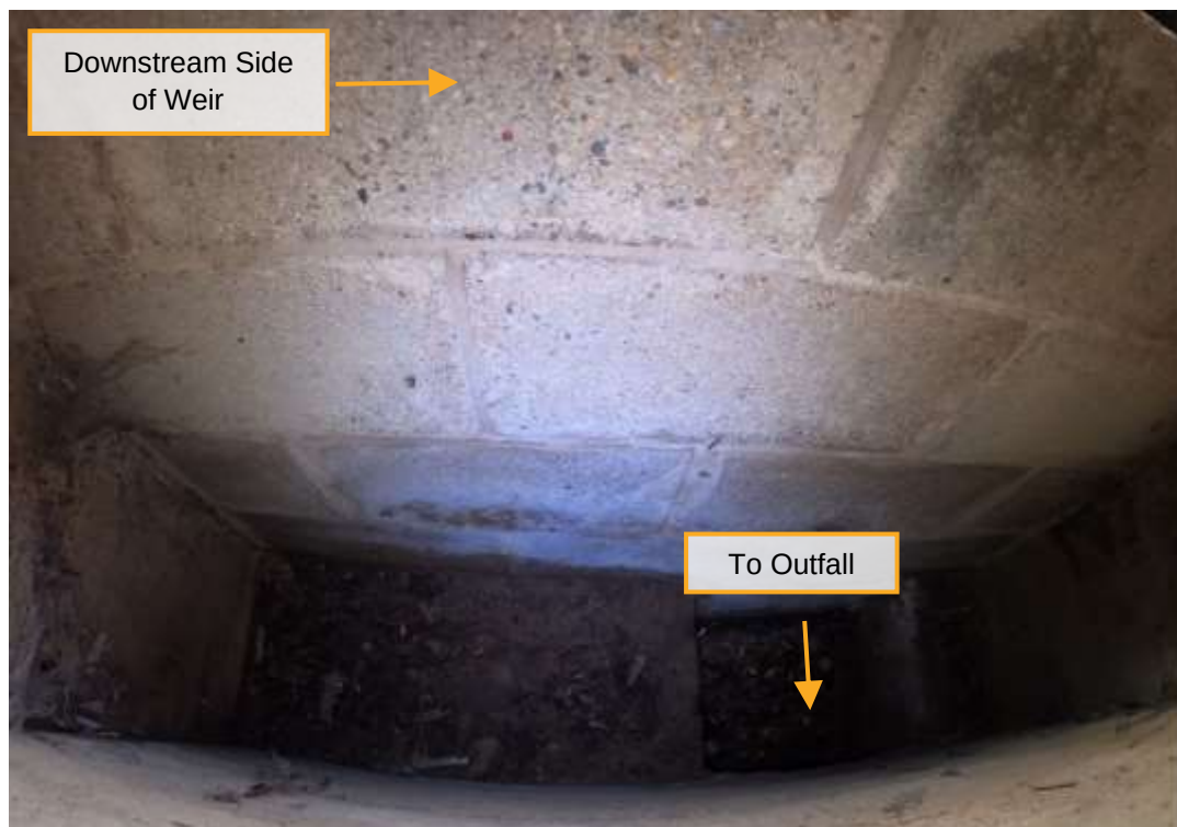
Figure 21 | Harrison Regulator, from Overflow Side of Weir
