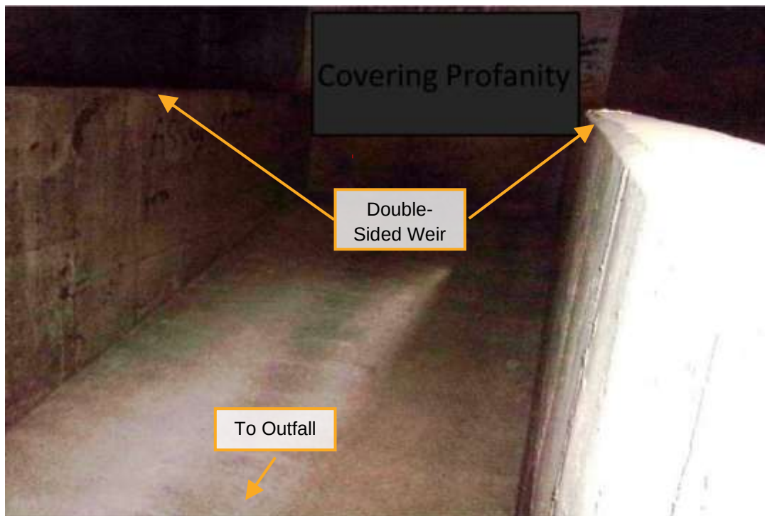
Figure 44 | Spring Regulator, from Overflow Side of Weir
