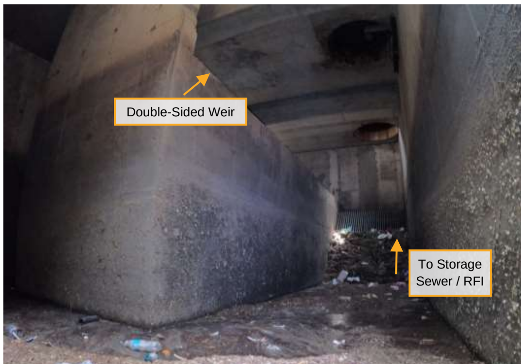
Figure 43 | Spring Regulator, Effluent Side of Structure
