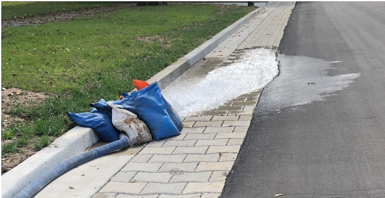
Figure 3 | Hydrant Testing to evaluate the Subsurface Native Soil Infiltration Rate below Permeable Pavers in Peoria
