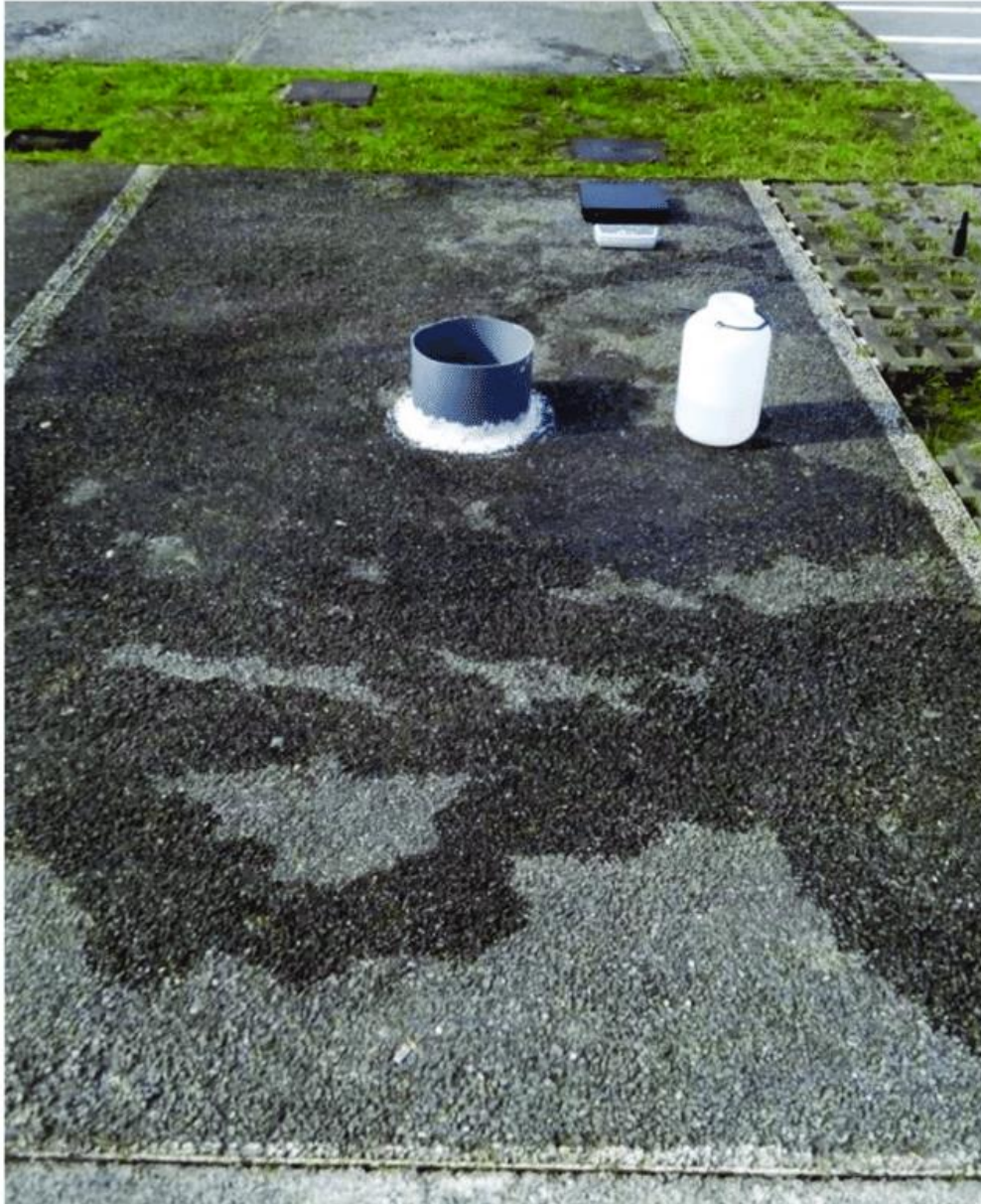
Figure 5 | Test Set Up Using ASTM C1701 for Porous Pavements
