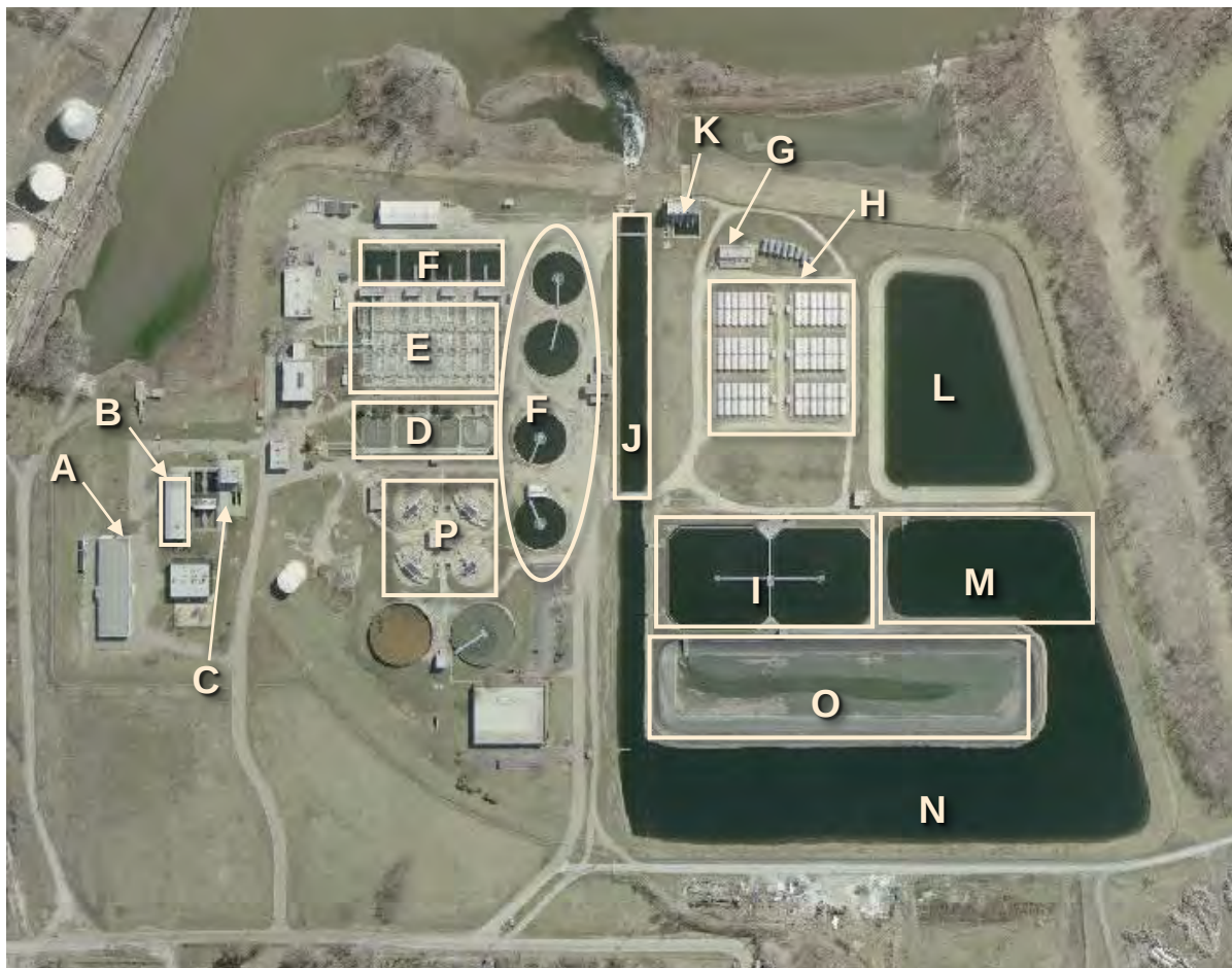
Figure 1 | Greater Peoria Sanitary District Wastewater Treatment Plant & Treatment Processes
