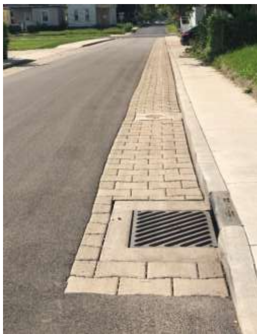
Figure 3 | Representative Photo of Permeable Pavers in Year 2 Project Area. Photo taken August 23, 2024.
