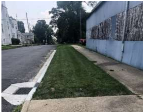
Figure 5 | Representative Photo of Stormwater Bump-Ins in Year 2 Project Area. Photo taken August 20, 2024.
