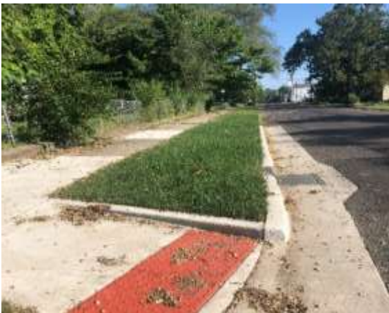
Figure 4 | Representative Photo of Stormwater Bump-Ins in Year 2 Project Area. Photo taken August 27, 2024.
