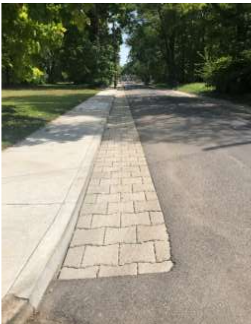
Figure 2 | Representative Photo of Permeable Pavers in Year 2 Project Area. Photo taken August 23, 2024.
