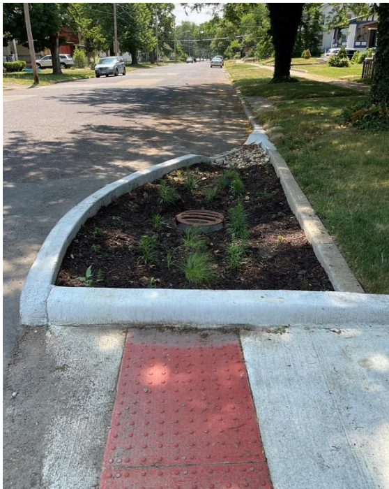
Figure 4 | Representative Photos for Bump Outs in Year 1 Project Area. Photos taken August 21, 2023.
