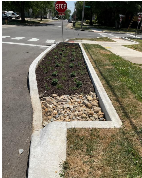
Figure 5 | Representative Photos for Bump Outs in Year 1 Project Area. Photos taken August 21, 2023.
