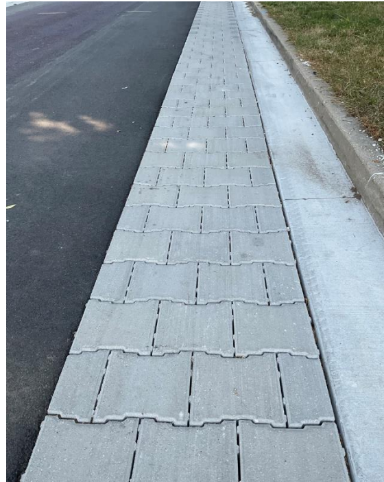
Figure 3 | Representative Photos for Permeable Pavers in Year 1 Project Area. Photo taken July 30, 2023.
