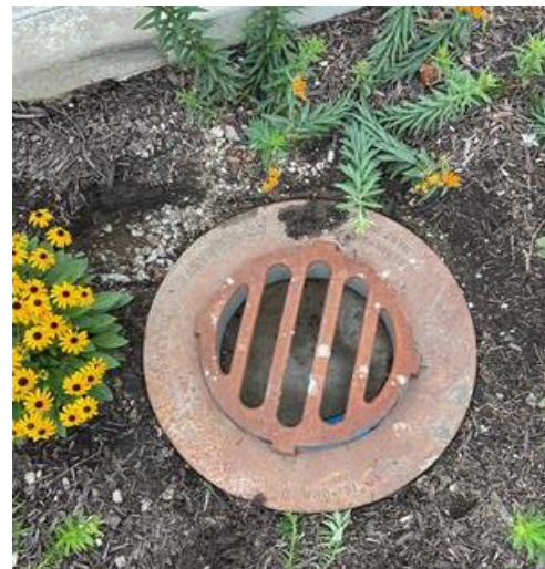
Figure 7 | Showing Inlets in Bump-Outs in Year 1 Project Area. Photos taken August 29, 2023.
