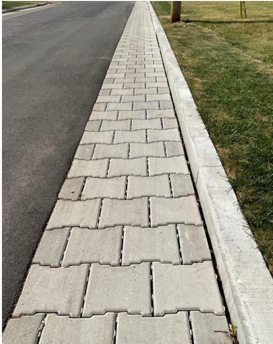
Figure 2 | Representative Photos for Permeable Pavers in Year 1 Project Area. Photo taken July 30, 2023.
