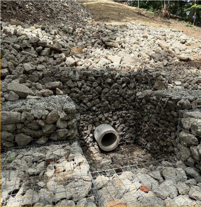
Golden Acres Subdivision Drainage Improvements, 2025
