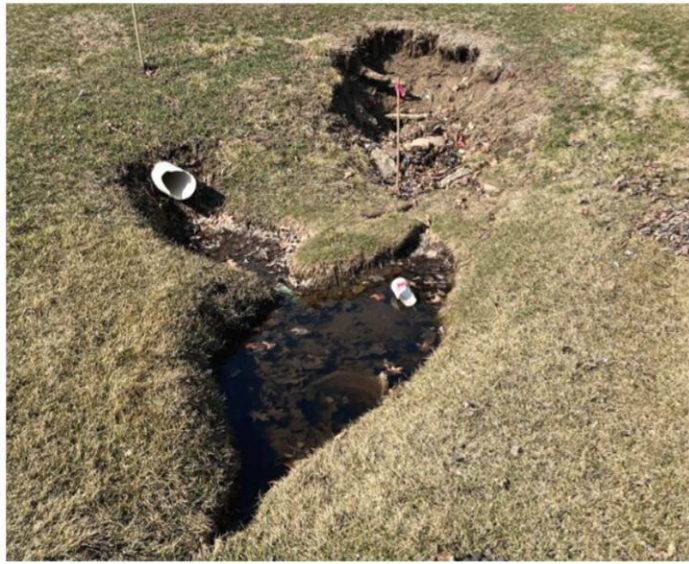
North Sheridan Reconstruction and Storm Sewer Improvement 2027
