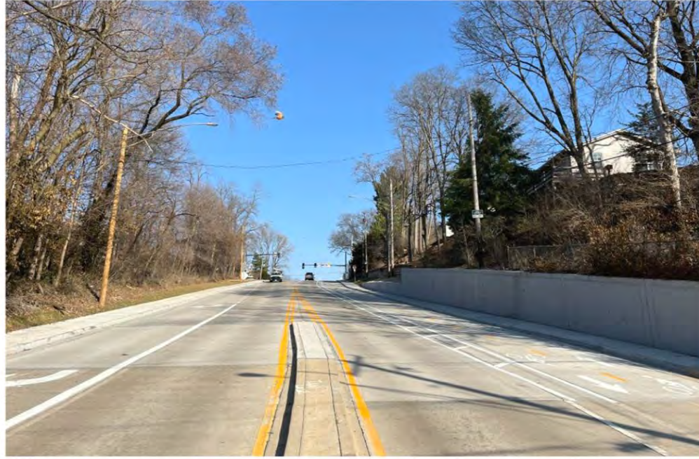
MacArthur Moss to Bridge - Roadway and Drainage Improvement
