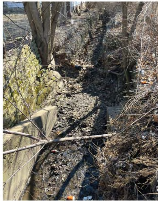
Tributary A Culvert Improvements - Gift to MacQueen
