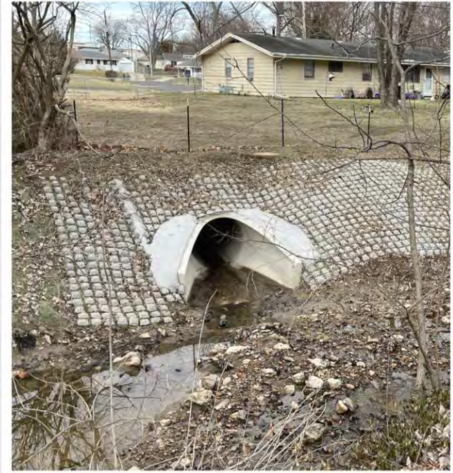
Ronald Road Storm Sewer Improvement
