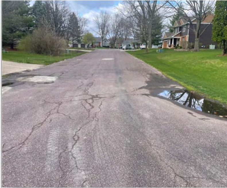
Deerbrook Drive Reconstruction & Drainage Improvements
