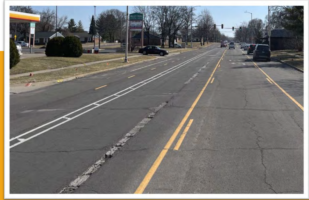
MacArthur Ave – Roadway and Drainage Improvements
