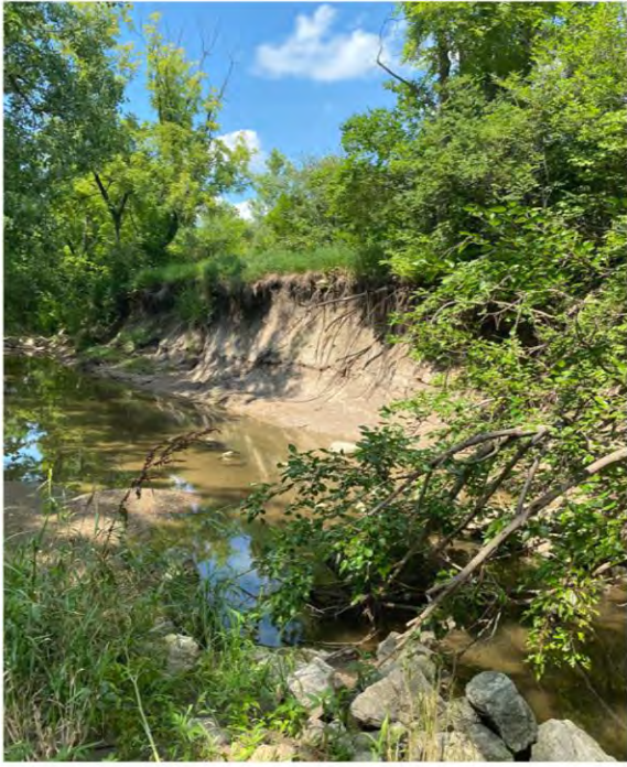
Stone Creek Stabilization at Wilhem Bridge
