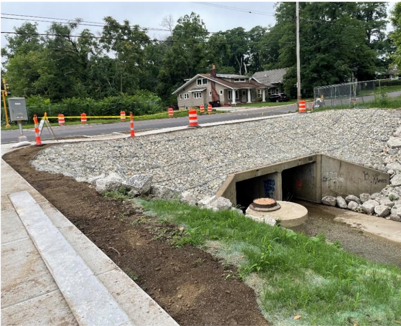
Erosion Control Improvements – East Branch Dry Run Creek at McClure
