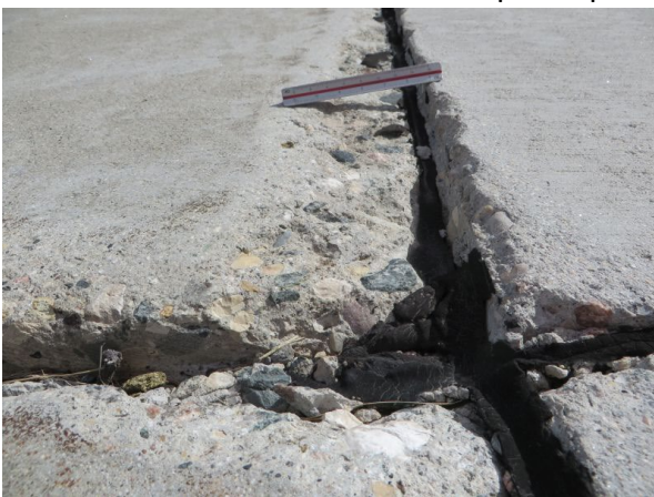
Figure 1-4: Faulting on Taxiway Connector
