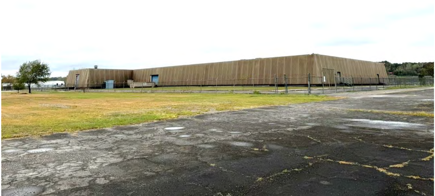
Photo 2. Building #201, oblique of rear (south) and side (east) elevations, view facing northwest.
