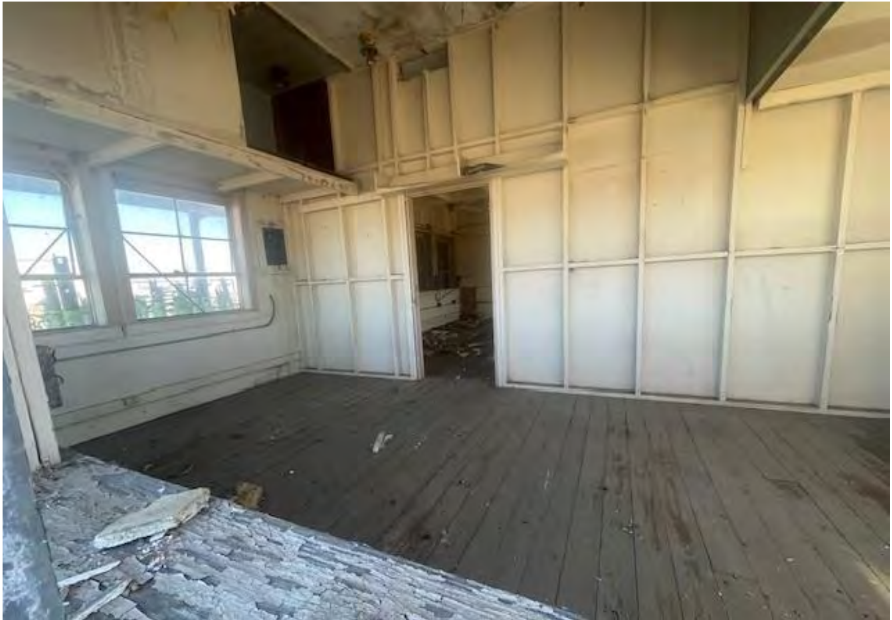
Photo 7. Storage shed, interior.
