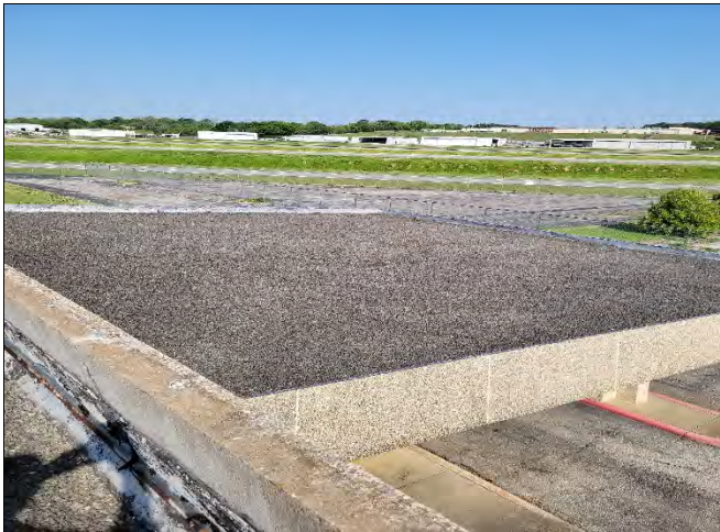
Roof View, North
