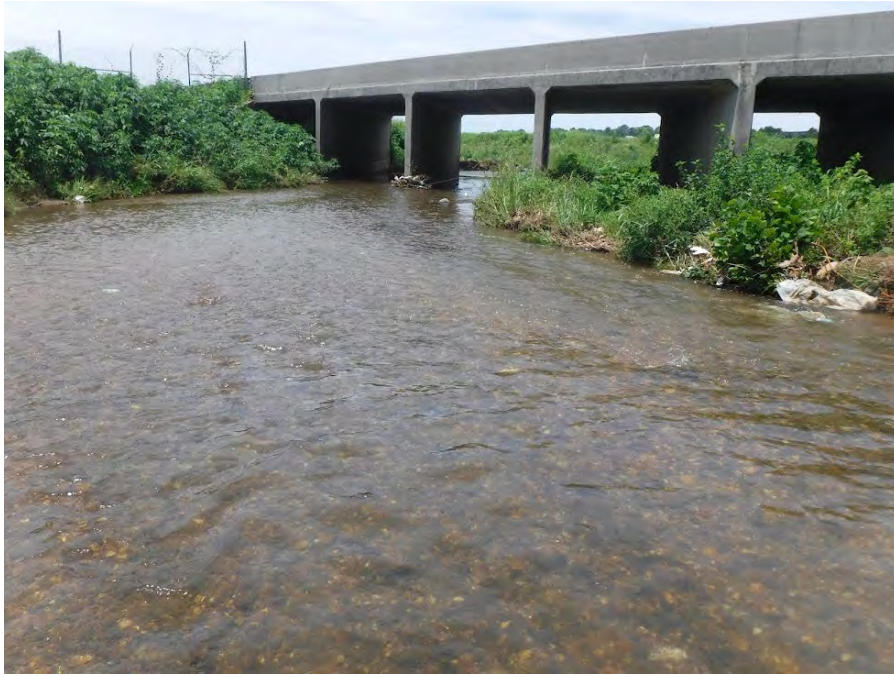
Village Creek facing west / downstream from a location near the upstream project limits. Taken by Mike McConnell, 6-26-2025.
