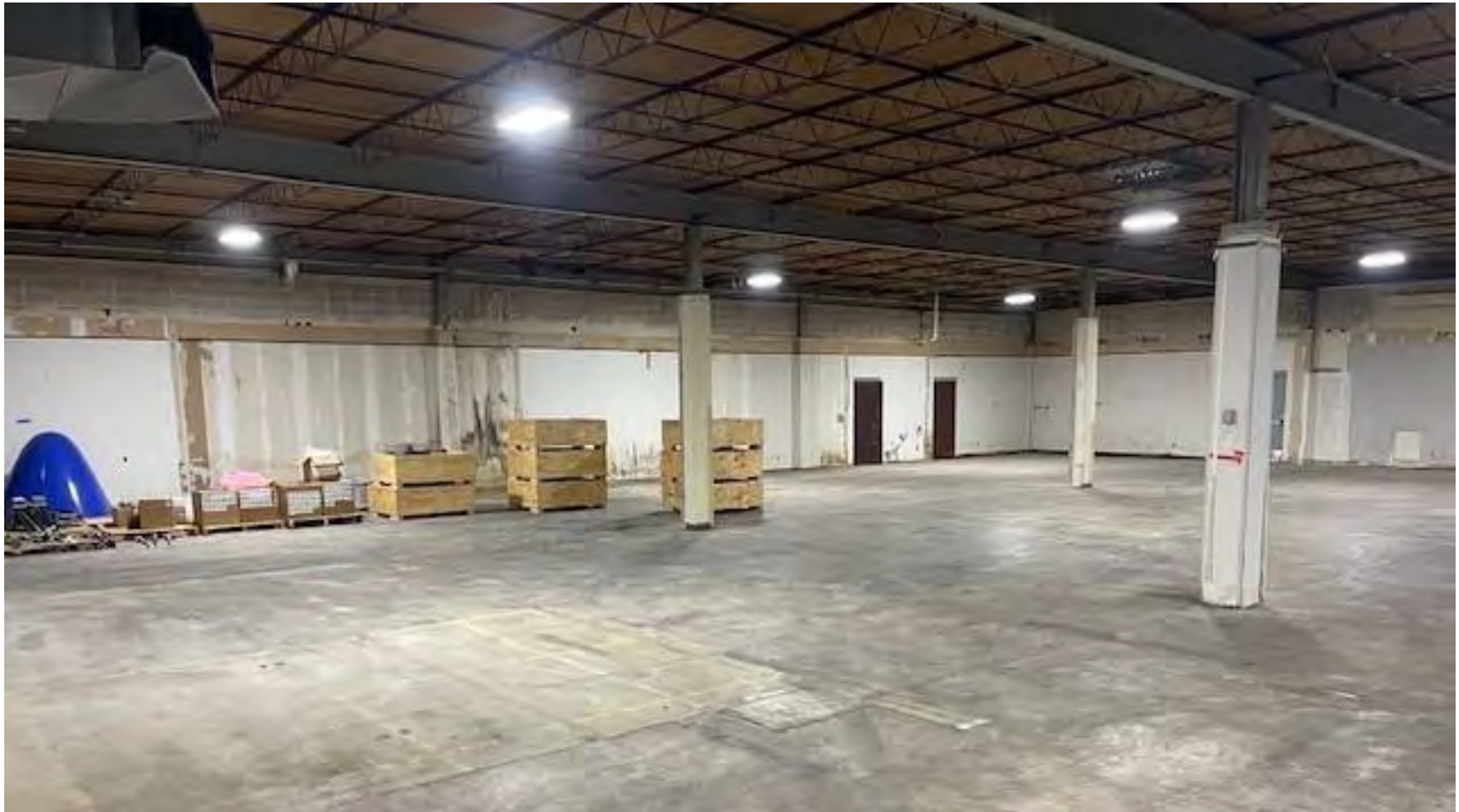
Photo 4. Building #201, interior research area.
