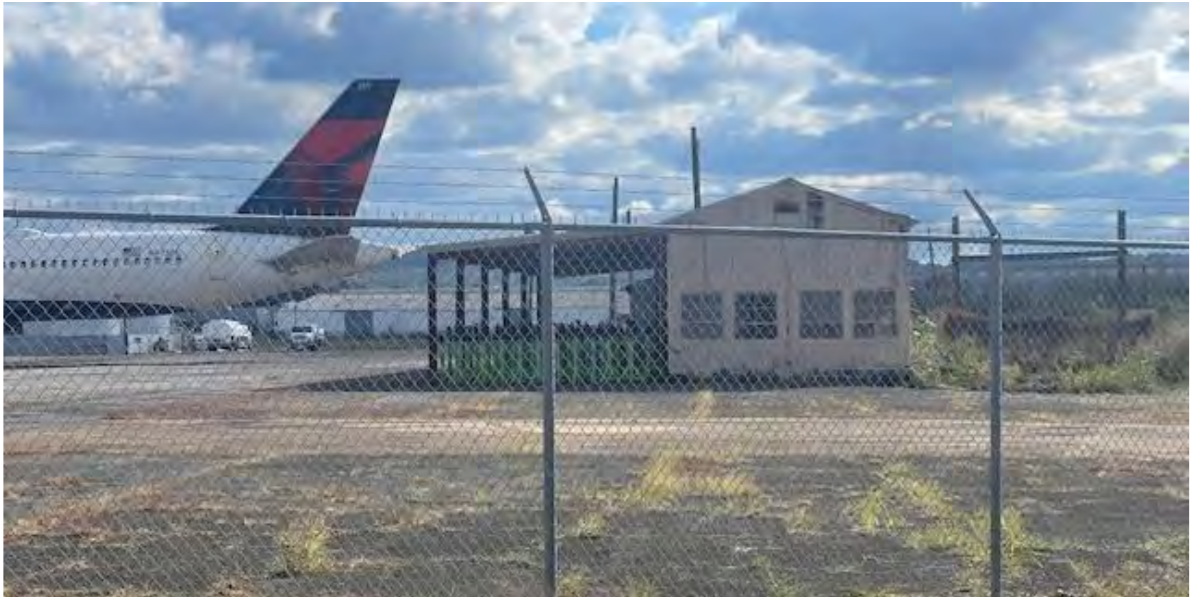
Photo 6. Storage shed, north elevation, view facing south.
