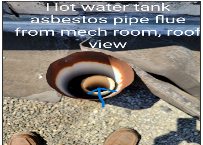
Asbestos Cementitious Hot Water Flue Pipe, Mech Room to Roof
