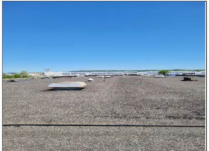
Roof View, East
