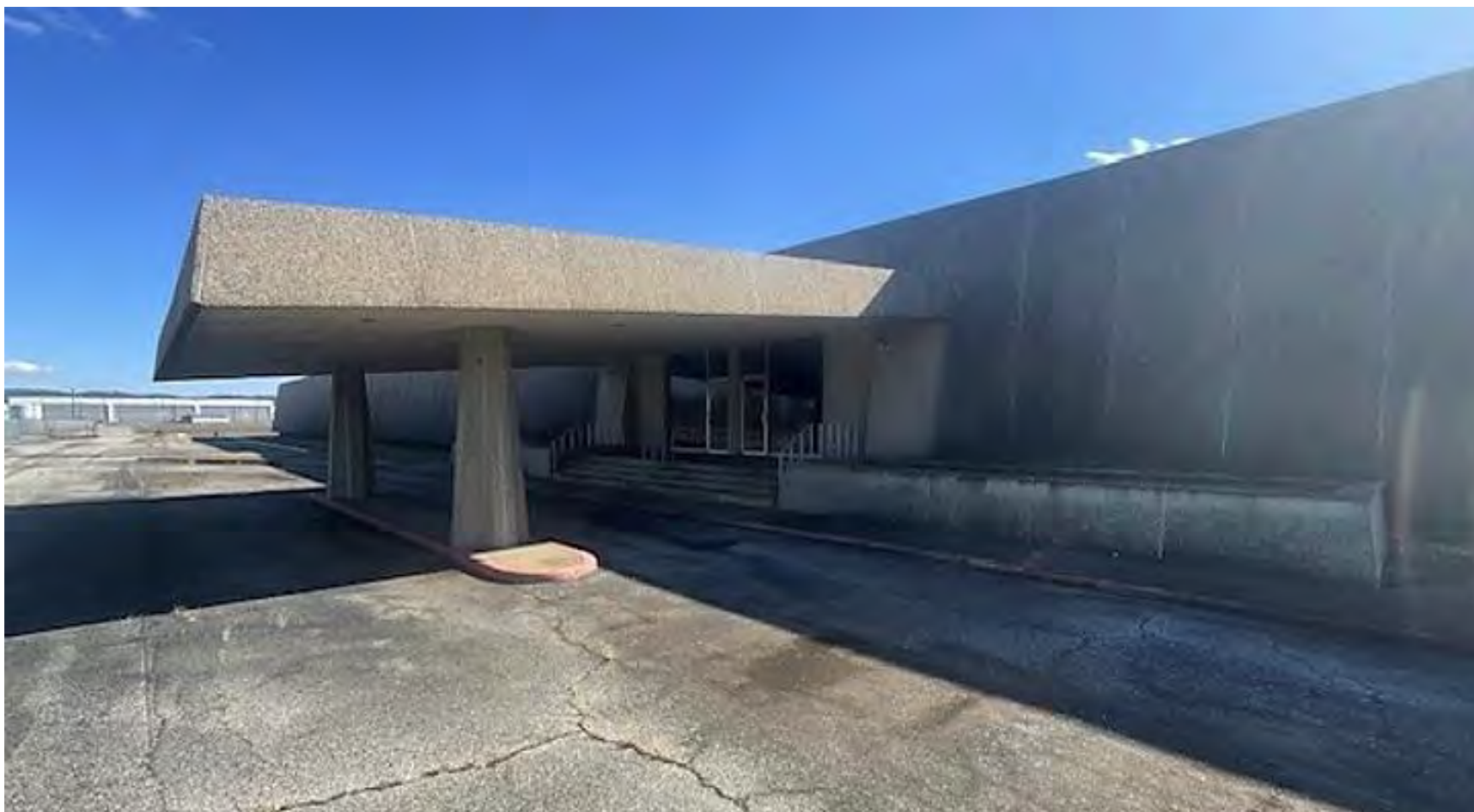
Photo 3. Building #201, front (north) facade entryway and carport, view facing southwest.
