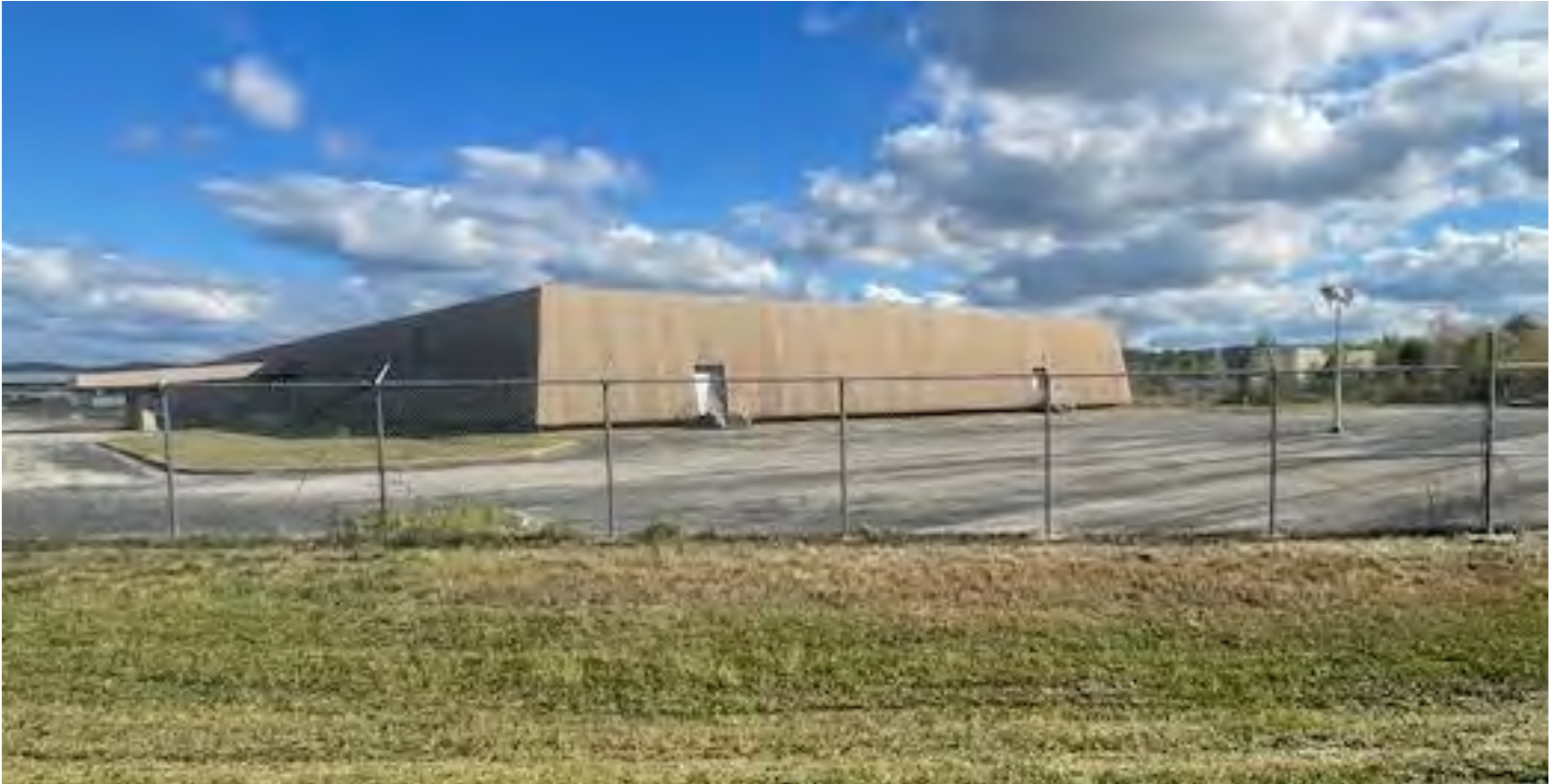
Photo 1. Building #201, oblique of front (north) facade and side (west) elevation, view facing southeast.
