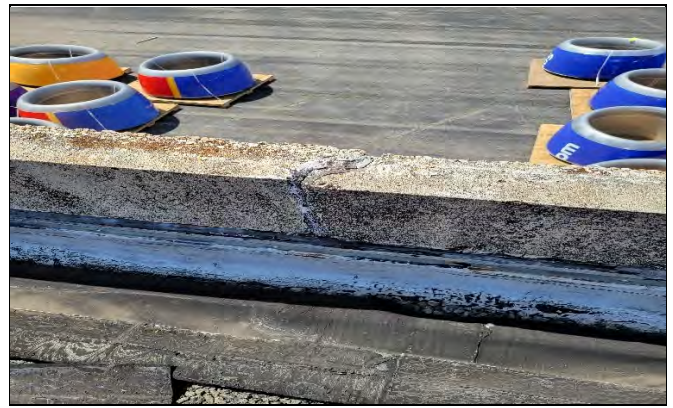
Asbestos Gray Felt Paper and Asbestos Black Mastic
