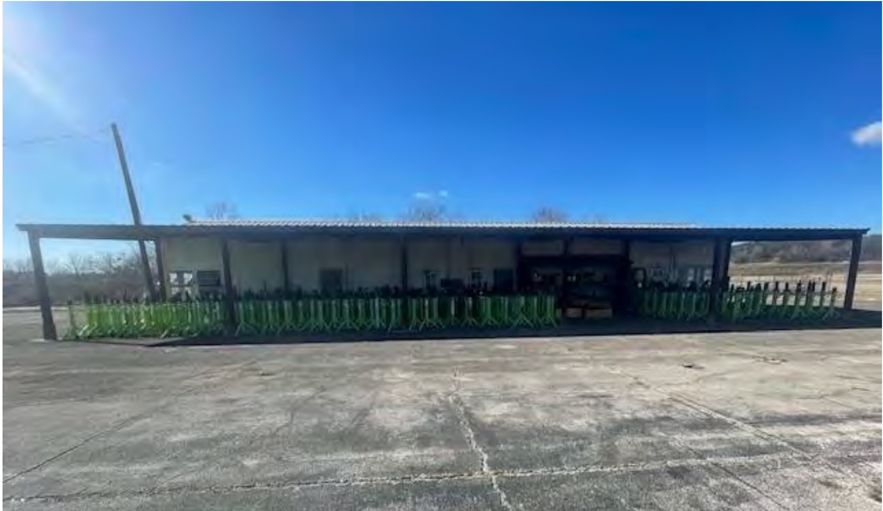
Photo 5. Storage shed, east elevation, view facing west.
