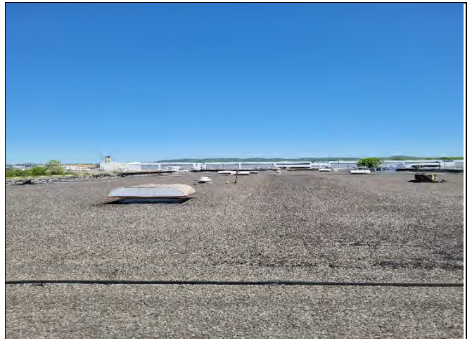
Roof View, East
