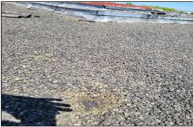
Non-Asbestos Main Roof, Asbestos Flashing and Silver Paint
