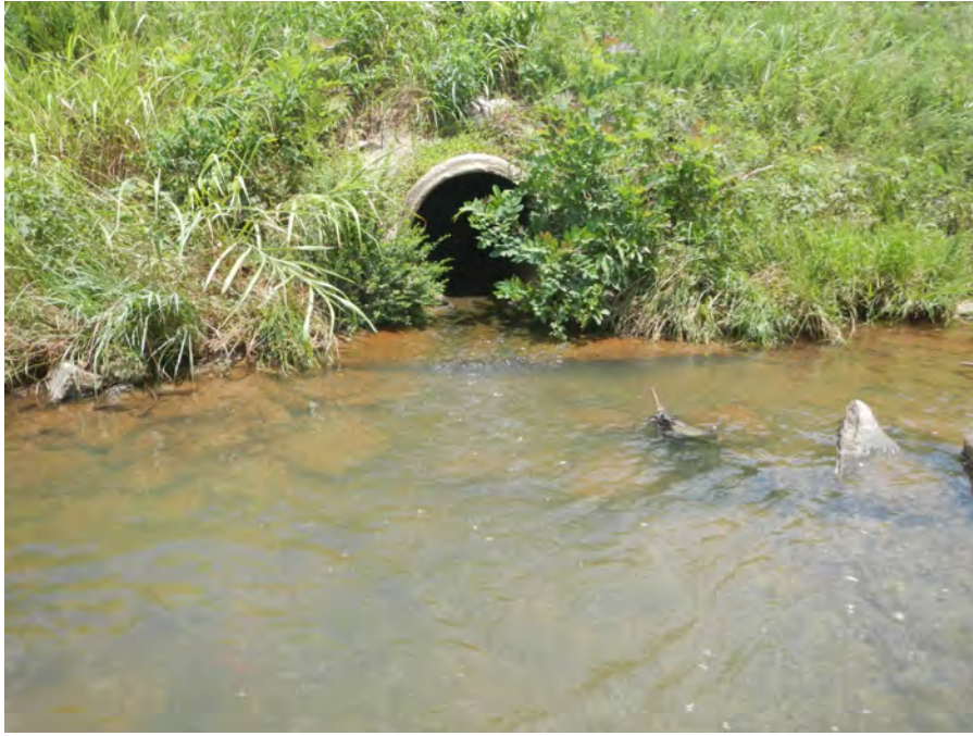
Culvert within Village Creek. Located near the middle portion of the survey reach. Taken by Jeff Selby, 6-18-2025.
