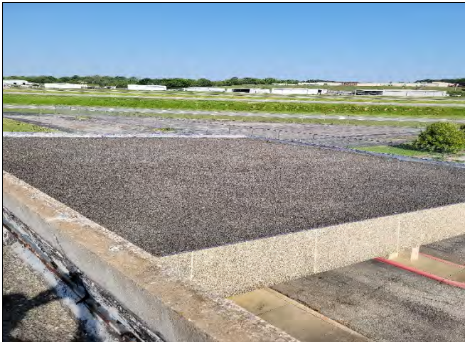
Roof View, North
