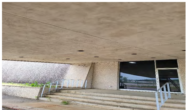
Exterior North View
